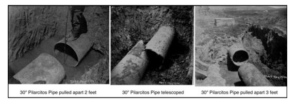
Figure 6. Damage to Pilarcitos Pipeline
