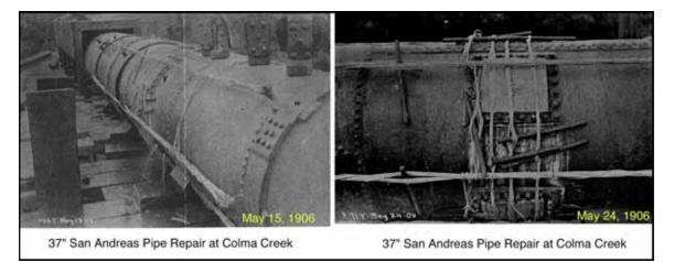
Figure 4. Damage to San Andreas Pipeline
