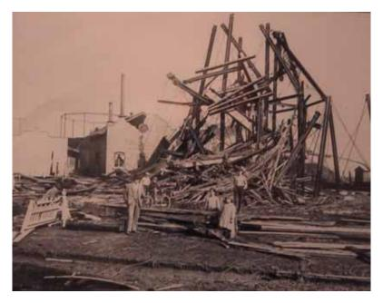
Figure 9. Collapsed Water Tanks in Santa Clara (c. April 1906)
