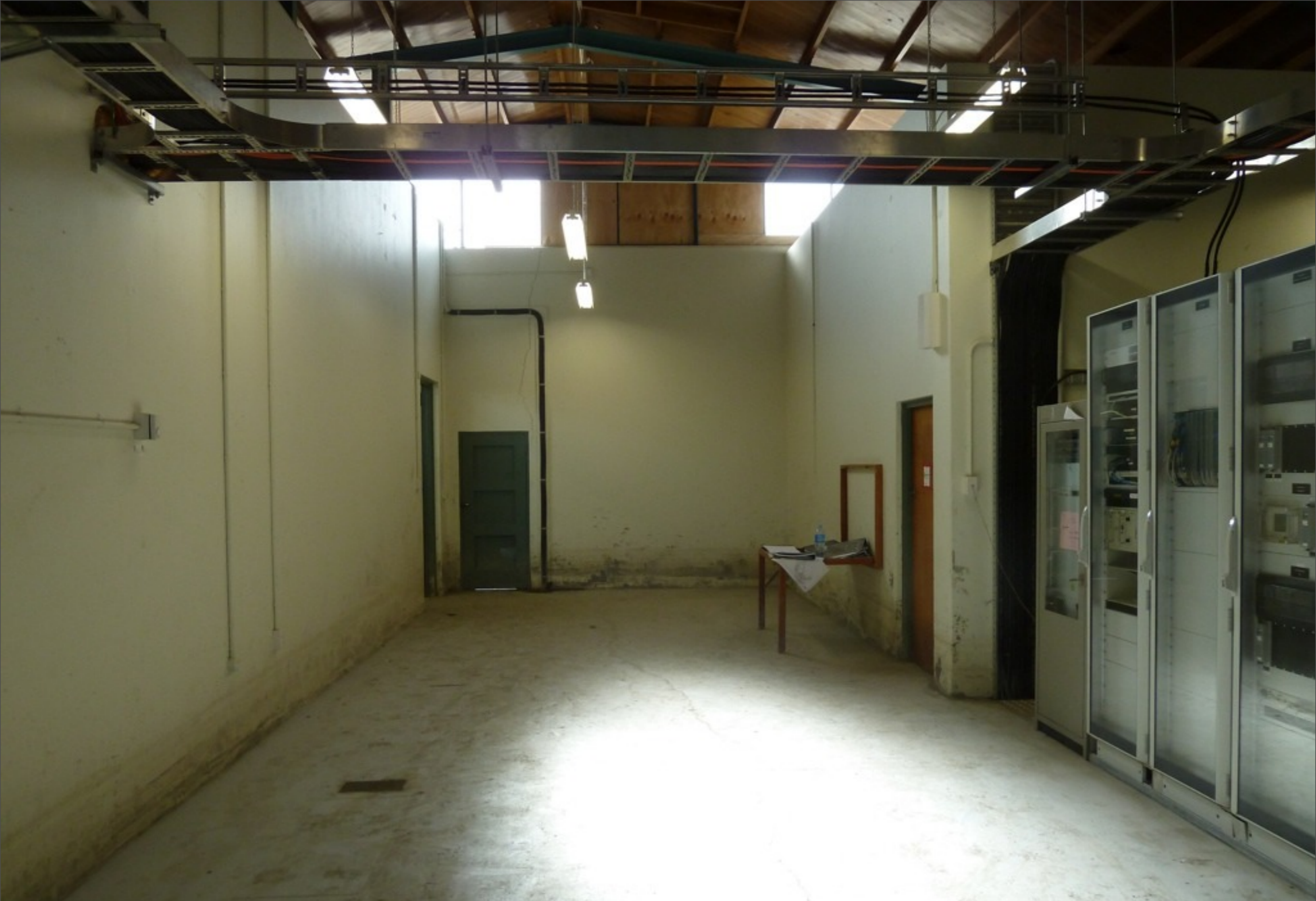
After removal of mud and replacement of damaged equipment
