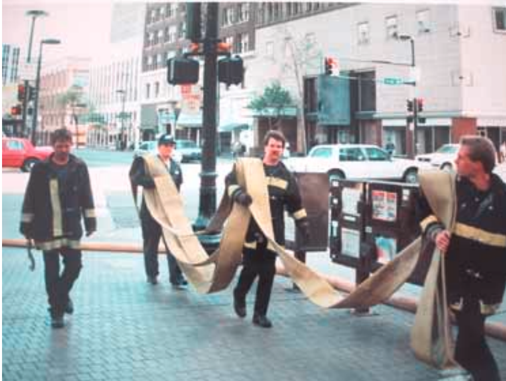
Figure 13-7. Deployment of Medium Diameter Flex Hose
