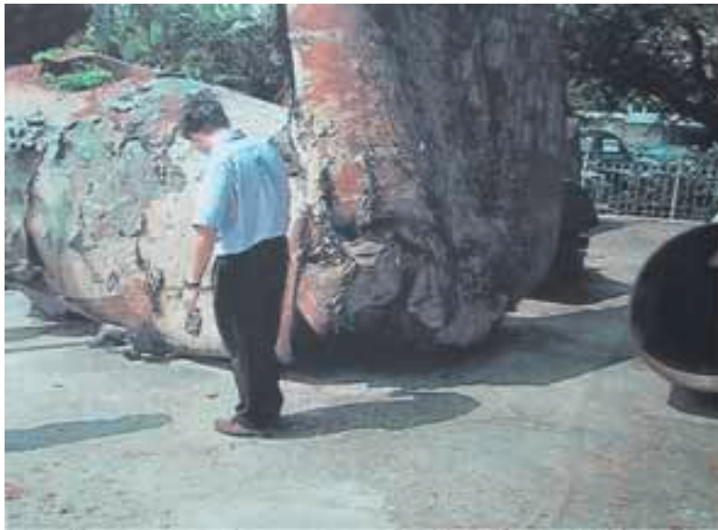
Figure 6-8. Damaged Steel Transmission Pipe, Chi-Chi Earthquake 1999
