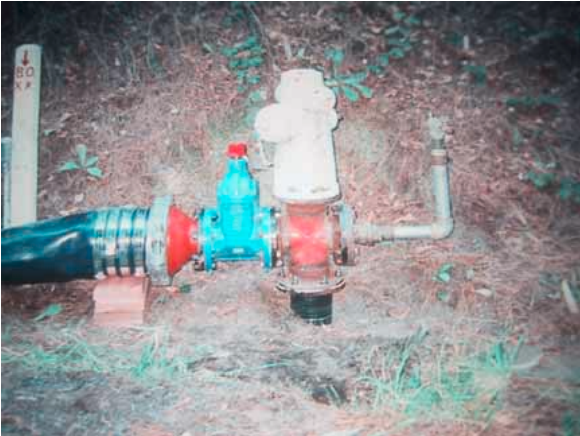
Figure 13-3. Flex Hose Attachment To Fire Hydrant
