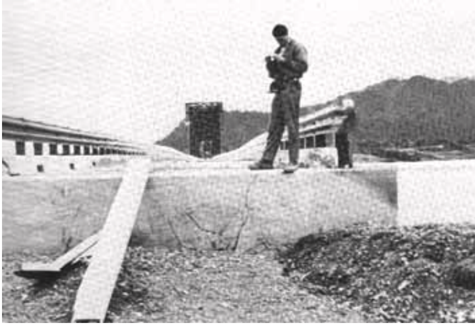
Figure 10-2 The Copper River Bridge #2 was closed after the 1964 Great Alaska earthquake due to approach settlement and shifted truss spans (NAS, 1973).
