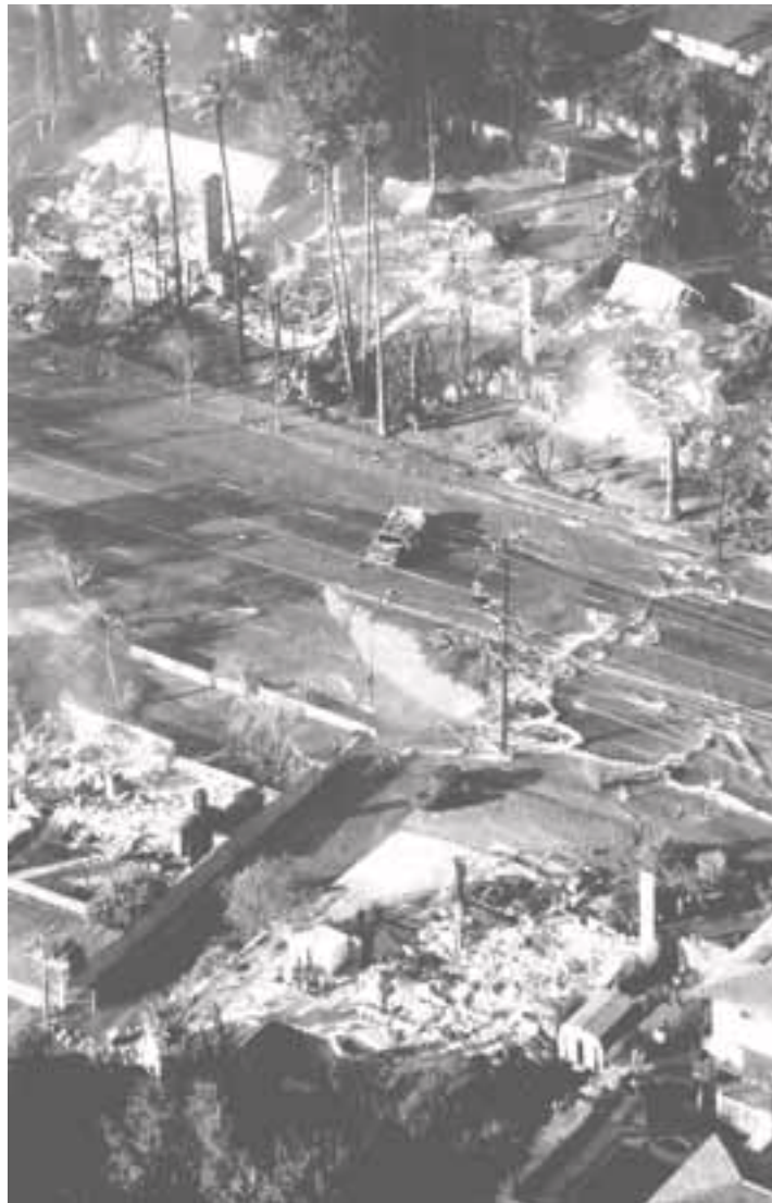
Figure 10-4 Ignition of gas line under Balboa Blvd (after the 1994 Northridge earthquake) resulted in several homes burning down (L.A. Times photo).
