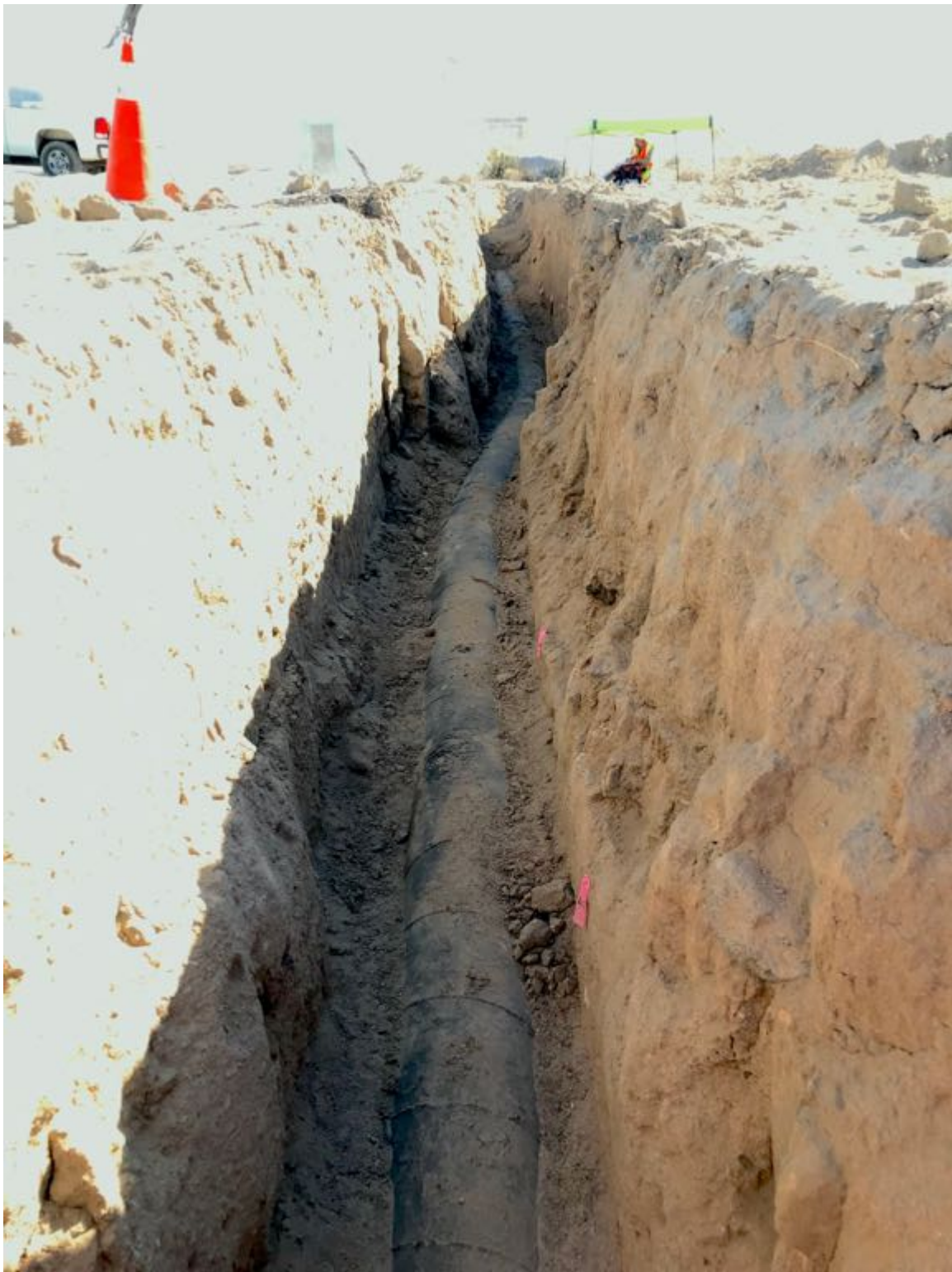
Figure 6.18-4. Line 311 after Trench and Pipe were Partially Exposed (Courtesy PG&E)
