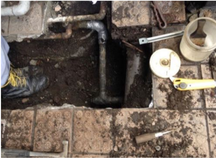
Figure 6.34-4. Repair to low pressure service lateral
