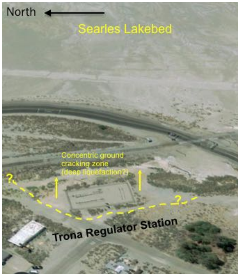
Figure 6.18-8. Trona Gas Regulator Station
