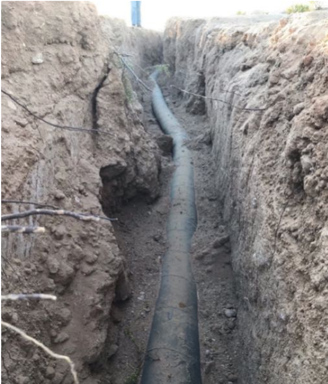
Figure 6.18-5. Line 372 after Trench and Pipe were Partially Exposed (Courtesy PG&E)
