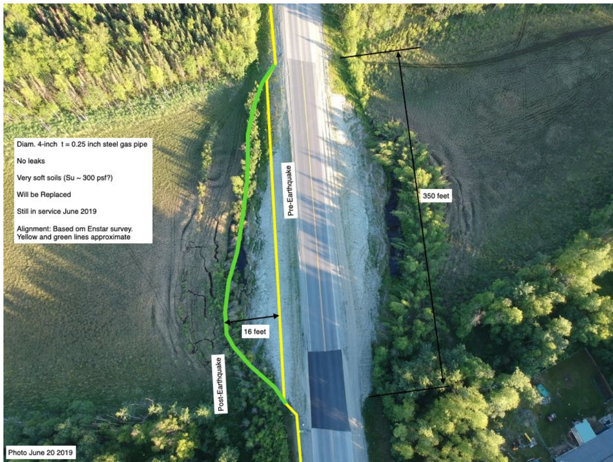
Figure 6.36-3. Gas Pipe Location (June 20 2019)
