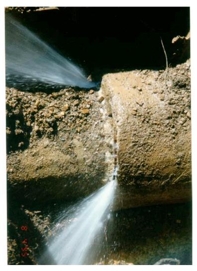
Figure 1. Leaking 30-inch diameter water pipe, damaged due to fault creep on the Hayward fault
