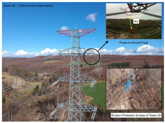
Fig. 8. Tower 29, Line Fault
