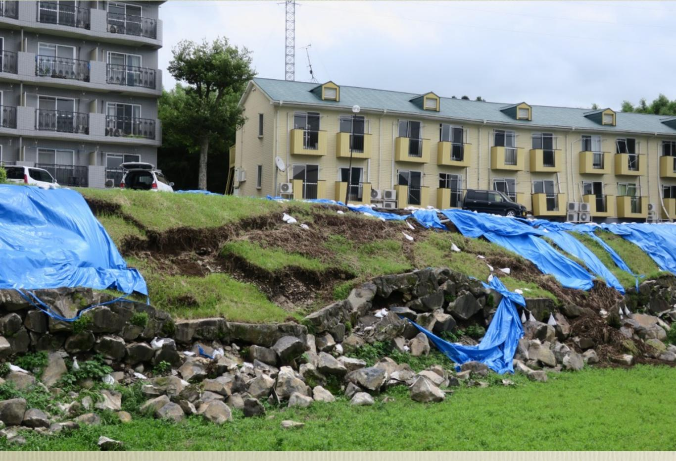
PGA -0.7g+. Embankment failure
