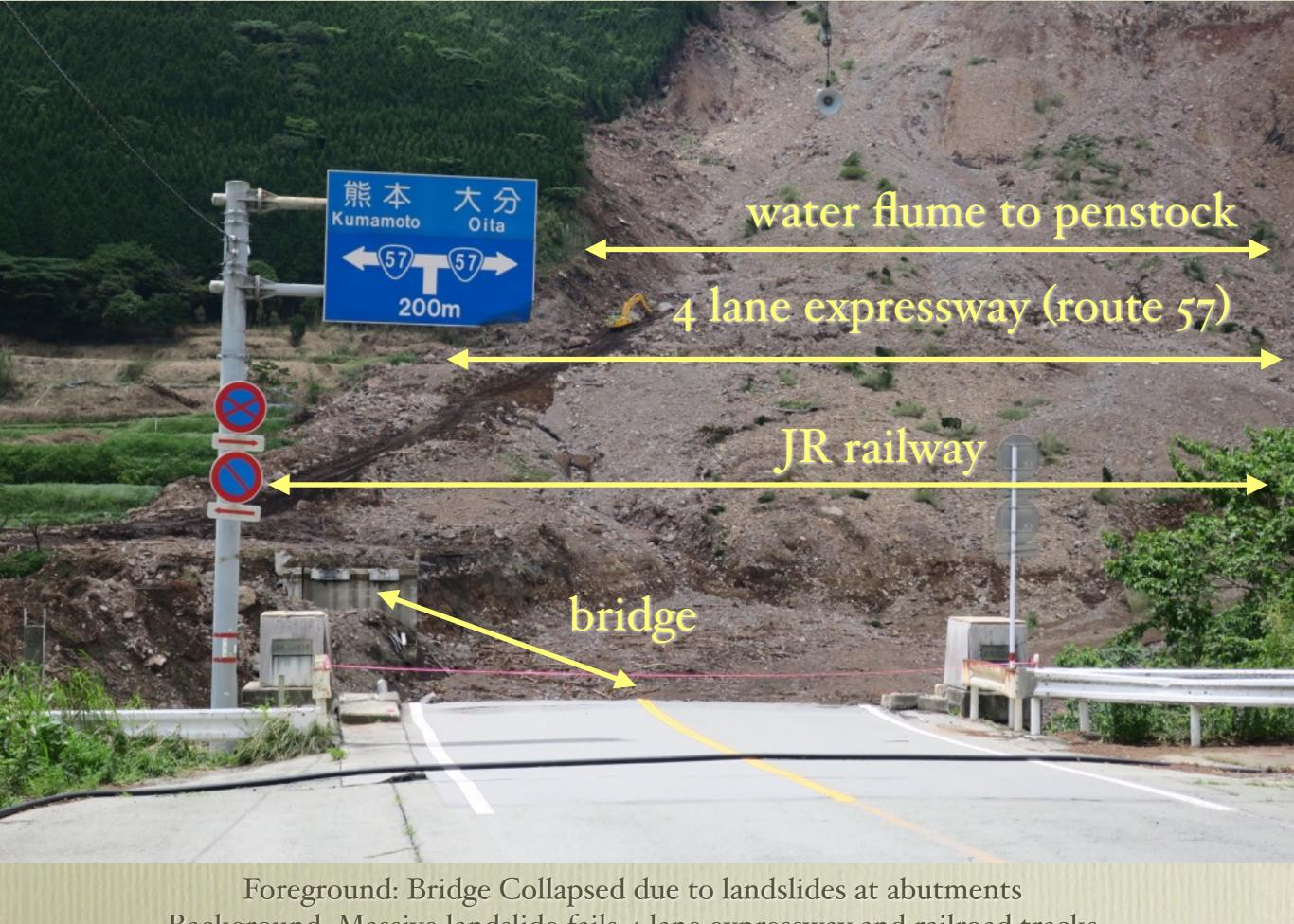
Background. Massive landslide fails 4 lane expressway and railroad tracks
