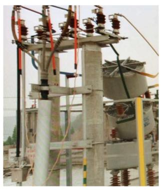
Figure 4-11. Damaged Air Core Reactors
