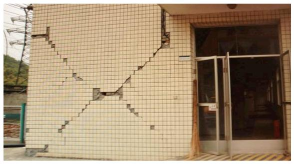
Figure 4-3. Damage to URM Control Building (Also houses low voltage feeder equipment)
