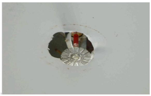
Figure 12-4. Sprinkler head moved sideways and impacted the suspended ceiling.
