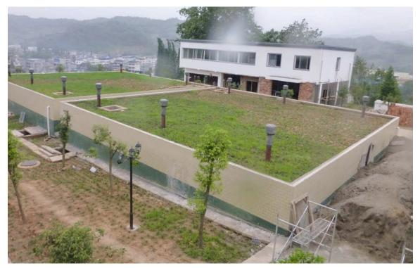
Figure 5-3. Two Partially Buried Clearwells
