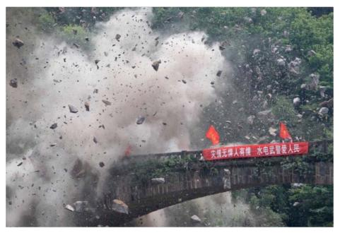
Figure 7-9. Blasting of large boulder to remove it from stone arch bridge
