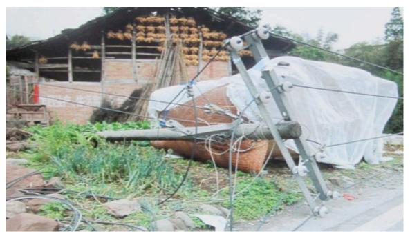
Figure 4-21. Damaged Power Pole
