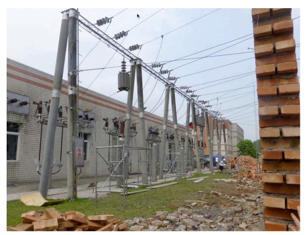
Figure 4-1. Damage to URM Wall, Cut Side. Some low voltage circuits were still not in service as of May 27 2013.
