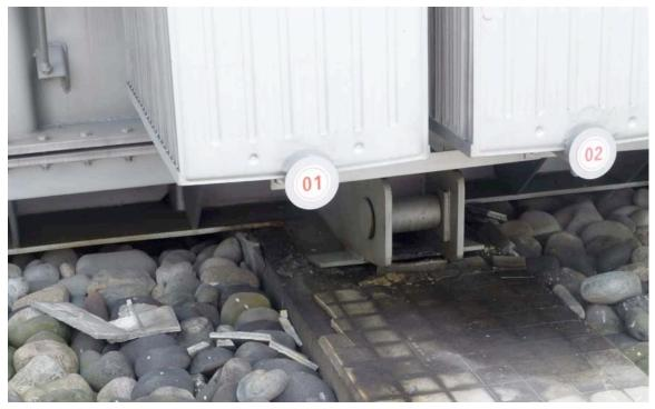
Figure 4-5. Bank 1 Transformer – Evidence of sliding (broken tiles over concrete foundation) and leakage of oil. The transformer was pushed back to its original position.
