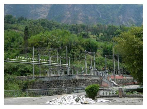
Figure 4-16 Dayanqiang ( $\mathbf{x} \neq \mathbf{k}$ ) 35kV substation with the power feed from the left.
