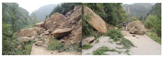
Figure 7-5. Lushan County roads damaged and blocked by falling rock debris
