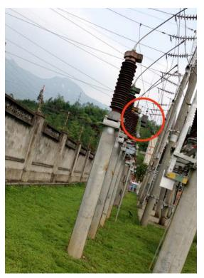
Figure 4-10. 110 kV Yard – After Repair – Wave Traps Highlighted in Red Circle
