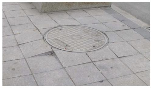
Figure 6-1. Floated Manhole
