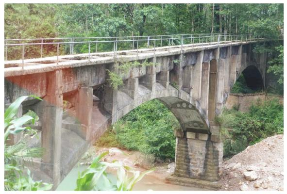
*Figure 4-25. Undamaged Water Flume over River (PGA ~0.35g)*
