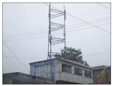
Figure 8-5. The cell tower at this site in Longmenxiang showed no damage, but the building showed large cracks on the side and front walls. Estimated PGA = 0.35g
