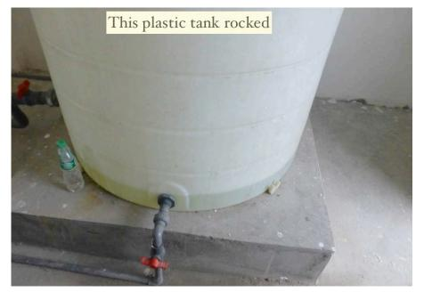
Figure 5-5. Plastic Tank for Chlorine Dioxide Disinfectant
