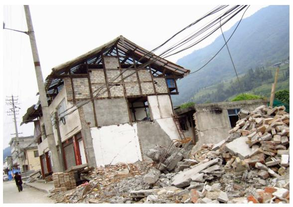
Figure 11-4. Construction Style of Common Buildings (PGA ~ 0.35g)
