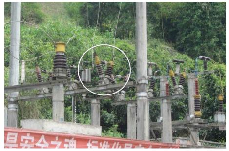
Figure 4-18 V-shape disconnect switch.
