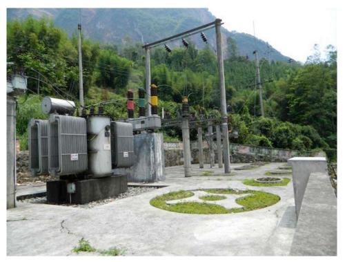
Figure 4-17 35kV transformer at Dayanqiang (大岩腔) 35kV substation
