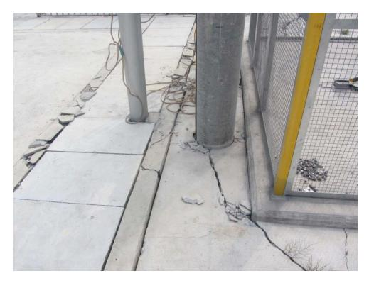
Figure 4-14. Cracks in the concrete pavement / cable trench due to the permanent ground movement
