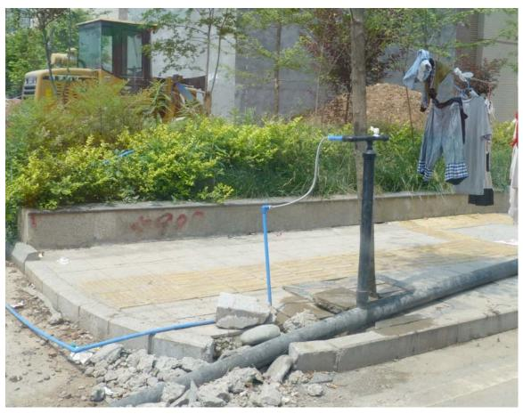
Figure 5-8. Above Ground Temporary Water Pipe
