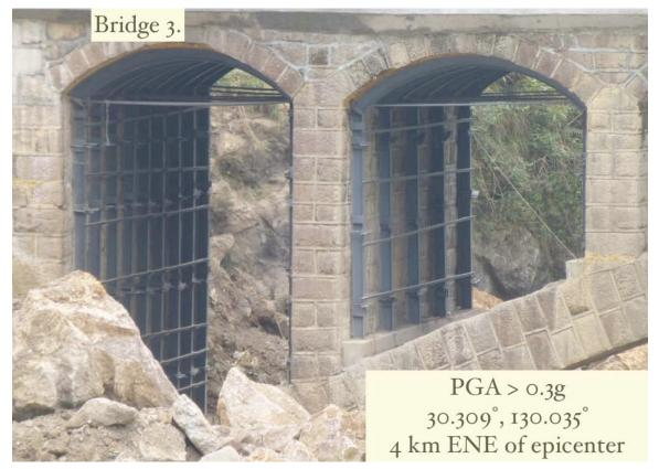
Figure 7-10. Steel Reinforcement Placed in Bridge 3 (May 31, 2013)
