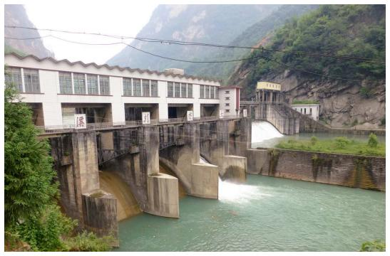
Figure 4-23. Undamaged Dam (PGA ~0.35g)
