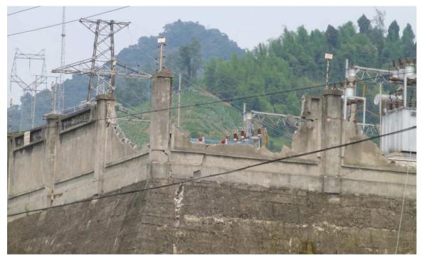
Figure 4-2. Damage to URM Wall, Fill Side
