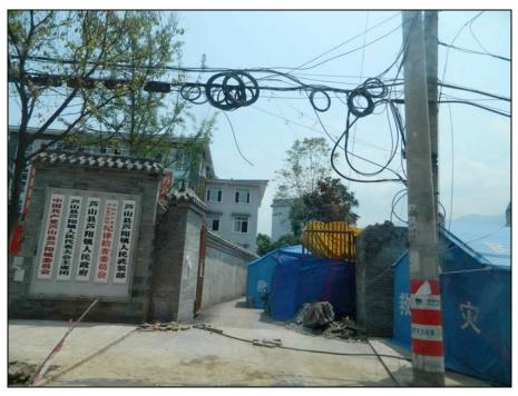
Figure 8-12. Example of poor cable management in Lushan
