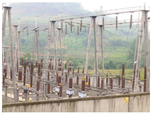
Figure 4-14. Undamaged 110 kV Yard at Substation 2
