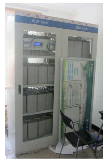
Figure 4-13. Sliding Batteries within Cabinets (uneven spaces between batteries due to sliding)
