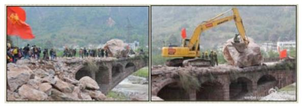
Figure 7-8. Damage to stone arch Bridge 3 in Lushan County, Blossom Sector Road from large boulders. Left Image: Large boulder rolls onto bridge, destroys masonry rails. Right image: excavator attempts to remove large boulder.
