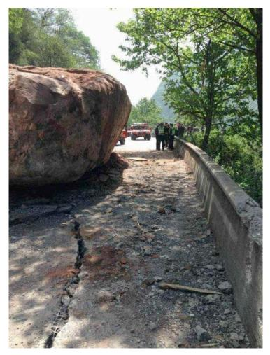
Figure 7-3. S210 damage on Feixianguan (飞仙关) Road by large boulders
