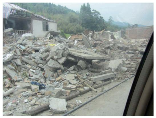
Figure 11-5. Severe Damage in Shuangshi Township (PGA ~ 0.5g).
