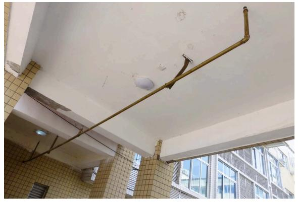
Figure 10-5. Damaged Sprinkler Pipe Support
