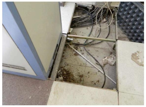
Figure 12-6. Raised Floor at Power Plant
