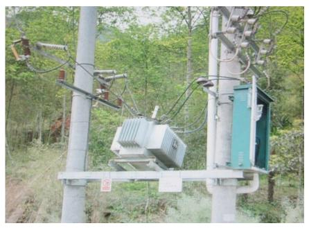
Figure 4-22. Damaged Platform-Mounted Transformer
