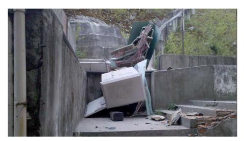
Figure 8-11. This cross connect cabinet in Tianquan (天全) town was destroyed by the rocks from above.
