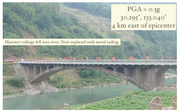
Figure 7-6. Damage to stone arch Bridge 1 in Lushan County (photo date May 31 2013)
