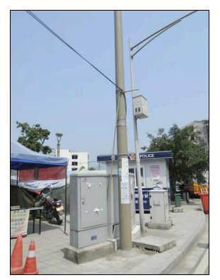
Figure 8-3. This fiber optic cable provided temporary connection to the hospital. All three telecommunication service providers placed their cabinets close to the power termination box (the small cabinet to the right).
