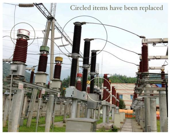
Figure 4-9. 110 kV Yard – After Repair
