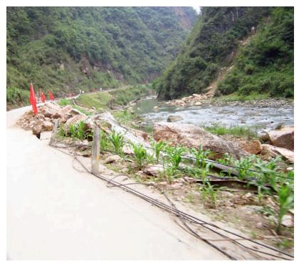
Figure 8-10. On the right side of the road, a bunch of fiber optic cables were placed on the ground without any protection. It is a temporary fix to provide connection to the network.
