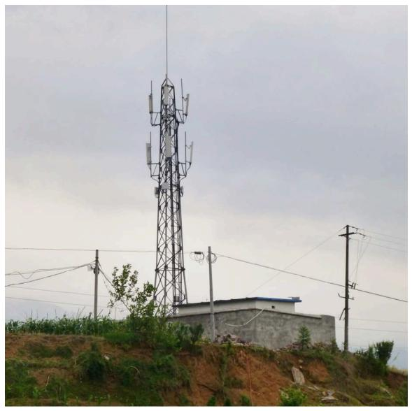
Figure 8-6. This cell cite did not show any sign of failure to the tower and to the building.
