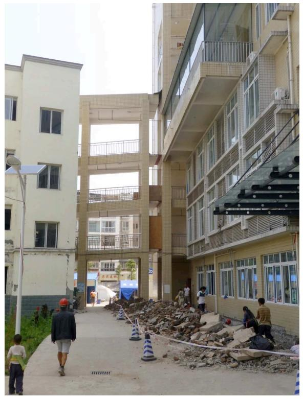
Figure 10-3. Base Isolated Hospital Building (on Right) with Walkway to Conventional Building (on Left)
