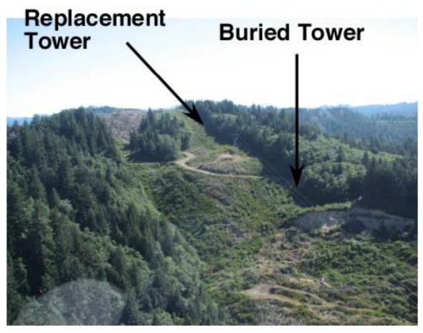
Figure 6. Transmission Tower Buried by Landslide
