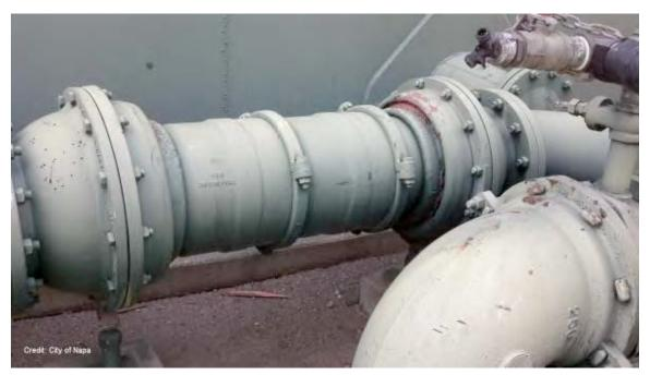
Figure 4-10. Movement of Attached Pipes
