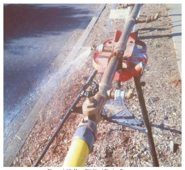
Figure 4-15. Hose Bib Used During Recovery
