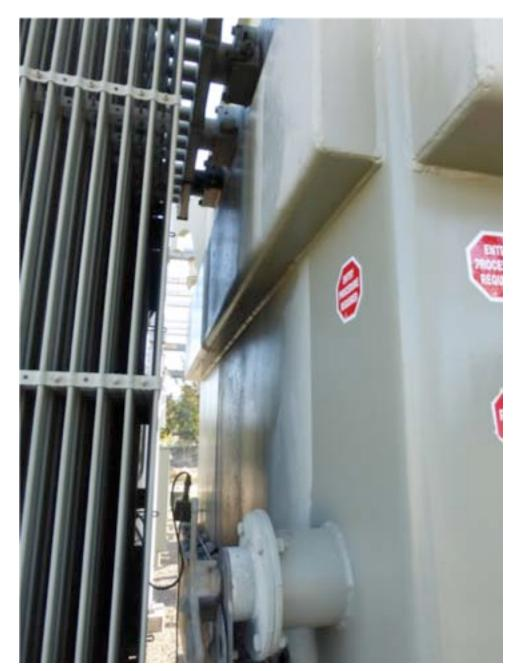
Figure 3-4. Transformer Oil Leak
