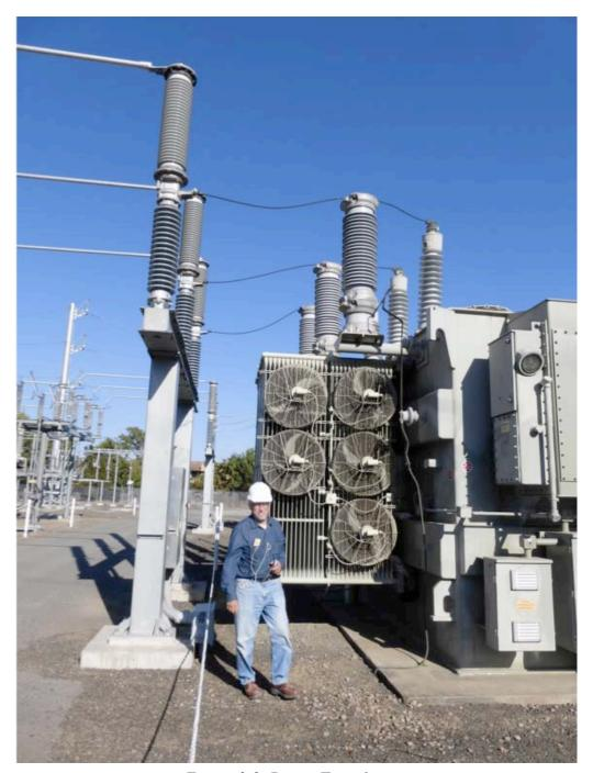
Figure 3-2. Power Transformer
