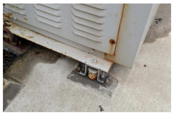
Figure 4-21. Spring-Mounted Motor Assembly
