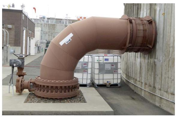
Figure 4-20. Steel Pipe with Dresser-Type Coupling
