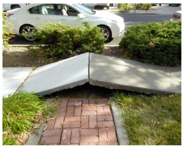
Figure 2-21. Buckled Sidewalk at Fault Offset Location
