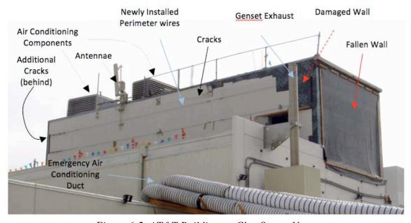
Figure 6-2. AT&T Building on Clay Street, Napa
