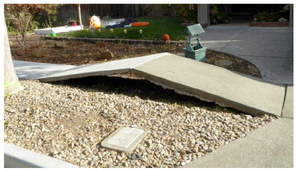
Figure 2-20. Buckled Sidewalk at Fault Offset Location
