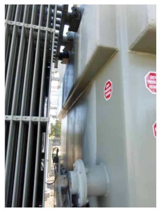
Figure 3-4. Transformer Oil Leak
