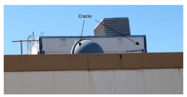
Figure 6-3. Additional cracks in the wall opposite to the one that fell
