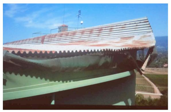
Figure 4-9. Damaged Roof of Steel Tank "B"
