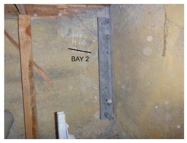
Figure 5-18. Restrainer damage at Hinge 10, Bay 2 of Napa River (W. Imola Ave) Bridge
