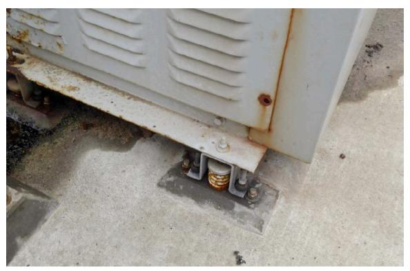
Figure 4-21. Spring-Mounted Motor Assembly
