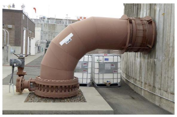
Figure 4-20. Steel Pipe with Dresser-Type Coupling
