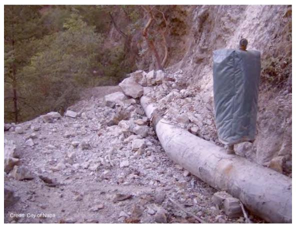
Figure 4-6. Damaged Transmission Pipe due to Rockfall
