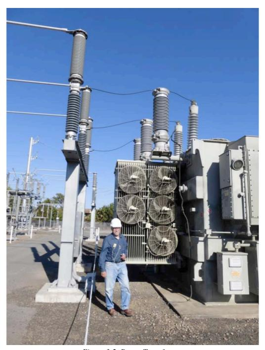
Figure 3-2. Power Transformer
