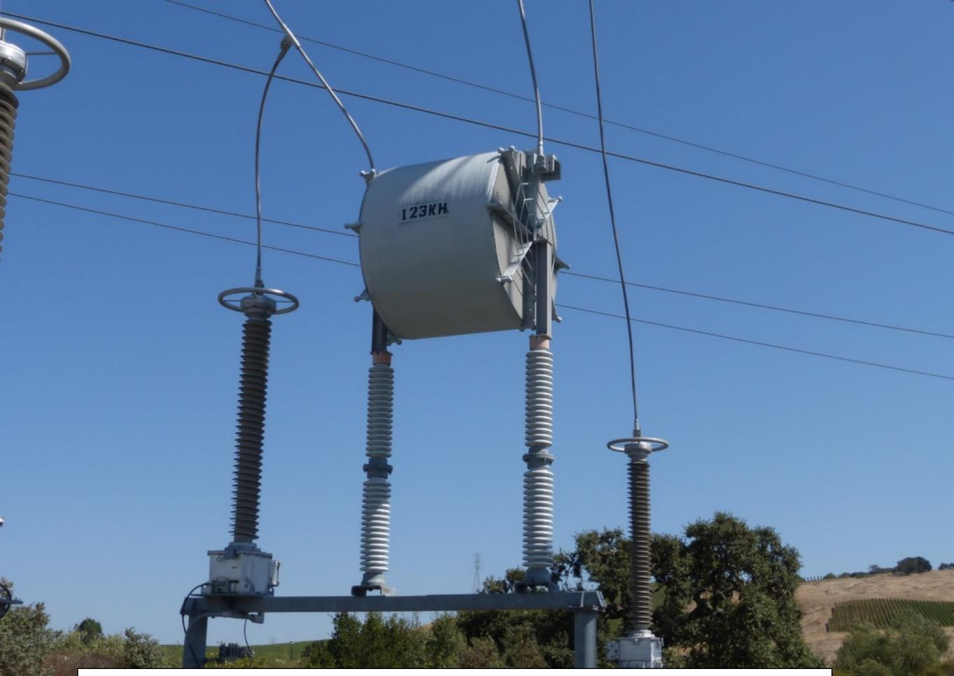
230 kV. Wave trap supported buy two post-insulators, on same stand with Trench CCVT (composite)
