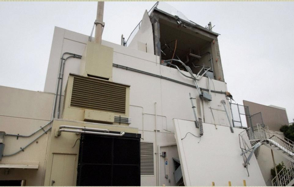
Wall Panel Fell. Was held by 4 tabs, for future expansion. Building racking damaged the tabs. Panel fell onto HVAC equipment, damaging cooling system.
