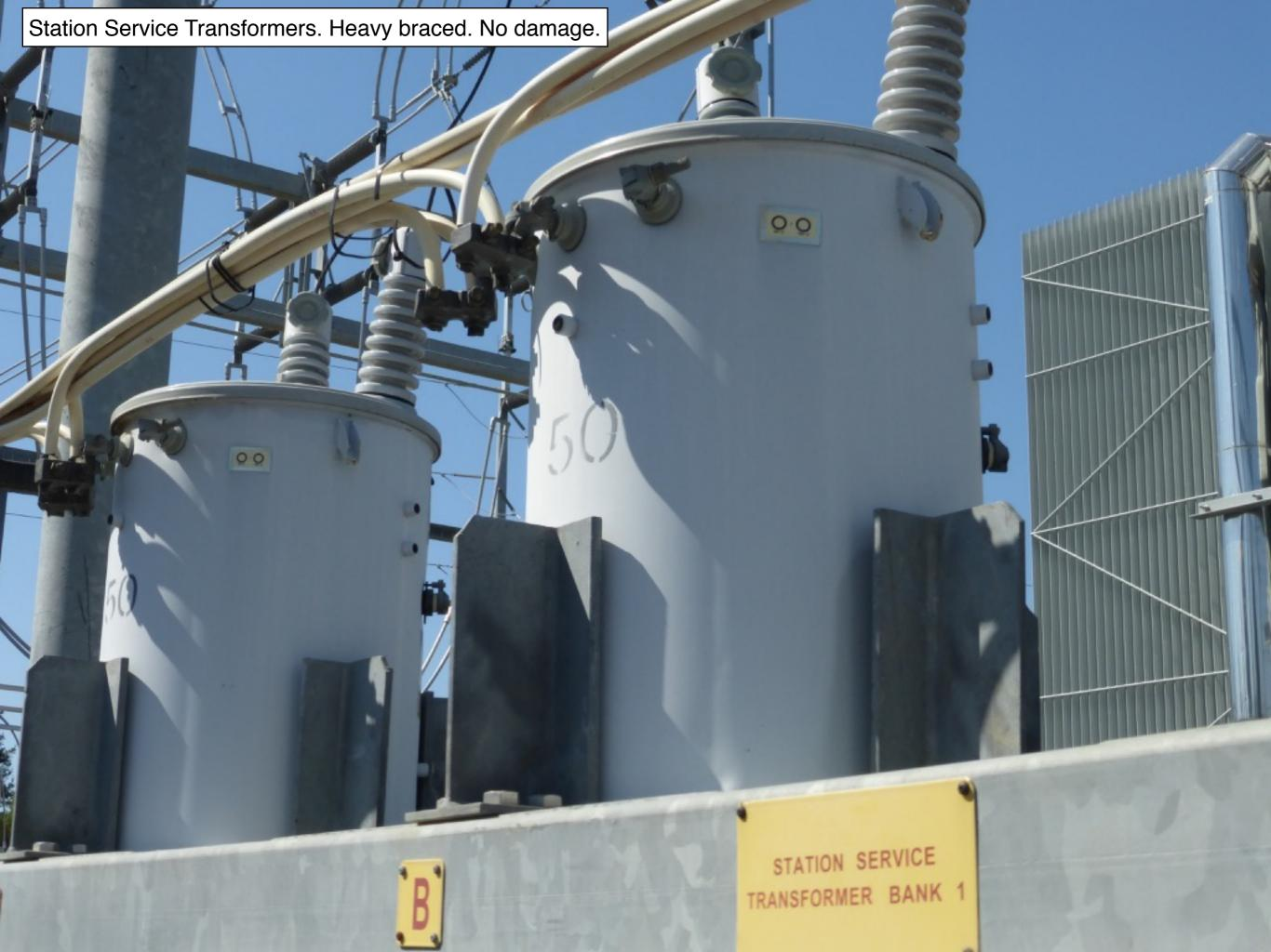
Vintage transformers. No damage at PGA ~0.30g. Well anchored. A new parallel transformer bank was installed so these are somewhat "Redundant" Upgrades of heavily loaded scaffolding might be a good thing.
