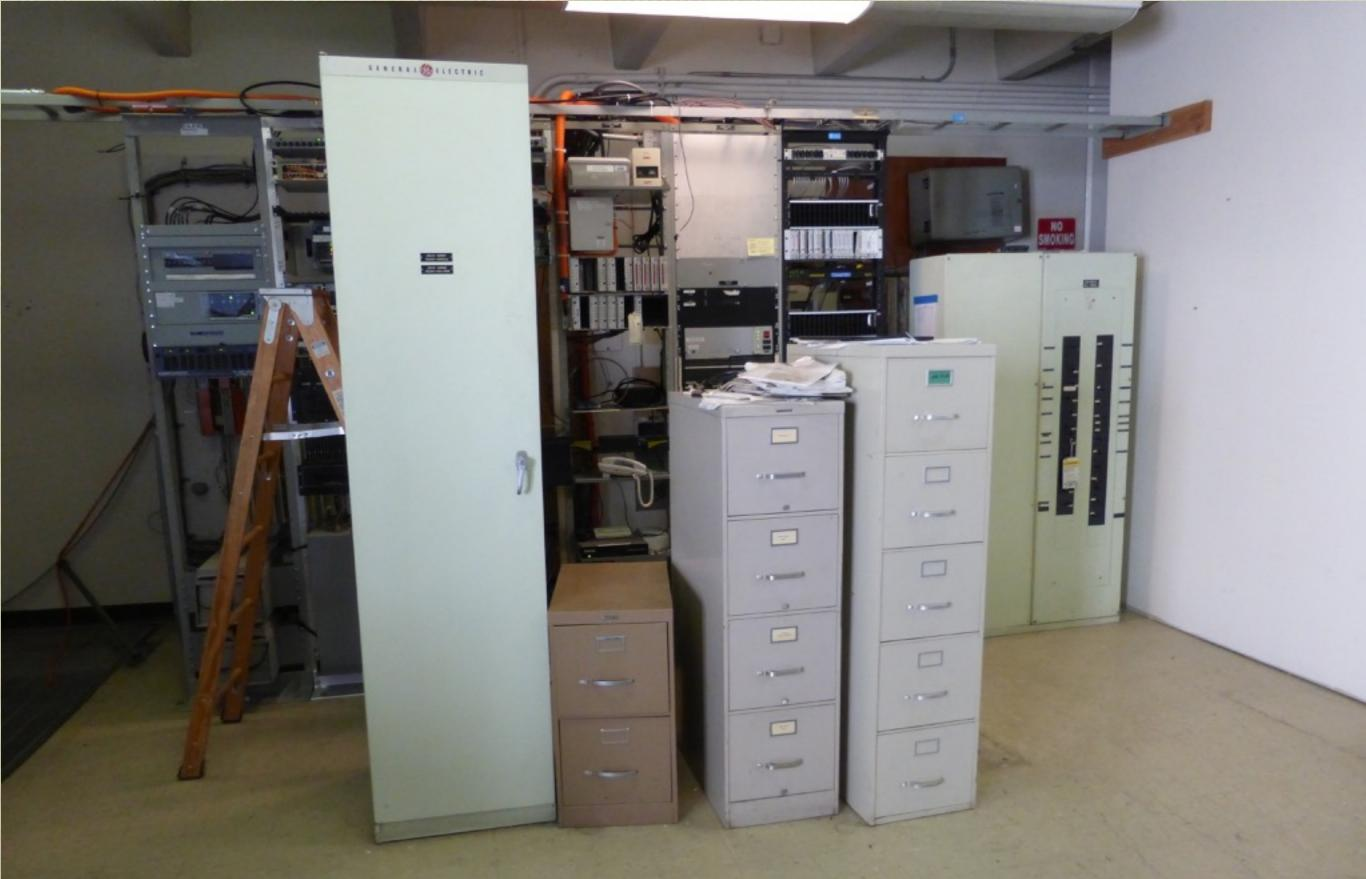
Unanchored Cabinets rocked to these positions (formerly cabinets were tight against each other). Mitigating this "housekeeping" weakness is an ongoing process.
