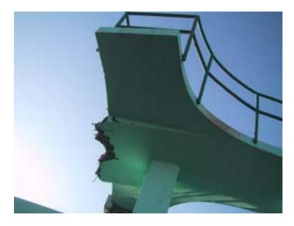
Figure 4-8. Damage to Reinforced Concrete Walkway
