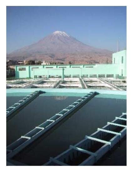
Figure 4-5. Metal Troughs – Out of Alignment (El Misti in background)
