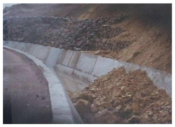
Figure 5-4. Landslide Debris into Canal Near Moquegua
