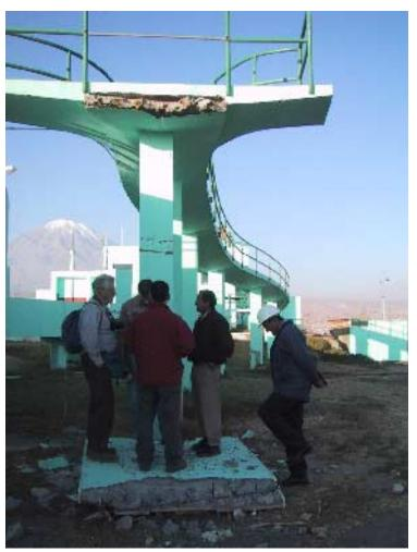
Figure 4-9. Damage to Reinforced Concrete Walkway
