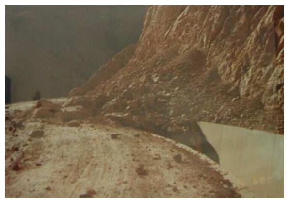
Figure 5-3. Landslide Debris into Canal Near Moquegua
