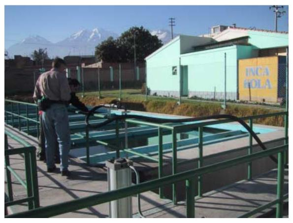
Figure 4-2. Arequipa WTP. No damage to concrete troughs, no sloshing over freeboard
