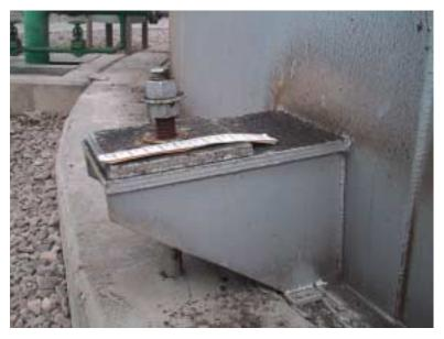
Figure 4-19. Stretched anchor bolt – 1,500,000 tank near Ilo
