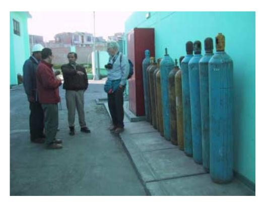
Figure 4-3. Arequipa WTP. Small Chlorine Tanks
