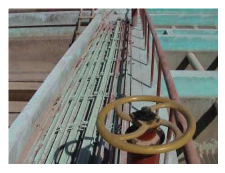
Figure 4-13. Baffle Support Channels – Removed from Service, Moquegau WTP
