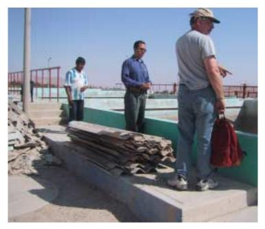
Figure 4-12. Broken Baffles, Moquegua WTP
