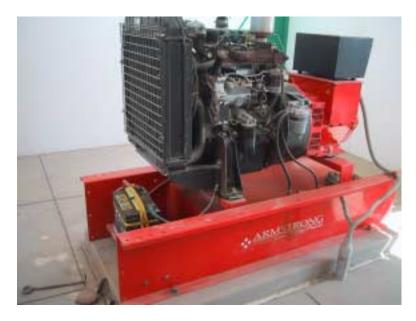
Figure 4-16. Emergency Generator – Moquegua WTP
