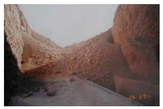
Figure 5-2. Landslide Debris into Canal Near Moquegua
