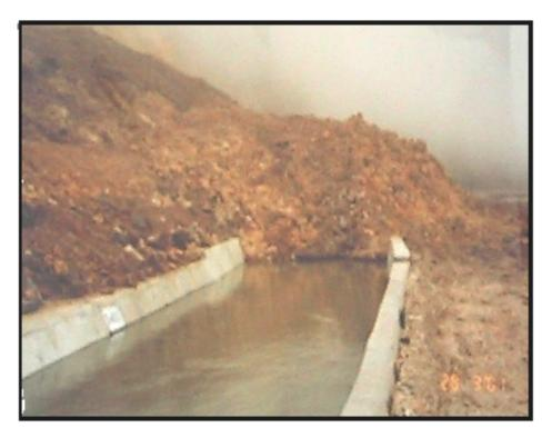
Figure 5-1. Landslide Debris in Canal Near Moquegua
