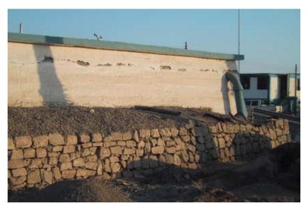
Figure 4-17. Tacna WTP – Damage to Walls of Reinforced Concrete Clearwell
