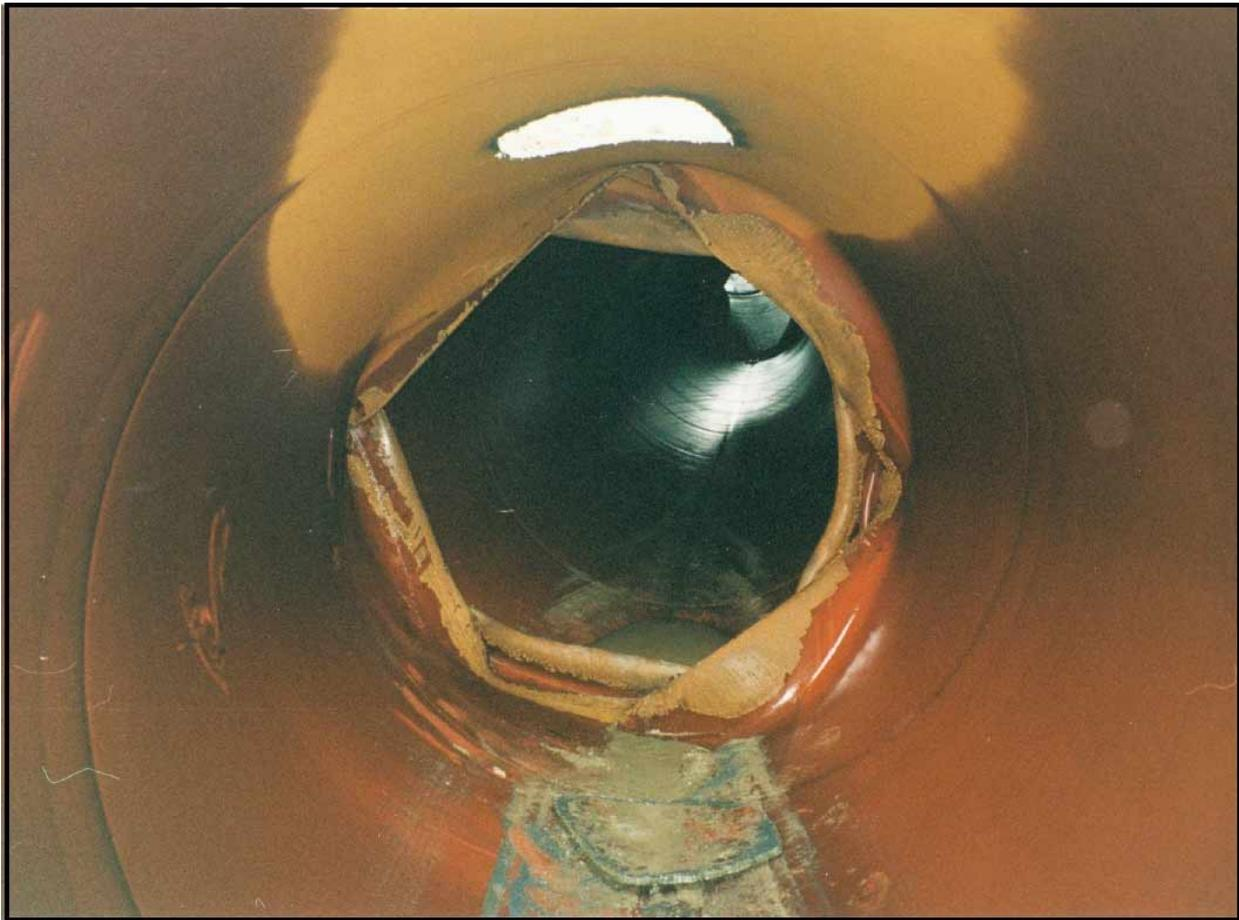
Figure 2. Major Wrinkle. Note Steel Plate at Invert from Manhole
