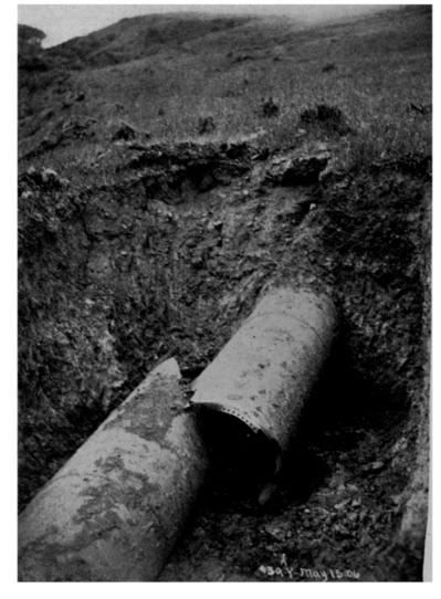
6. 30" Pilarcitos Pipe telescoped
