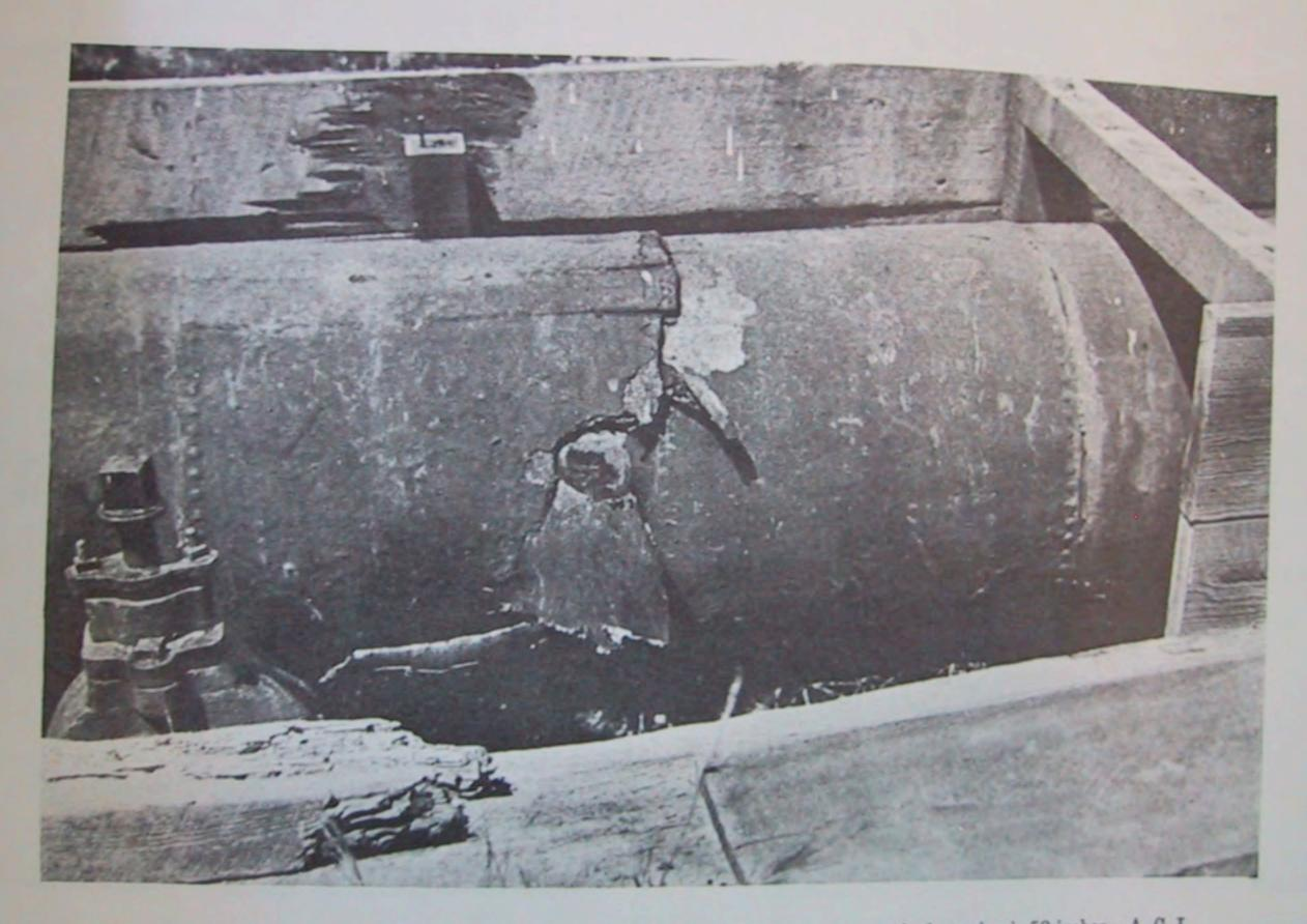
B. Thrust of 30-inch water-pipe by fault, northwest of San Andreas Lake. Amount of telescoping is 58 inches. A. C. L.
