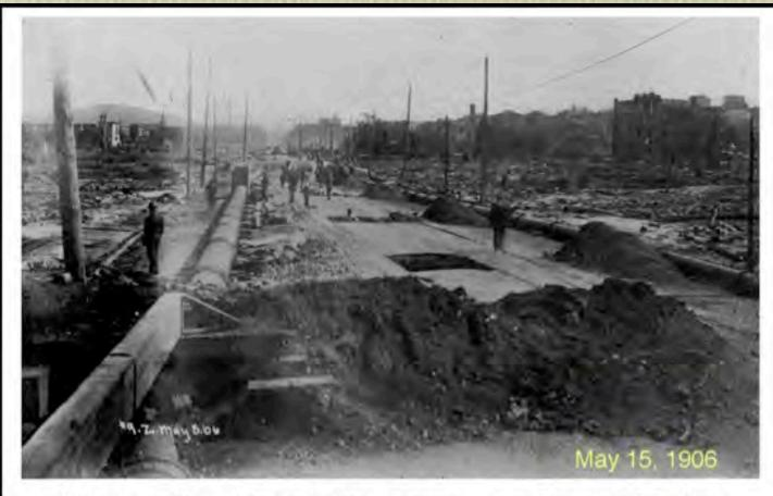
58. View south on Valencia Street showing new 24" and 16" pipes on top of pavement of sunken street
