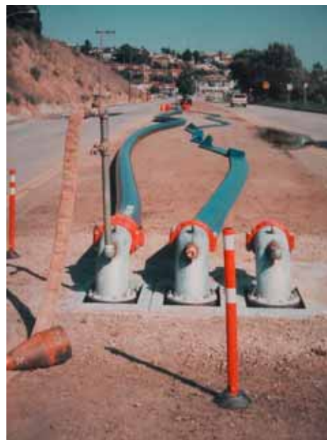
Figure 9-3. Flex Hose Attached to Manifold Outlets
