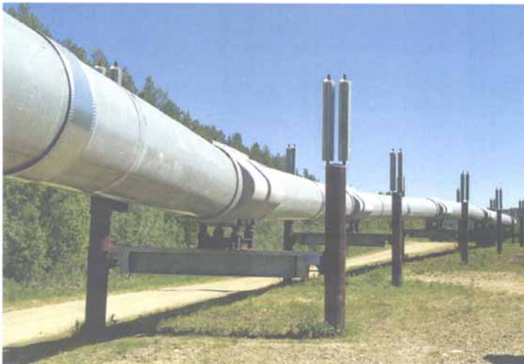
Figure 8-13. Alyeska Oil Pipeline (Elevated Section, Not at a Fault Crossing)
