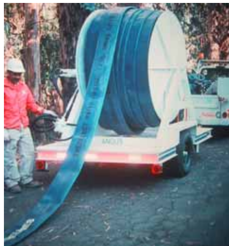
Figure 9-5. Deployment Using Hose Reel
