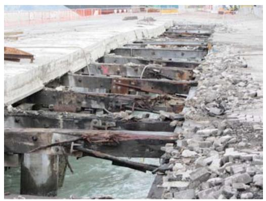
Figure 9-13. Damaged piles and beams at berth CQ2 (looking west).
