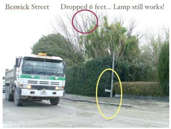
Figure 4-57. Electrified Lamp – September 4 2010 – 1.8 meter movement
