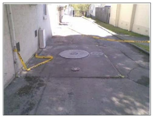
Figure 5-7. The manhole outside Halswell Exchange was also raised due to liquefaction (Courtesy of Telecom New Zealand)
