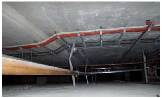
Figure 17-17. Damaged Vertical Struts, February 2011
