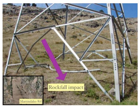
Figure 4-32. Damaged 66 kV Transmission Tower
