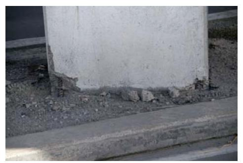
Figure 11-24. Flexural crack and buckling of rebar in column of Port Hills Road Overbridge
