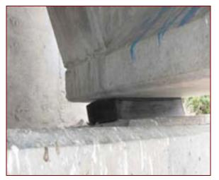
Figure 11-2. Rubber bearing deformed
