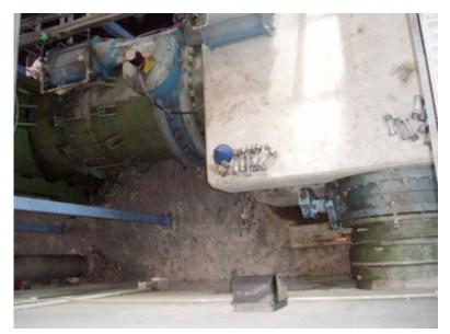
Figure 7-46. Pumping Station B leak at mechanical coupling, Bromley WWTP
