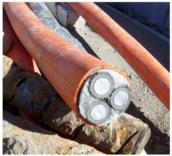
Figure 4-55. Cross Section of 11 kV Buried Cable
