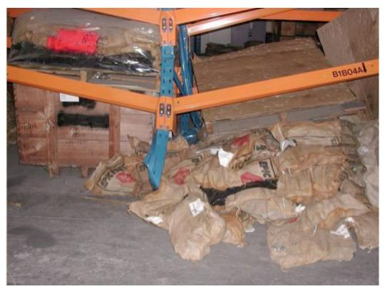
Figure 17-2. Damaged Column Leg, Addington Warehouse
