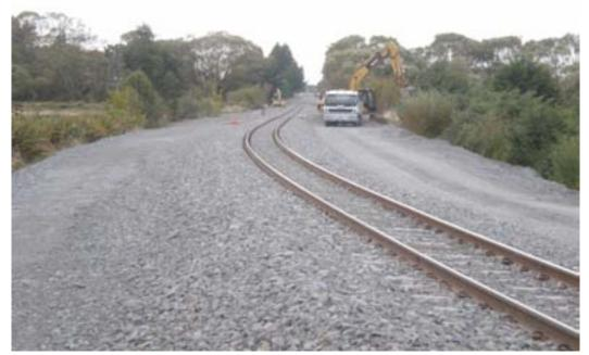
Figure 12-18. Re-ballasting the Main North Line (also, compare with Figures 12-14, 12-15)
