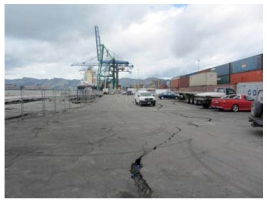
Figure 9-11. Ground cracks at berth CQ2 (looking west).
