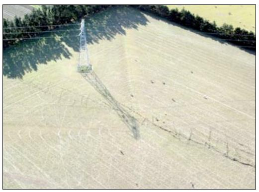
Figure 4-4. Surface Fault Offset Approaches the Tower in Figures 4-3, 4-5
