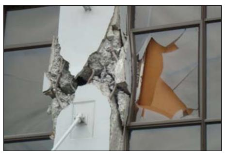
Figure 5-25. TVNZ Building - close up of one of the columns damaged.
