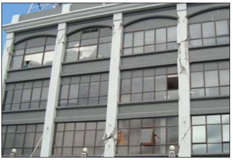
Figure 5-24. The front columns of the building sustained significant damage.
