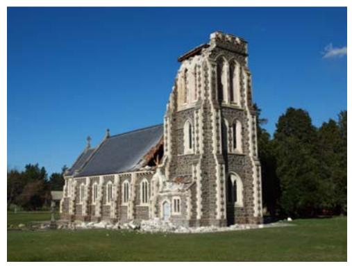
Figure 16-2. Damage (Parapets, Falling Debris Damaged Roof) to URM Church
