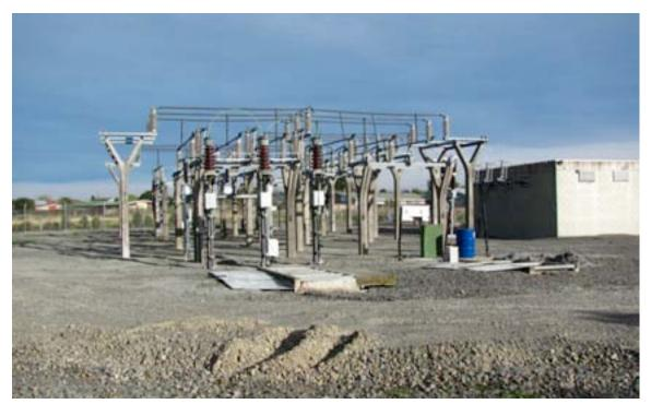
Figure 4-44. Pages Substation endings for the two 66 kV lines to New Brighton Substation.
