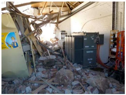
Figure 4-37. Damaged Switchgear Within Avalanche-Impacted Substation
