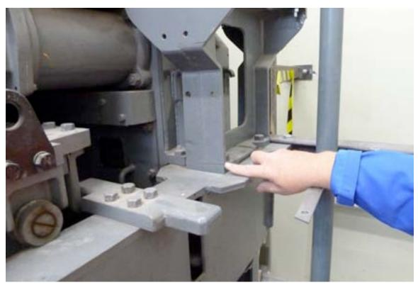
Figure 4-26. Cracked Steel Frame for Circuit Breaker 37, Bromley Substation
