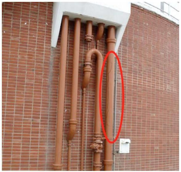
Figure 7-41 shows a cracked pipe leading to one of the digesters. There was no leak, as the pipe has an internal liner (and the digester was out of service).
