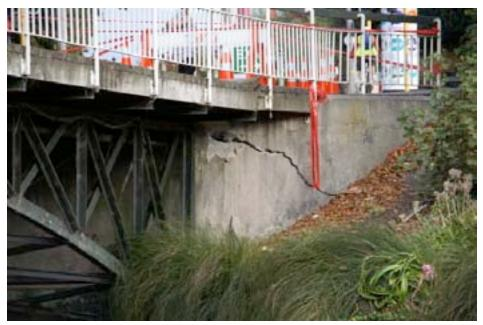
Figure 11-14. Abutment failure of Boathouse Bridge.
