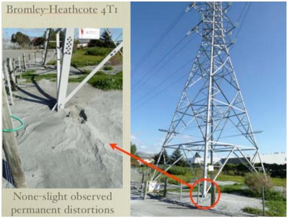
Figure 4-34. Liquefaction at 66 kV Transmission Tower
