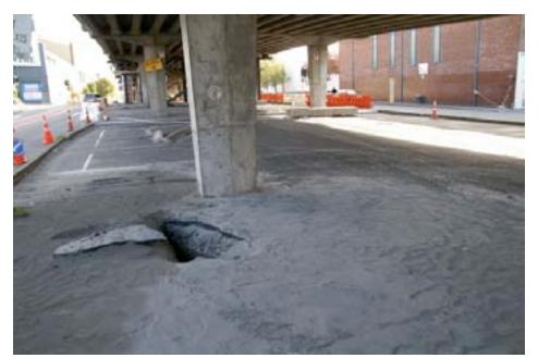
Figure 11-12. Liquefaction .of foundation soil at Moorhouse Ave Bridge at Colombo St.
