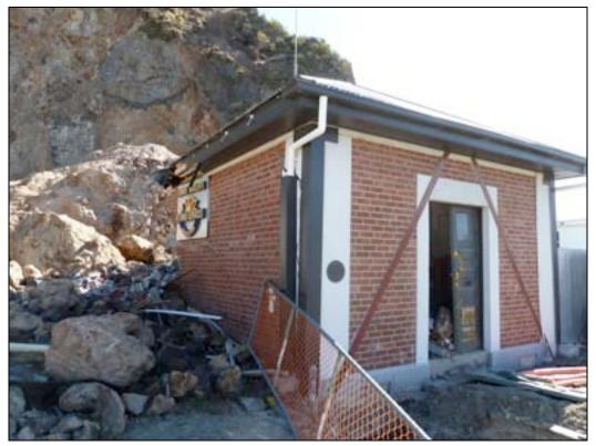
Figure 4-36. Substation Impacted by Rock Fall (Sumner Redcliffs Area) Feb 22 2011
