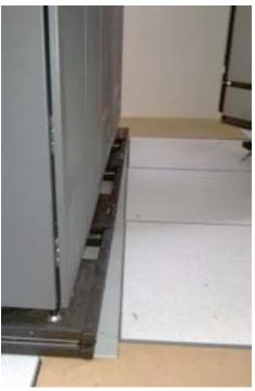
Figure 17-6. Triple Base Isolation Units – Slid 50 mm, Lost 3 of 18 Balls
