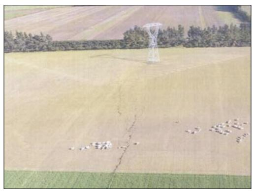
Figure 4-3. Surface Fault Offset Approaches the Tower in Figures 4-4, 4-5
