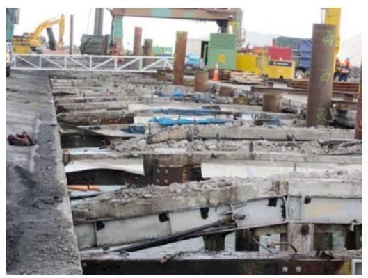
Figure 9-15. Damaged piles and beams at berth CQ1 (looking east).
