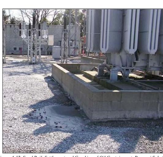
Figure 4-12. Sand Boil, Settlement and Cracking of Oil Containment, Papanui Substation
