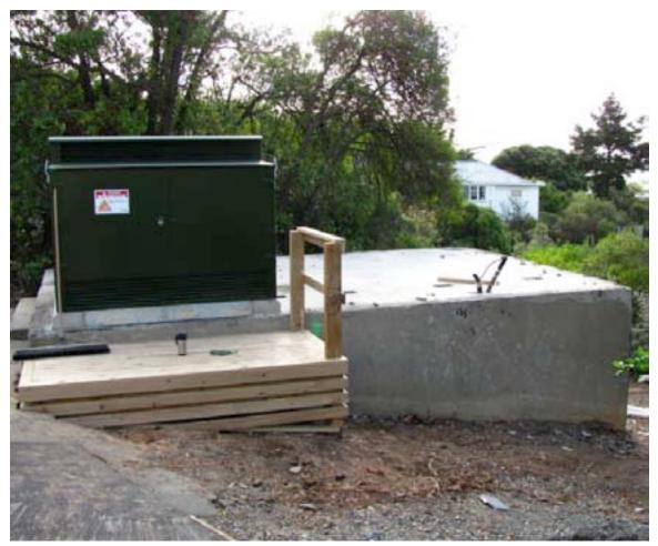
Figure 4-49. The pad-mounted transformer that replaced the one inside the substation in Figure 4-47.
