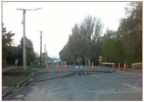
Figure 11-1. Road surface up heaving due to permanent ground deformation
