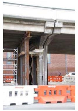
Figure 11-11a. Column bent with expansion joint
