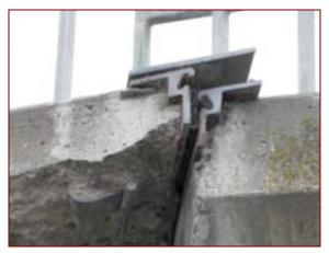
Figure 11-3. Deck and abutment impact damage
