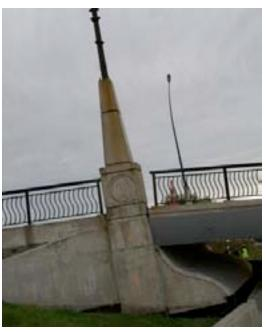
Figure 11-19. Rotation of left abutment of Anzac Drive Bridge (February 2011)
