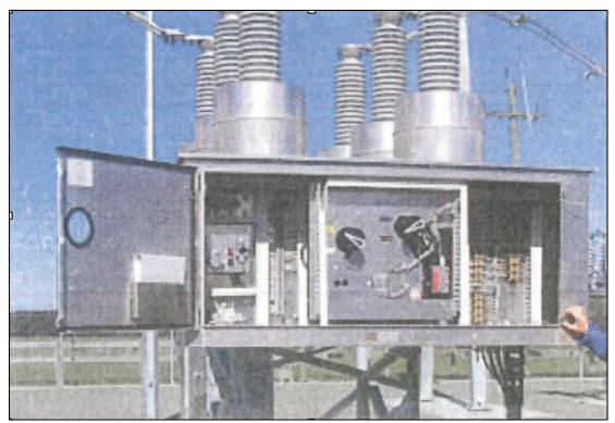
Figure 4-9. One of Two Cabinet Doors Broke Off, SF6 Circuit Breaker
