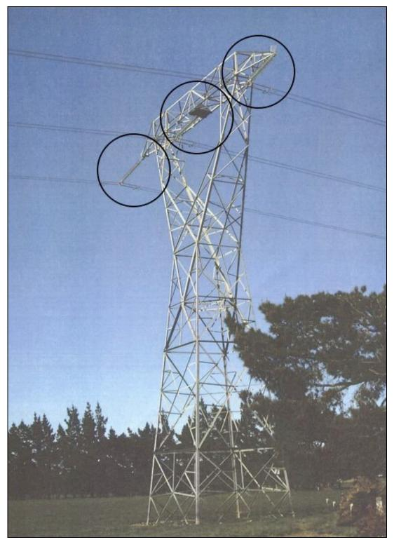
Figure 4-5. Displaced Insulators on Suspension Tower Adjacent to Fault Offset
