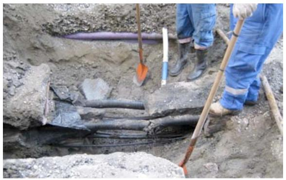
Figure 4-51. Failure of Two 66 kV Buried Oil-Filled Cables, Feb 22 2011
