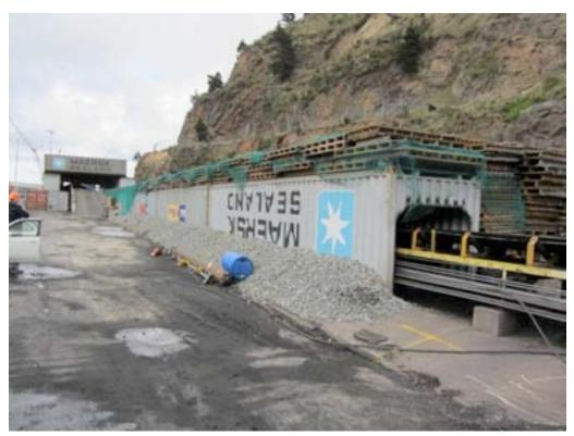
Figure 9-20. Ballasted shipping containers placed at the coal facility to protect against rock falls following the February 22, 2011 earthquake (looking west).
