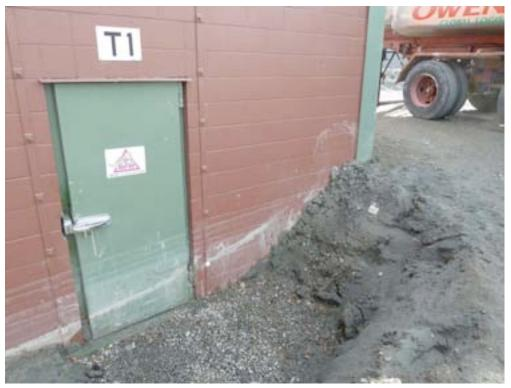
Figure 4-40. Liquefaction at Brighton Substation, Feb 22 2011
