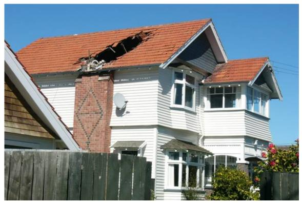
Figure 16-6. Damage to URM Chimney
