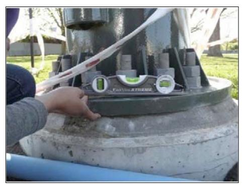
Figure 5-2. Antenna tower base at Gailbraith Exchange rotated 5° (Courtesy Telecom New Zealand)
