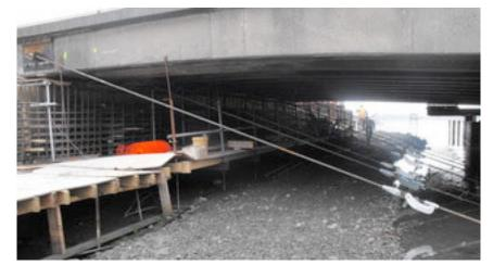
Figure 11-8. Temporary tie-back measure to arrest further lateral movement of pier/pile of Ferrymead Road Bridge (Photo: Lloyd Greenfield)
