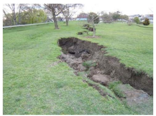
Figure 14-7. Levee Damage - Kaiapoi (Sept 2010)
