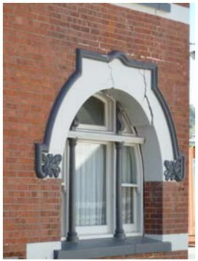
Figure 16-9. Sumner District Council Building (Failed Masonry Arch)
