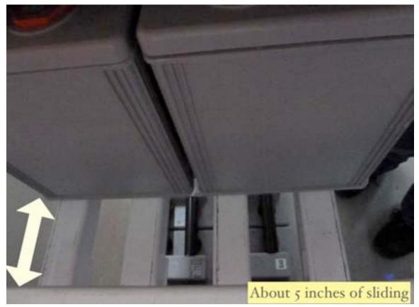
Figure 4-24. Sliding of Batteries in Battery Rack at Bromley Substation
