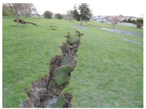
Figure 14-6. Levee Damage - Kaiapoi (Sept 2010)
