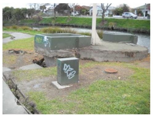
Figure 7-5. Floated and Tilted Wastewater Life Station 27, Avonside
