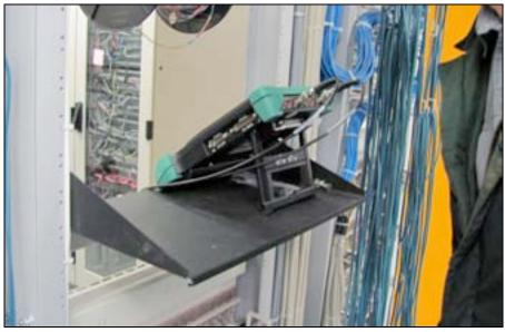
Figure 5-14. Test equipment shown was not secured to the shelf.
