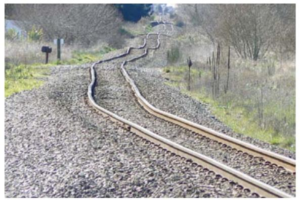
Figure 12-15. Ongoing Liquefaction along the Main North Line near Kaiapoi (mid-Sept 2010)
