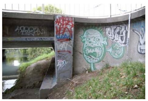
Figure 11-16. Shear crack in abutment of Fitzgerald Ave Bridge
