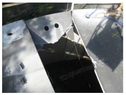
Figure 6-5. Damaged Segmented Concrete Roof, Detail, CCC (September 2010)
