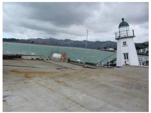
Figure 9-26. Lighthouse, Z Berth, Slumping of Eastern Mole following the February 22, 2011 earthquake (looking east).
