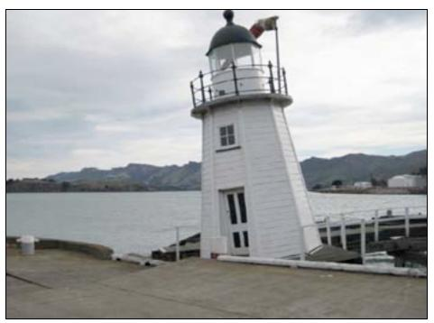
Figure 9-5. Lighthouse, Z Berth, Slumping of Eastern Mole
