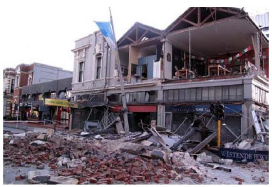
Figure 16-5. Damage to Walls for these URM Buildings
