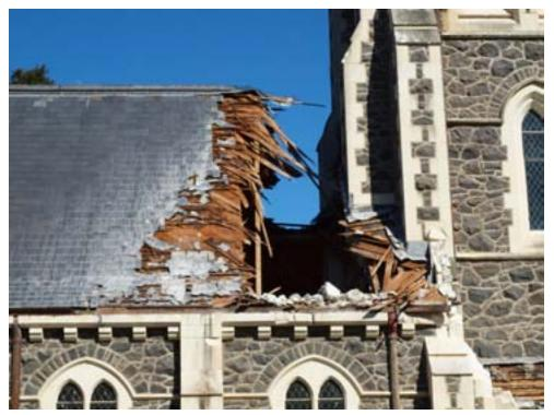
Figure 16-3. Fallen Debris Damaged Roof (Close Up from Figure 16-2)
