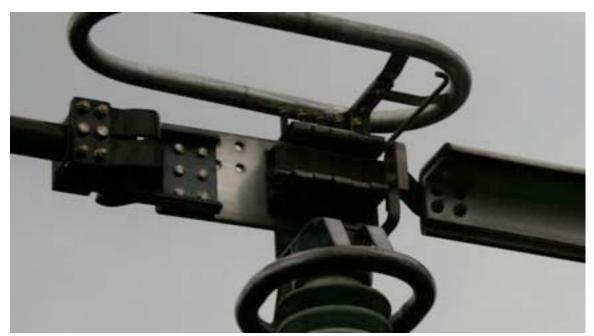
Figure 4-31. A disconnect switch with a 1cm offset in its contact.
