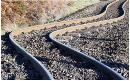
Figure 12-5. Buckling of Rails, Highlight of Figure 12-4 (Baxter)
