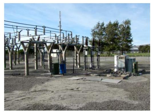
Figure 4-45. Pages Substation endings for the two 66 kV lines to Bromley Substation. A damaged bushing is observed on the left
