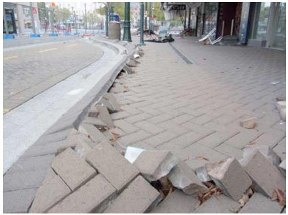
Figure 2-39. Liquefaction induced ground deformation in the Central Business District, February 22 2011
