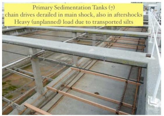
Figure 7-43. Scrapers, Bromley WWTP
