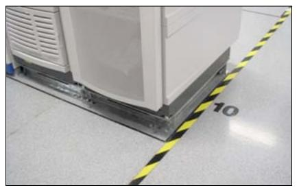
Figure 5-10. Equipment anchoring, Vodafone.
