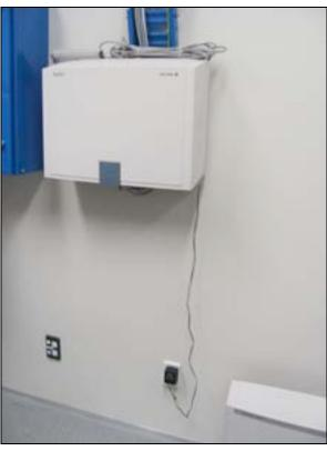
Figure 5-16. Power connection not protected from accidentally unplugged
