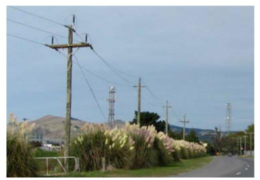
Figure 4-43. A temporary 66 kV line installed after the Feb 22 2011 and running from Bromley Substation (seen on the background behind the white gates on the left) and the temporary transformer shown in Figure 4-44.
