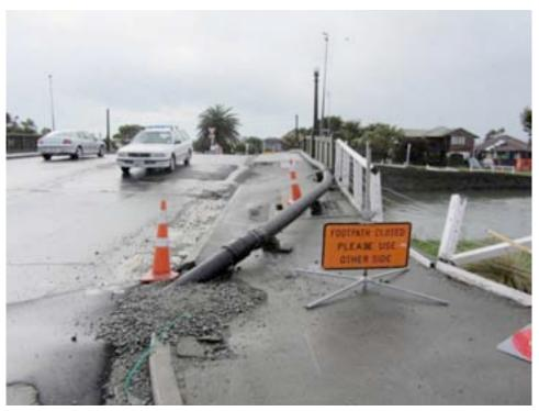
Figure 7-36. Sewer pipe bypass over the Avon River at Brighton Bridge.
