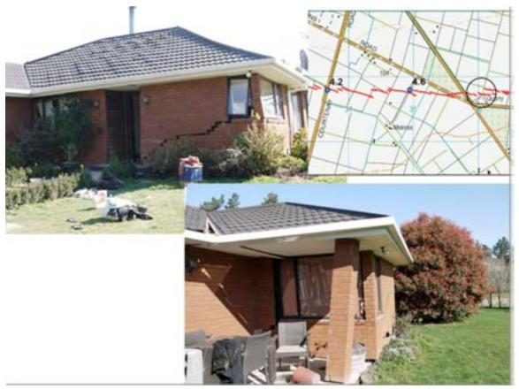
Figure 16-7. Fault Offset Through a House
