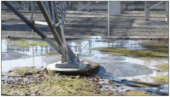
Figure 4-13. Sand Boil, Upgraded Tower, Papanui Substation
