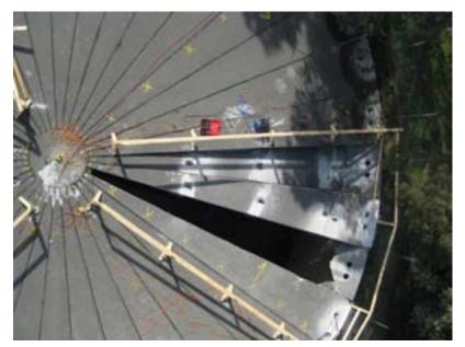
Figure 6-4. Damaged Segmented Concrete Roof, CCC (September 2010)
