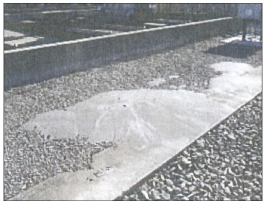
Figure 4-11. Sand Boils, Papanui Substation
