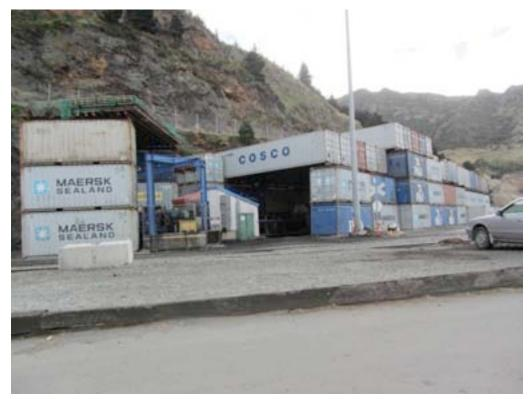
Figure 9-19. Ballasted shipping containers placed at the coal facility to protect against rock falls following the February 22, 2011 earthquake (looking east).
