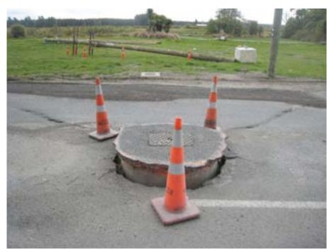
Figure 7-6. Floated Sewer Manhole, Brooklands (one of fifteen)
