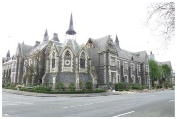
Figure 16-1. Damage to Parapets and End Gables for this URM Heritage Building
