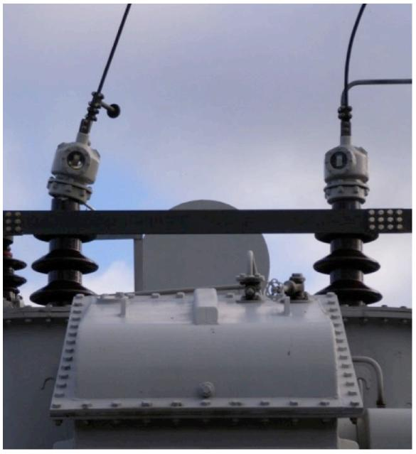
Figure 4-29. Broken Transformer Bushing, 66 kV, Bromley Substation
