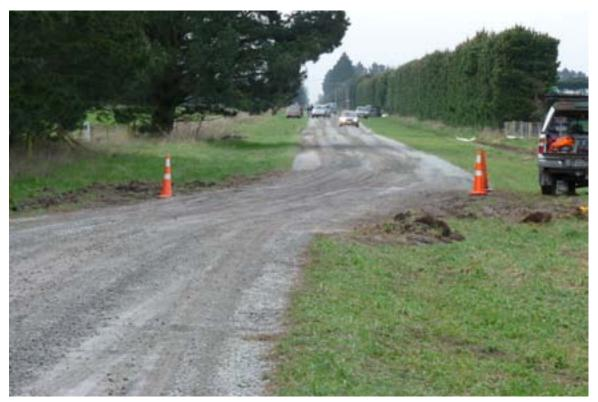
Figure 2-25. Fault Offset Through a Road
