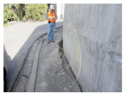
Figure 6-25. Evidence of Ground Failure, Southeast Corner of Huntsbury Concrete Reservoir
