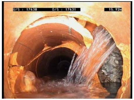
Figure 7-9. CCTV picture of Broken Sewer, WDC
