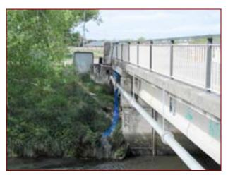
Figure 11-4. Plastic hose connected to broke pipe to discharge wastewater to stream
