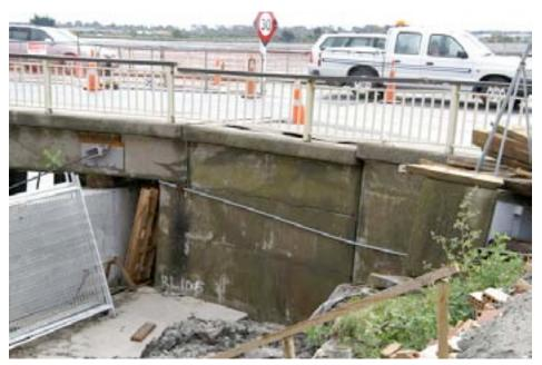
Figure 11-7. Rotation and lateral movement toward river of Ferrymead Road Bridge abutment and partial view of emergency tie-back measure to bridge pier/pile
