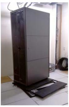
Figure 17-7. Base Isolation System as Found, Immediately Post-Earthquake
