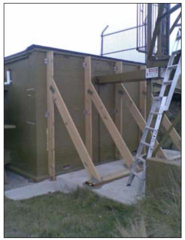
Figure 5-21. The URM wall was pulling on the cable tray at the MT Pleasant Radio site.(Courtesy Telecom NZ)
