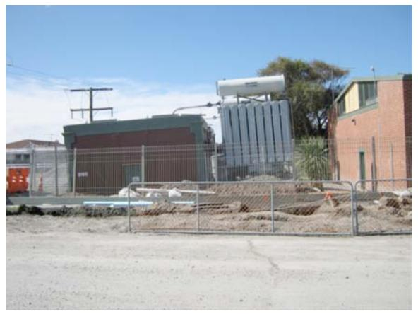
Figure 4-41. Liquefaction at New Brighton Substation, Feb 22 2011
