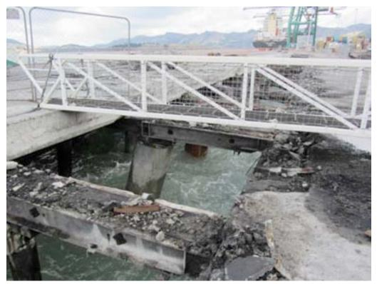
Figure 9-12. Damaged piles and beams at berth CQ2 (looking west).
