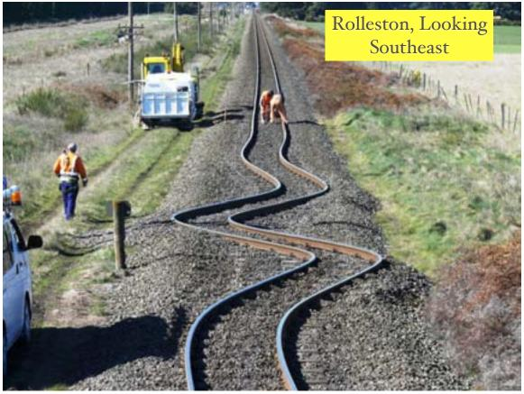
Figure 12-3. Buckling of Rails at Fault Offset Location
