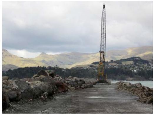
Figure 9-21. Breakwater east of harbor showing differential permanent deformations and ongoing repairs (looking south).
