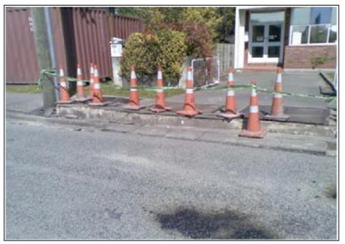
Figure 5-6. Halswell Exchange, the underground fuel tank was raised due to liquefaction (Courtesy of Telecom New Zealand)
