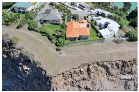
Figure 2-45. Cliff Edge Cracks, Sumner Head, February 22 2011
