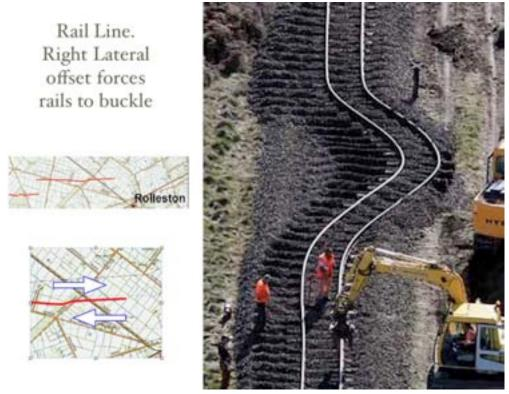
Figure 12-6. Rails Being Repaired
