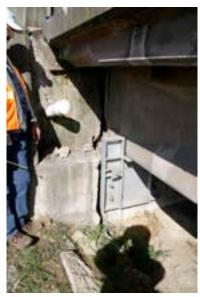
Figure 11-26. Cracks in abutment of Horotane Valley Road Overbridge
