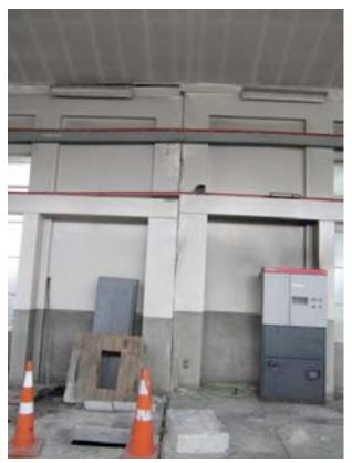
Figure 7-34. Pages Road Sewer Pumping Station differential movement.
