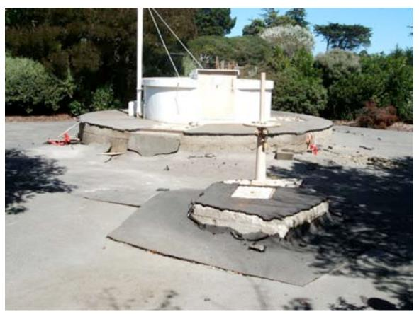
Figure 7-32. Flotation of Sewer Lift Station, April 2011
