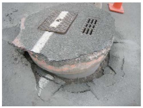
Figure 7-7. Floated Sewer Manhole, Brooklands (one of fifteen)
