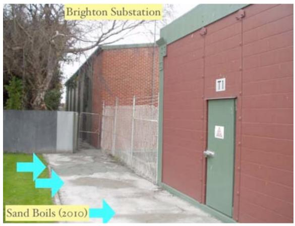
Figure 4-38. Liquefaction at Brighton Substation, September 4 2010
