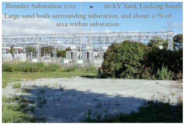
Figure 4-27. Liquefaction Outside the 66 kV Yard, Bromley Substation
