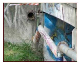
Figure 11-5. Close up of the damaged wastewater pipe
