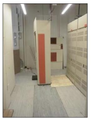
Figure 5-18. This equipment was straddled across a crack along the floor. It was relocated. (Courtesy Telecom NZ)
