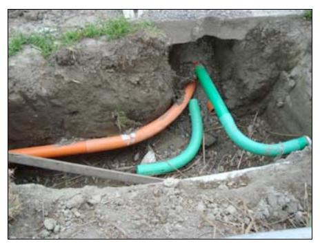
Figure 5-9. Under ground telecommunication cables repair, plastic ducts were used in this area northeast of Christchurch.
