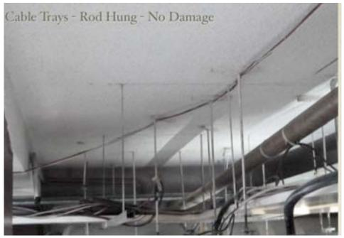
Figure 7-42. No Damage to Rod-Hung Cable Trays, Bromley WWTP
