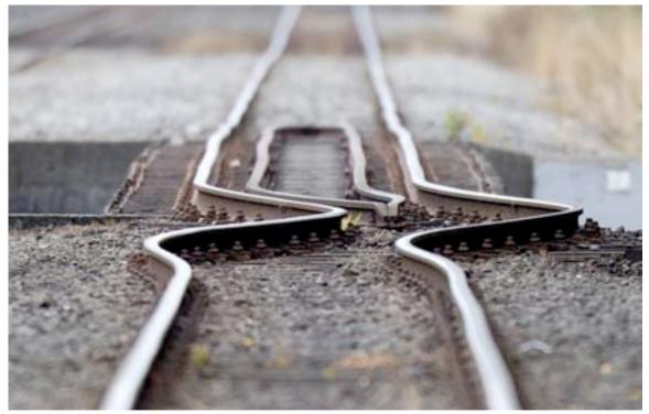
Figure 12-19 shows buckled tracks due to a lateral spread at a culvert.
