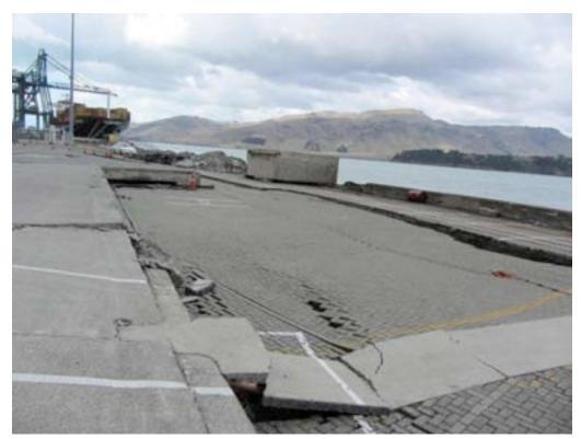
Figure 9-24. Ground settlements on north side of cool storage building (looking west, north of Figure 9-25).
