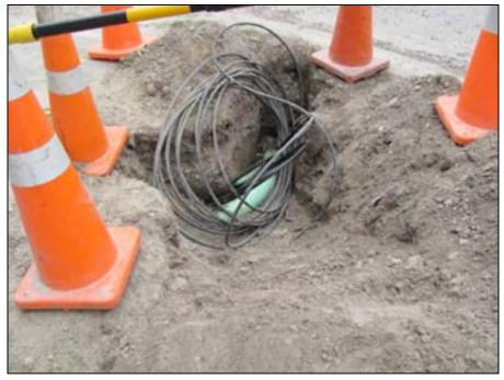
*Figure 5-8. In Christchurch, contractor was routing optical fiber cable to repair cable damage in this area.*
