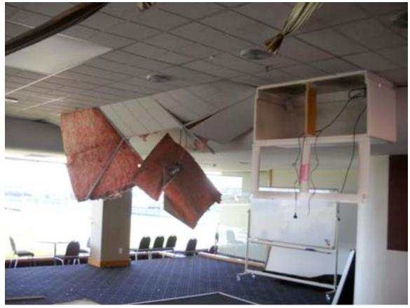
Figure 17-10. Suspended Ceiling (credit John Mackenzie) September 2010
