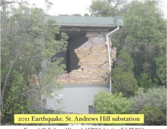
Figure 4-48. Failure of Upgraded URM Substation, Feb 22 2011
