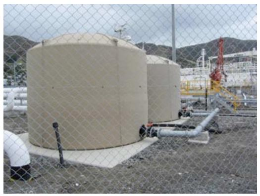
Figure 9-34. Flexible pipe connection to tank at the Lyttelton Port oil berth.
