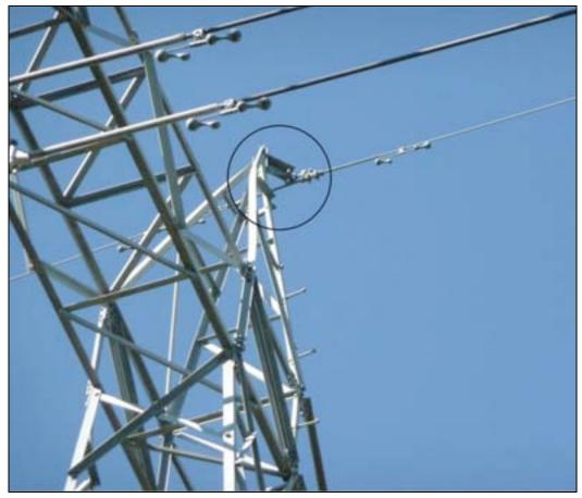
Figure 4-7. Damaged Tower Extension for Ground Wire
