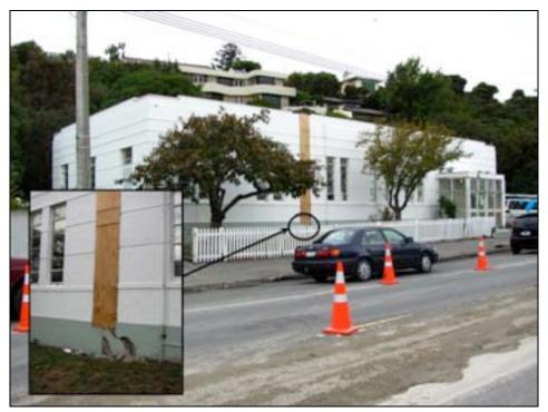
Figure 5-19. Weather seal was placed on the cracked expansion joint at Mt Pleasant Exchange.
