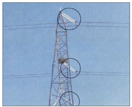
Figure 4-6. Displaced Insulators on Suspension Tower Adjacent to Fault Offset
