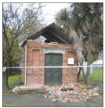
Figure 4-20. Orion URM Non-Upgraded Former Small Substation
