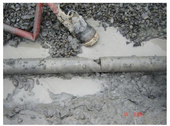
*Figure 6-8. Broken Barrel of Water Pipe (September 2010)*
