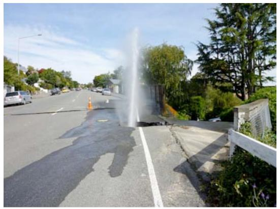
Figure 6-29. Water Leak, February 2011 Earthquake
