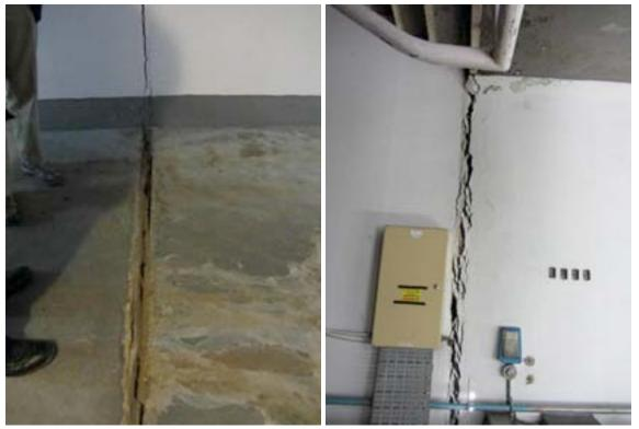
Figure 7-50. Gallery Damage, Bromley WWTP
