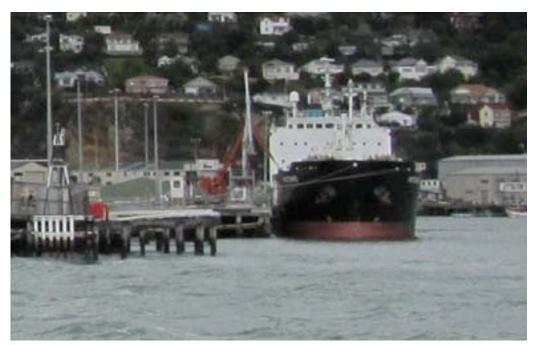
Figure 9-30. Oil berth wharf (looking west) showing backward rotation resulting from deep slide movement.
