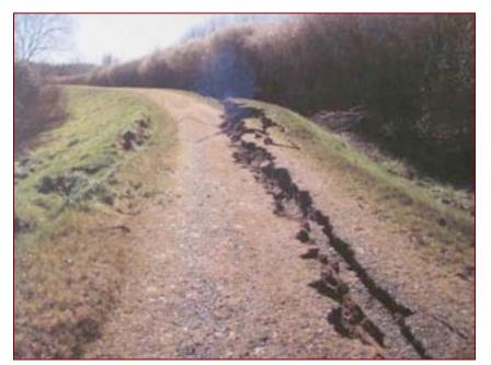
Figure 14-3. Severe Damage – Stopbank
