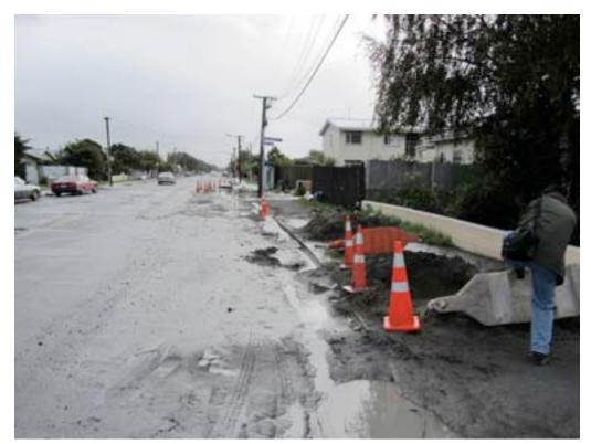
Figure 2-38. Liquefaction induced ground deformation on Palmers Road, Feb 22 2011
