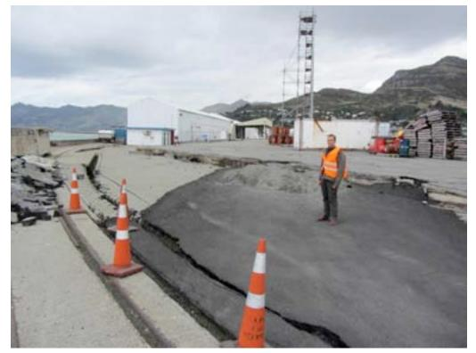
Figure 9-22. Ground deformations on east end of CQ4 at transition toward Z berth (looking west).
