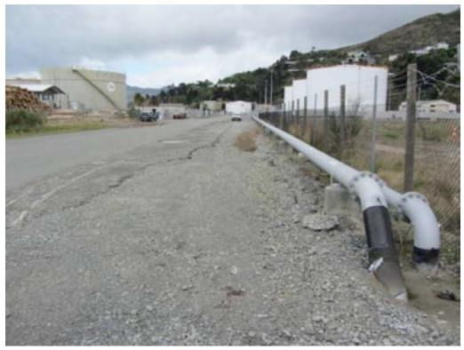
Figure 9-32. Ground cracking at the Lyttelton Port oil berth.
