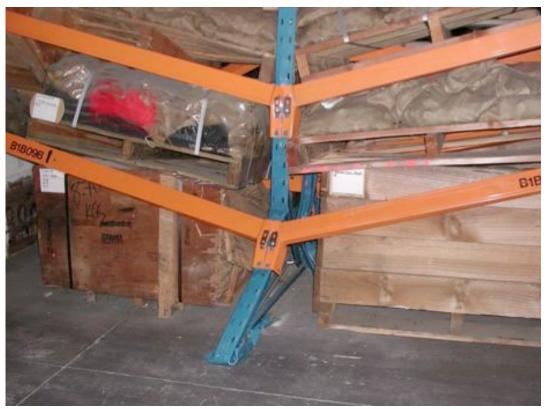
Figure 17-3. Damaged Column Leg, Addington Warehouse
