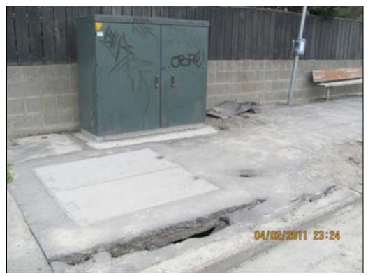
Figure 5-17. Street Cabinet impacted by liquefaction, note the slight uplift of the manhole
