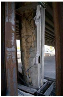
Figure 11-11(b). Shear failure and buckled smooth rebar of column of Moorhouse Avenue Bridge at Colombo Street
