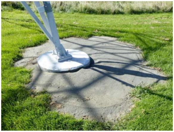
Figure 4-33. Liquefaction at 220 kV Transmission Tower
