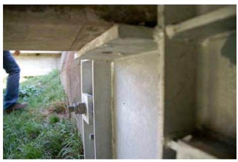
Figure 11-27. Shear-off of anchor bolt of seat width extension bracket of Horotane Valley Road Overbridge
