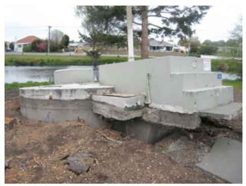
Figure 7-4. Floated and Tilted Wastewater Life Station 26, Porritt Park, Avonside
