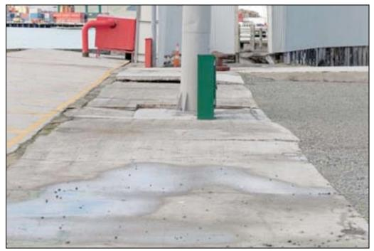
Figure 9-7. Slumping of the Rubble Mound Sea Wall, Oil Berth
