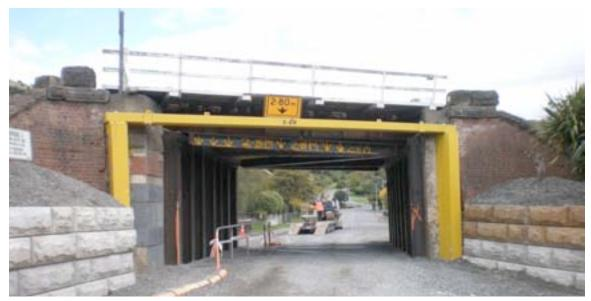
Figure 12-17. Bracing with steel supports
