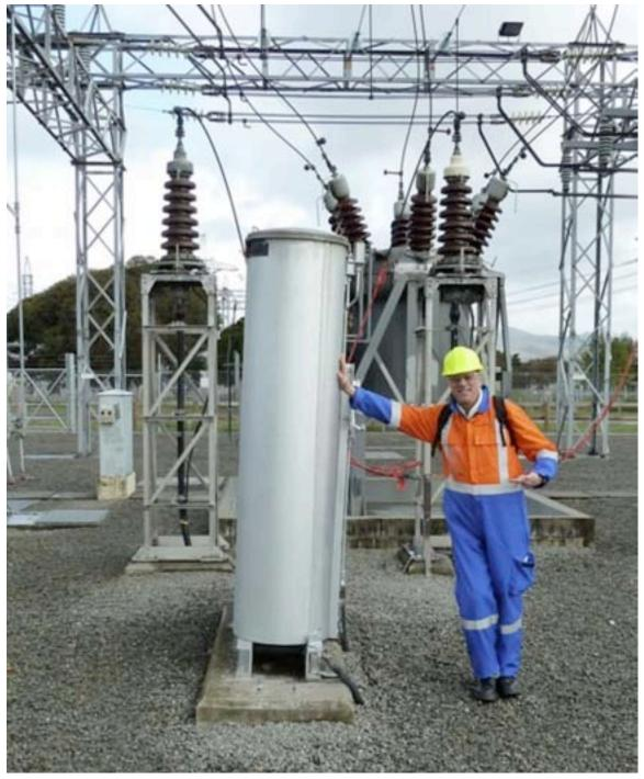
Figure 4-56. Oil Tank at Bromley Substation for Dallington No. 2 66 kV Cable.
