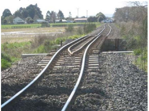
Figure 12-10. Soil Movement Next to Bridge Abutments
