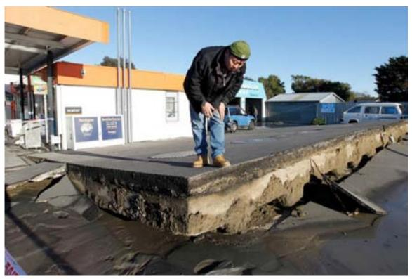
Figure 2-35. Floated Gas Tank, Bexley
