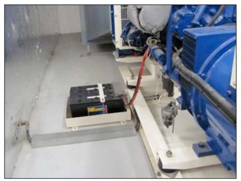
Figure 5-13. Starter battery mount for the backup power generator, Vodafone
