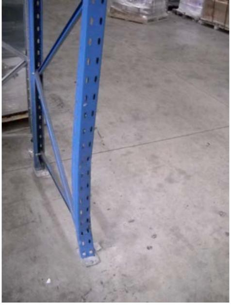
Figure 17-5. Storage Rack Leg, Incipient Failure, September 2010
