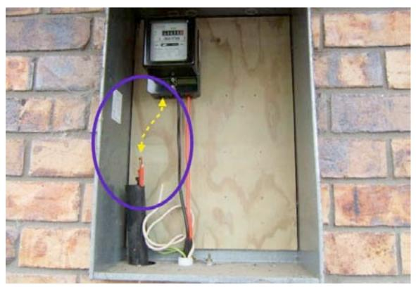
Figure 4-59. Damaged Cable to House Electric Meter – Kaiapoi – Sept 2010
