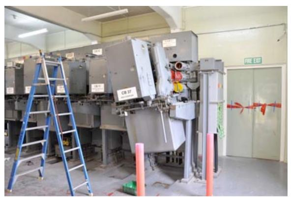
Figure 4-25. Toppled Circuit Breaker at Bromley Substation
