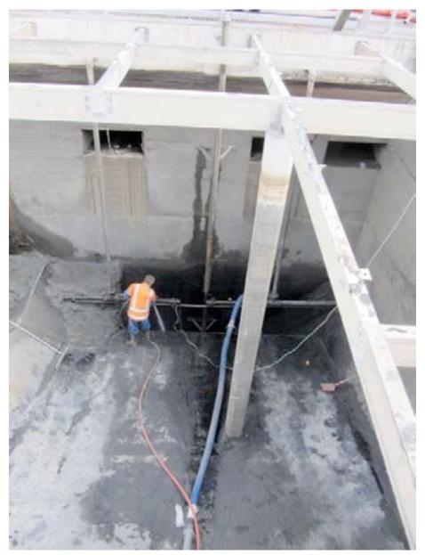
Figure 7-44. Grit Chamber cleaning, Bromley WWTP
