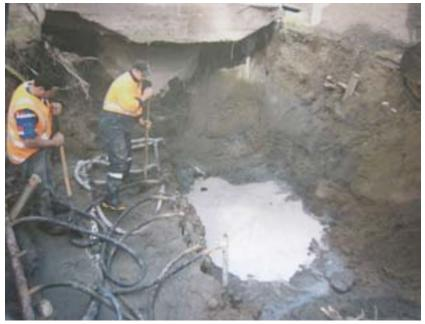
Figure 7-16. Repair of Sewer Pipe
