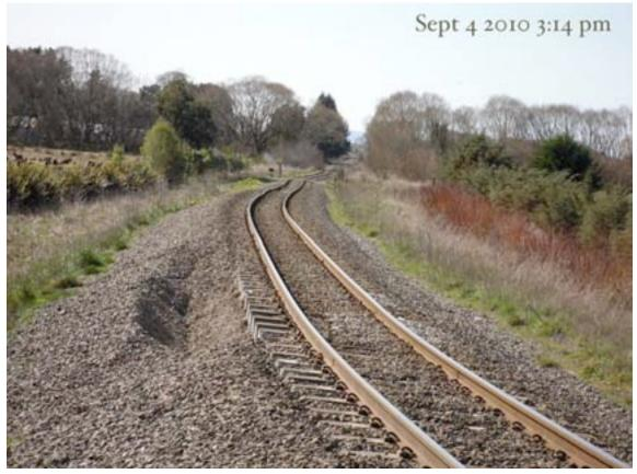
Figure 12-14. Liquefaction along the Main North Line near Kaiapoi (Sept 4 2010)
