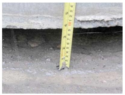
Figure 6-34. Well-head Differential Settlement
