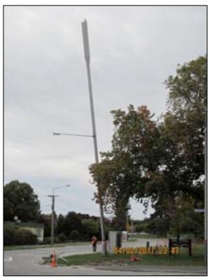
Figure 5-26. The cell site antenna pole tilted due to liquefaction in the Avon River area.
