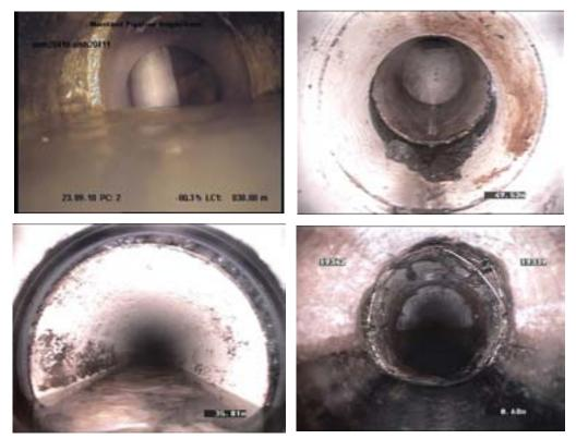
Figure 7-12. CCTV picture of Broken Sewers, WDC
