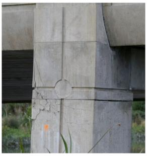
Figure 11-21. Flexural and shear cracks in column of Anzac Drive Bridge
