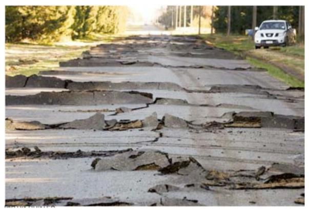
Figure 2-26. Fault Offset Through a Road, West of Rolleston
