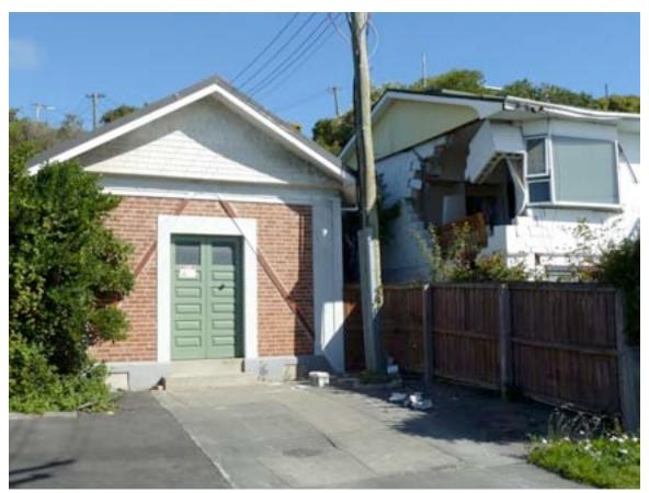
Figure 4-47. Success of Upgraded URM Substation, Feb 22 2011
