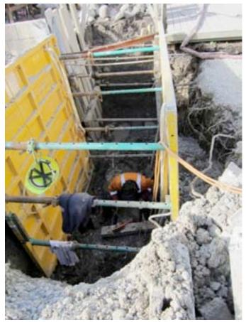
Figure 6-24. Repair of Outlet Pipe, Huntsbury Concrete Reservoir
