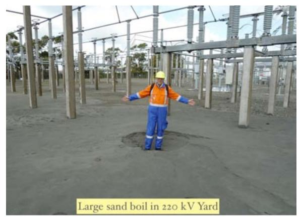
Figure 4-28. Sand Volcano, ~ 1 Foot Deep, inside the 220 kV Yard, Bromley Substation
