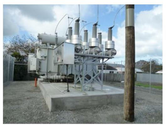
Figure 4-42. Temporary transformer installed after the Feb 22 2011 earthquake in order to restore service to the New Brighton Substation area.
