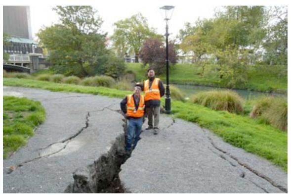
Figure 2-41. Liquefaction, Avon River Bank, CBD, February 2011
