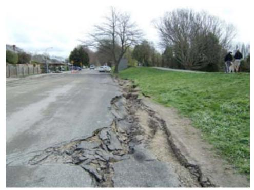
Figure 14-8. Levee Damage - Kaiapoi (Sept 2010)
