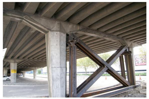
Figure 11-10. Temporary bracing support of column bent with expansion joint of Moorhouse Ave Bridge at Colombo Street
