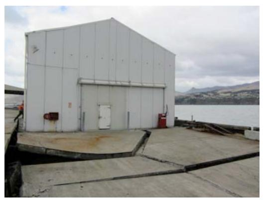
Figure 9-25. Deformations on west side of cool storage building (looking east).
