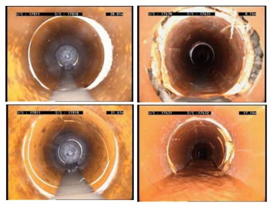
Figure 7-11. CCTV picture of Broken Sewers, WDC
