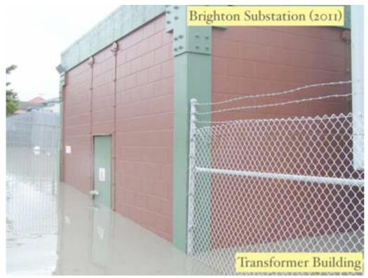
Figure 4-39. Liquefaction at Brighton Substation, Feb 22 2011
