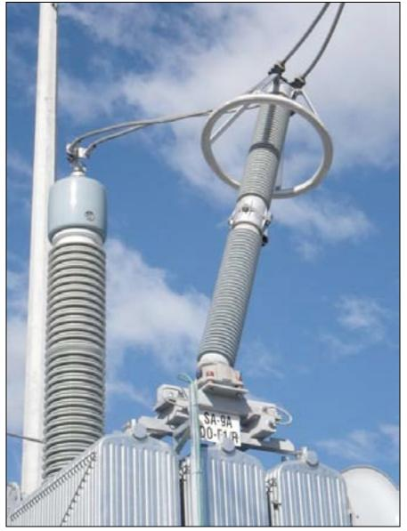
Figure 4-10. Broken Lightning Arrestor
