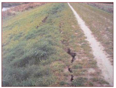
Figure 14-5. Moderate Damage – Stopbank
