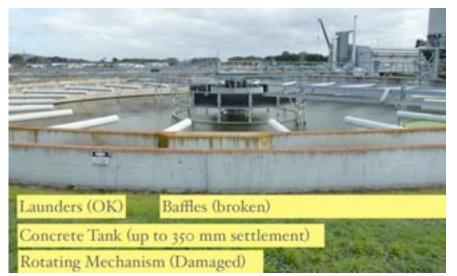
Figure 7-48. Broken Secondary Clarifier, Bromley WWTP
