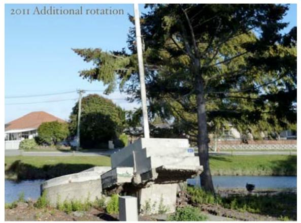
*Figure 7-31. Rotation and Sewer Lift Station, April 2011 (see Fig 7-4 for Comparison)*
