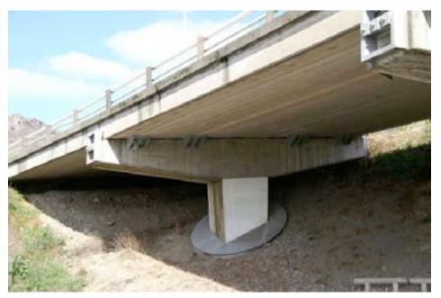
Figure 11-23. Retrofit measures of lateral restrainer, span tie-link/seat width extension bracket, and short column collar on Port Hills Road Overbridge on SH74
