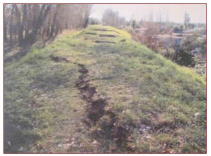
Figure 14-4. Major Damage – Stopbank
