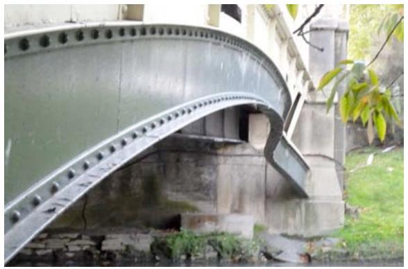
Figure 2-42. Damaged Bridge Girder due to Lateral Spread, CBD, February 2011
