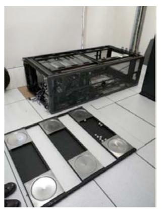
Figure 17-8. Base Isolation System, Disassembled
