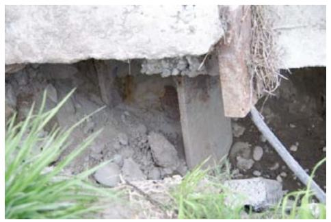
Figure 11-20. Damaged rotated pile at abutment of Anzac Drive Bridge
