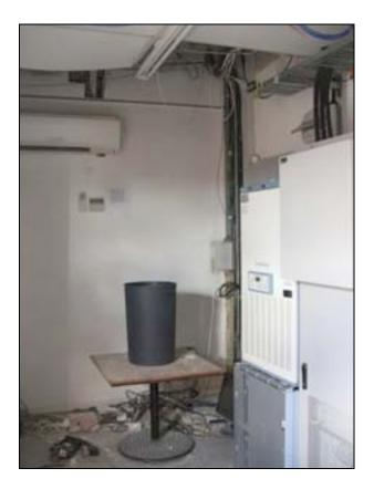
Figure 5-20. Liwood Mall Cell Site, fallen ceiling tiles, the site was operational. (Courtesy Telecom NZ)
