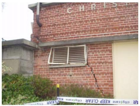
Figure 6-7. CCC Pump Station Damaged due to Differential Settlement
