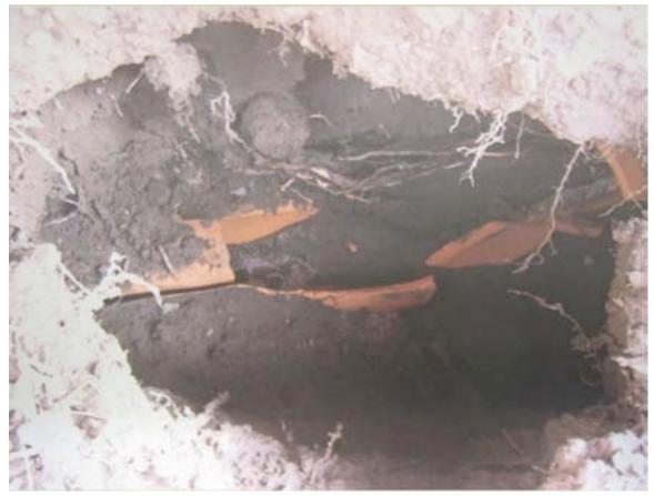
Figure 7-17. Repair of Vitrified Clay Sewer Pipe
