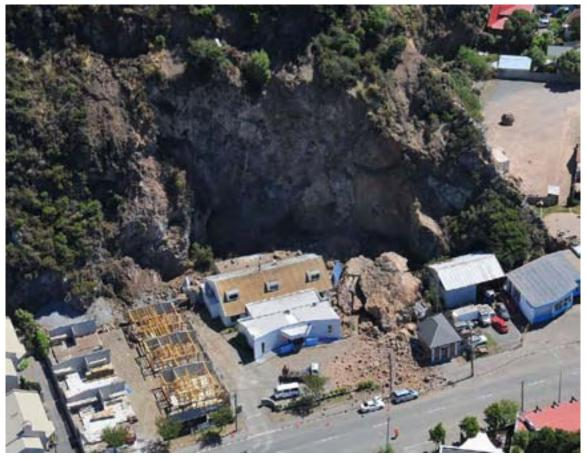
Figure 4-35. Substation in Summer damaged by a large boulder that fall in its back.
