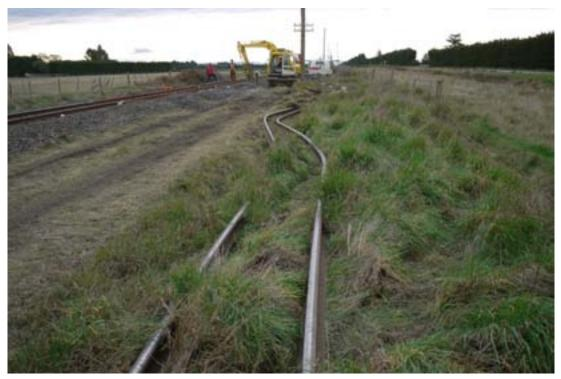
Figure 12-8. Removed Rail Segments
