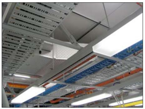
*Figure 5-12. Cable rack structural frame securing the cable racks and light fixtures, Vodafone.*
