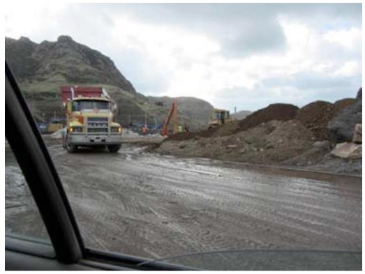
Figure 9-27. Processing and placement of rubble for the Te Awaparahi Bay reclaimation.
