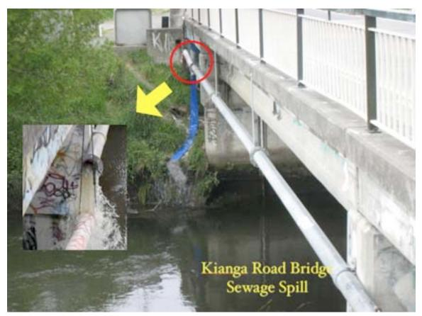
Figure 7-14. Broken Sewer Pipe
