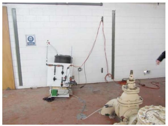
Figure 6-39. Temporary Chlorination System Deployed for First time in Christchurch
