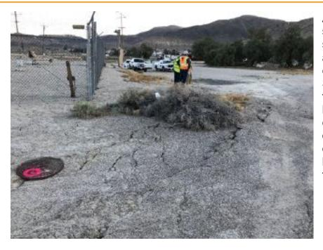
Apparent settlement/lateral spread headscarp at northwest corner of station. Searles Lake is off the photo to the left (east), and crack patterns and direction of extension suggest lateral movements toward the lake.
