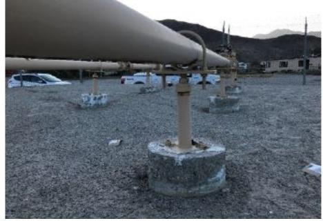
Differential settlement and lateral displacement across the station pad and foundations
