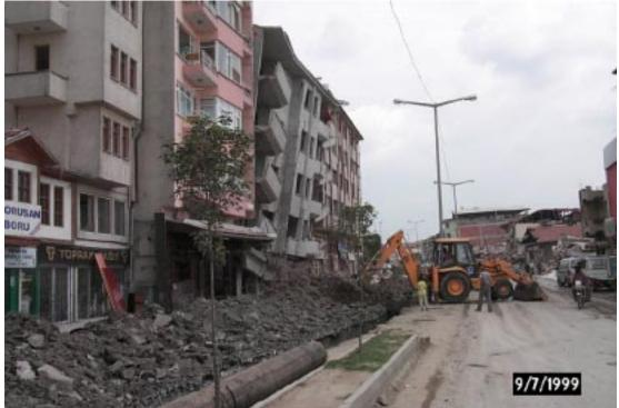
Figure 14. Installation of New Butt Welded Steel Pipe – Adapazari
