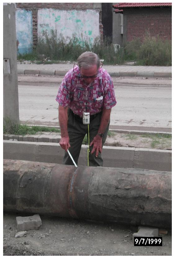
Figure 13. New 16" Diameter Butt Welded Pipe for Replacement of AC Pipe
