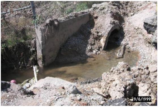
Figure 5. Fault Offset Through Storm Drain, Arifiye
