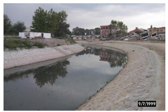
Figure 16. Solids in Storm Canal Due to Combined Flow from Broken Sanitary Sewers
