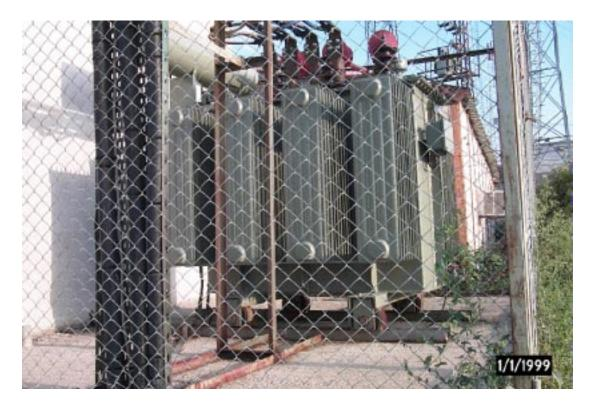
Figure 9. Unanchored Transformer Serving Maltepe WTP. A Bushing was Damaged.
