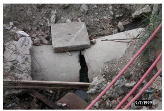
Figure 15. Broken Sanitary Sewer in Adapazari.
