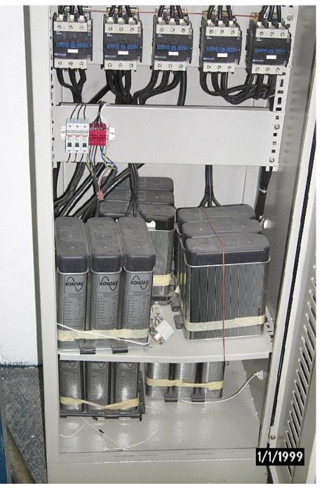
Figure 8. Unanchored Batteries at Maltepe WTP. They Tipped Over in the Earthquake
