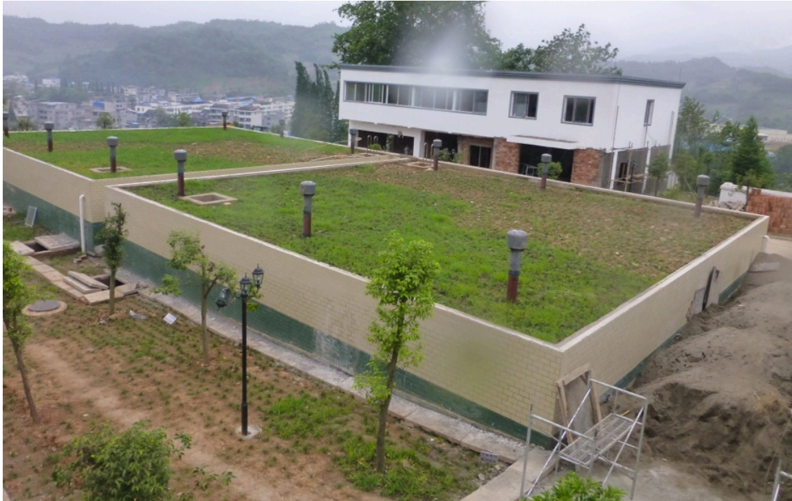
Figure 8. Two Partially Buried Clearwells
