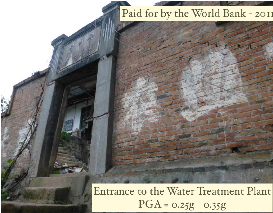
Figure 6. Entrance to Water Treatment Plant
