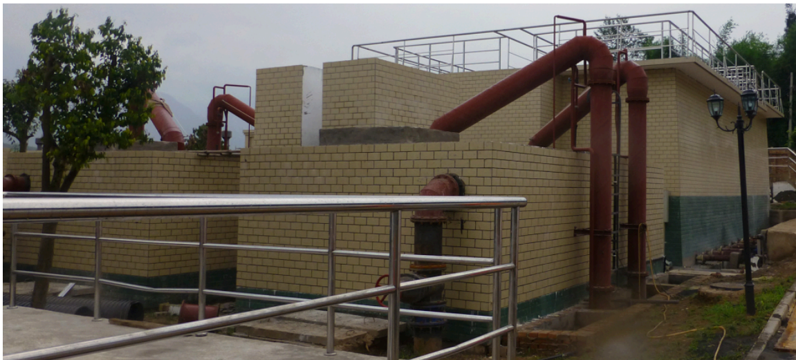
Figure 7. Settling and Filter Basin Structures
