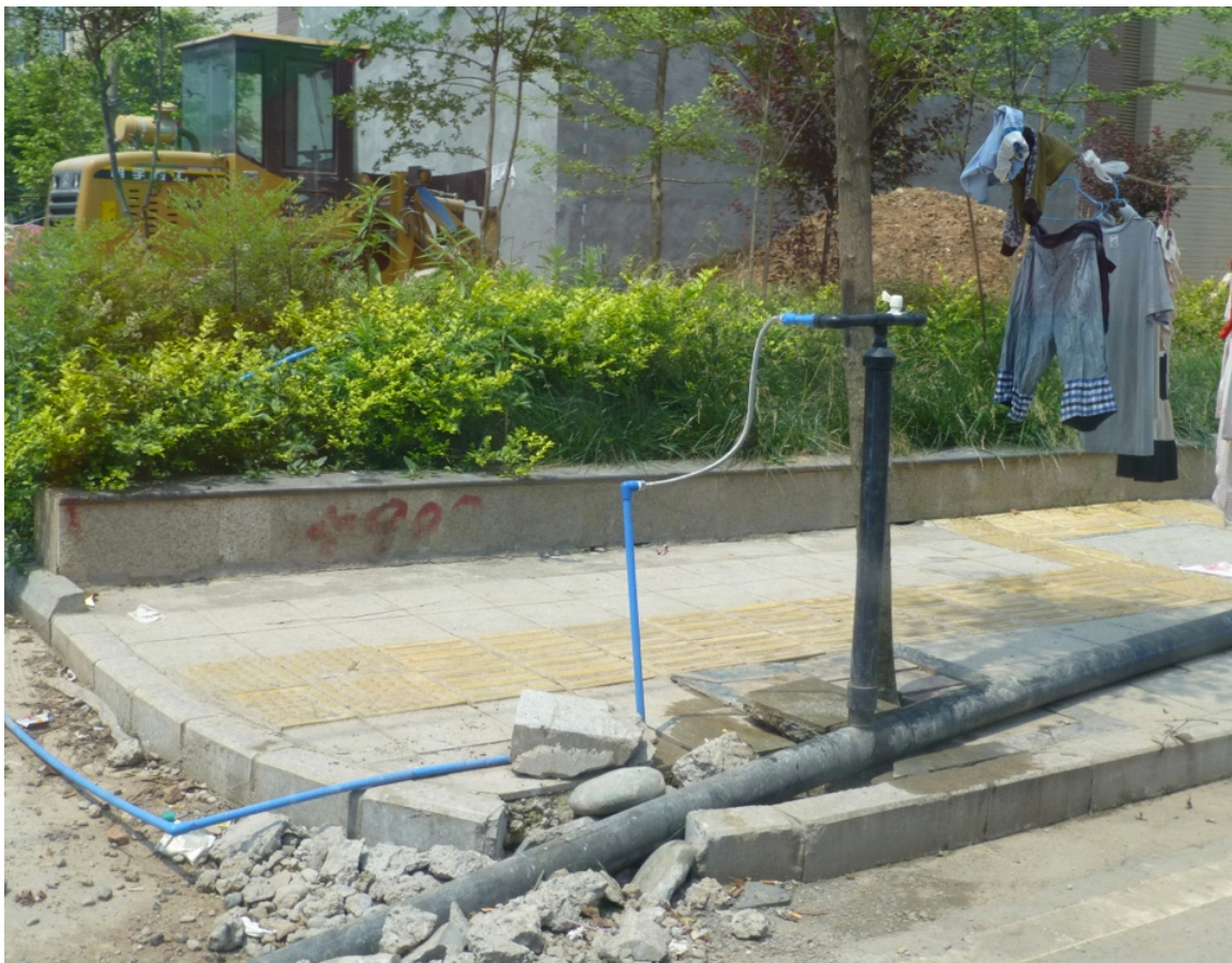
Figure 13. Above Ground Temporary Water Pipe
