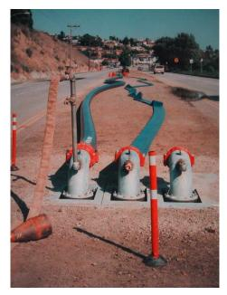
Figure 2. Flex Hose Deployment in EBMUD System
