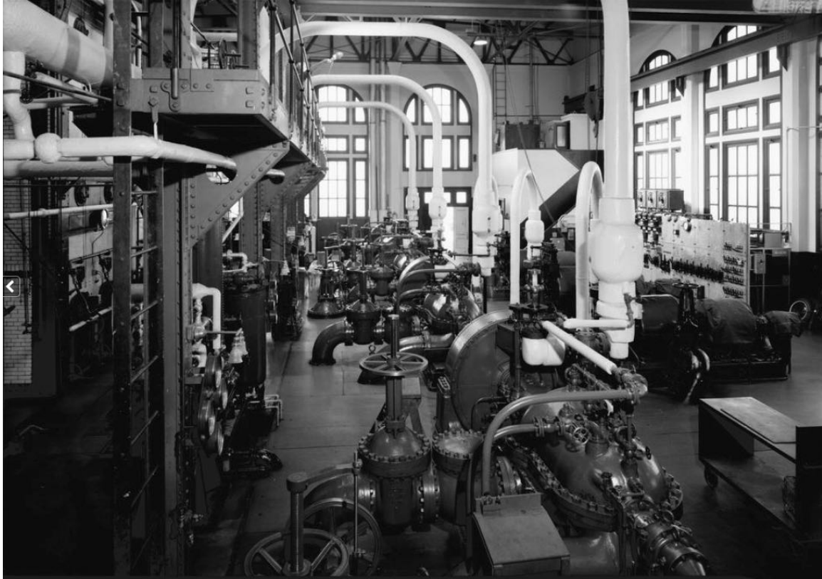
Figure 8-6. Interior of AWSS Pump Station 2, c. 1912 (photo: Manson)
