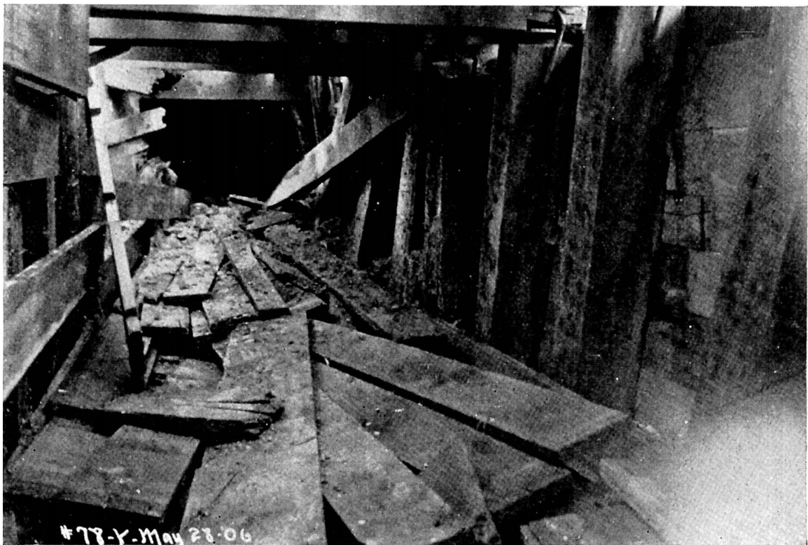
Figure 4.1.12-5. Interior of Wastewater Flume, Looking Northeasterly (photo: Schussler 1906)
