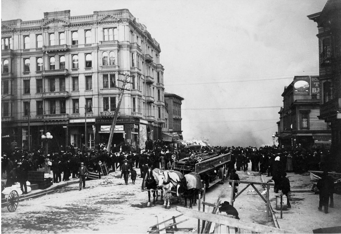
Figure 7-16. April 18. Looking southerly along 7th Street. Mission Street is the cross street the foreground. The tilted wood pole reflects the major liquefaction movements at this corner. There is no water available at any hydrant near here. The fire is burning near 7th and Howard.
