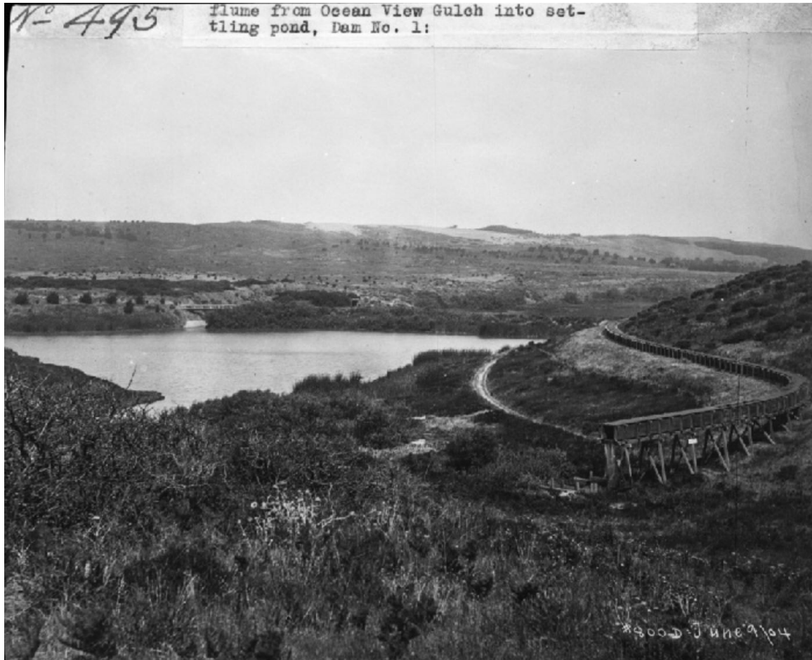
Figure 4.5-1. SVWC Flume discharging water into a Lake Merced settling pond, June 9, 1904 (credit: San Francisco Library)
