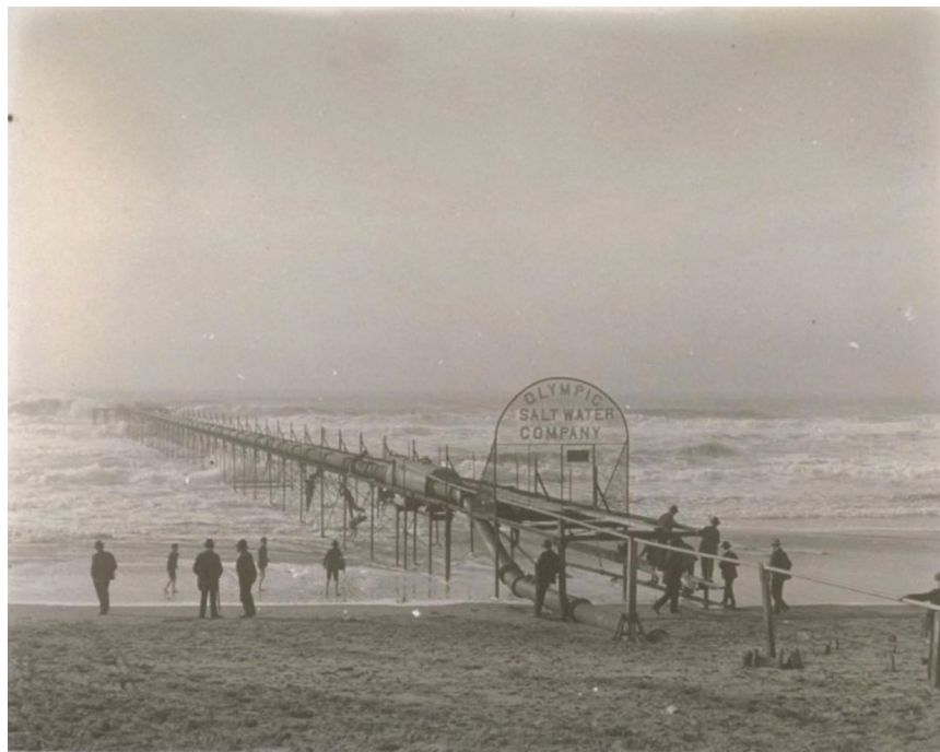
Figure 2-13. Salt Water Intake Pipe (Bancroft Library)
