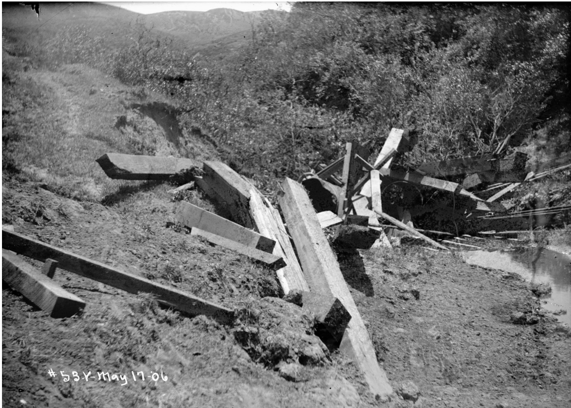
Figure 4.1.1-3. Large Frawley Canyon. View downstream, looking easterly Shows debris of the bridge that has been thrown 40' to 50' to the east. (Photo: Schussler 1906, HS10)
