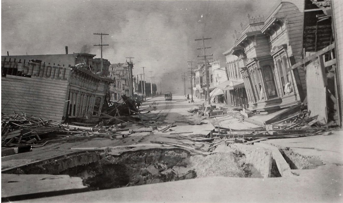
Figure 7-44. April 19. Looking North. The fire that was burning near Market Street on April 18 has advanced and is making its way southwards along Valencia Street. Liquefaction had wrecked other wood buildings on the east side of Valencia Street. (Photo credit: Online Archive of California, The 1906 San Francisco Earthquake and Fire Digital Collection, U. C. Berkeley, Bancroft Library)
