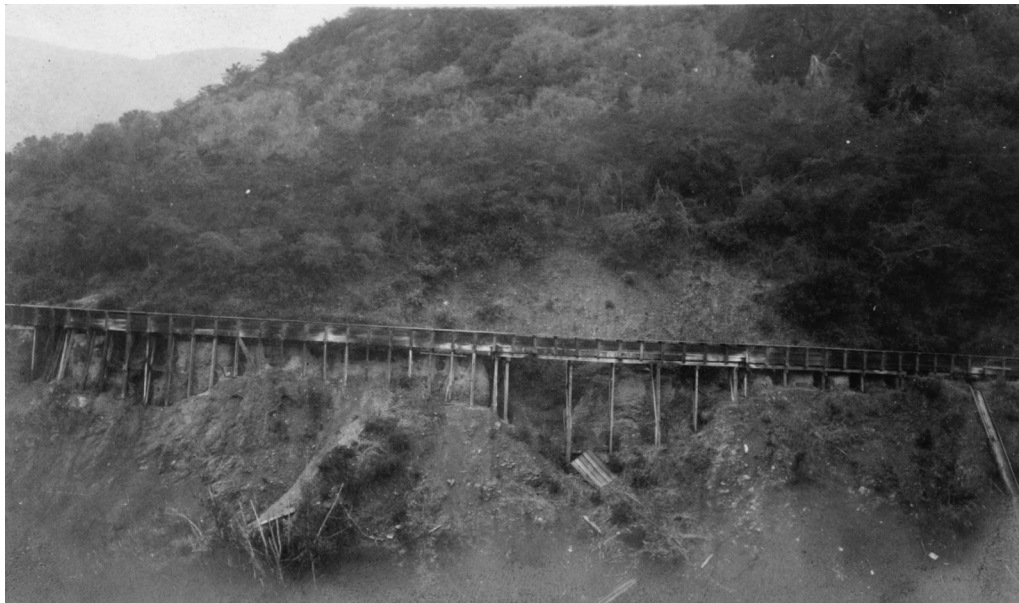
Figure 4.6-7. Repair of Flume. (Photo: SVWC).
