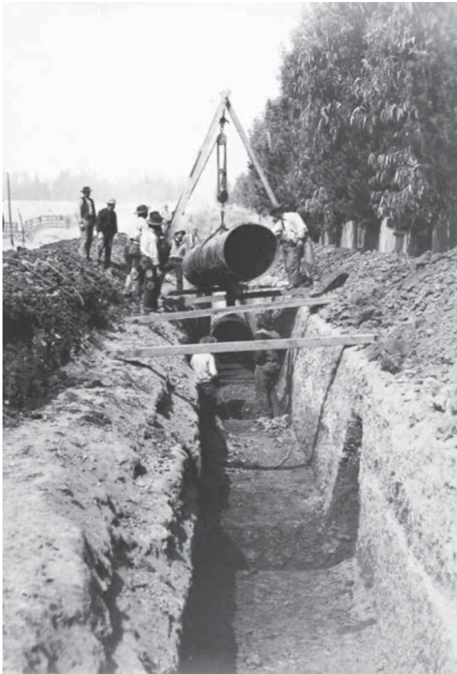
Figure 4.3-2. Crystal Springs 44" Pipeline Being Installed, El Camino Real, 1888 (Journal of the San Mateo County Historical Association, Volume xlvi, No. 1, 2018)
