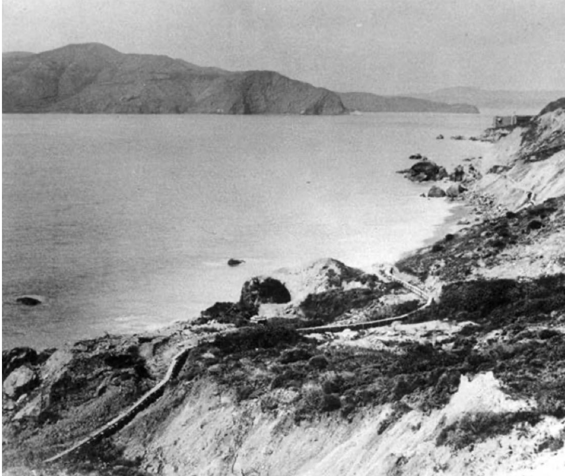
Figure 2-7. Lobos Flume Near Baker Beach (Photo: Bancroft Library, U. C. Berkeley)
