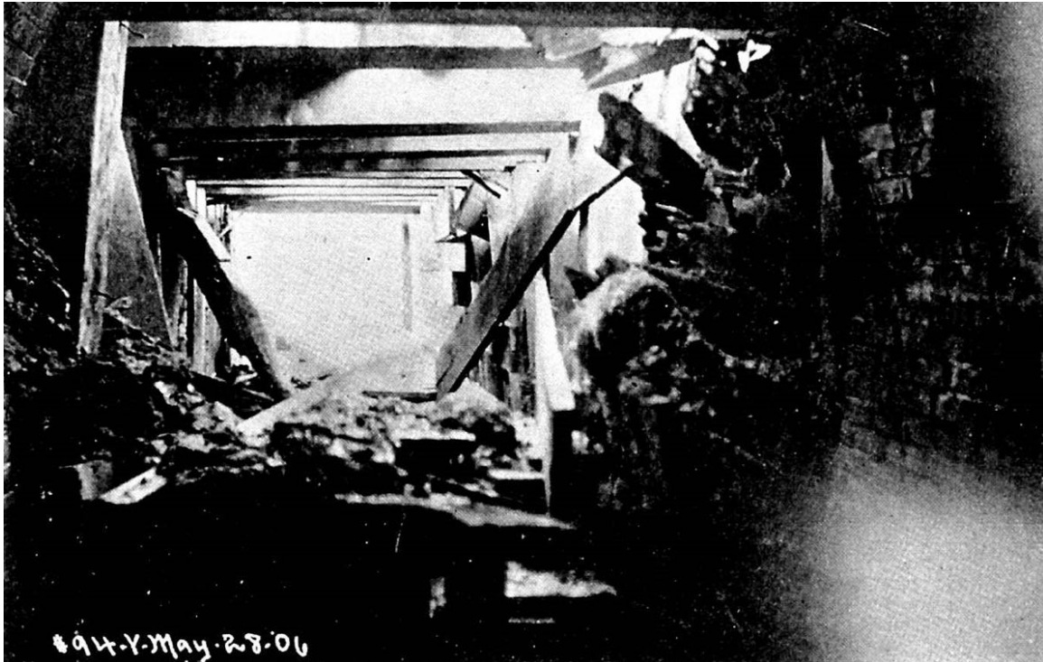
Figure 4.1.12-4. Interior of Wastewater Flume, Looking Southwesterly (photo: Schussler 1906)
