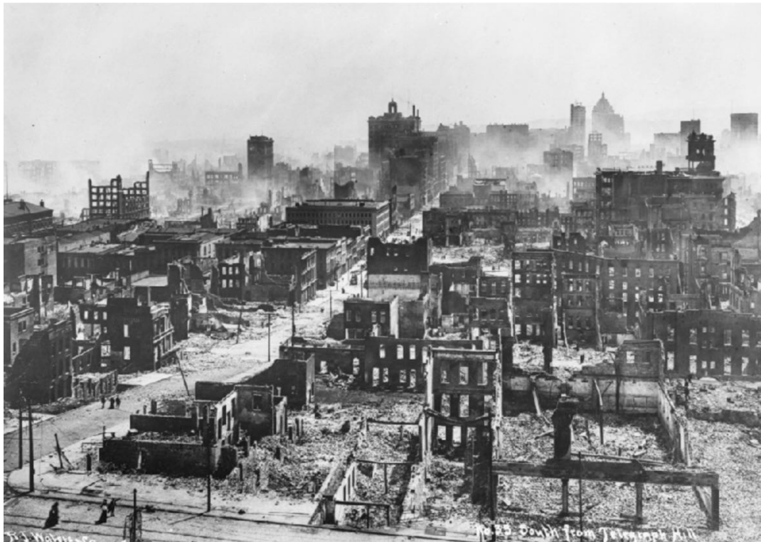
Figure 7-35. After the fire. Downtown Ruins, Looking southerly from Telegraph Hill. Broadway in foreground. Montgomery Street is long road leading to the distance.
