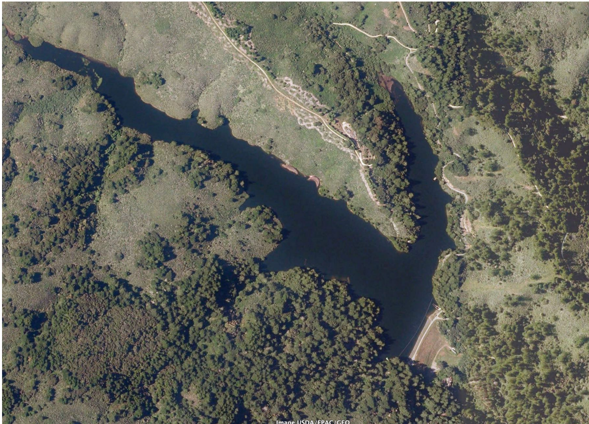
Figure 2-21. Pilarcitos Reservoir (Aerial image courtesy Google, April 2010)
