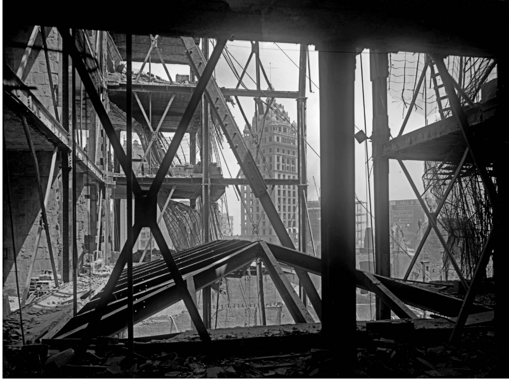
Figure 4.7-2. Interior of SVWC Office Building after 1906 earthquake. Call building in the background. (photo: Courtesy Mike Housh, SF Historian)
