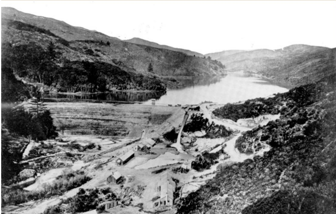
Figure 2-20. Pilarcitos Dam Under Construction, 1867-68 (SVWC, 1867)
