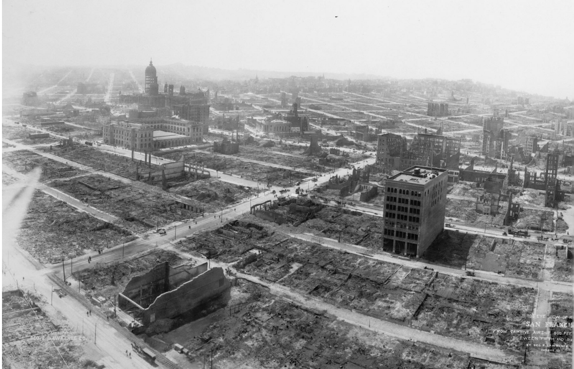
Figure 7-38. After the fire. View of the South of Market Street area, captured from the Lawrence Captive Airship from a height of 600 feet above Folsom, between 7 th (far left) and 6 th (center) streets. May 5, 1906. (Library of Congress, George Lawrence, 1906)
