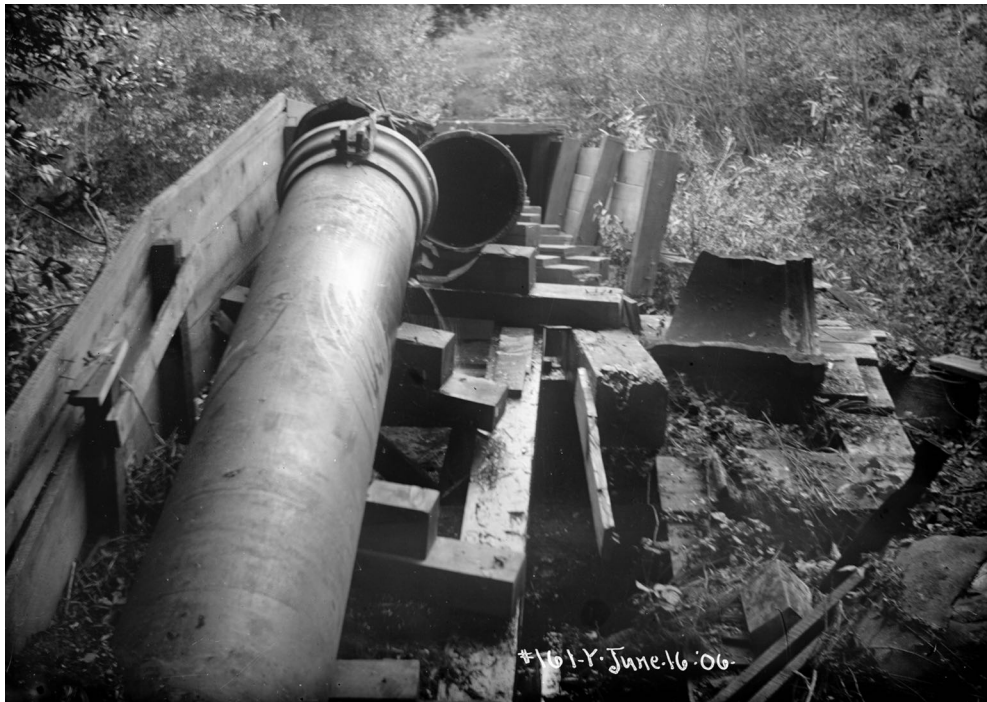
Figure 4.1.14-4. FX-5. 24" Pilarcitos Cast Iron Pipe, Looking east. East end of fault crossing zone. The pipe in the distance has moved to the right (southerly) relative to the pipe in the crossing zone. This is the same location as 4.1.14-3, but looking easterly along the pipe alignment. (Photo: Schussler 1906 HS12)
