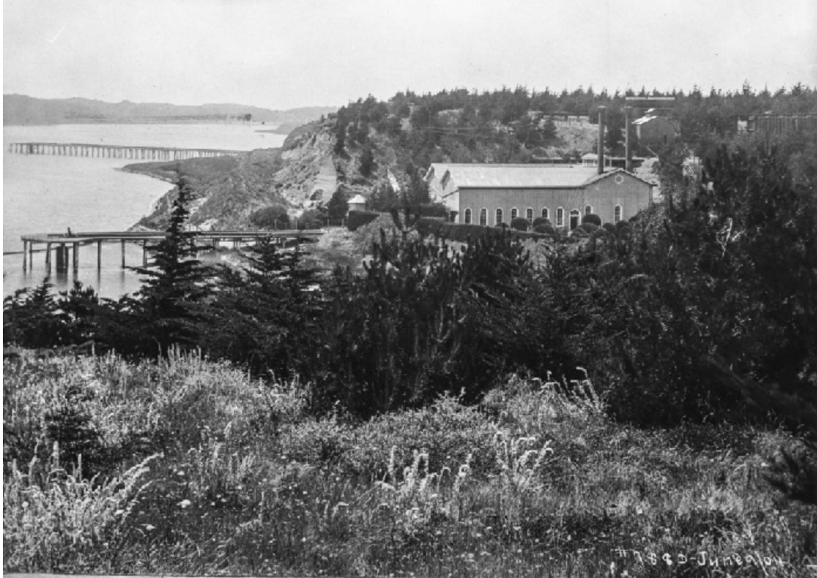
Figure 4.5-2. "New" Lake Merced pump station, near Brotherhood Way and Lake Merced Boulevard, looking north, June 9, 1904 (Credit: Schussler 1909)
