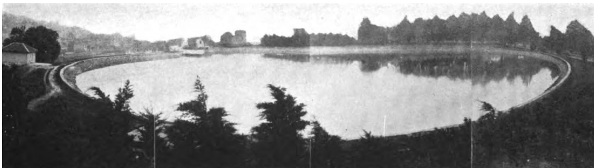
Figure 4.2-7. College Hill Reservoir, Terminus of San Andreas Pipeline (Credit: Schussler 1919)
