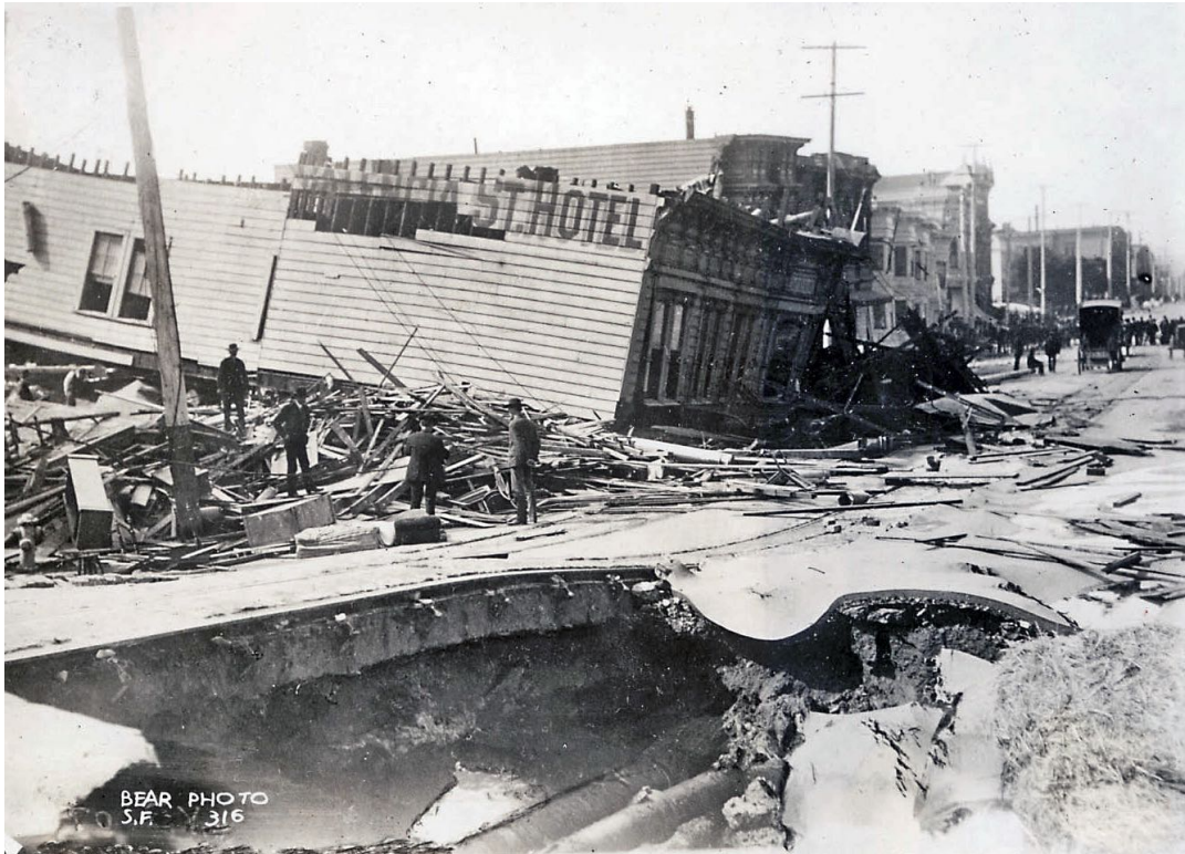
Figure 7-43. April 18 pm. Sink hole opened exposing broken SVWC 22" water main. It is unclear if the 4 people in the foreground are onlookers. (Photo credit: Bear Photo Co. 1906, Online Archive of California, The 1906 San Francisco Earthquake and Fire Digital Collection, U. C. Berkeley, Bancroft Library)
