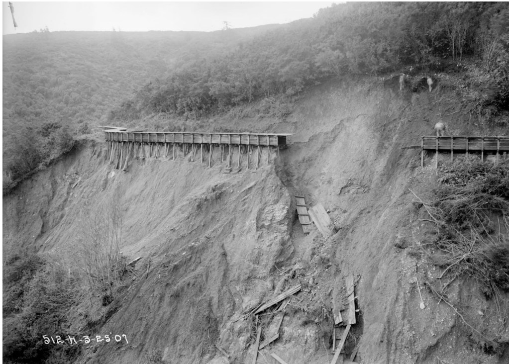
Figure 4.6-6. Collapse of Flume due to Landslide. (Photo: SVWC, 1907).
