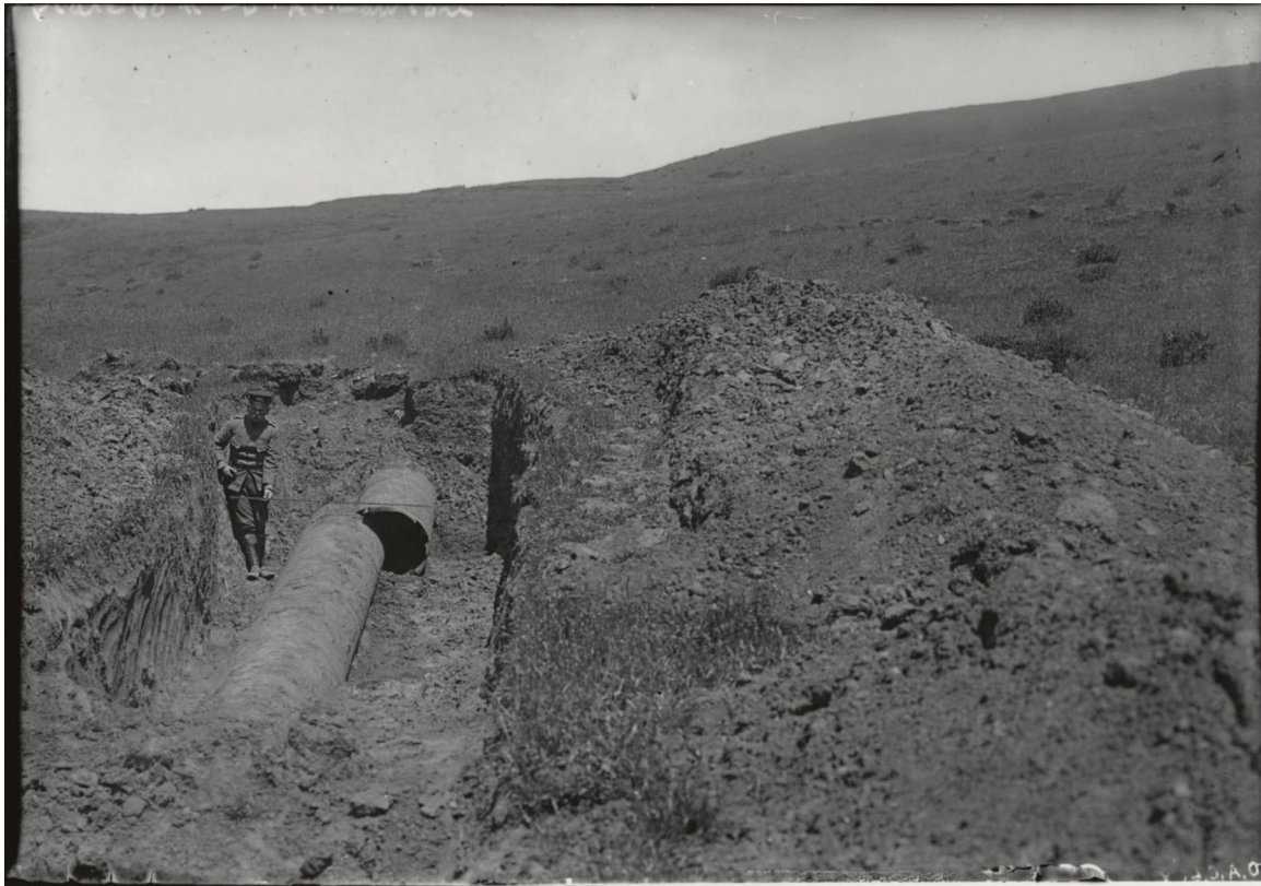
Figure 4.1.6-4. Crossing FX-3. Failure of Pilarcitos 30 inch pipe. (Photo: Lawson 1908)
