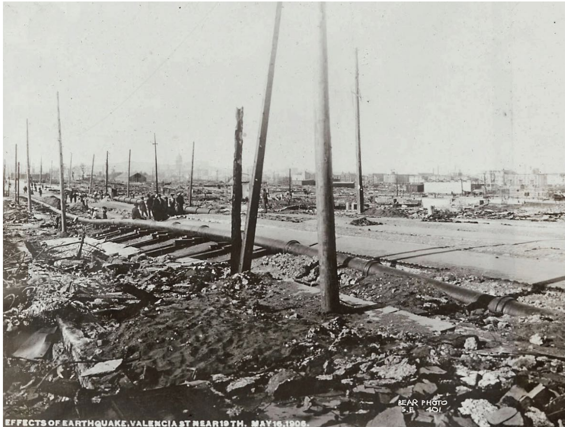
Figure 7-47. May 16, 1906. View of Valencia Street between 18 th and 19 th street, looking northeast. In the foreground is an above-ground 16" pipe laid by SVWC as a temporary bypass. In the background is the above-ground 22" pipe laid by SVWC as a temporary bypass on the east side of the street. City Hall dome is dimly seen in the distance just above the group of people in the center of the photo. The cross-arms on the power / telegraph poles have been lost to the fire, but most poles remain standing. (Photo credit: Bear Photo S.F. 401; Online Archive of California, The 1906 San Francisco Earthquake and Fire Digital Collection, U. C. Berkeley, Bancroft Library)
