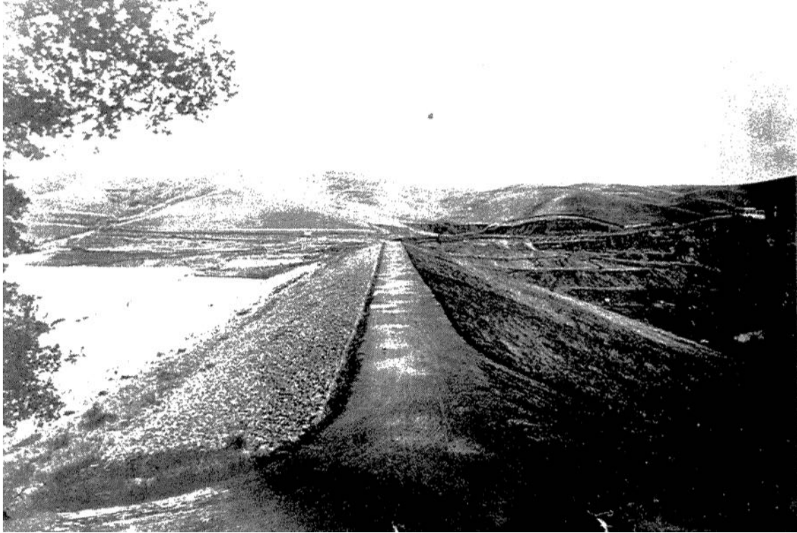
Figure 4.1.11-5. San Andreas Dam Soon after 1870 Construction, Looking Easterly (Babel, 1990)
