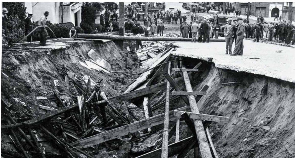
Figure 2-17. Collapsed street on 4 th Avenue between Anza and Balboa on March 18, 1930. (Horace Chaffee, SF Department of Public Works book A2488). Salt Water pipe runs perpendicular to the trench caused by erosion from the broken 12" pipe. It took 2 hours to isolate the leaking pipe.
