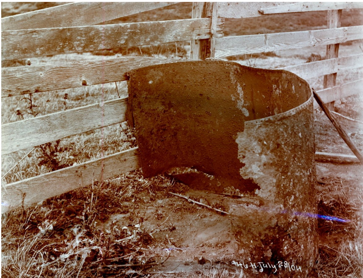
Figure 4-3. Failure of Pilarcitos 30" Low Pressure Pipe (WI-thin), July 28 1904 (Photo: SVWC 1904)
