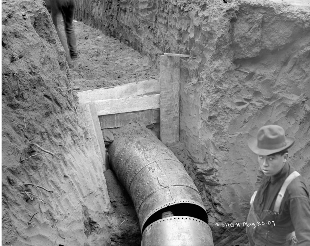
Figure 4-5. 30-inch Pilarcitos Pipe Preparation of a Riveted Joint (1907)
