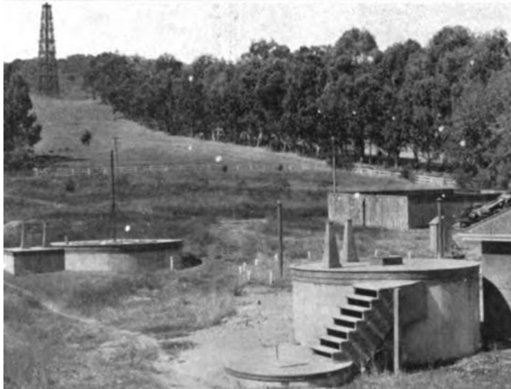
Figure 4.4-8. Belmont pump station works and standpipe (Schussler, 1909)
