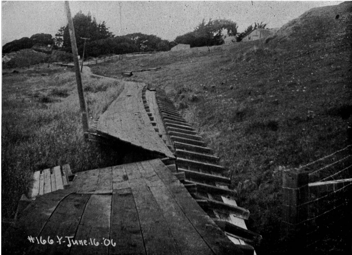
Figure 4.1.12-11. Failure of Stone Dam Flume, Looking Northerly (Photo: Schussler 1906 HS51)
