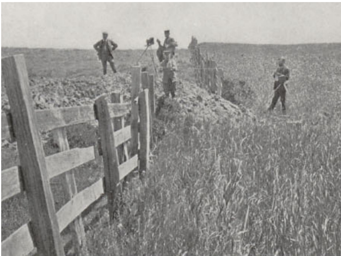
Figure 4.1.9-7 Fence C, View to Southwest (Photo: Lawson 1908 Plate 60C)
