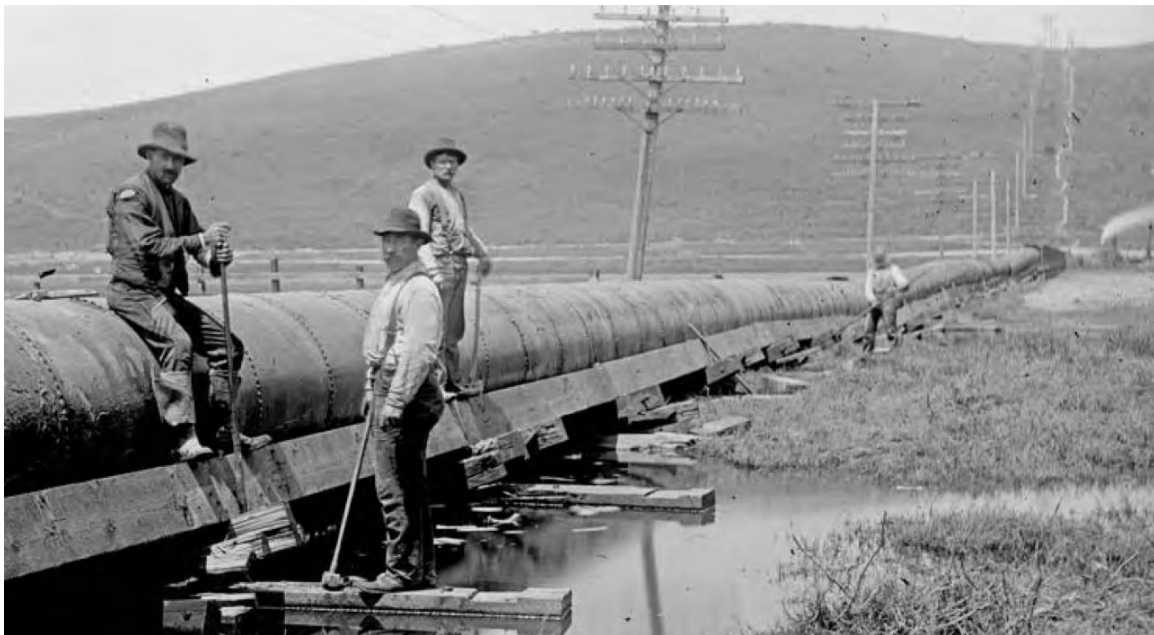
Figure 4.3-17. Crystal Springs Pipeline after the 1906 Earthquake, through San Bruno Marsh (Photo: SFPUC)
