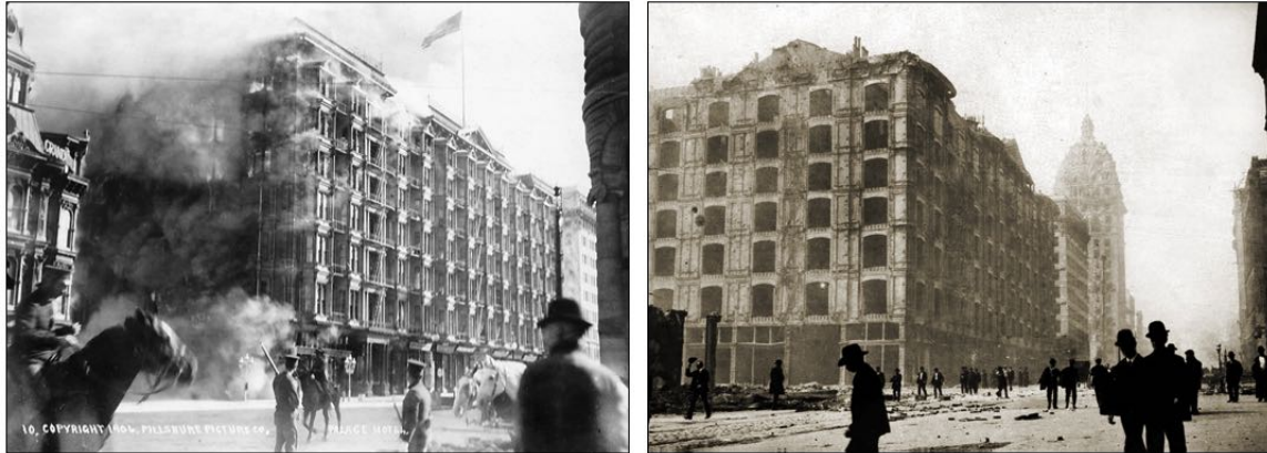
Figure 7-24. Left. April 18 By 2:30 pm. Left photo identified as copyright 1906. Right: after fire. Source: http://thepalacehotel.org
