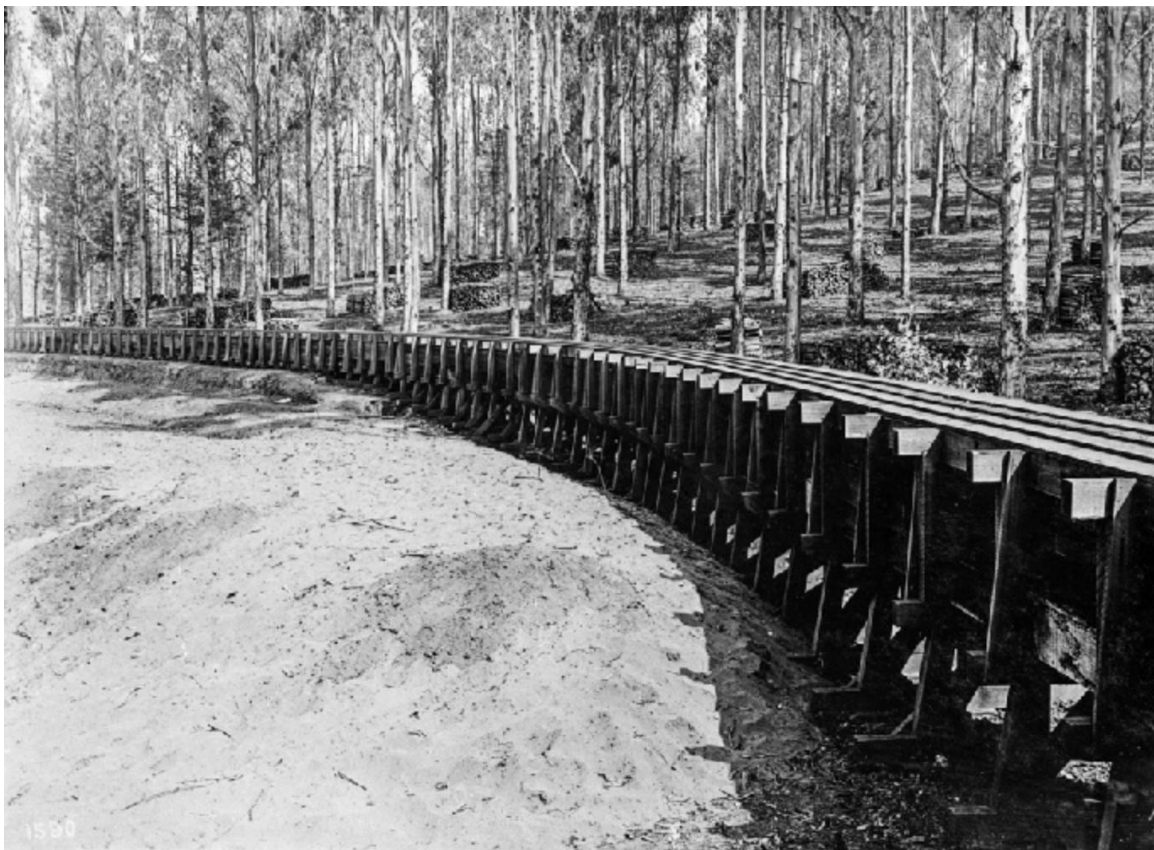
Figure 2-18. Pilarcitos Flume 1913. Looking north, near Ocean Avenue (Credit SF Library, dpwbook6 dpw 1590)
