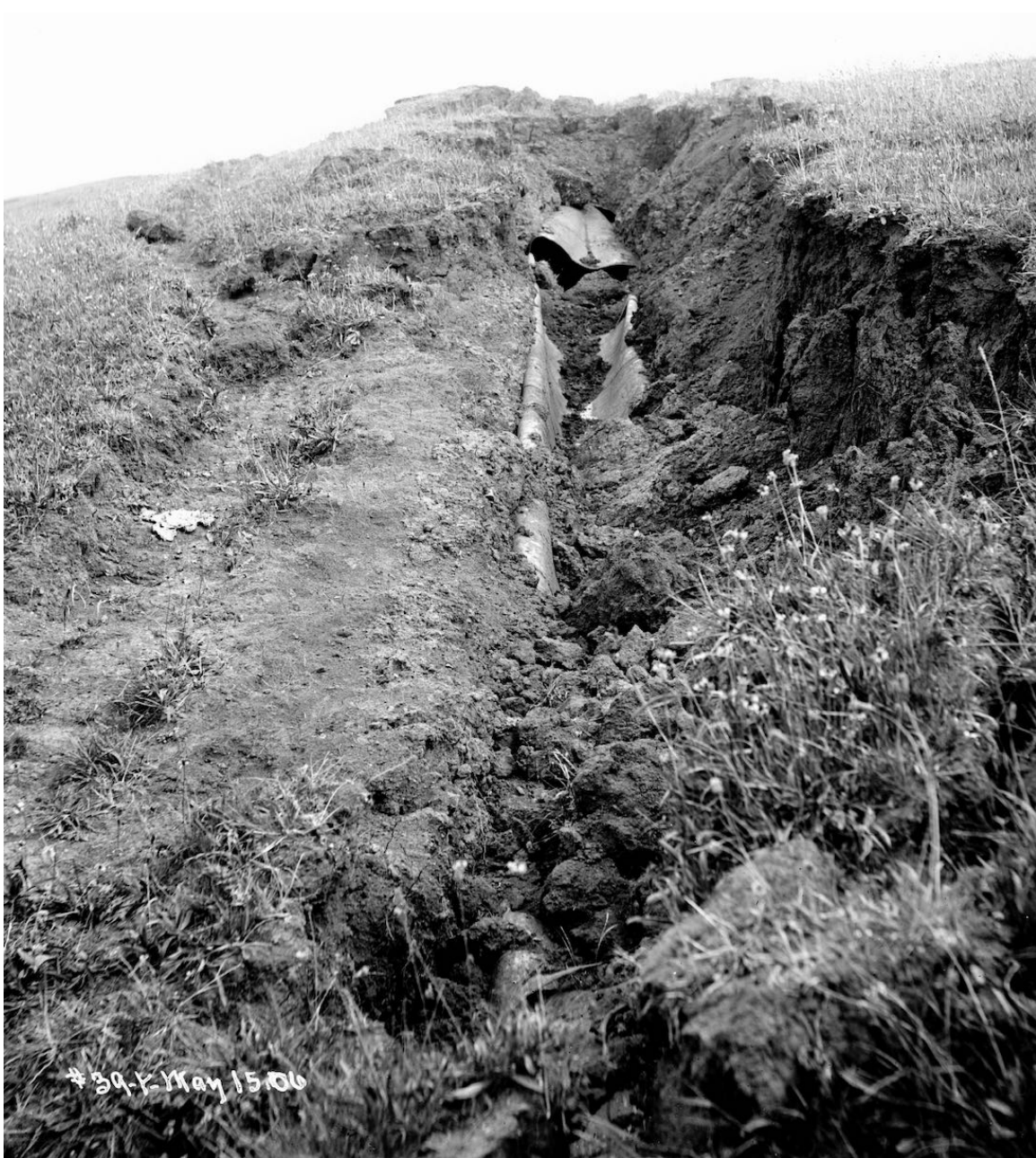
Figure 4.1.3-1. Failure of Pilarcitos 30 inch pipeline about 220 yards south of FX-1. Pipe is collapsed on itself. Looking southerly. (Photo: Schussler 1906, HS-4)
