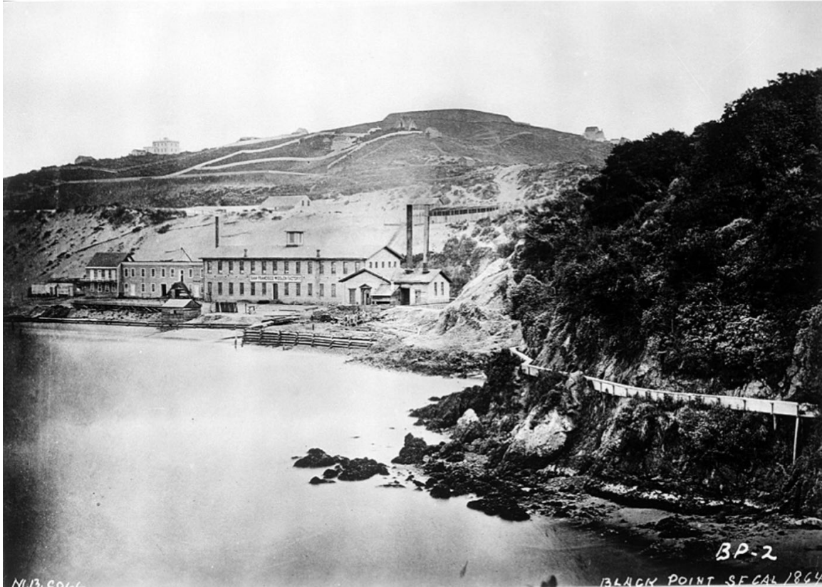
Figure 2-11. Black Point Pump Station and Lobos Flume, c. 1864. (Credit: GGNRA Archives)
