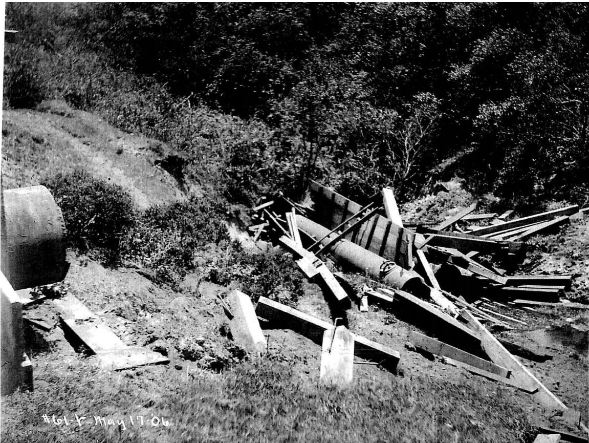
Figure 4.1.1-2. Large Frawley Canyon. View downstream, looking easterly. Pipe on left side is original Pilarcitos pipe at the north edge of the canyon. (Photo: Schussler 1906, HS9)
