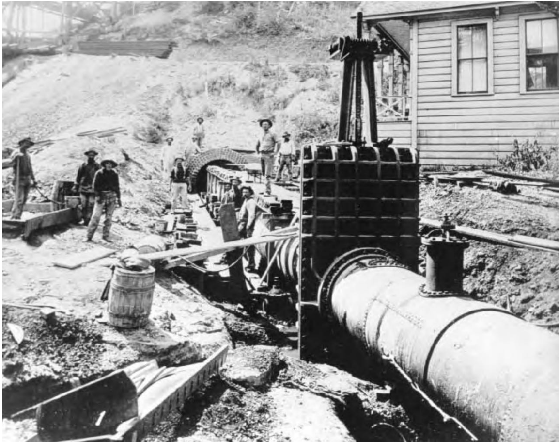
Figure 4.3-1. Crystal Springs 44" Pipeline and Gate Valve, At Lower Crystal Springs Dam outlet works, 1888. Note restrained slip joint in lower right of photo.
