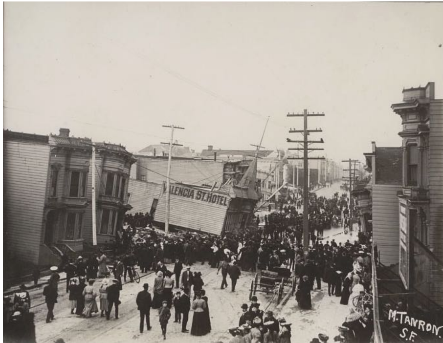
Figure 7-42. April 18 am. Collapse of Valencia Street Hotel (Photo credit Marcel Tanron, Camera Craft, Vol, 27 1921, Online Archive of California, The 1906 San Francisco Earthquake and Fire Digital Collection, U. C. Berkeley, Bancroft Library)
