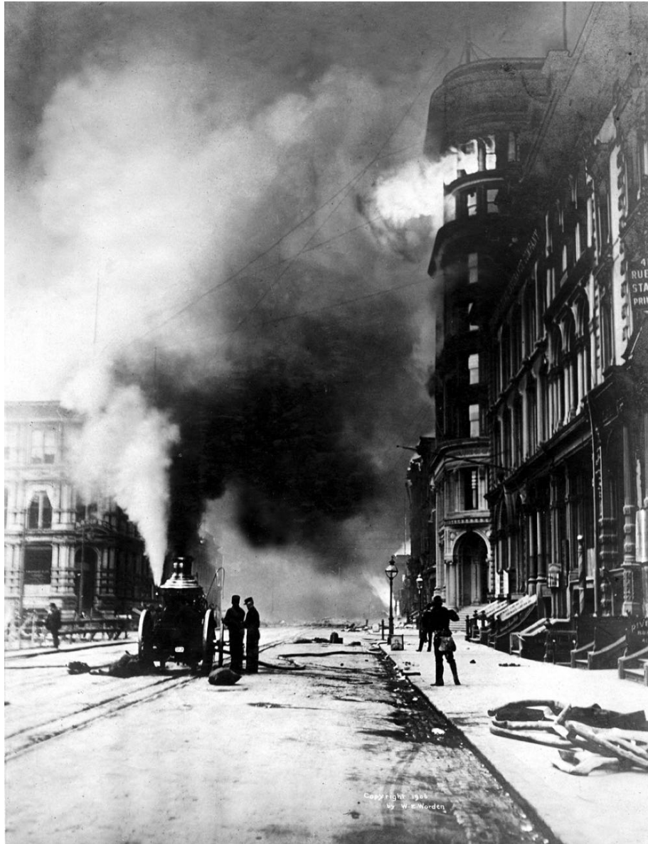
Figure 7-26. April 18 pm. California Street, between Sansome and Market. (Photo: W. E. Warden, 1906)
