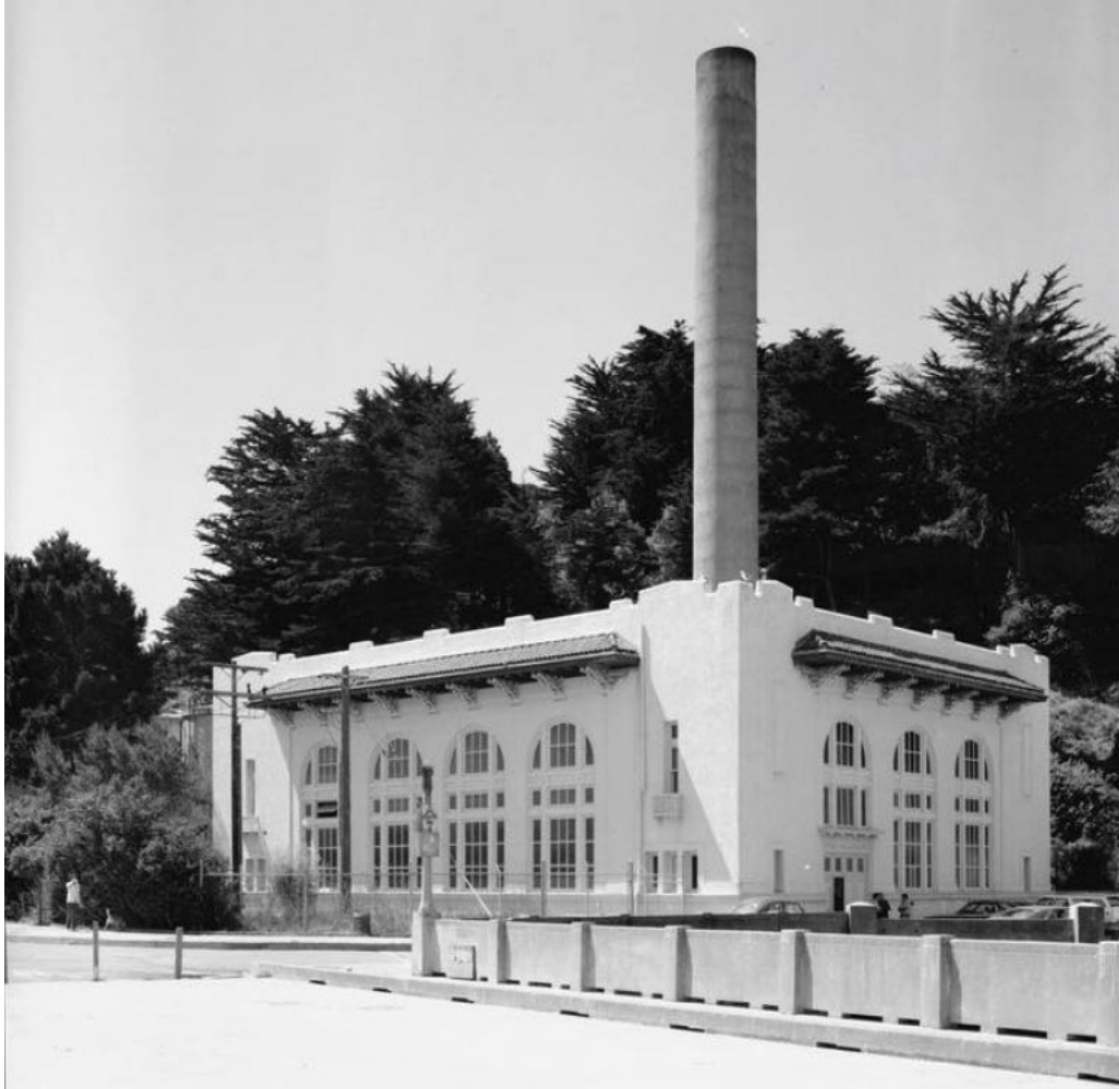
Figure 8-5. AWSS Pump Station 2, c. 1912 (photo: Manson)
