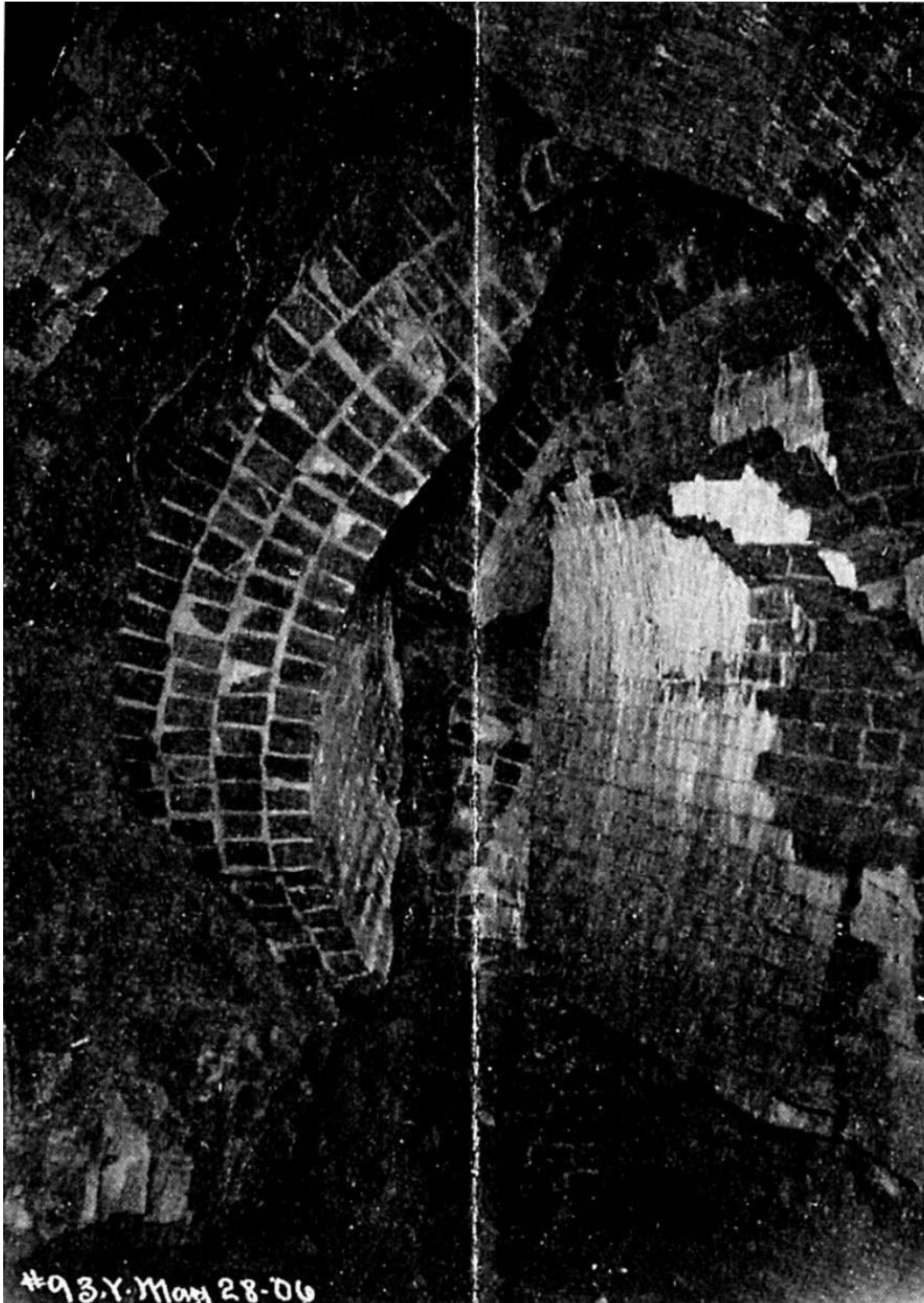
Figure 4.1.12-2. Wastewater Tunnel looking northerly (photo: Schussler 1906)
