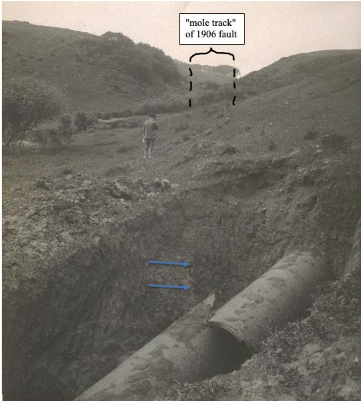
Figure 4.1.6-5. Crossing FX-3. Looking northwesterly along trace of 1906 fault rupture. Failure of Pilarcitos 30 inch pipeline. (Photo: ASCE 1907, p 16)
