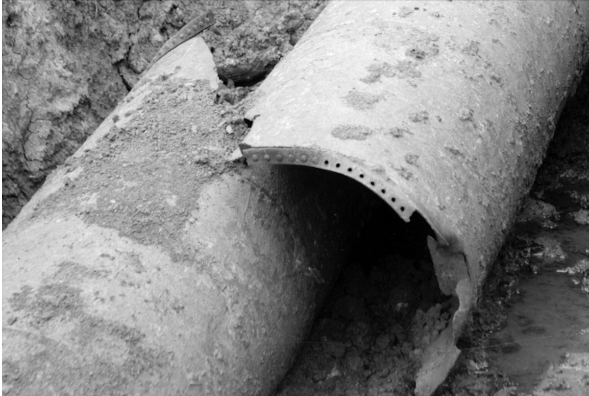
Figure 4.1.6-3. Closeup of Figure 4.1.6-2 showing rivets.
