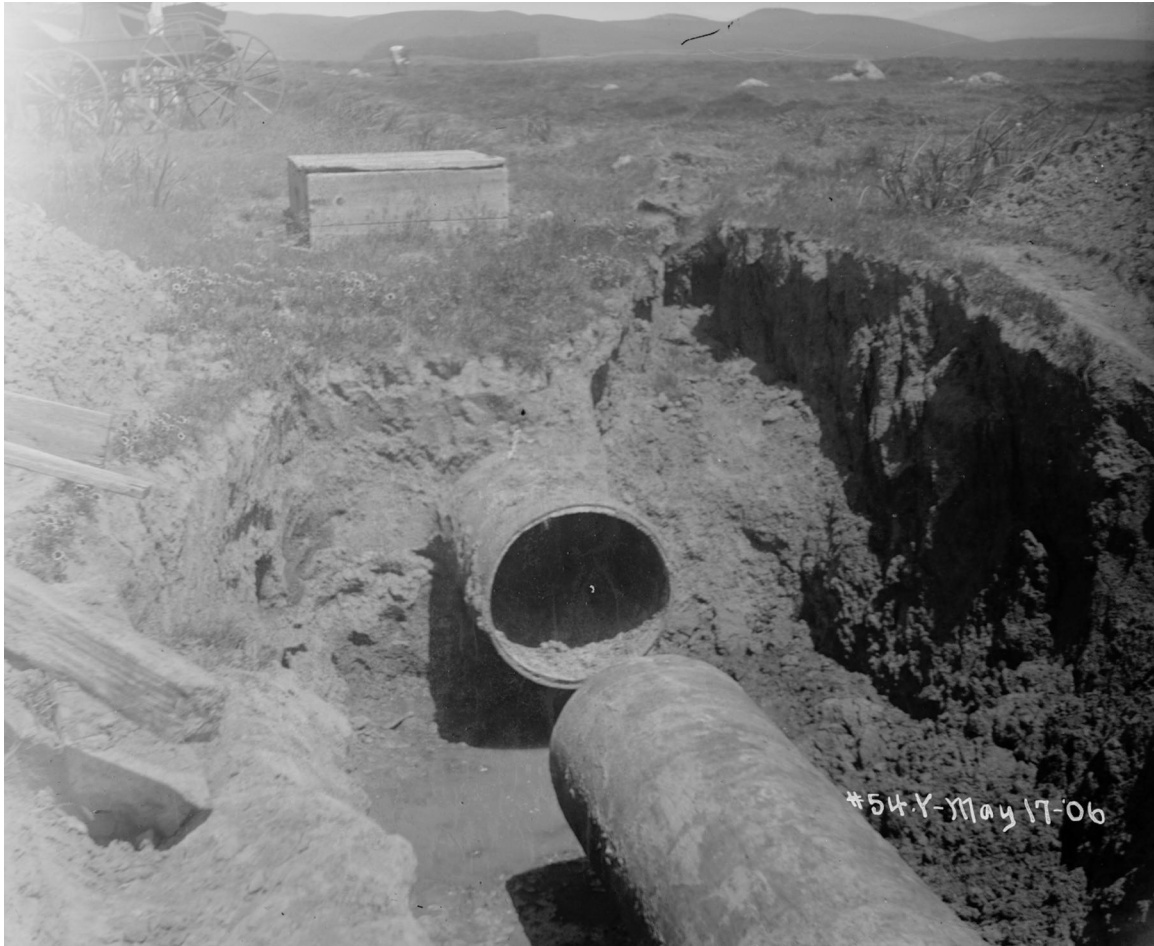
Figure 4.1.8-2. FX-4. Failure of Pilarcitos 30 inch pipeline. At north end of San Andreas Reservoir. Looking Northwesterly. Pull Apart ~59". North segment of pipe is ~4" to the right (transverse) of the south segment. The wood box seen in this photo encapsulates a valve, and is so-marked in Figure 4.1.8-3; it is the same wood box seen in Figures 4.1.9-4 and -5. (Photo: Schussler HS7 1906)
