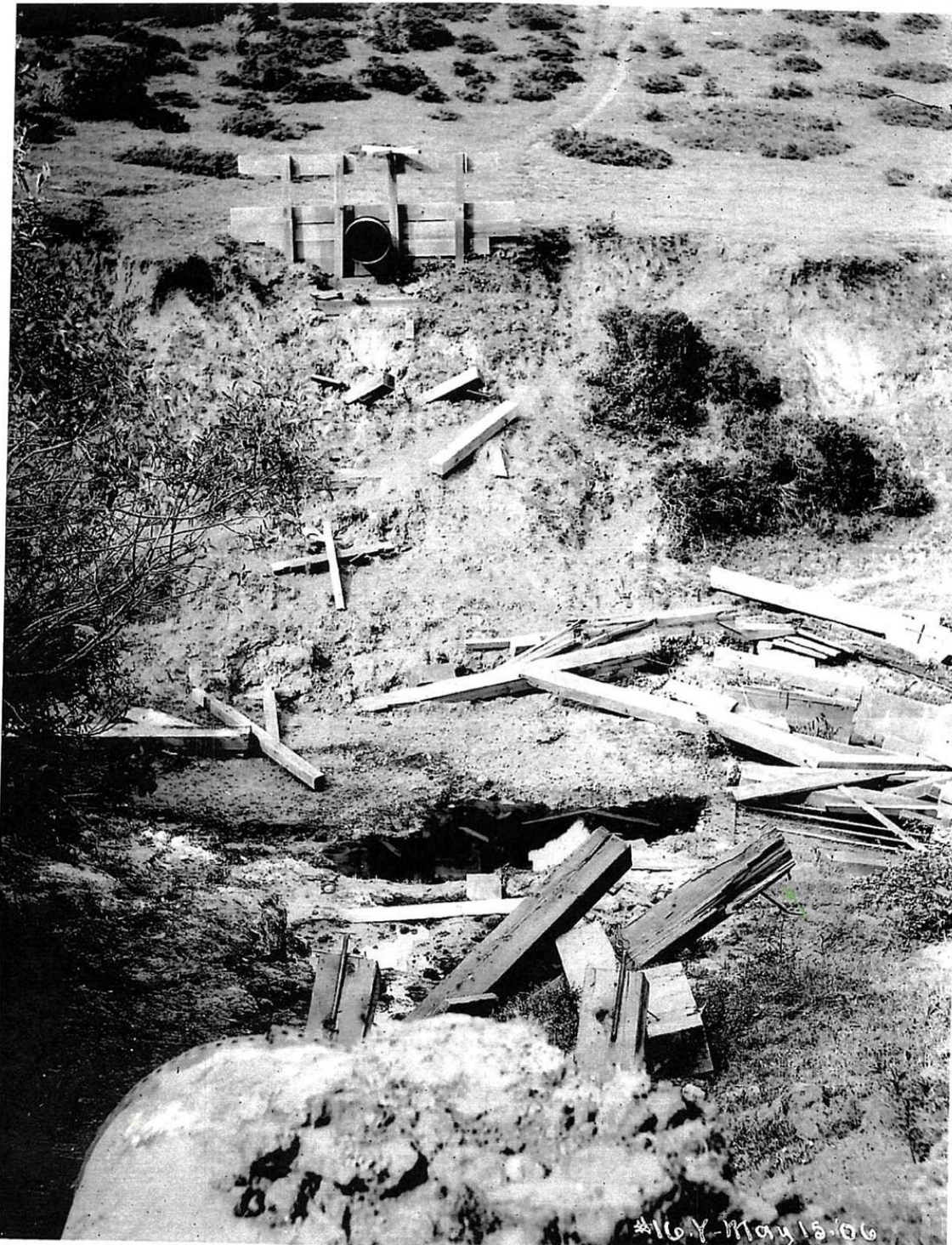
Figure 4.1.1-1. Large Frawley Canyon. Destruction of heavy bridge and 30-inch Pilarcitos pipe over Large Frawley Canyon. The pipe was torn in three locations and thrown sideways over 50 feet to the east into the canyon below. View looking northerly. (Photo: Schussler 1906, HS8)
