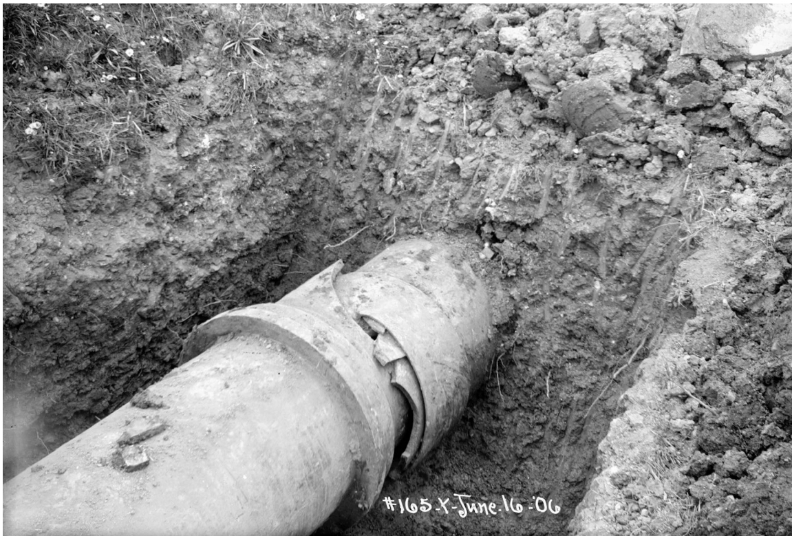
Figure 4.1.14-5. FX-5. 24" Pipe has telescoped \pm 1' . About 100' north of FX-5. (Credit: Schussler 1906 HS13)
