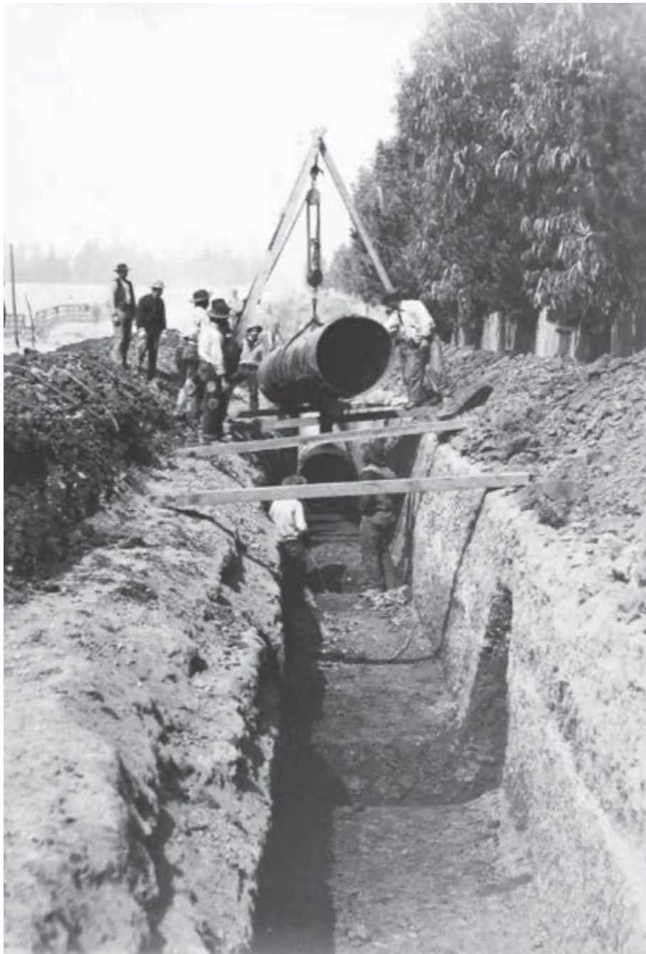
Figure 4.3-2. Crystal Springs 44" Pipeline Being Installed, El Camino Real, 1888 (Journal of the San Mateo County Historical Association, Volume xlv, No. 1, 2018)
