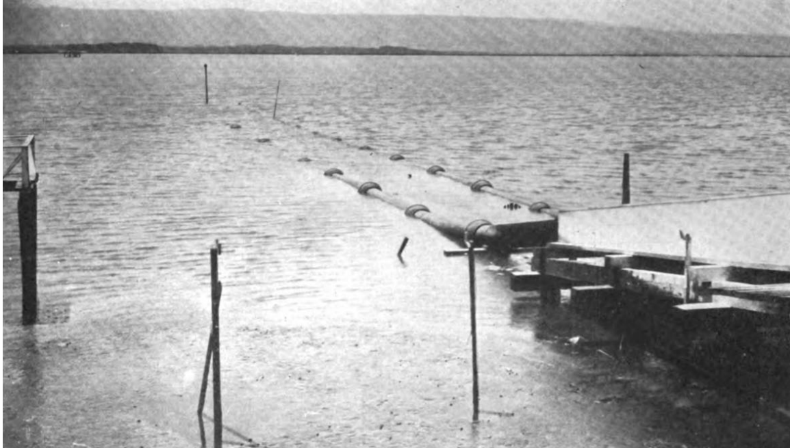
Figure 4.4-5. Twin 16" submarine pipes at the west shore of San Francisco Bay, Looking Easterly (Schussler, 1909)
