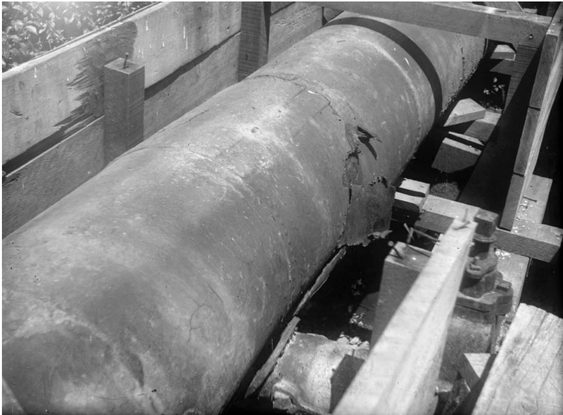
Figure 4.1.7-3. South of FX-3. Pipe has telescoped on the bridge. Looking southerly. (Photo: SVWC 1906)
