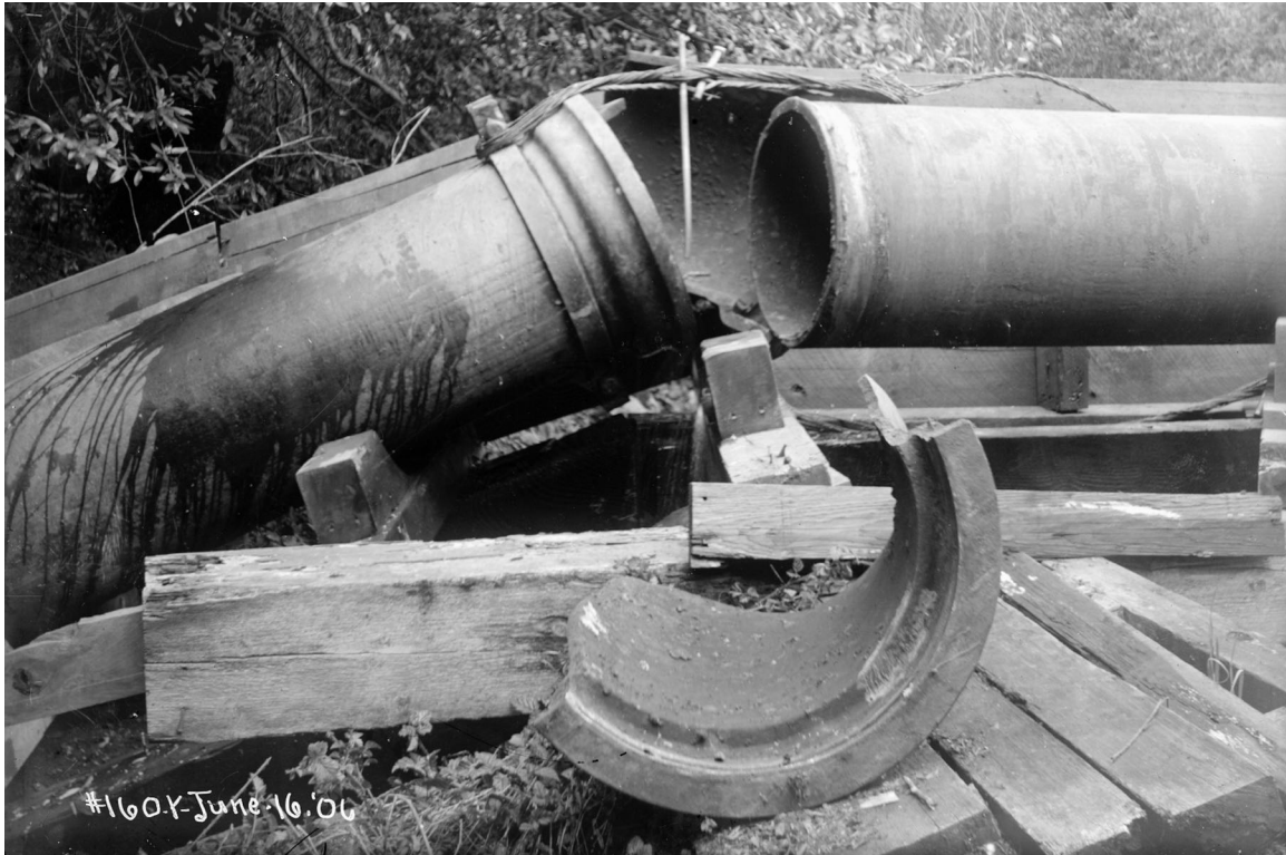
Figure 4.1.14-3. Crossing 5. 24" Pilarcitos Cast Iron Pipe. Elbow crushed. View looking north. (Photo: Schussler 1906 HS11)
