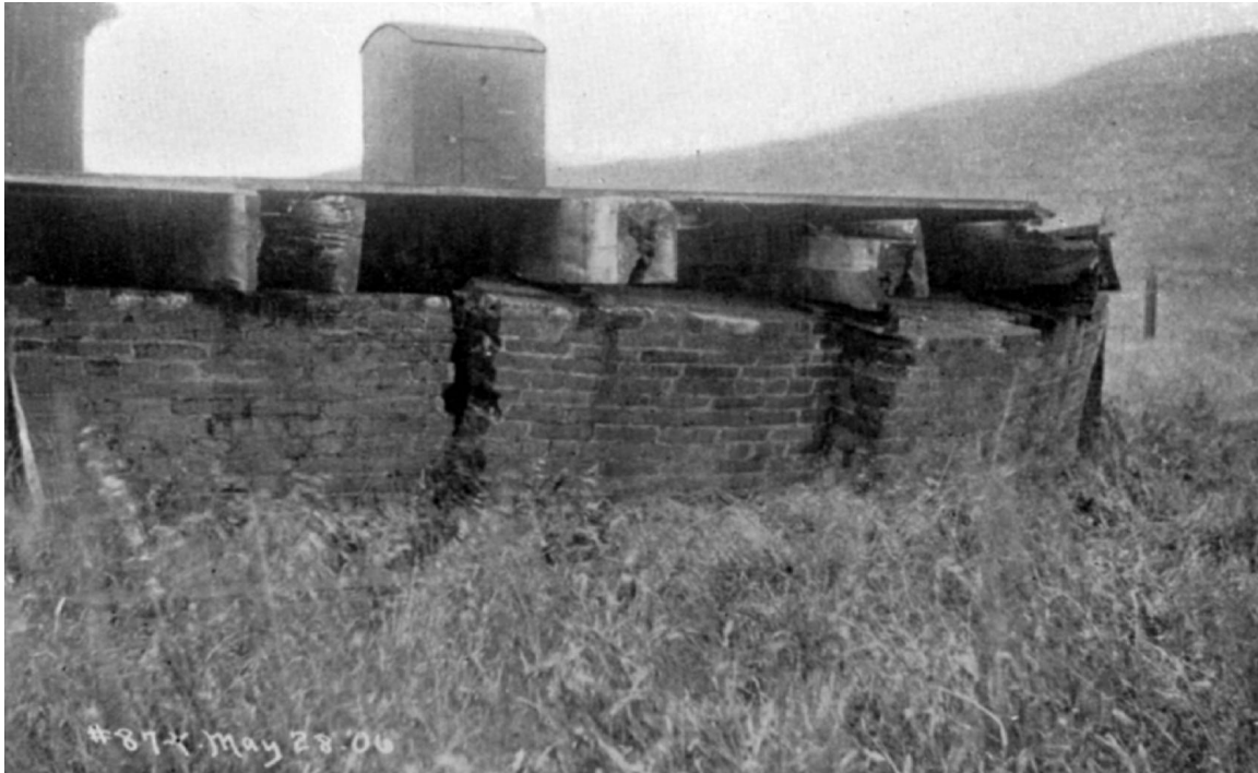
Figure 4.1.10-6. Brick forebay damage (view looking northerly) (Photo: Schussler)
