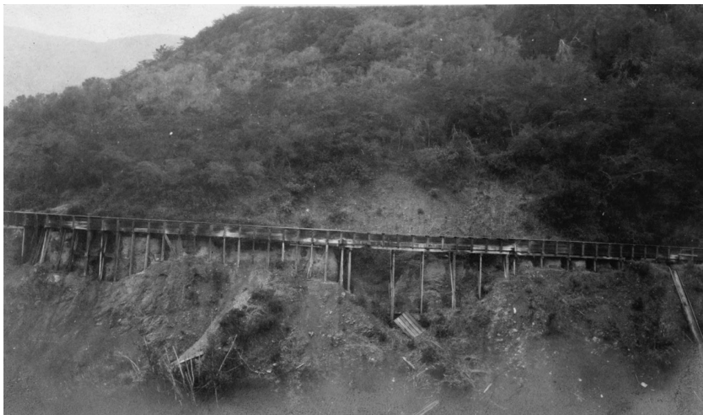
Figure 4.6-7. Repair of Flume. (Photo: SVWC).
