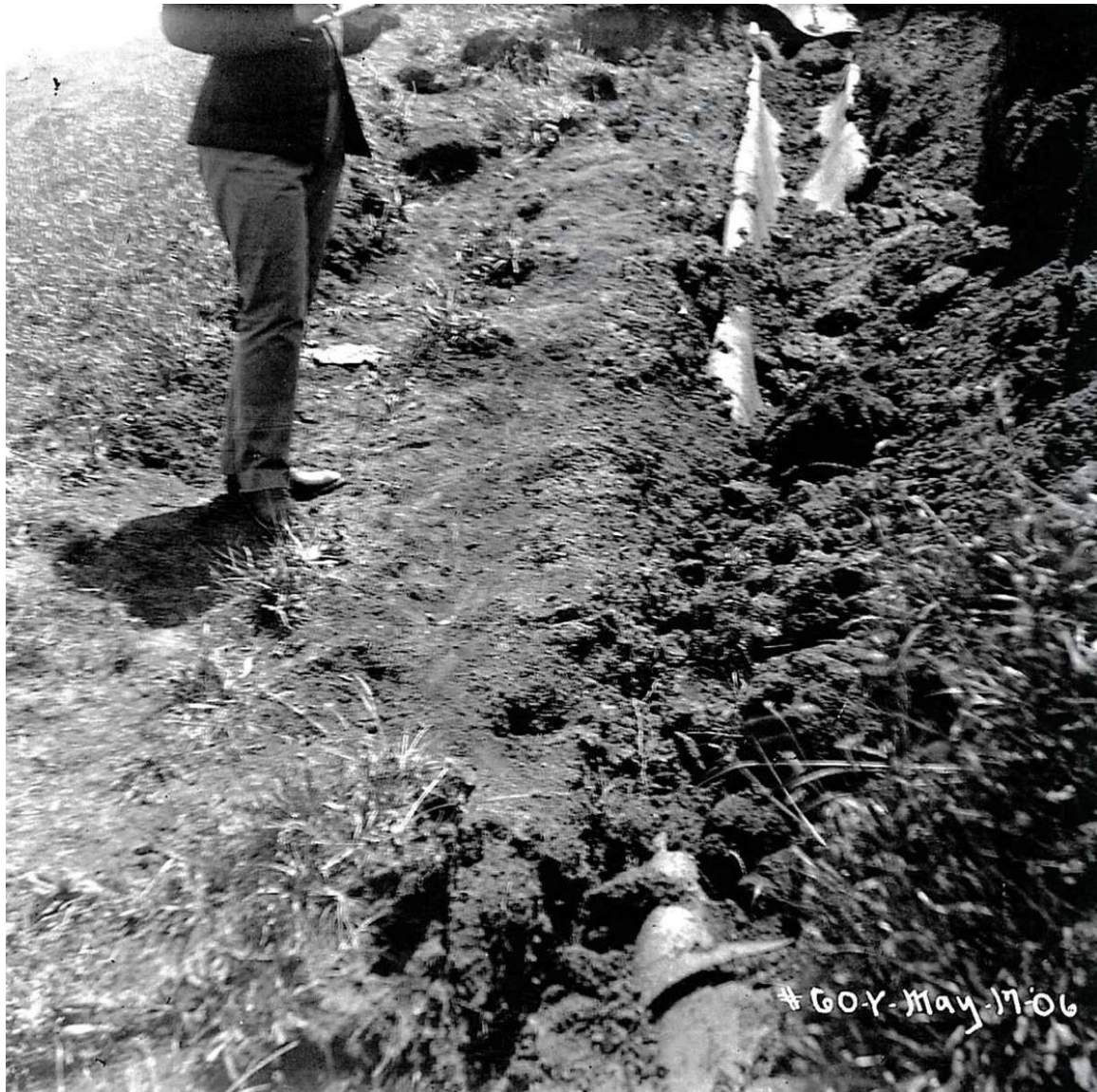
Figure 4.1.3-2. Failure of Pilarcitos 30 inch pipeline about 220 yards south of FX-1. Pipe is collapsed on itself. Looking southerly. (Photo: Schussler 1906)
