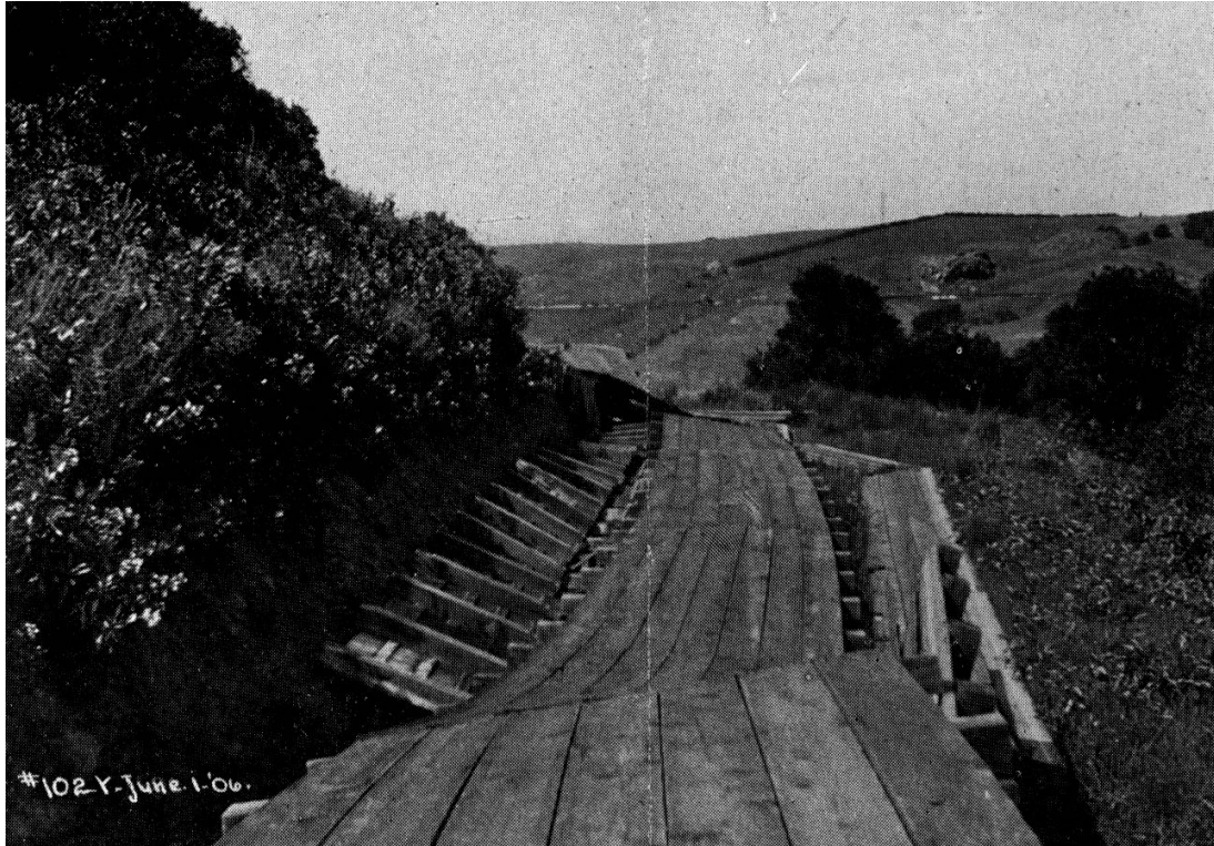
Figure 4.6-3. Failure of Pilarcitos Waste Water (Side) Flume to San Andreas Reservoir, Looking Northerly (Photo: Schussler 1906 HS47)
