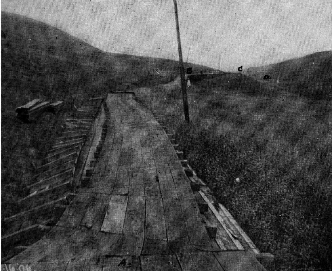
Figure 4.1.12-12. Failure of Stone Dam Flume, Looking Southerly (Photo: Schussler 1906 HS49)
