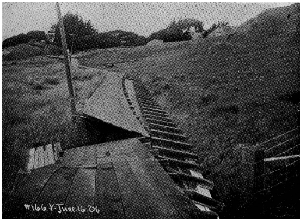
Figure 4.1.12-13. Failure of Stone Dam Flume, Looking Northerly (Photo: Schussler 1906 HS51)
