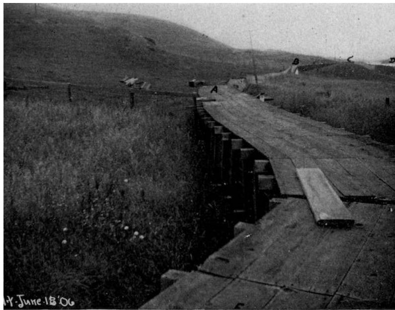
Figure 4.1.12-11. Failure of Stone Dam Flume, Looking Southerly (Photo: Schussler 1906 HS50)
