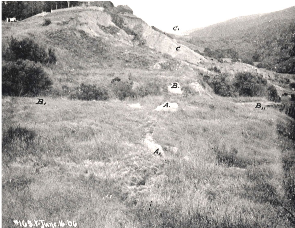
Figure 4.1.12-1. San Andreas Fault Track through A 1 – A – B – C – C 1 ). Dotted line B I – B II is the alignment of the buried wastewater tunnel outlet. Looking Southeasterly (Credit: Schussler HS31)
