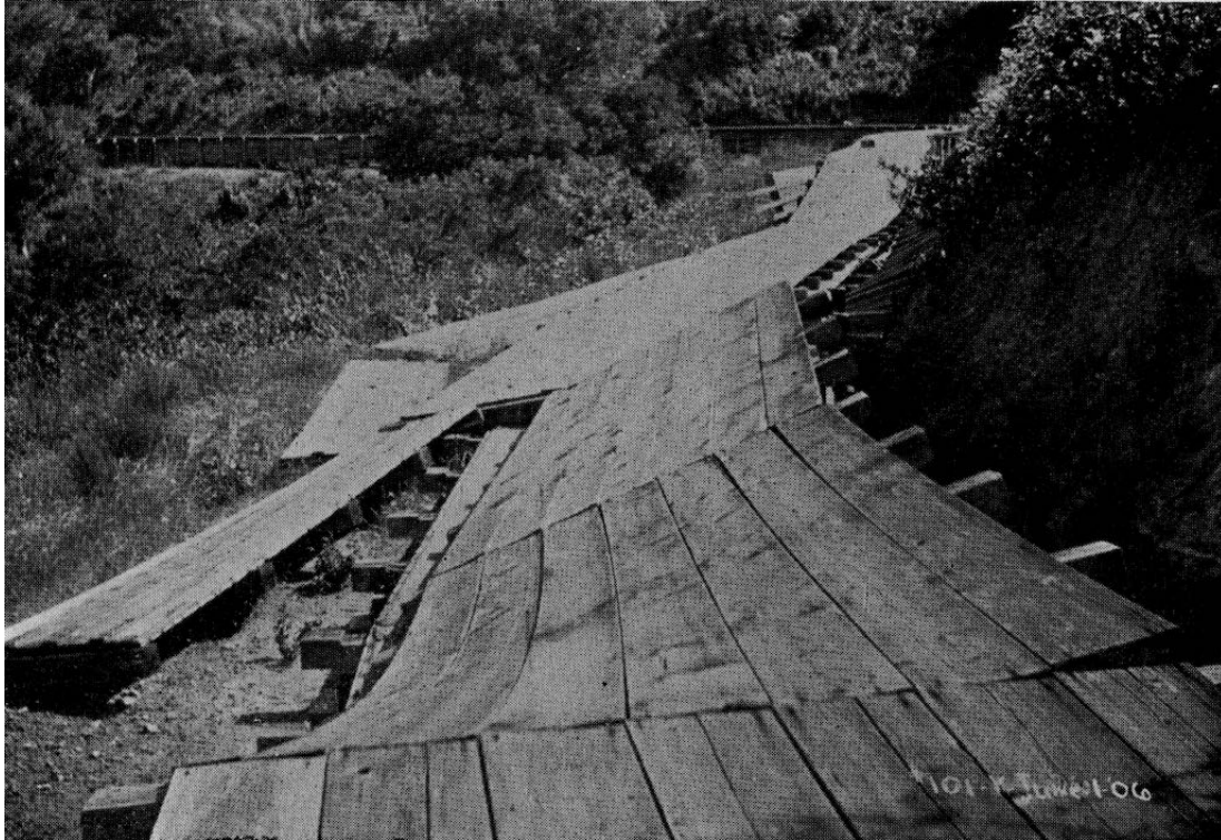
Figure 4.6-4. Failure of Pilarcitos Waste Water (Side) Flume to San Andreas Reservoir, Looking Southerly (Photo: Schussler 1906 HS48)
