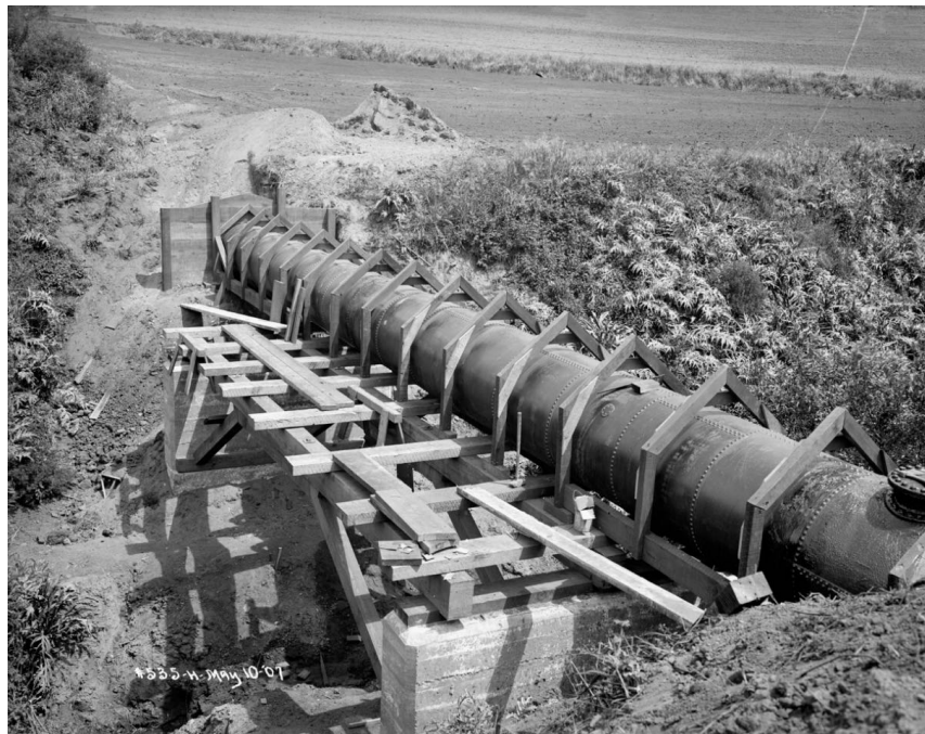
Figure 4-4. Construction of the Baden-Merced 30-inch Pipe at Creek Crossing (using former Pilarcitos Pipe segments) (SVWC 1907)
