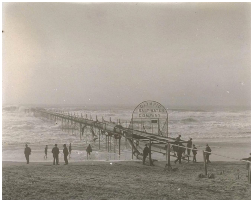
Figure 2-13. Salt Water Intake Pipe (Bancroft Library)
