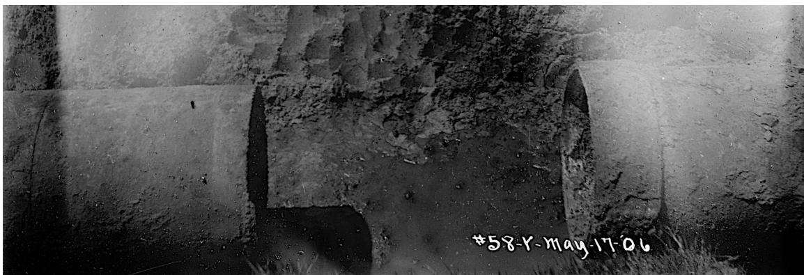
Figure 4.1.8-5. Crossing 4. Failure of Pilarcitos 30 inch pipeline at the main trace. Looking Westerly (Photo: SVWC 1906)
