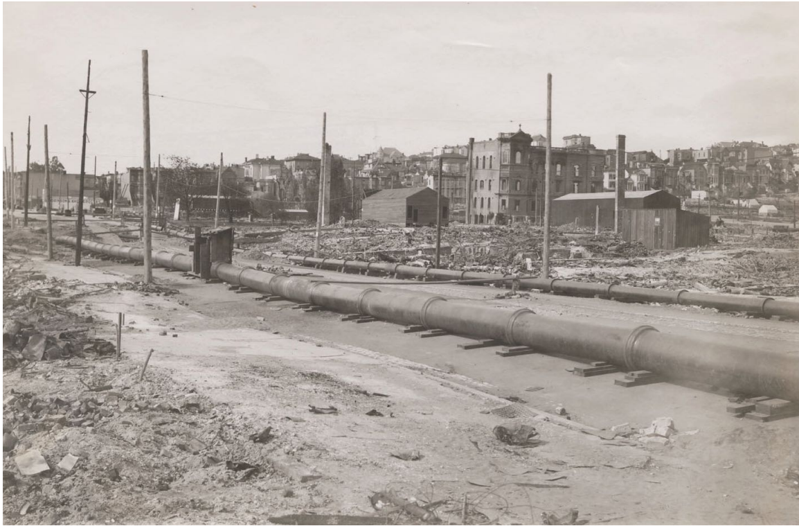
Figure 7-49. c. May 16 1906. View of Valencia Street between 18 th and 19 th street, looking southwesterly. The two temporary pipes are cast iron with belled joints; no restraints are seen placed across the segmented joints. Each segment is typically supported by two sets of wooden planks. (Photo credit: Online Archive of California, The 1906 San Francisco Earthquake and Fire Digital Collection, U. C. Berkeley, Bancroft Library)
