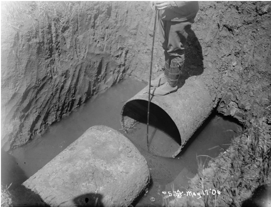
Figure 4.1.8-6. Site 8. FX-4N. Failure of Pilarcitos 30 inch pipeline. Pull Apart ~ 21.5 inches. (Photo: Schussler HS3 1906)
