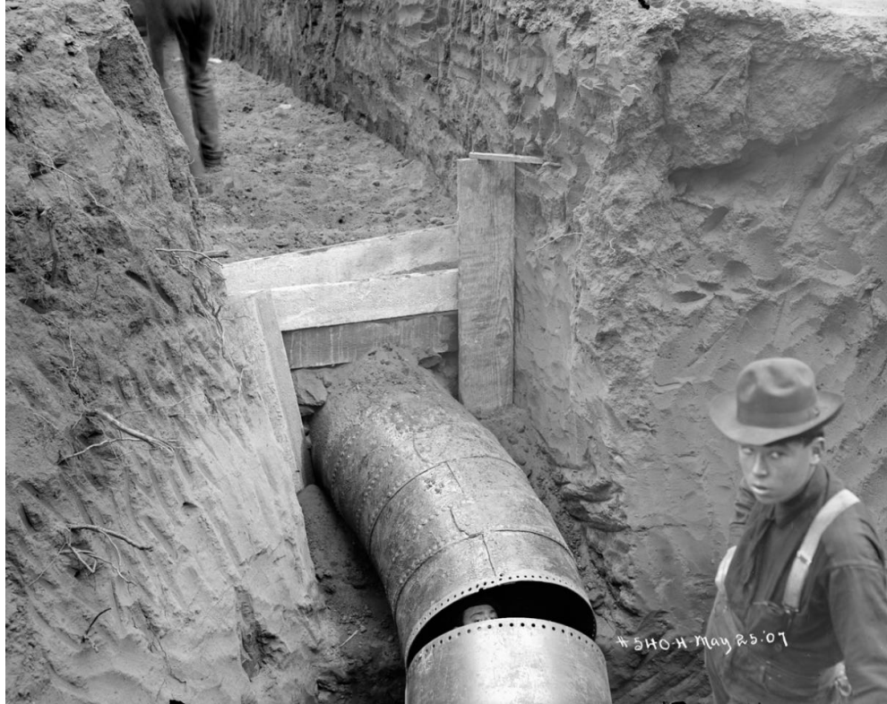
Figure 4-5. 30-inch Pilarcitos Pipe Preparation of a Riveted Girth Joint (SVWC 1907)
