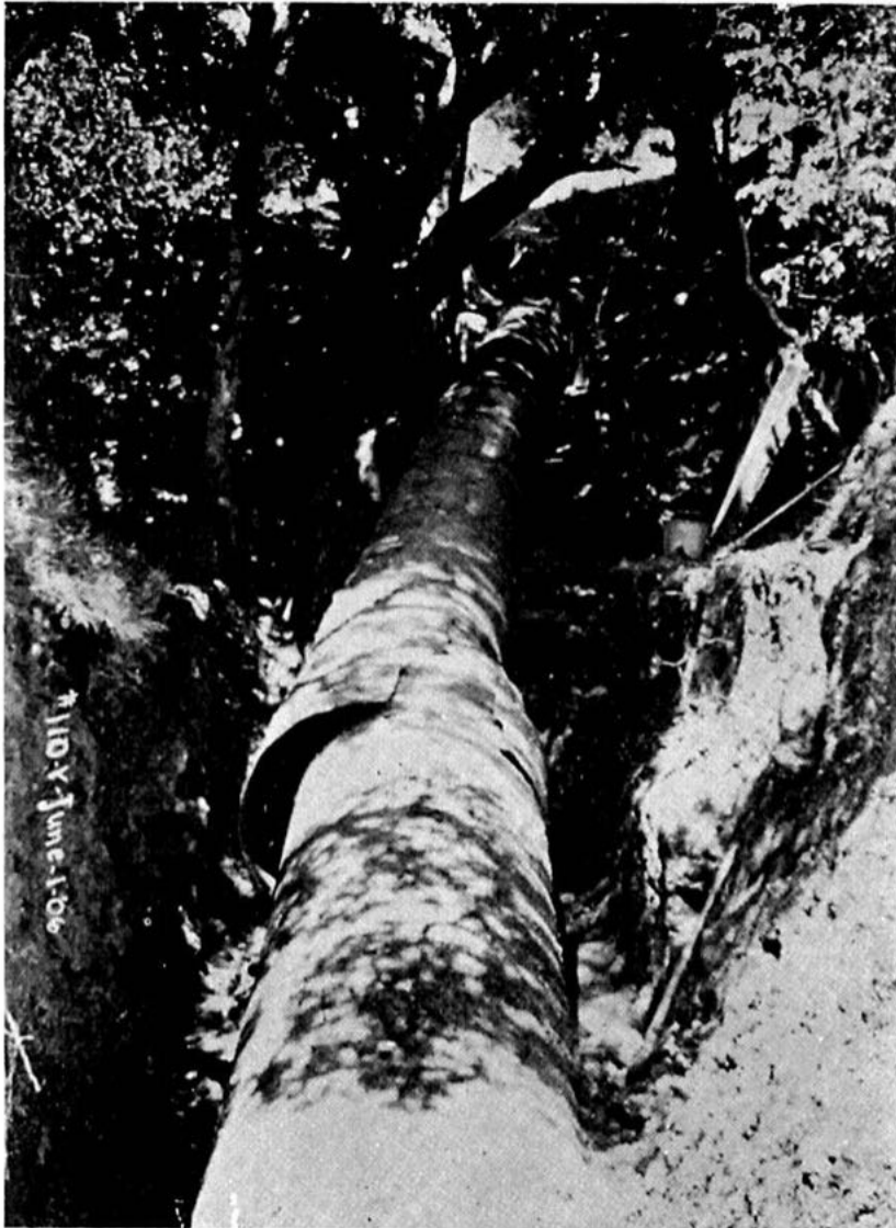
Figure 4.1.17-3. FX-6. Locks Creek 37.5" Wrought Iron Pipe is offset to the north about 14" and telescoped about 51". Looking easterly. Location is about 50 feet east of the County road between the San Andreas and Crystal Springs reservoirs. (Photo: Schussler 1906 HS14)
