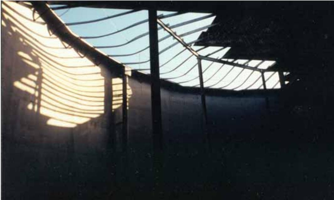
Figure 13. Damaged Roof Rafters
