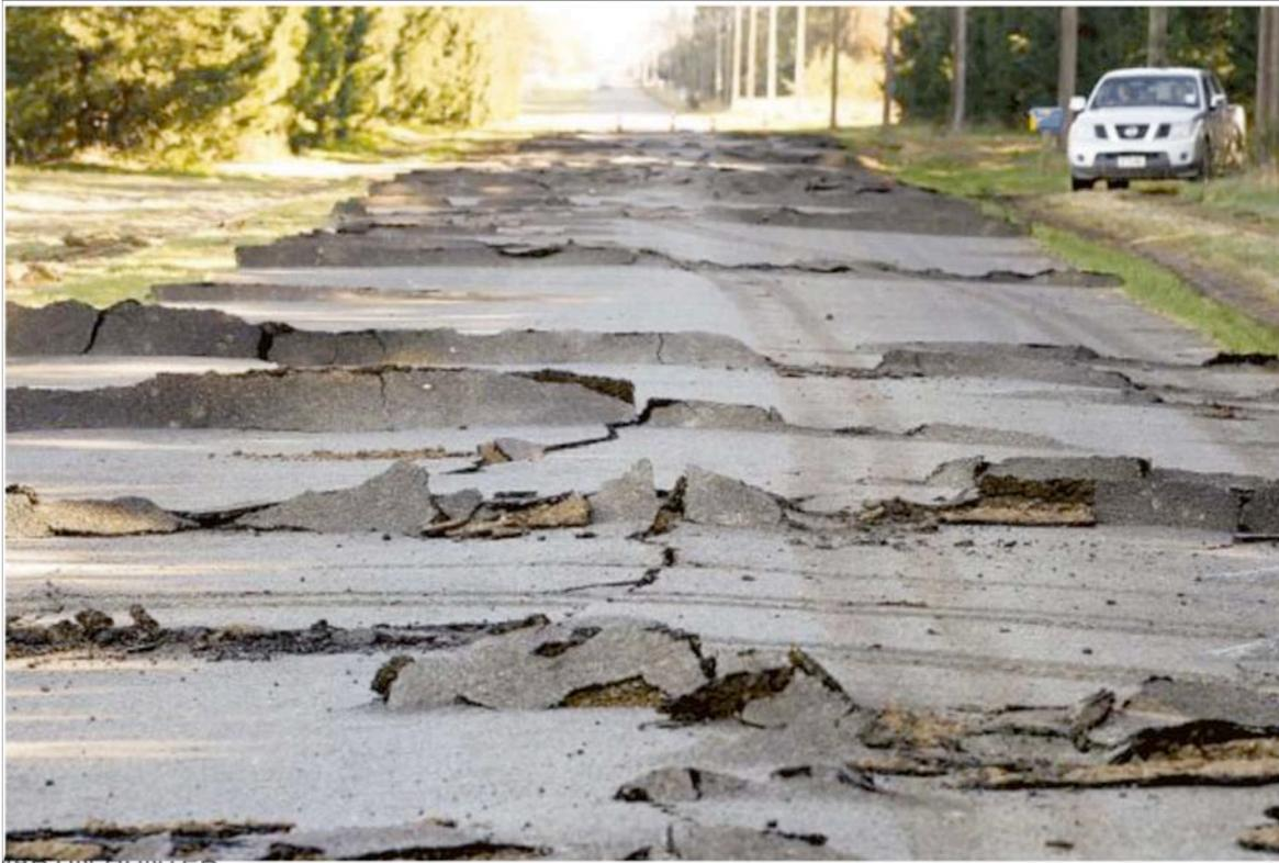
*Figure 9. Fault Offset Through a Road*
