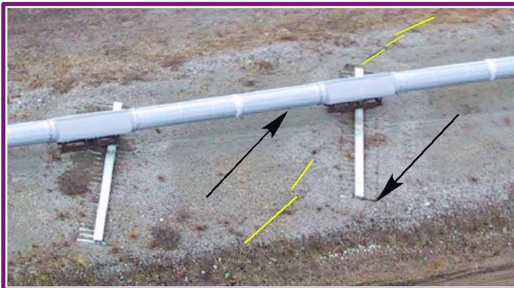
*Figure 3.11. Location of Surface Fault Rupture (Alyeska)*
