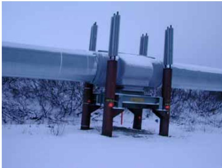
*Figure 3.5. Four-legged anchor support.*
