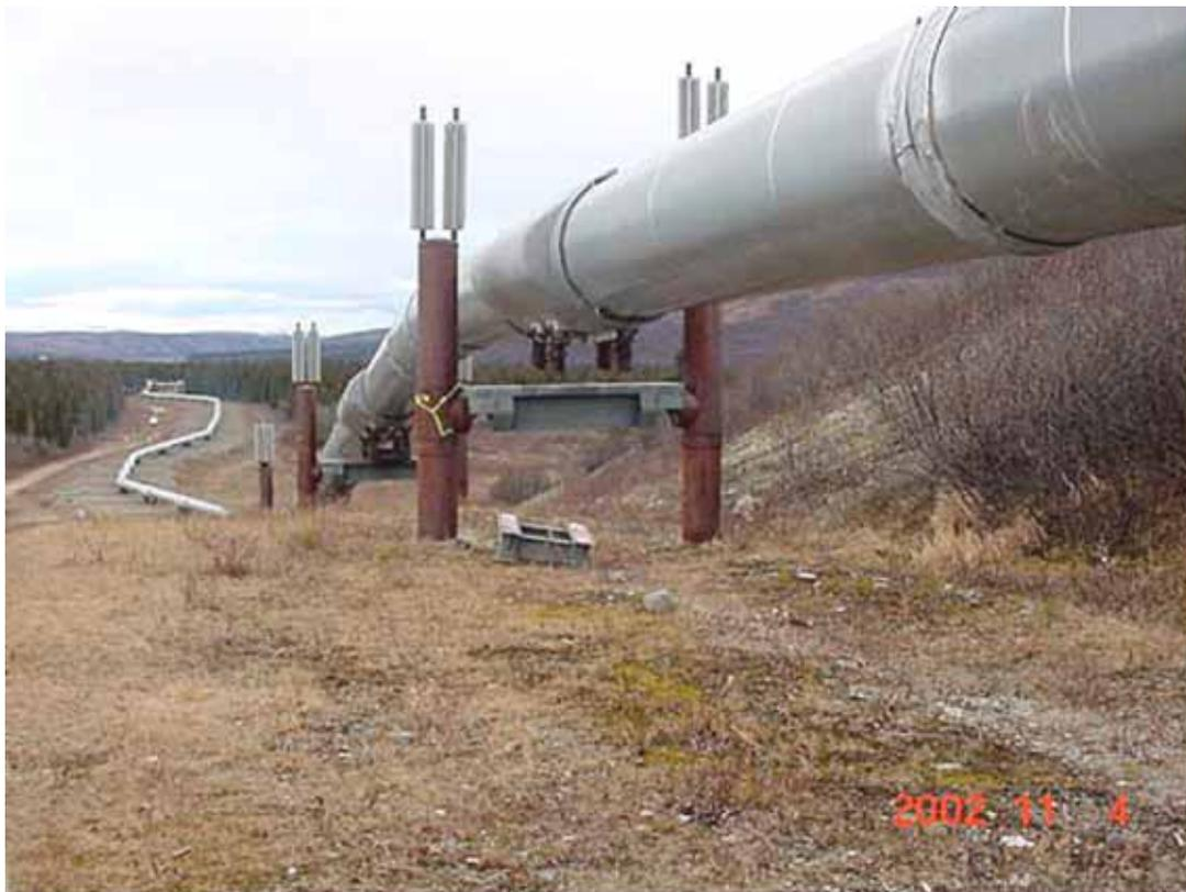
Figure 3.13. Dropped Shoe on elevated portion at north end of Fault Crossing Zone (Alyeska)
