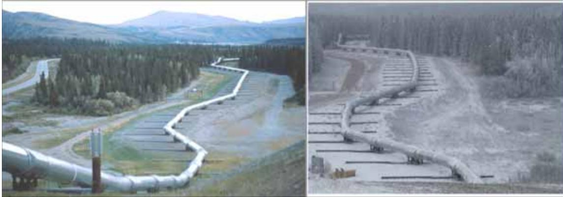
*Figure 3.16. TAPS pipeline, before (left image) and after (right image) earthquake*
