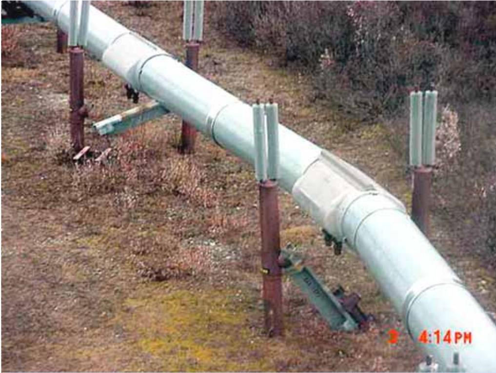
*Figure 3.14. Consecutive fallen beams leaving pipeline unsupported for three spans (Alyeska)*
