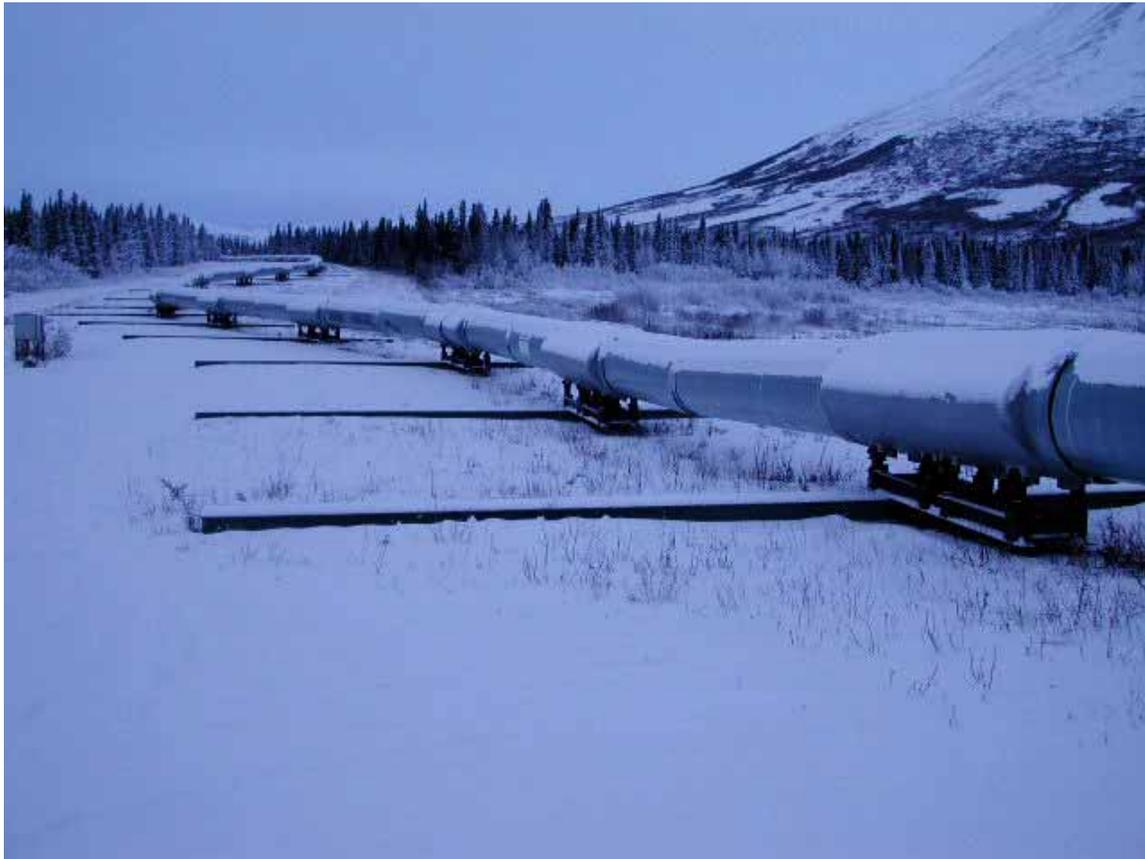
*Figure 3.8. Concrete 'sleepers' supporting pipeline in fault crossing zone (post-earthquake)*
