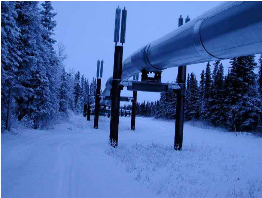
*Figure 3.7. Raised pipeline to allow work pad to cross underneath.*
