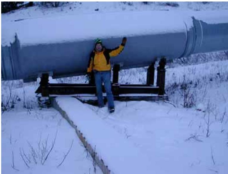
*Figure 3.15. Perched Shoe at end of 'sleeper.'*
