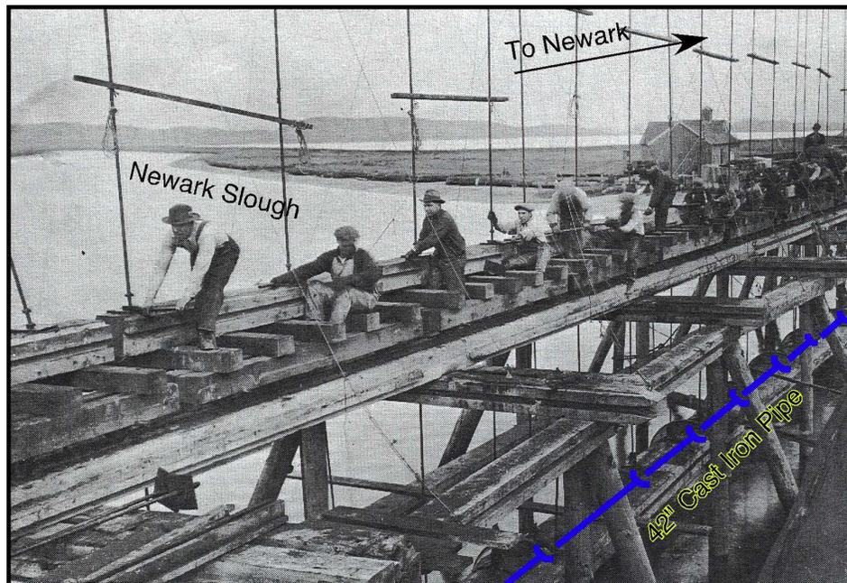
Figure 8. BDPL 1, Installation of 42" CI Pipe, 1924
