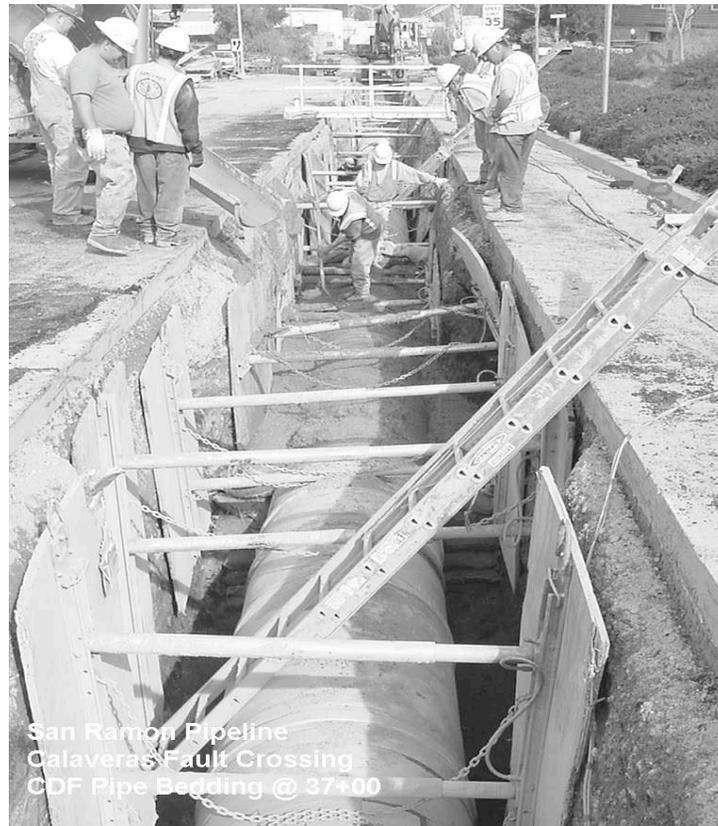
*Photo 1. Placement of CDF Around the Pipeline*
