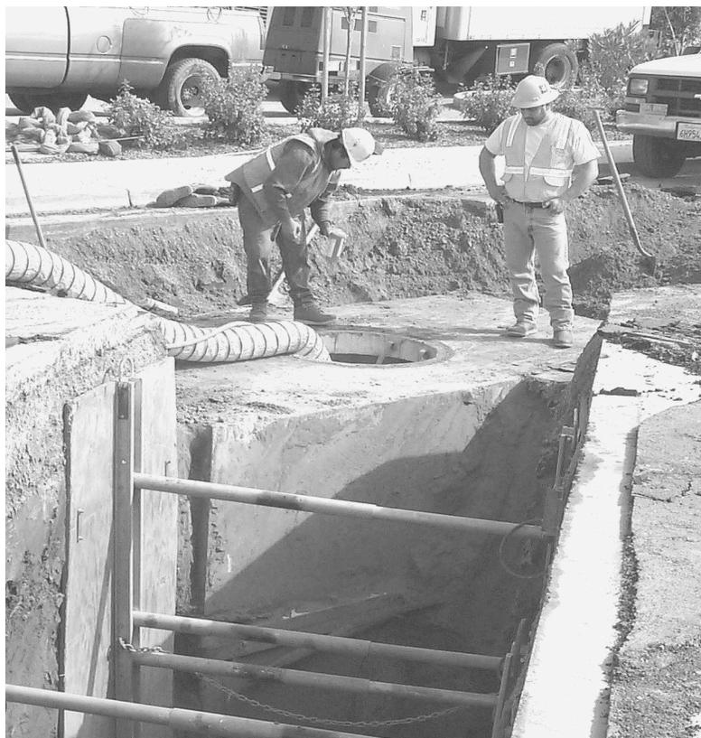
*Photo 2. Large Concrete Vault Discovered in Pipeline Alignment*
