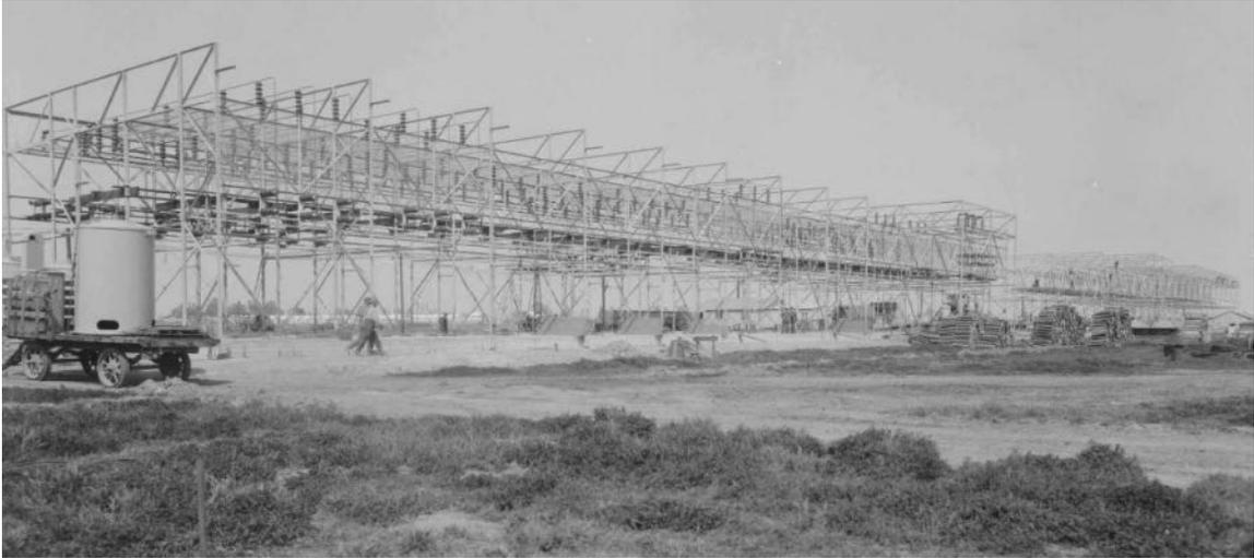
*Figure 2. Lighthiye Steel 66 kV Switchrack (photo dated 1927)*
