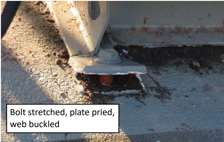
Bolt broke, TR slid ~1 inch, web buckled
