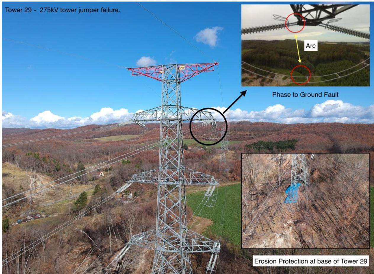
Fig. 8. Tower 29, Line Fault
