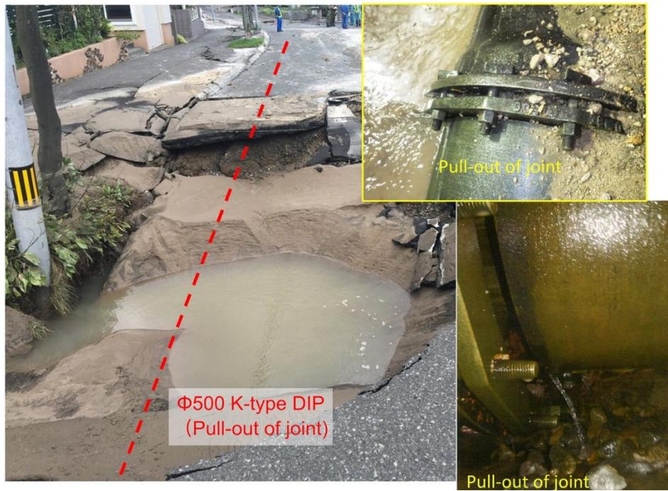
Fig. 10. Pipe Damage in the Liquefaction Zone (credit: Kubota)
