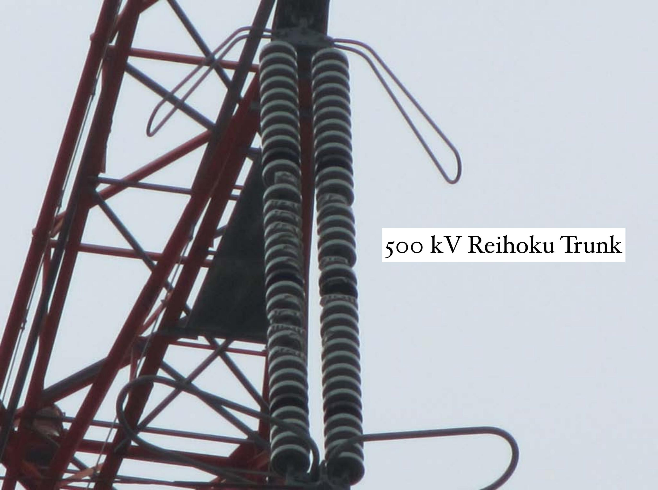
A photograph of a high-voltage power line tower. The tower is a lattice structure of reddish-brown metal. Two large, vertical insulators are mounted on the tower. Each insulator consists of many dark, cylindrical discs stacked on top of each other. The background is a clear, light blue sky. The text "500 kV Reihoku Trunk" is overlaid on the right side of the image.
