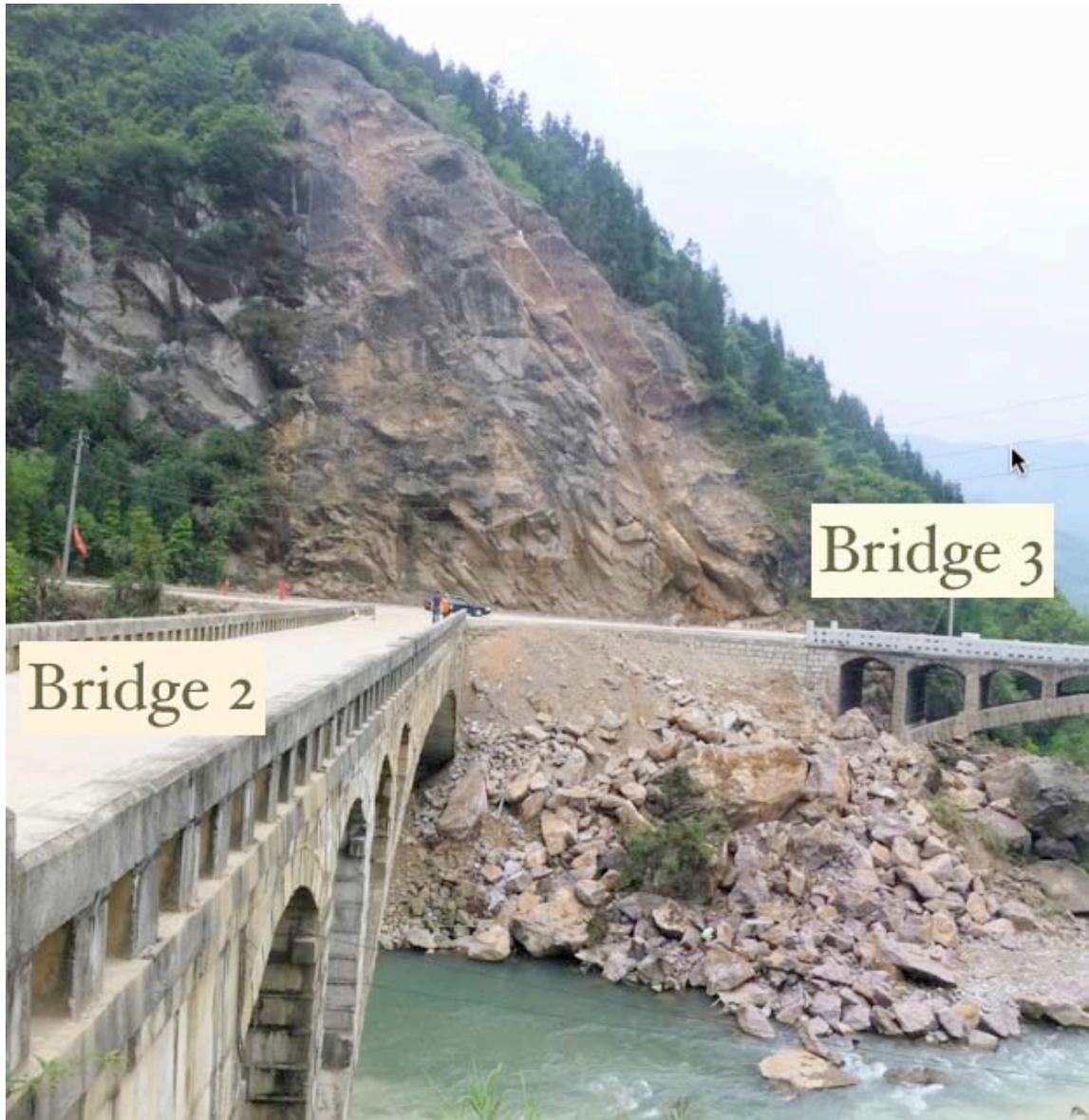
*Figure 7-7. Source Rockfall zone that Impacted Bridges 2 and 3 (photo date May 31, 2013)*
