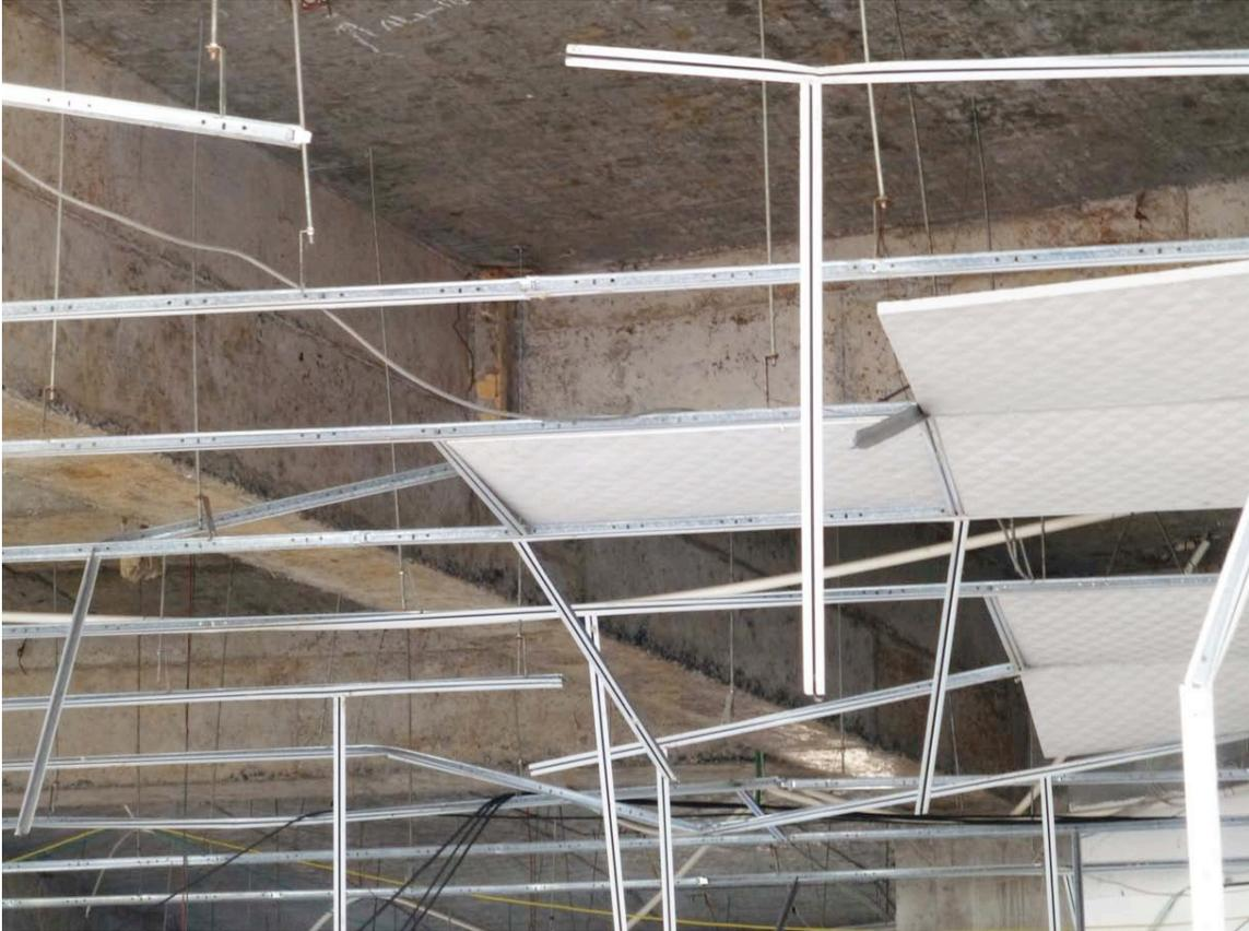
*Figure 12-2. Suspended Ceiling at Lushan Hospital (PGA ~0.25g to 0.35g) (Non-base-isolated). About 60% of the area of the suspended ceilings were heavily damaged, with those over larger rooms being relatively in worse condition*
