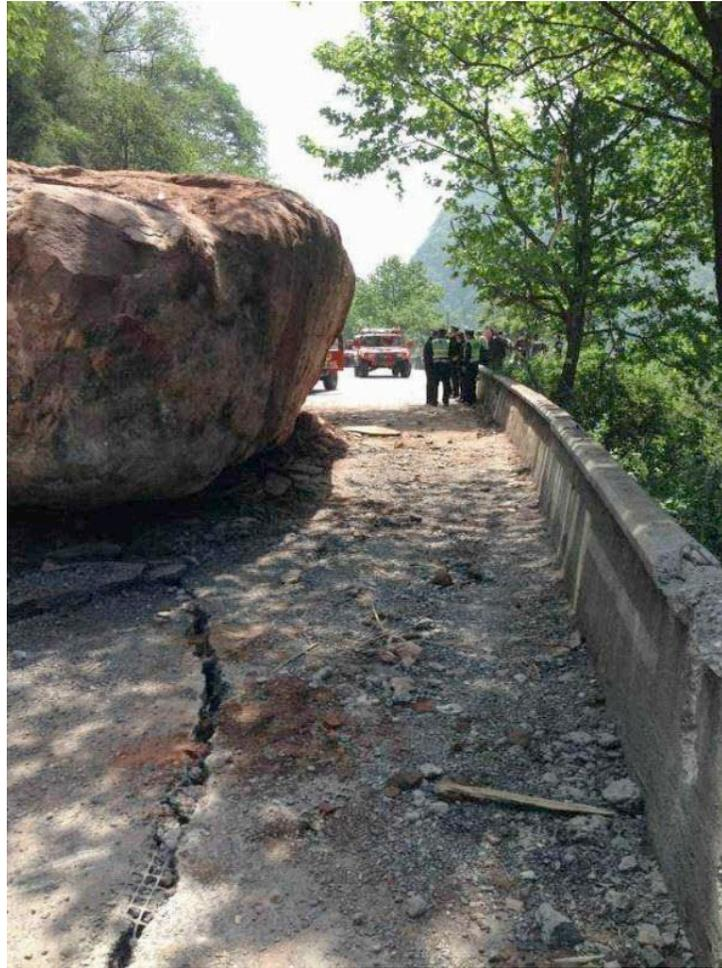
*Figure 7-3. S210 damage on Feixianguan (飞仙关) Road by large boulders*
