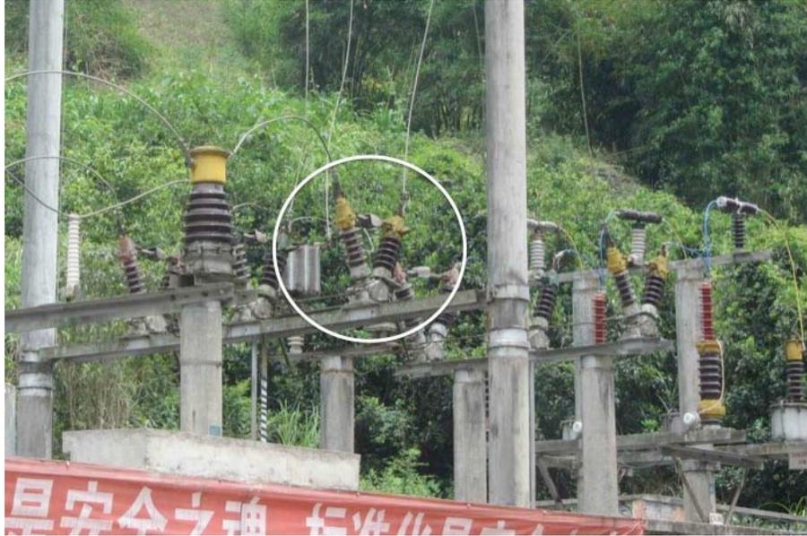
Figure 4-18 V-shape disconnect switch.
