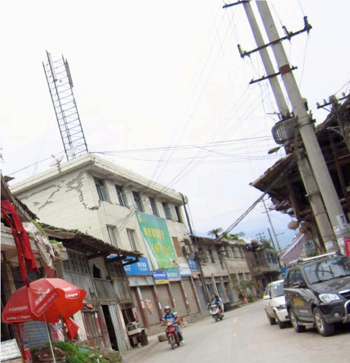
*Figure 8-4a. The white building with the tower on top, showed large cracks on the wall. See Figure 8-4b for cable management issue.*
