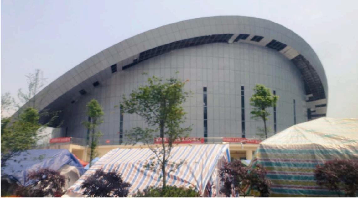
*Figure 10-7. Post-2008-Constructed Building in Lushan (Dropped Exterior Panels)*
