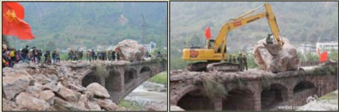
*Figure 7-8. Damage to stone arch Bridge 3 in Lushan County, Blossom Sector Road from large boulders. Left Image: Large boulder rolls onto bridge, destroys masonry rails. Right image: excavator attempts to remove large boulder.*
