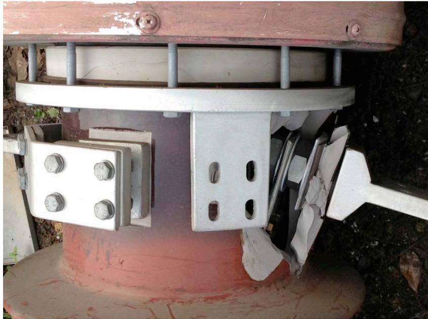
*Figure 4-8. 110 kV Broken Current Transformers*
