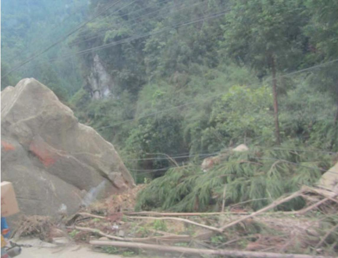
*Figure 2-20. Rockfall into road and damage of power poles*
