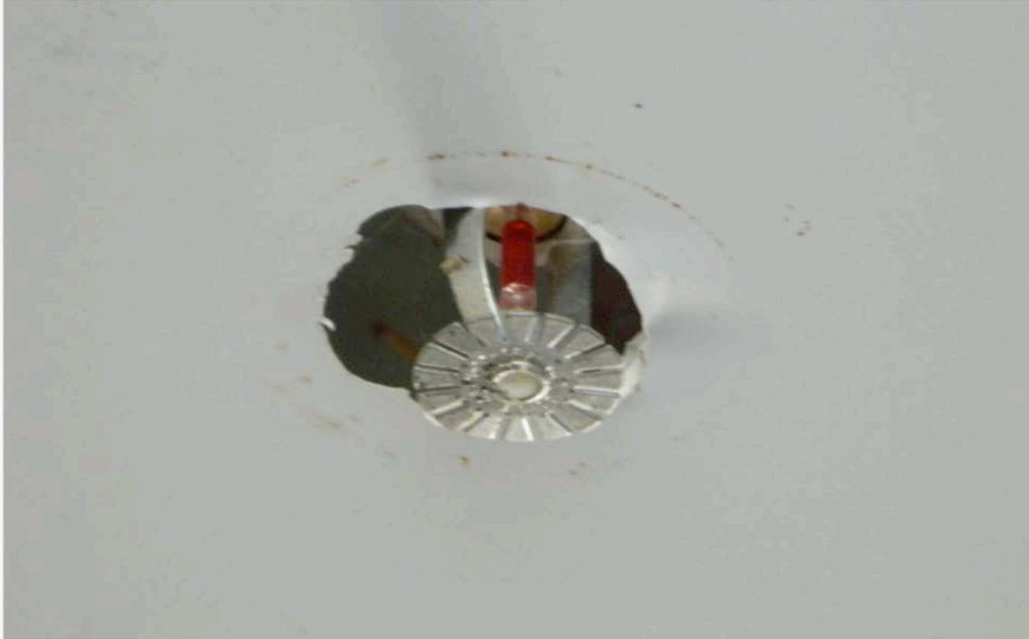
*Figure 12-4. Sprinkler head moved sideways and impacted the suspended ceiling.*
