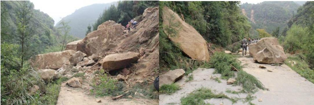
*Figure 7-5. Lushan County roads damaged and blocked by falling rock debris*
