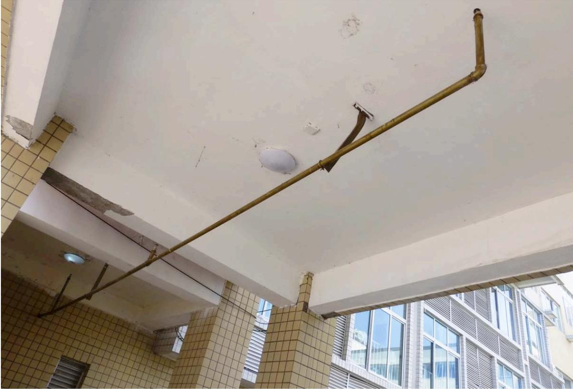
*Figure 10-5. Damaged Sprinkler Pipe Support*
