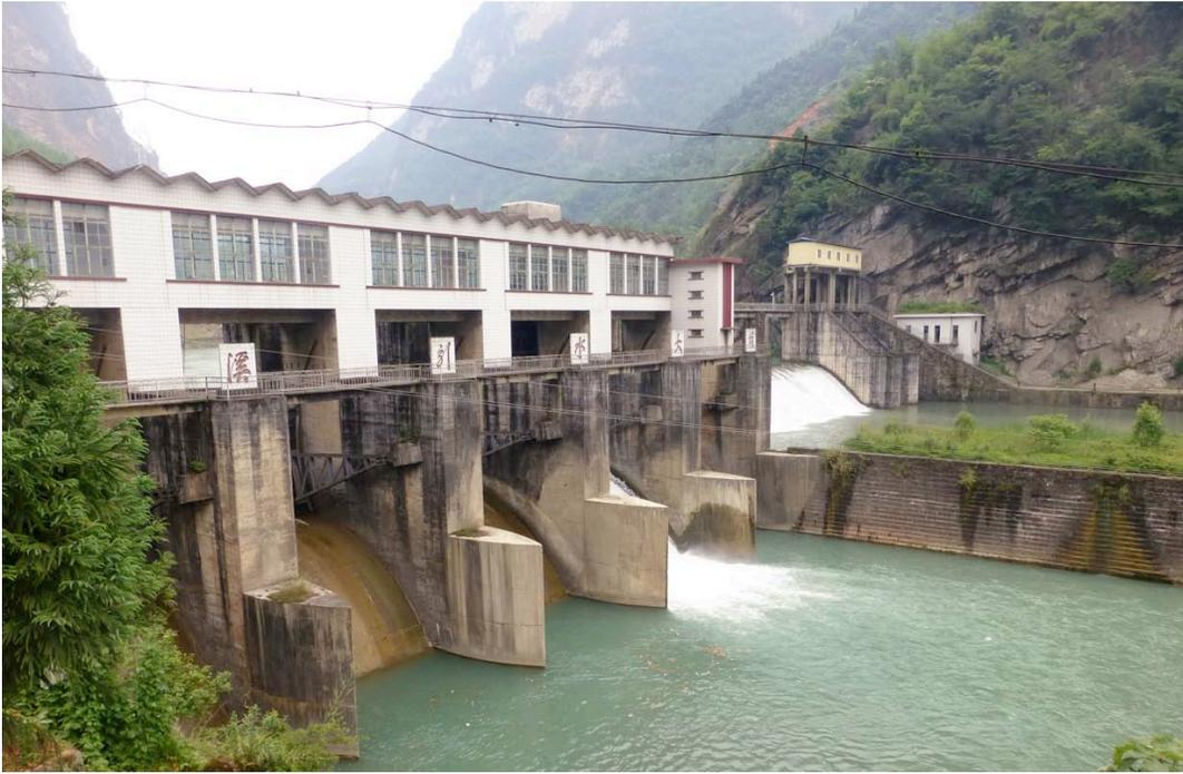
*Figure 4-23. Undamaged Dam (PGA ~0.35g)*
