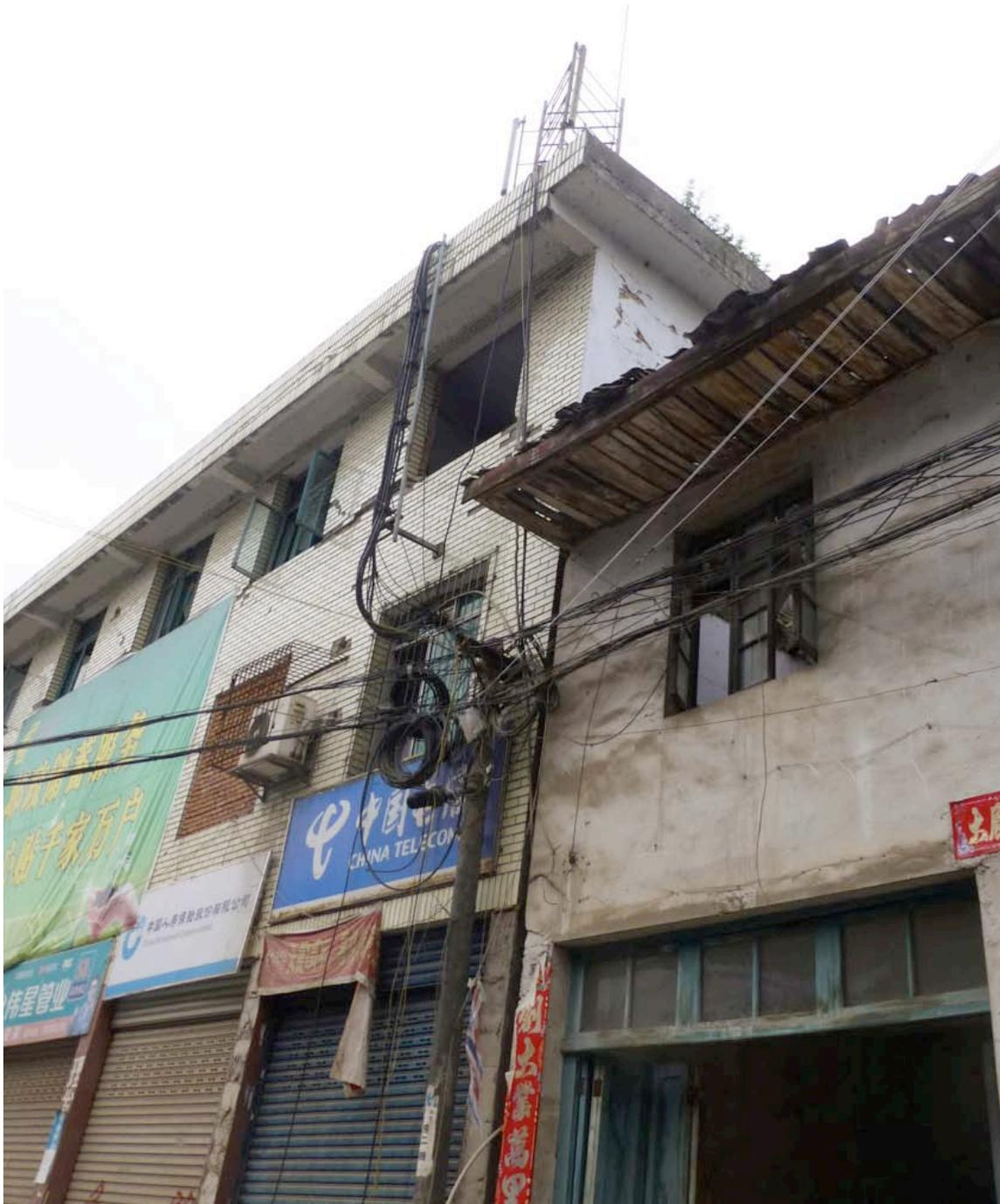
*Figure 8-4b. Note that cable management is poor, the cables were dropped from the edge of roof to the head of the pole, site in Fig 8-4a.*
