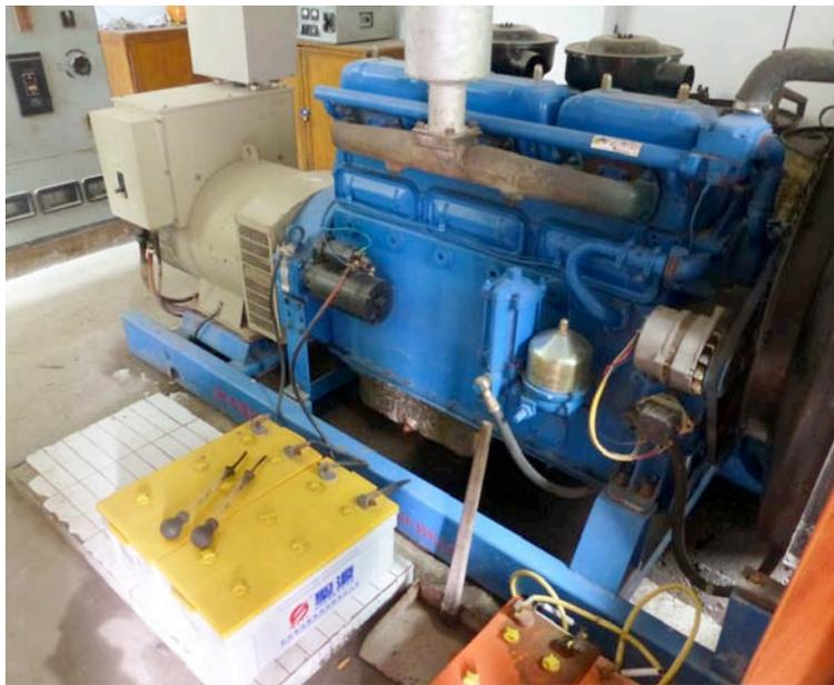
*Figure 4-24. Emergency Generator with Unrestrained Startup Batteries*
