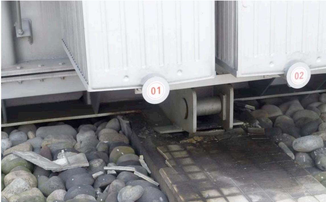
*Figure 4-5. Bank 1 Transformer – Evidence of sliding (broken tiles over concrete foundation) and leakage of oil. The transformer was pushed back to its original position.*
