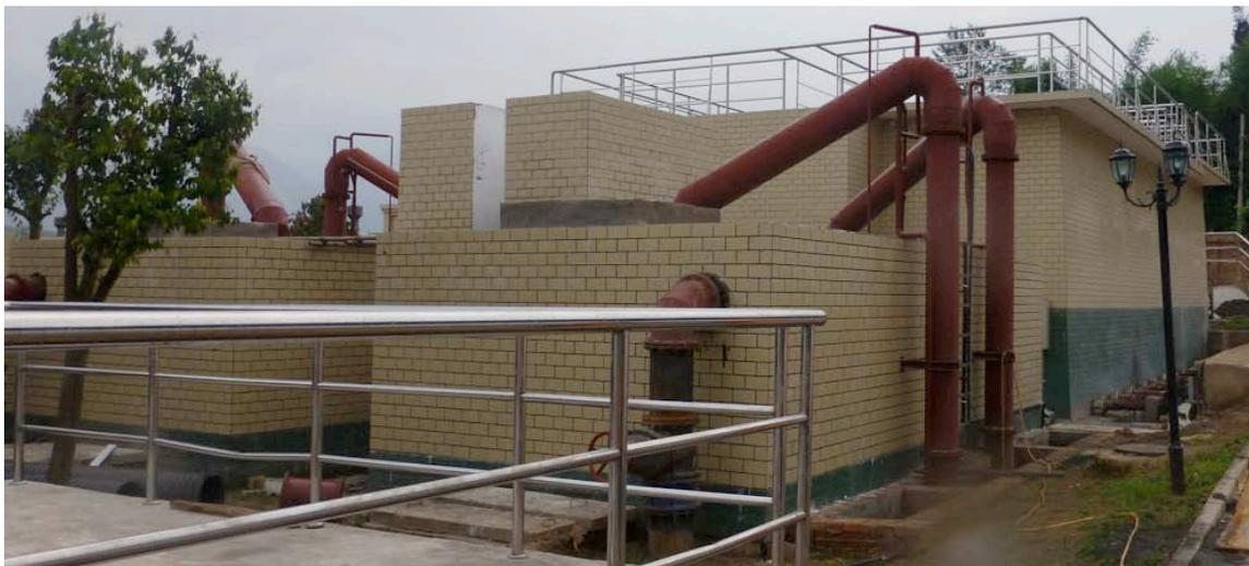
*Figure 5-2. Settling and Filter Basin Structures*
