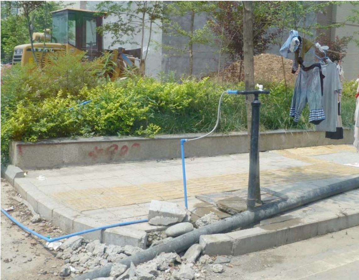
*Figure 5-8. Above Ground Temporary Water Pipe*
