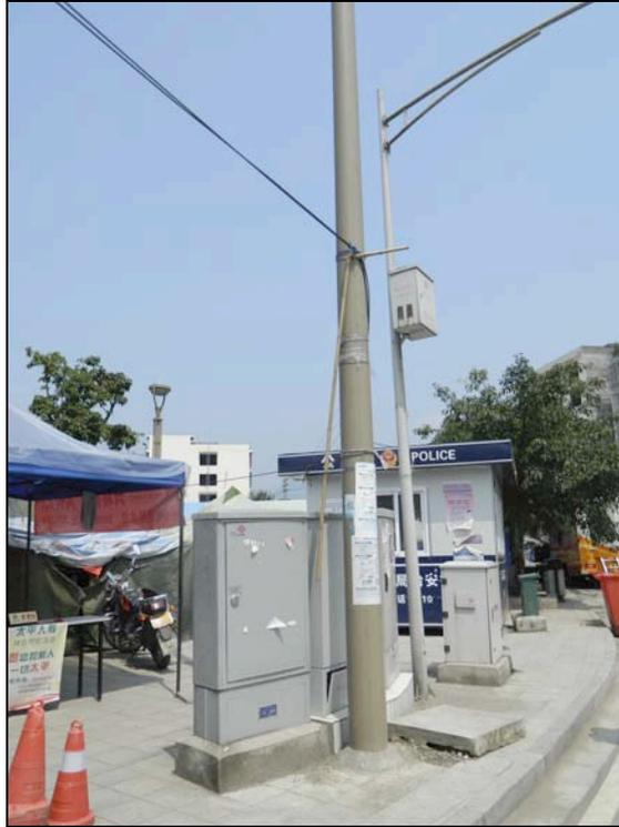
*Figure 8-3. This fiber optic cable provided temporary connection to the hospital. All three telecommunication service providers placed their cabinets close to the power termination box (the small cabinet to the right).*
