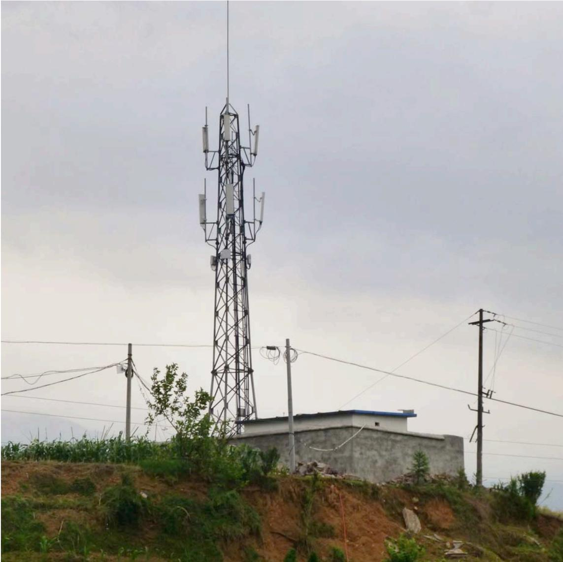
*Figure 8-6. This cell site did not show any sign of failure to the tower and to the building.*
