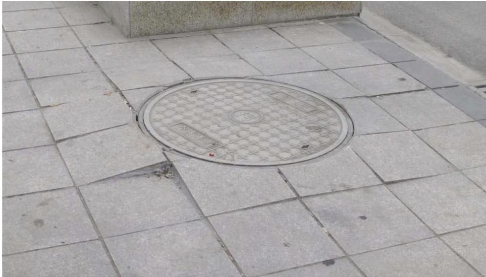
*Figure 6-1. Floated Manhole*
