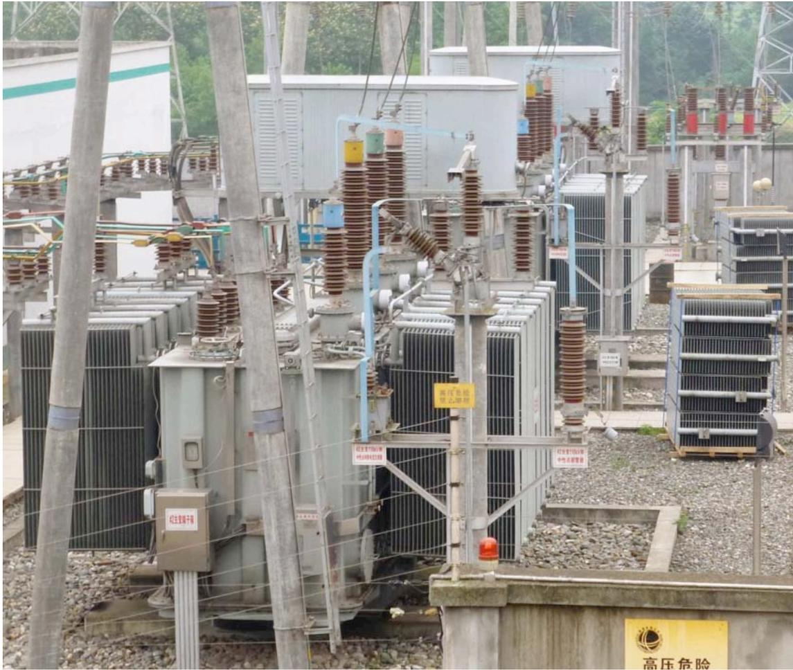
Figure 4-15. 110 kV Transformers and Radiators at Substation 2
