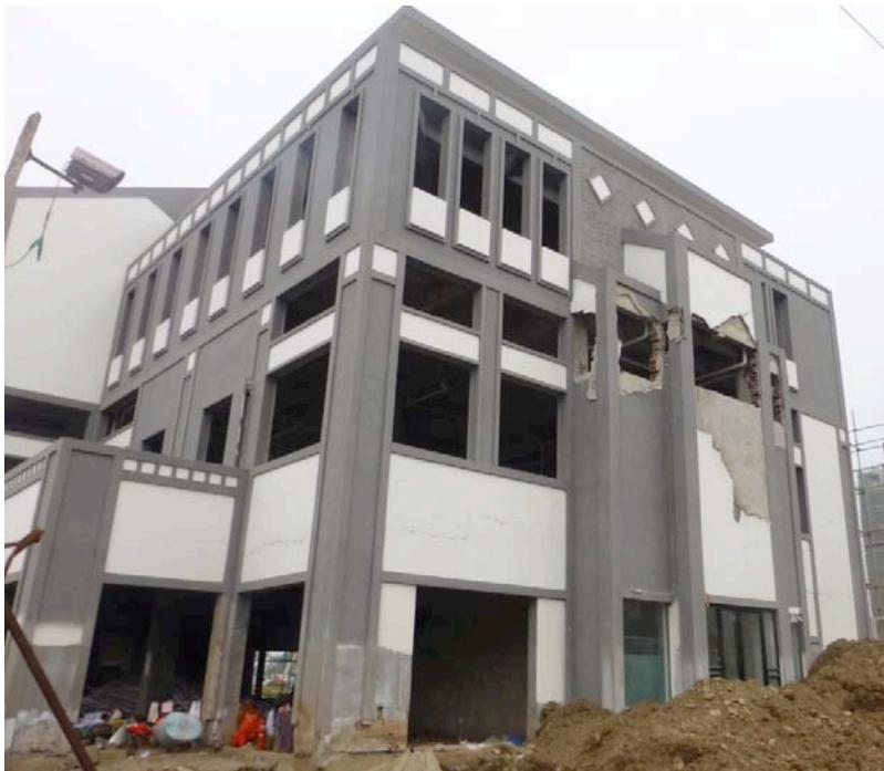
*Figure 10-8. Post-2008-Constructed Building in Lushan (Failed Masonry Walls)*
