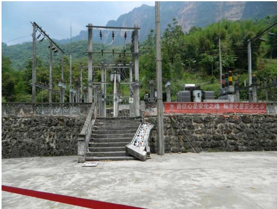
Figure 4-19 Entrance to the Dayanqiang (大岩腔) 35kV substation yard. Note the broken railing and part of the wall.
