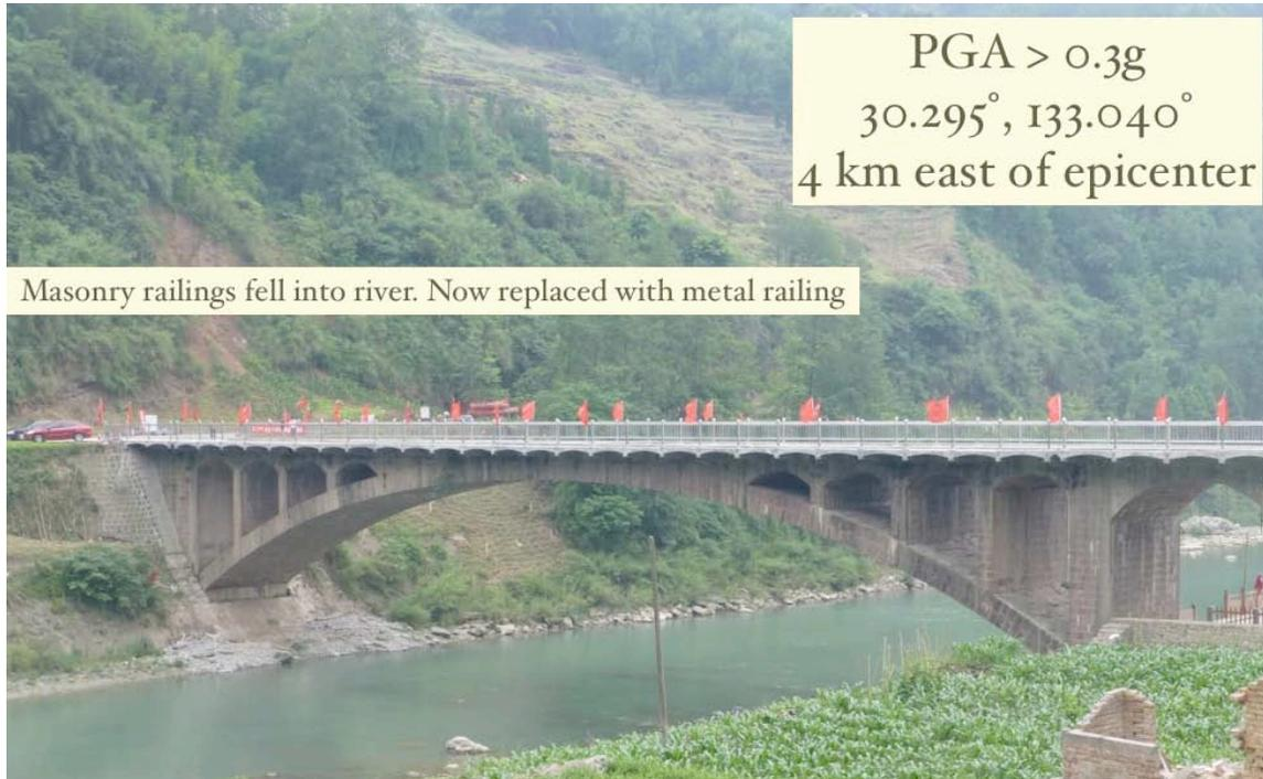
*Figure 7-6. Damage to stone arch Bridge 1 in Lushan County (photo date May 31 2013)*
