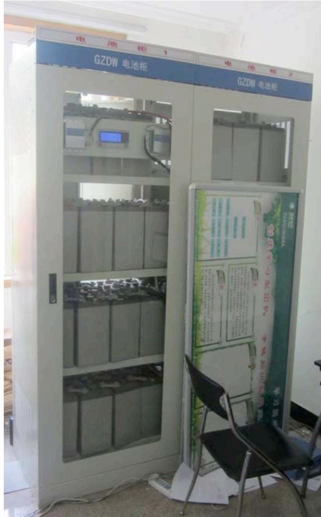
*Figure 4-13. Sliding Batteries within Cabinets (uneven spaces between batteries due to sliding)*
