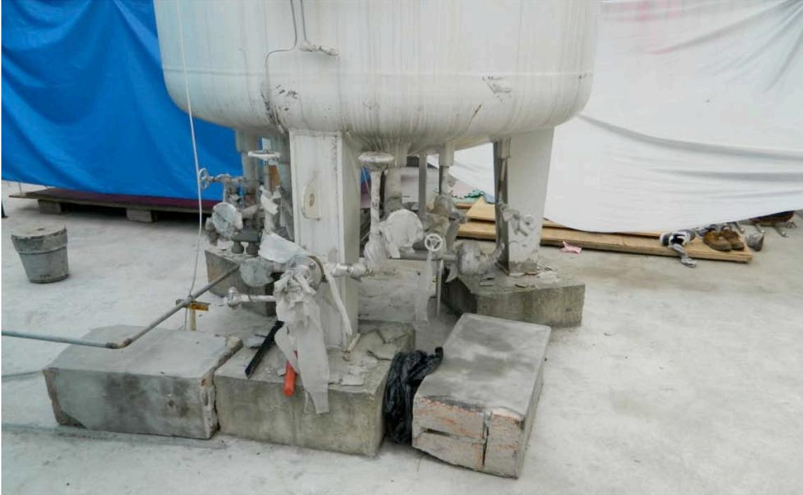
*Figure 12-3. Unanchored Liquid Oxygen tank rocked at the hospital in Lushan. The rocking resulted in failure of the attached pipe. All liquid oxygen evaporated.*
