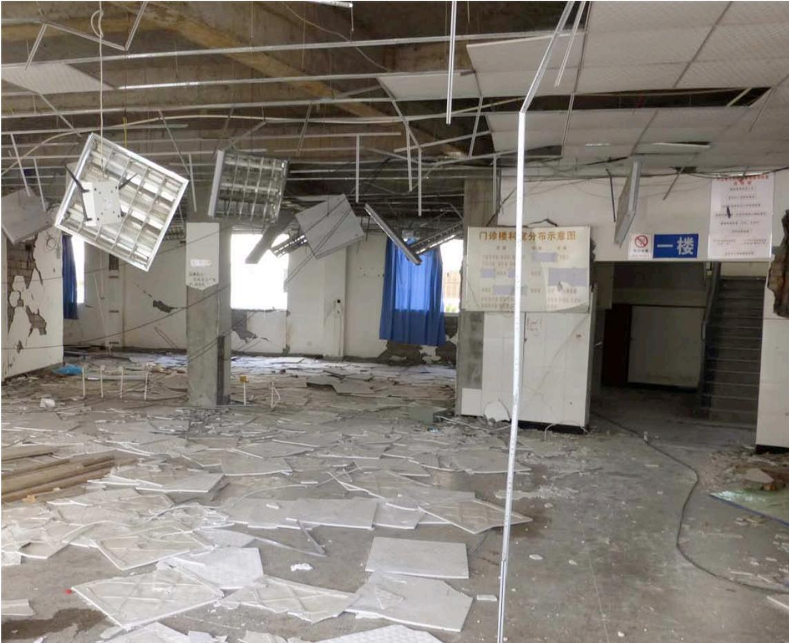
*Figure 12-1. Suspended Ceiling at Lushan Hospital (PGA ~0.25g to 0.35g) (Non-base-isolated)*
