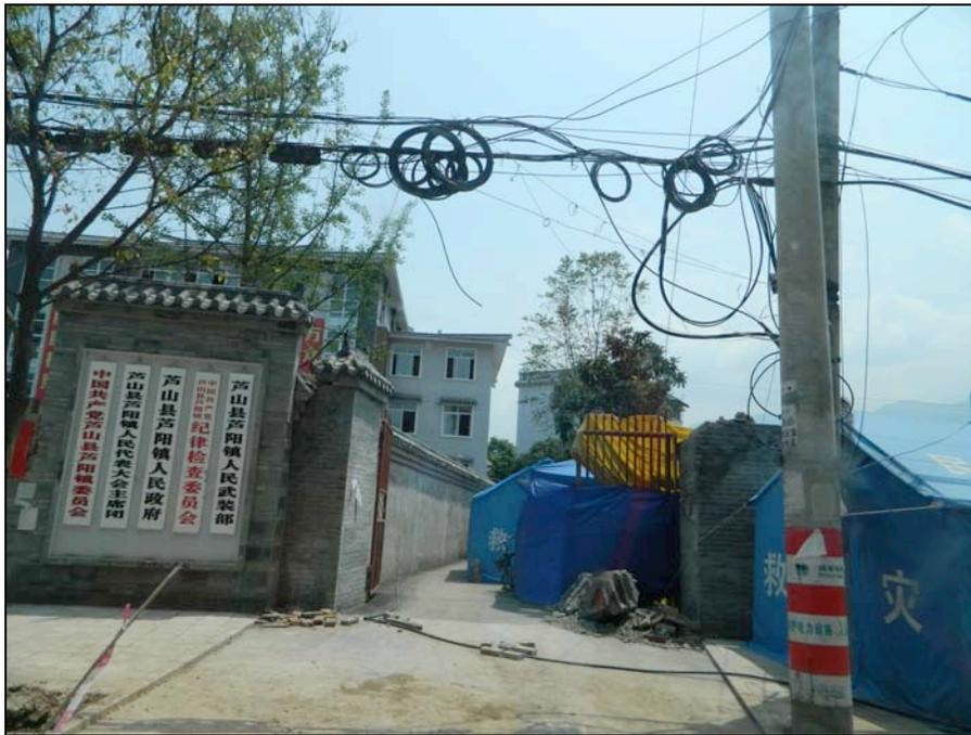
*Figure 8-12. Example of poor cable management in Lushan*
