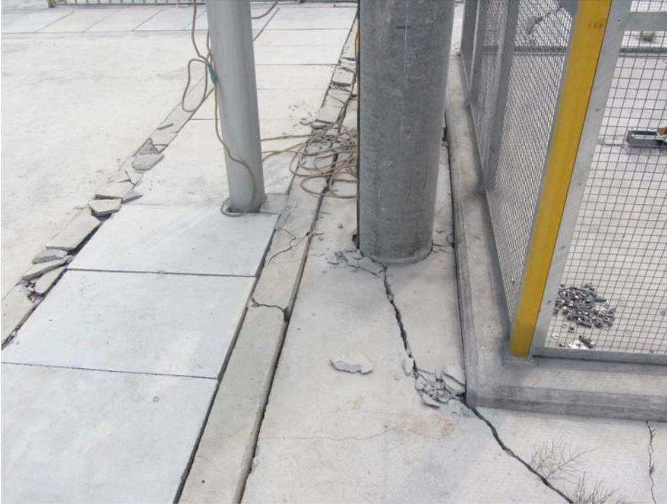
*Figure 4-14. Cracks in the concrete pavement / cable trench due to the permanent ground movement*
