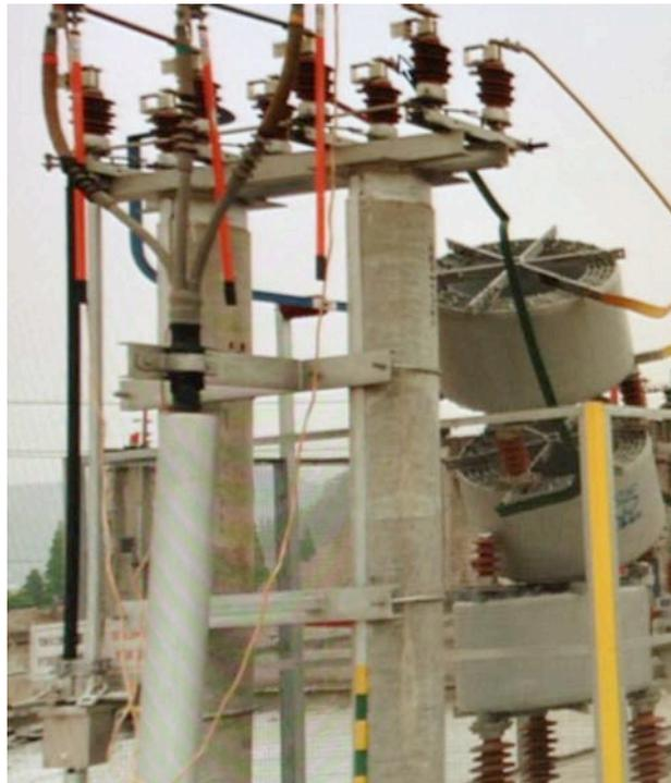
*Figure 4-11. Damaged Air Core Reactors*
