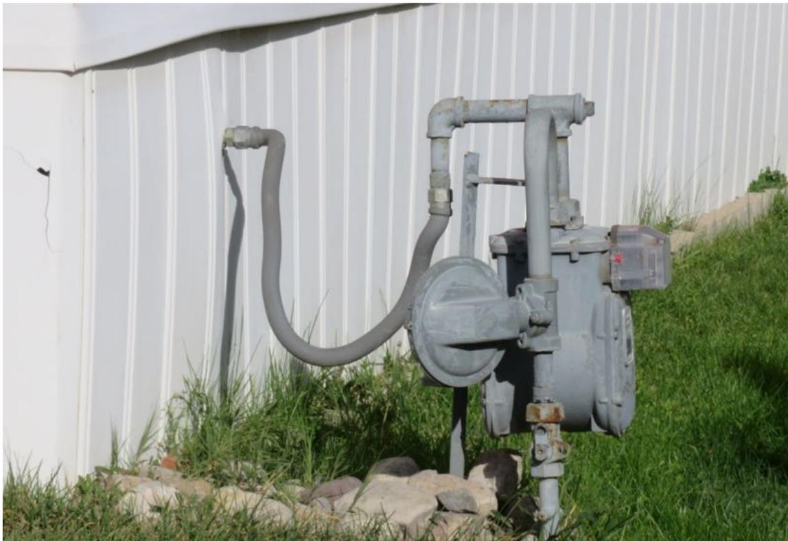
*Figure 24. Structure 7. Original Meter. Post-type supplementary support. No impacts.*
