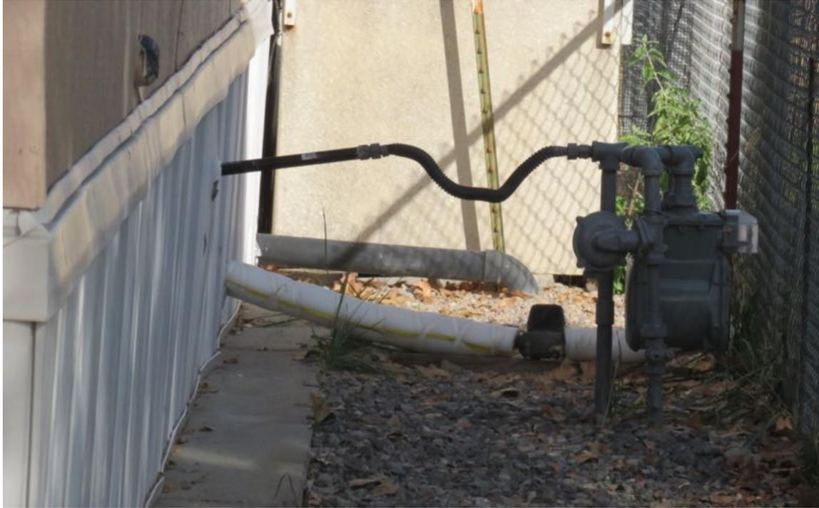
*Figure 23. Structure 6. Original Meter. Tube-type supplementary support. No impacts.*
