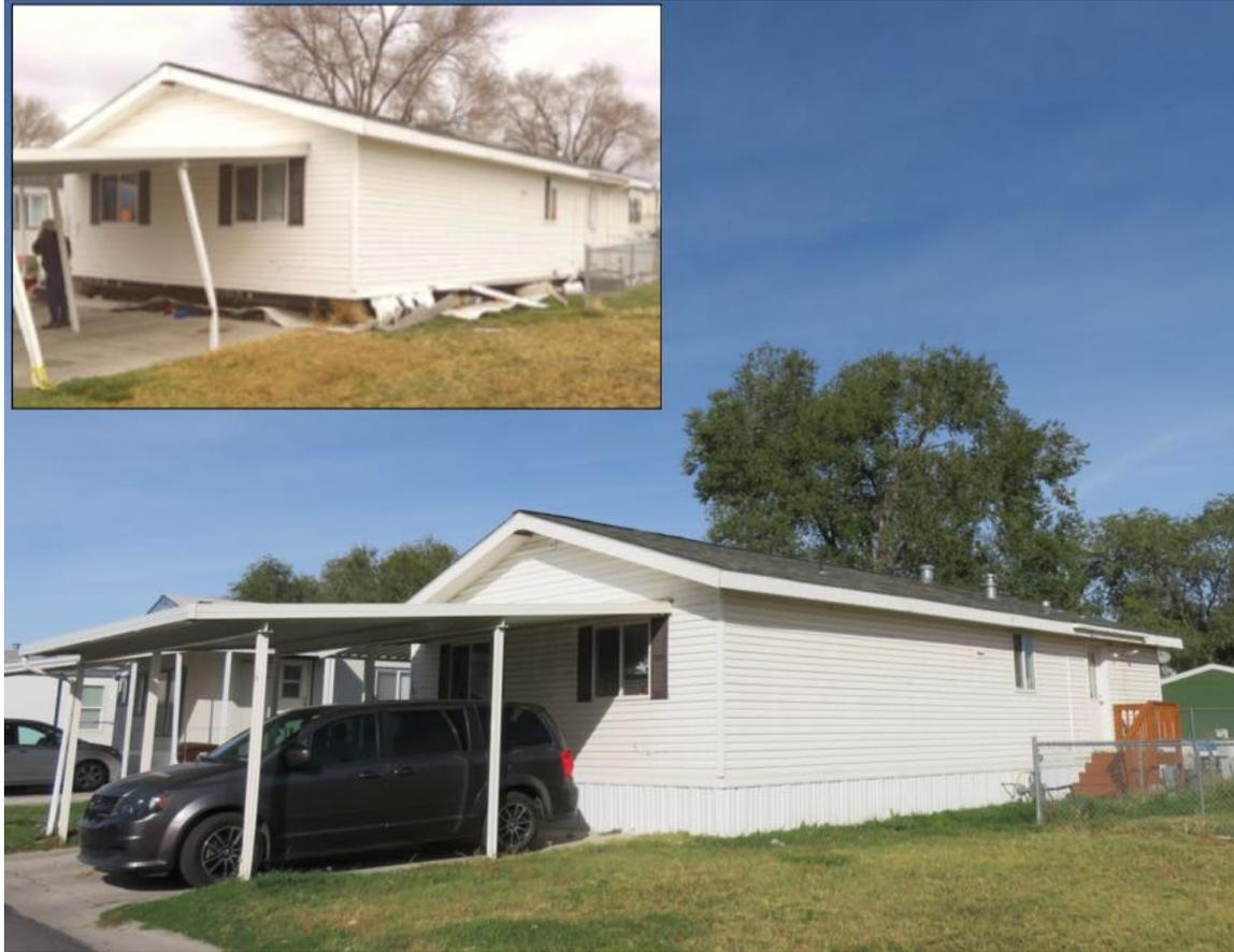
*Figure 32-a. Structure 75. Inset Photo shows structure immediately post-earthquake. Main photo shows structure after repair. Figure 32-b shows gas meter set after repair.*
