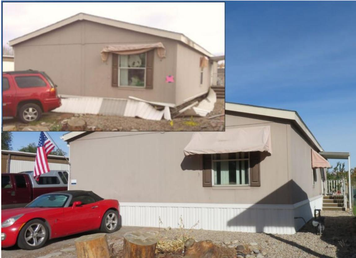
*Figure 26-a. Structure 18. Inset Photo shows structure immediately post-earthquake. Main photo shows structure after repair. Inset photo indicates impacted gas meter set. See Fig 24b for meter.*
