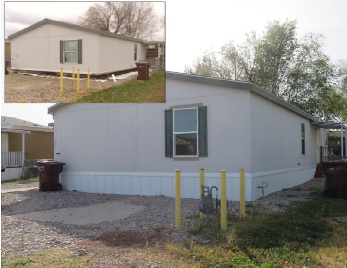
*Figure 33-a. Structure 141. Inset Photo shows structure immediately post-earthquake. Main photo shows structure after repair. 4 yellow bollards (foreground) intended to protect meter from impacts from vehicles. Replacement meter set back from low pressure customer pipe with new yellow flex hose (Figure 33-b).*
