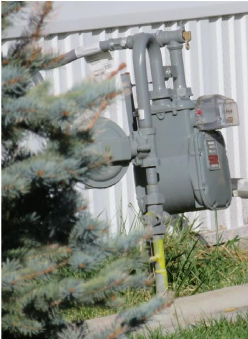
*Figure 22. Structure 5. Meter tilted (towards structure).*
