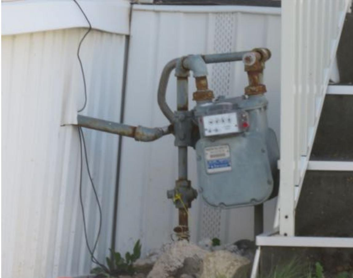
*Figure 29. Structure 44. Original Gas Meter Set (Tube Support). Tilted*
