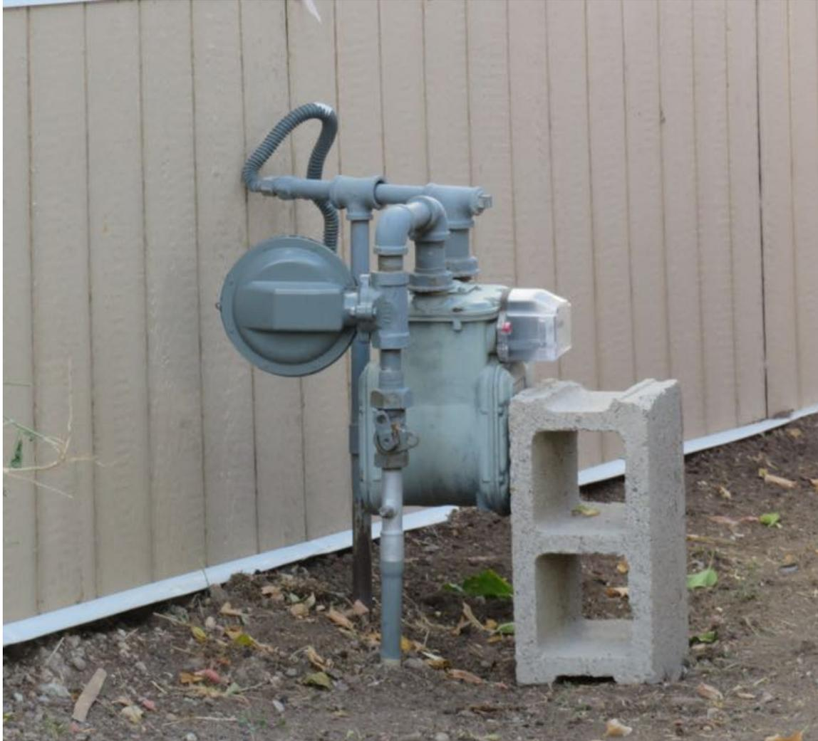
*Figure 25. Structure 16. Original Meter. Tube-type support. Limited clearance D.*
