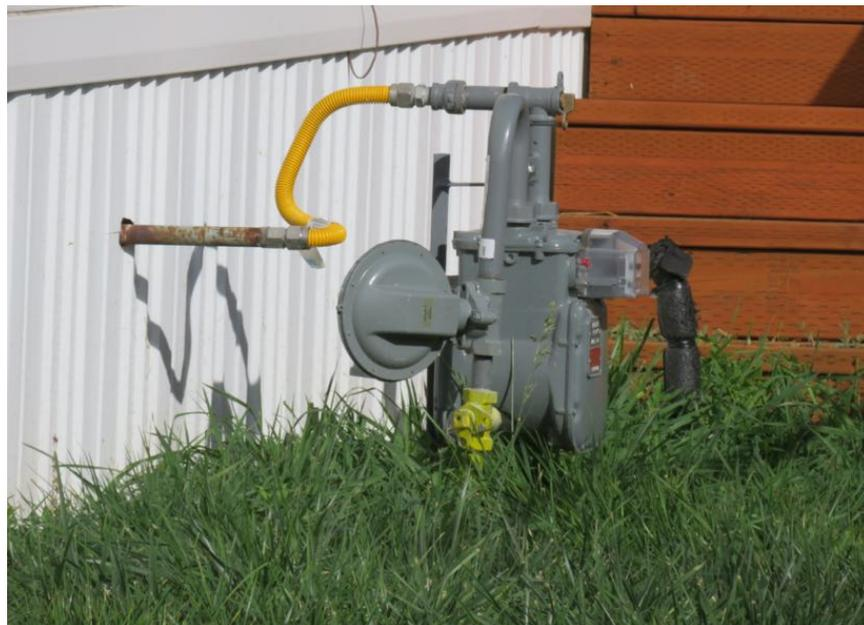
*Figure 32-b. Structure 75. New flex hose (yellow). New Meter and Regulator. Original customer-side pipe (with rust).*
