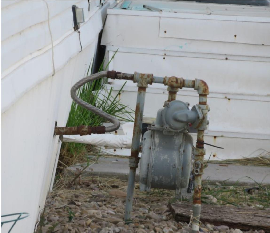
*Figure 31. Structure 67. Tilted Gas Meter Set. Damage to MH suggests the meter was impacted during the earthquake.*
