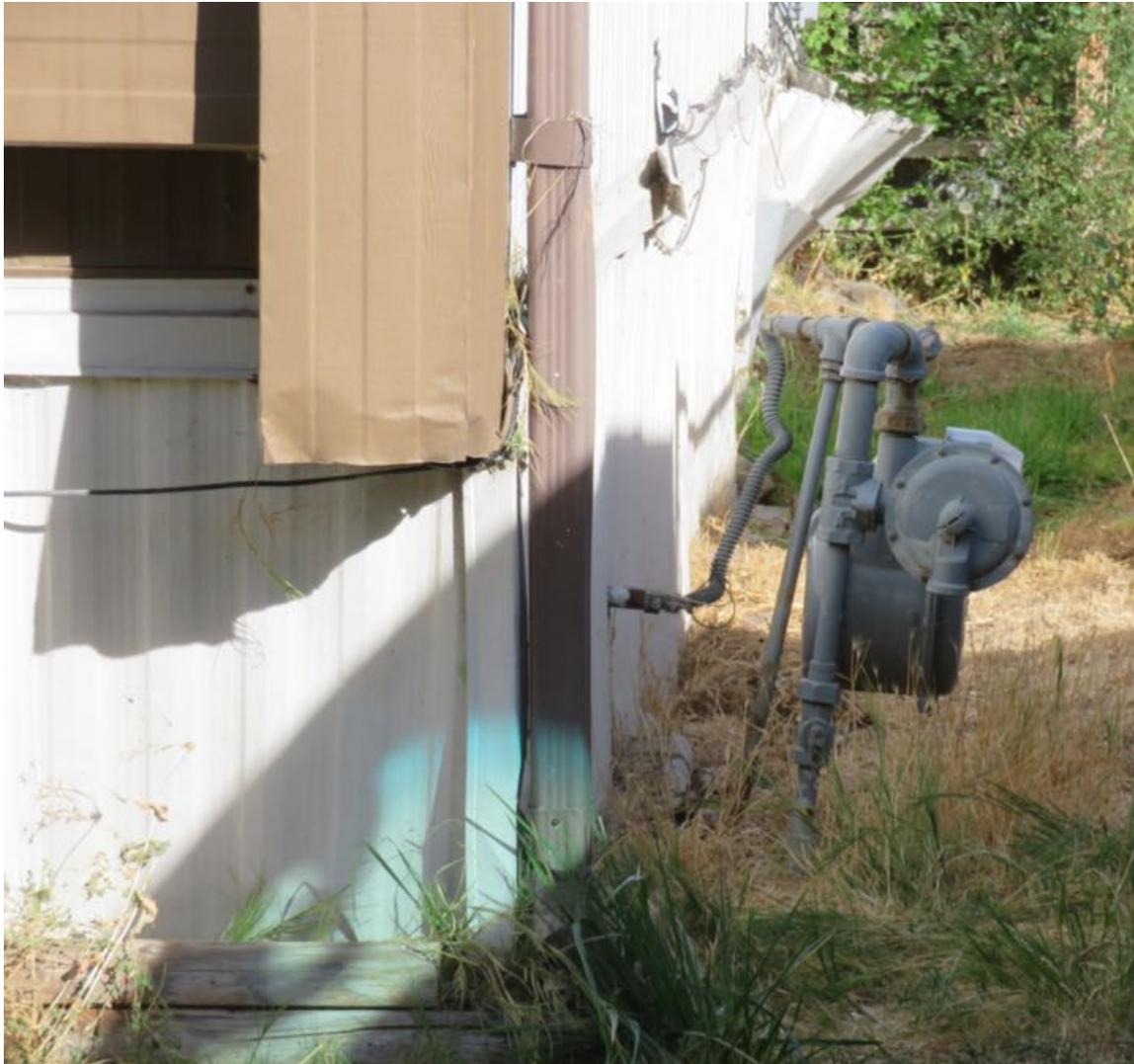
*Figure 27. Structure 19. Tilted Gas Meter Set (Tube Support). Indication is that the MH impacted the tube type support*
