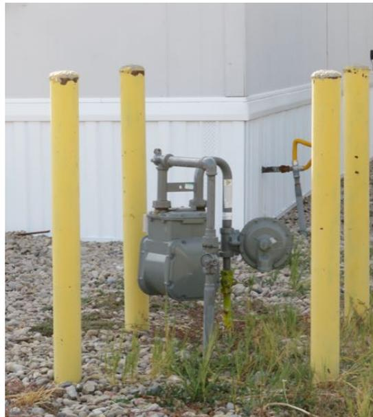
*Figure 33-b. New meter (foreground) new flex hose (yellow). Bollards are original.*
