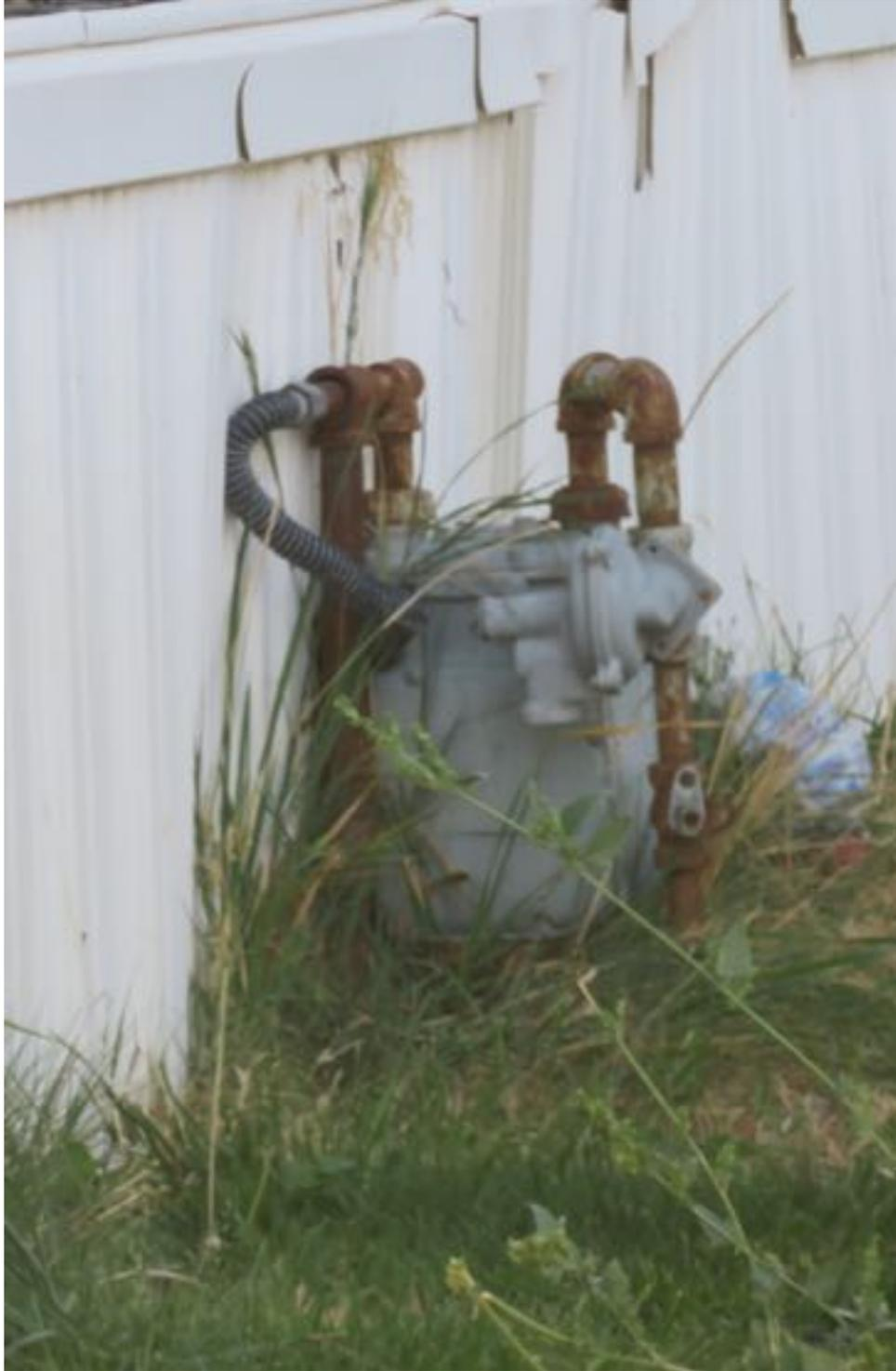
*Figure 28. Structure 33. Original Gas Meter Set (Tube Support). Limited clearance D.*
