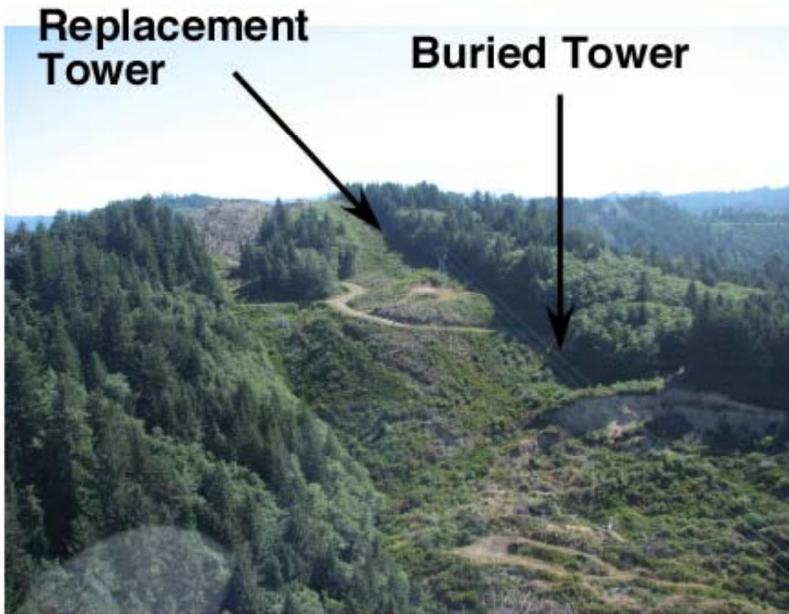
Figure 6. Transmission Tower Buried by Landslide
