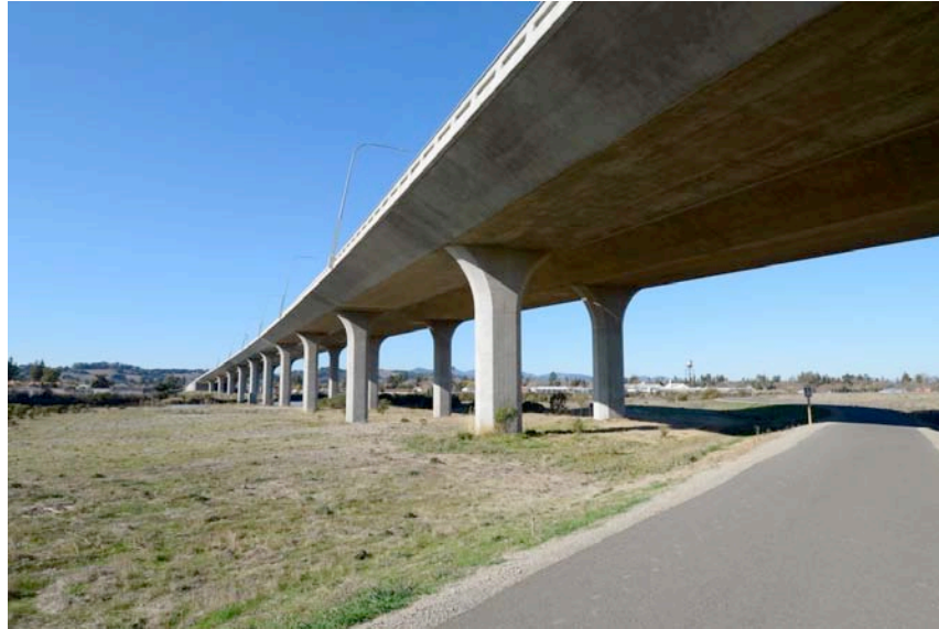
Figure 5-15. Napa River (West Imola Avenue) Bridge Br. #21 0108L/R (38.2814°, -122.2842°)
