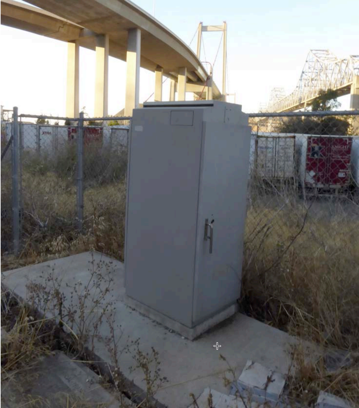
Figure 2-30. Instrument with New (Left) and Old (Right) Carquinez Bridges in Background
