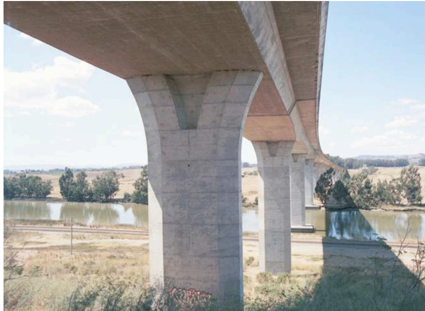
Figure 5-11. Napa River Bridge on Route 29 Br. #21 0049 (38.1245°, -122.285°)
