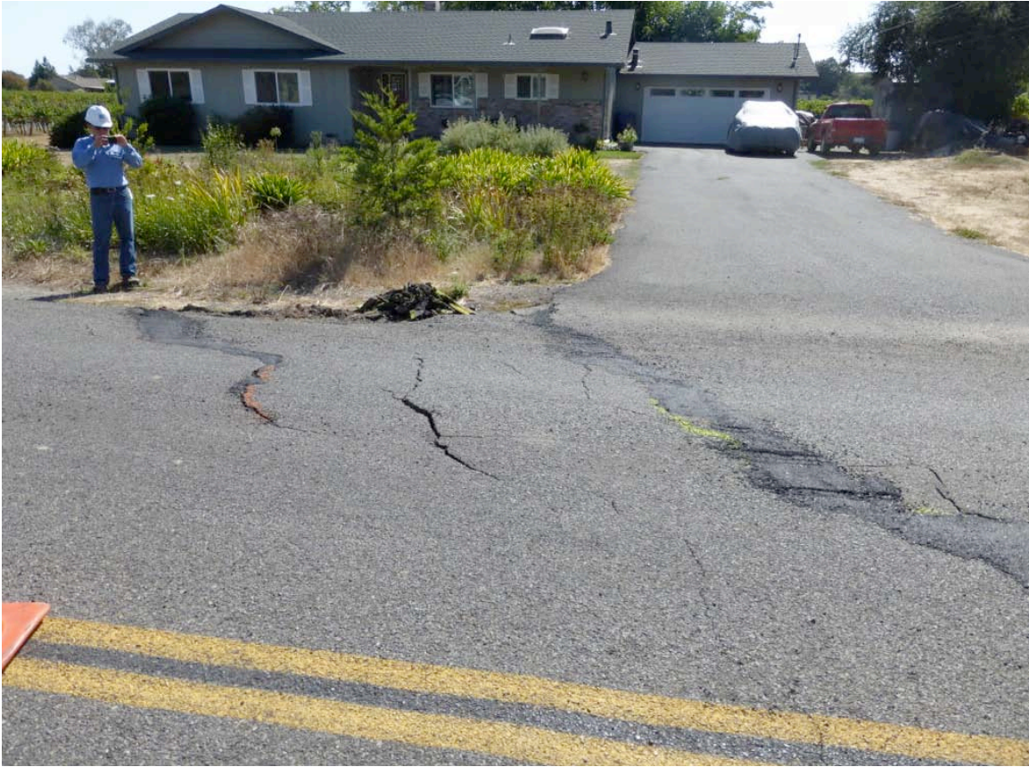
Figure 2-25. Repaired and newly formed cracks in street
