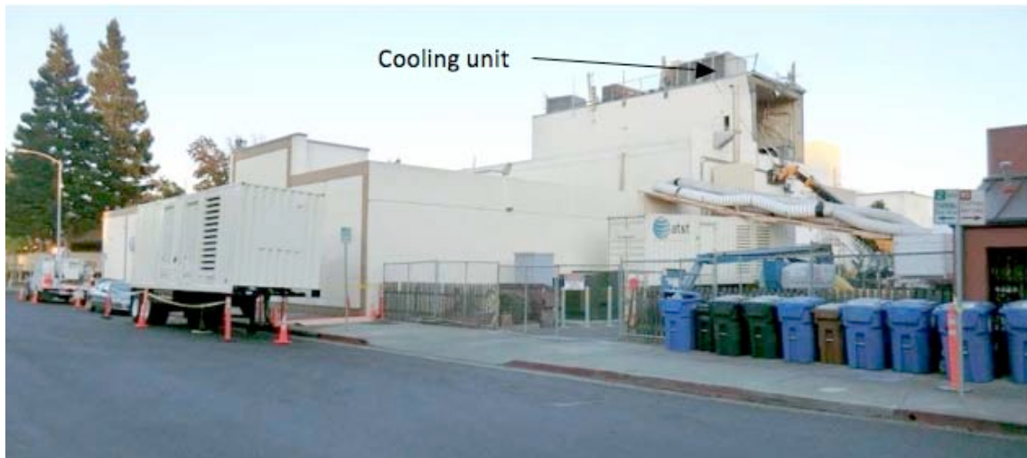
Figure 6-5. AT&T Building on August 25, 2014
