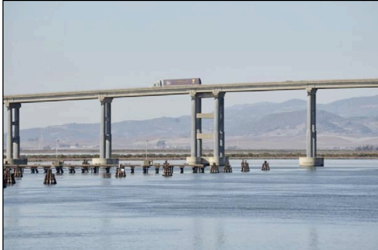
Figure 5-6. Retrofitted Napa River Bridge with Steel Column Casings and Enlarged Footings
