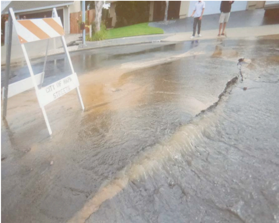
Figure 4-7. Water Leaking from a Damaged Distribution Pipe
