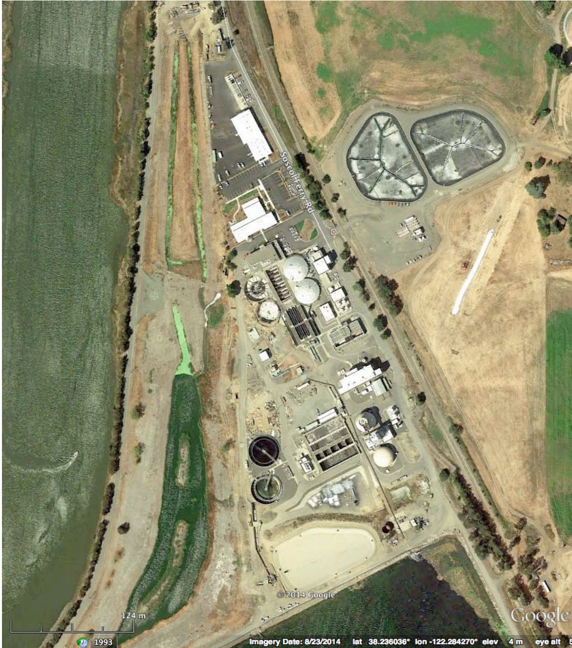
Figure 4-16. Suscol Wastewater Treatment Plant
