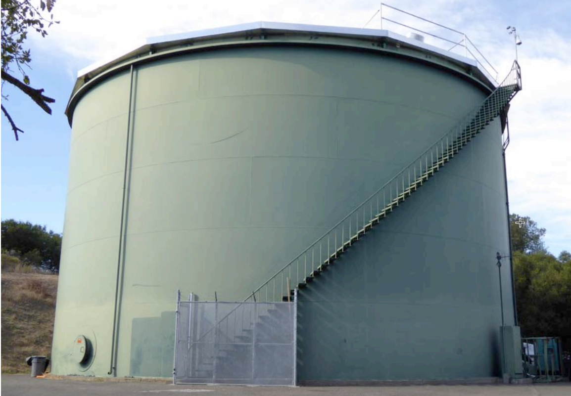
Figure 4-11. Tank B, with New Aluminum Dome Roof
