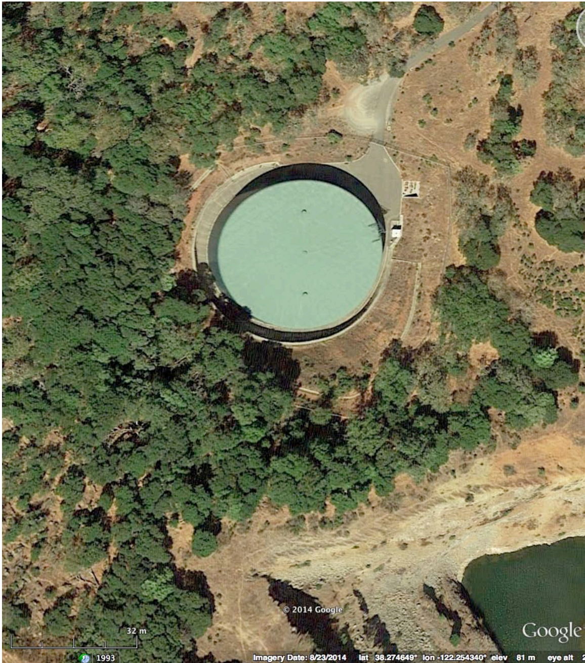
Figure 4-18. Recycled Storage Reservoir
