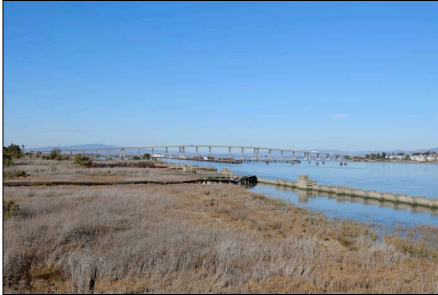
Figure 5-4. Napa River Bridge on Route 37 Br. #23 0064
