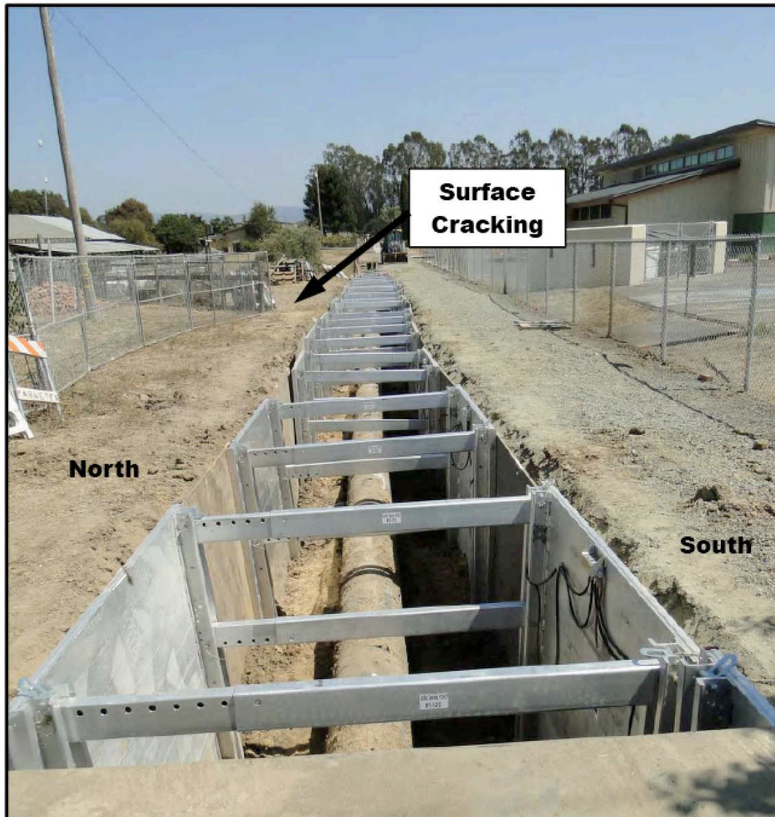
Figure 8-2. PG&E Gas Pipe Trench Excavation, Sept 1 2014, Looking East
