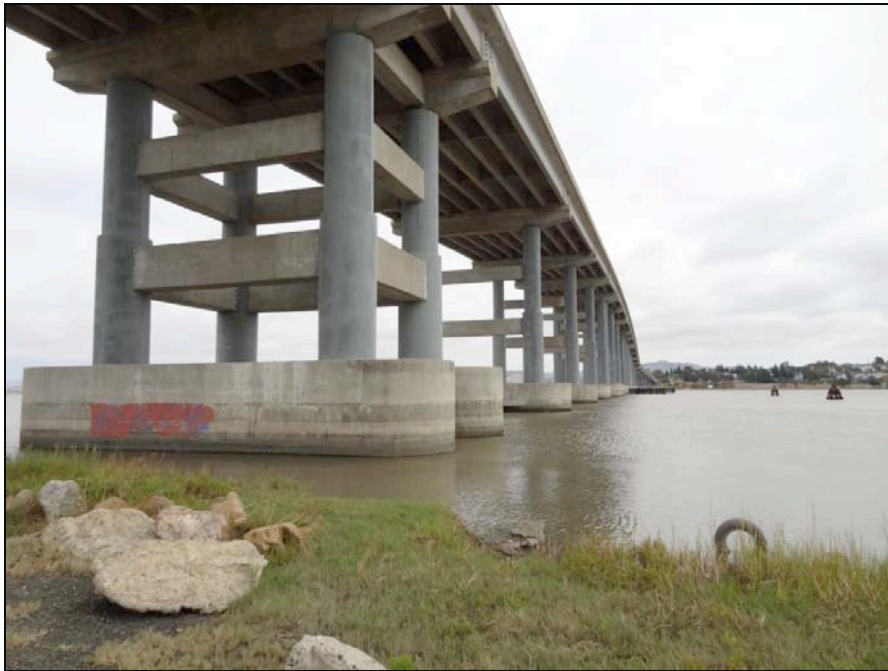
Figure 5-3. Napa River Bridge on Route 37 Br. #23 0064 (38.1203°, -122.2800°)
