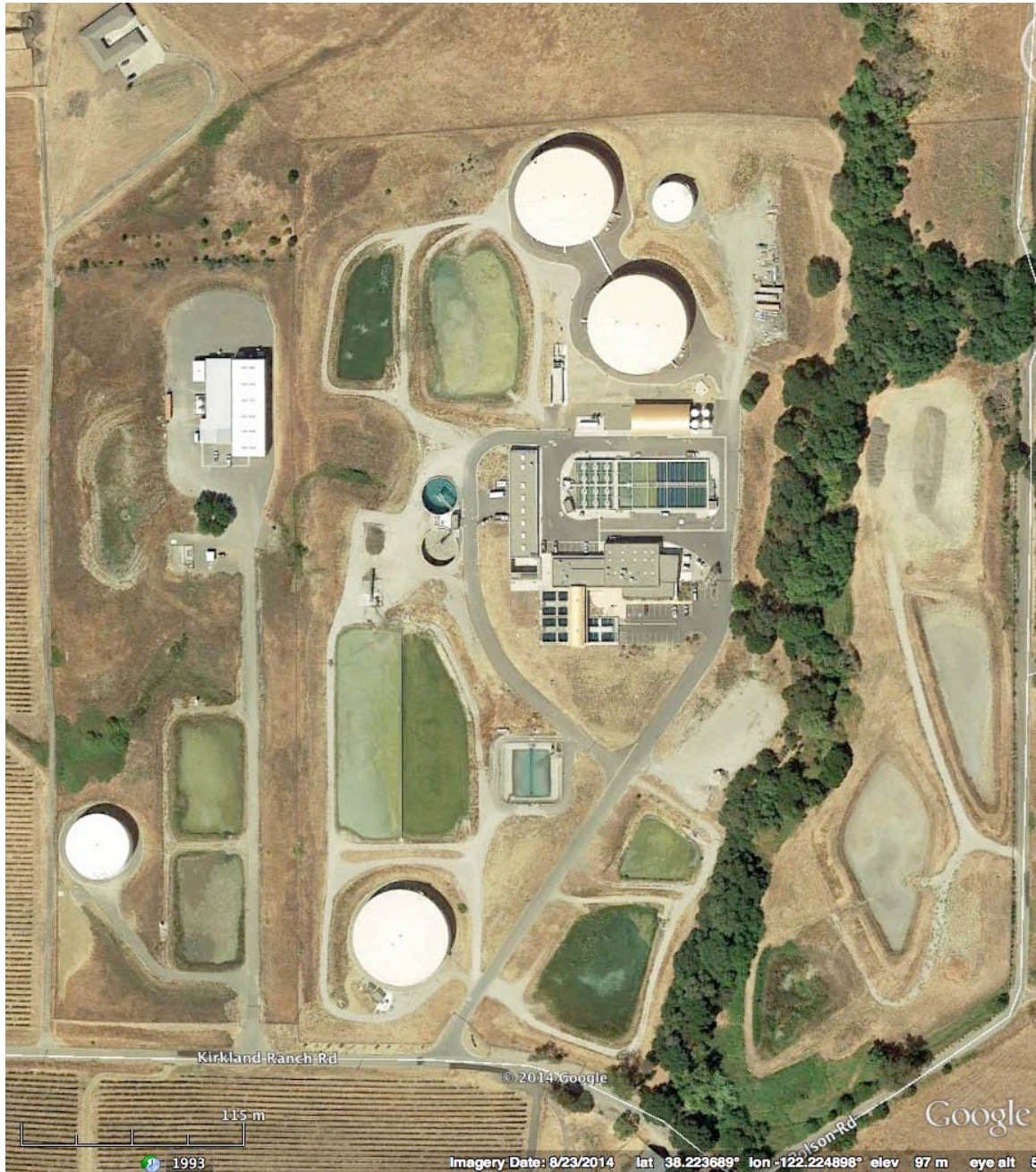
Figure 4-4. Jamieson Water Treatment Plant (38.2236, -122.2249)
