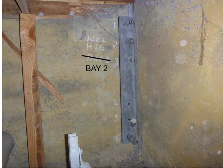
Figure 5-18. Restrainer damage at Hinge 10, Bay 2 of Napa River (W. Imola Ave) Bridge
