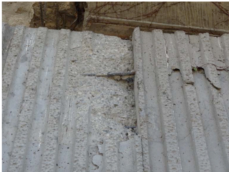
Figure 5-17. Close-up of damaged curtain walls on the Napa River (West Imola Ave) Bridge
