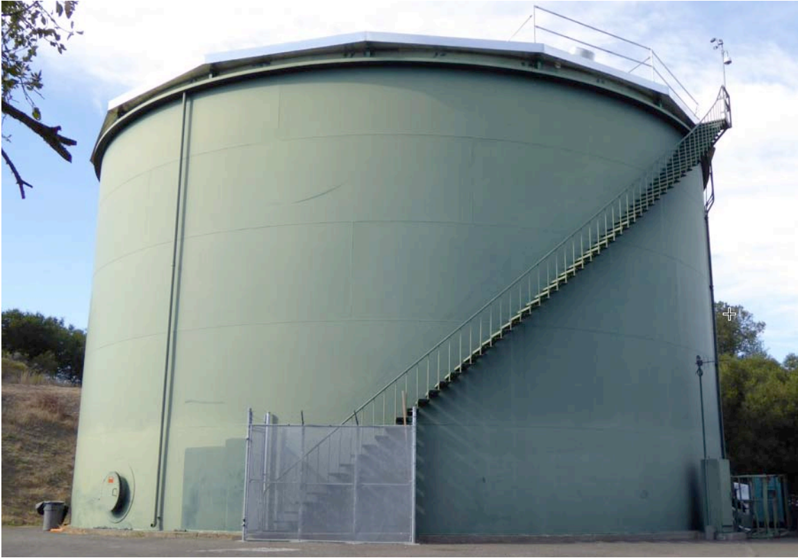
Figure 4-11. Tank B, with New Aluminum Dome Roof
