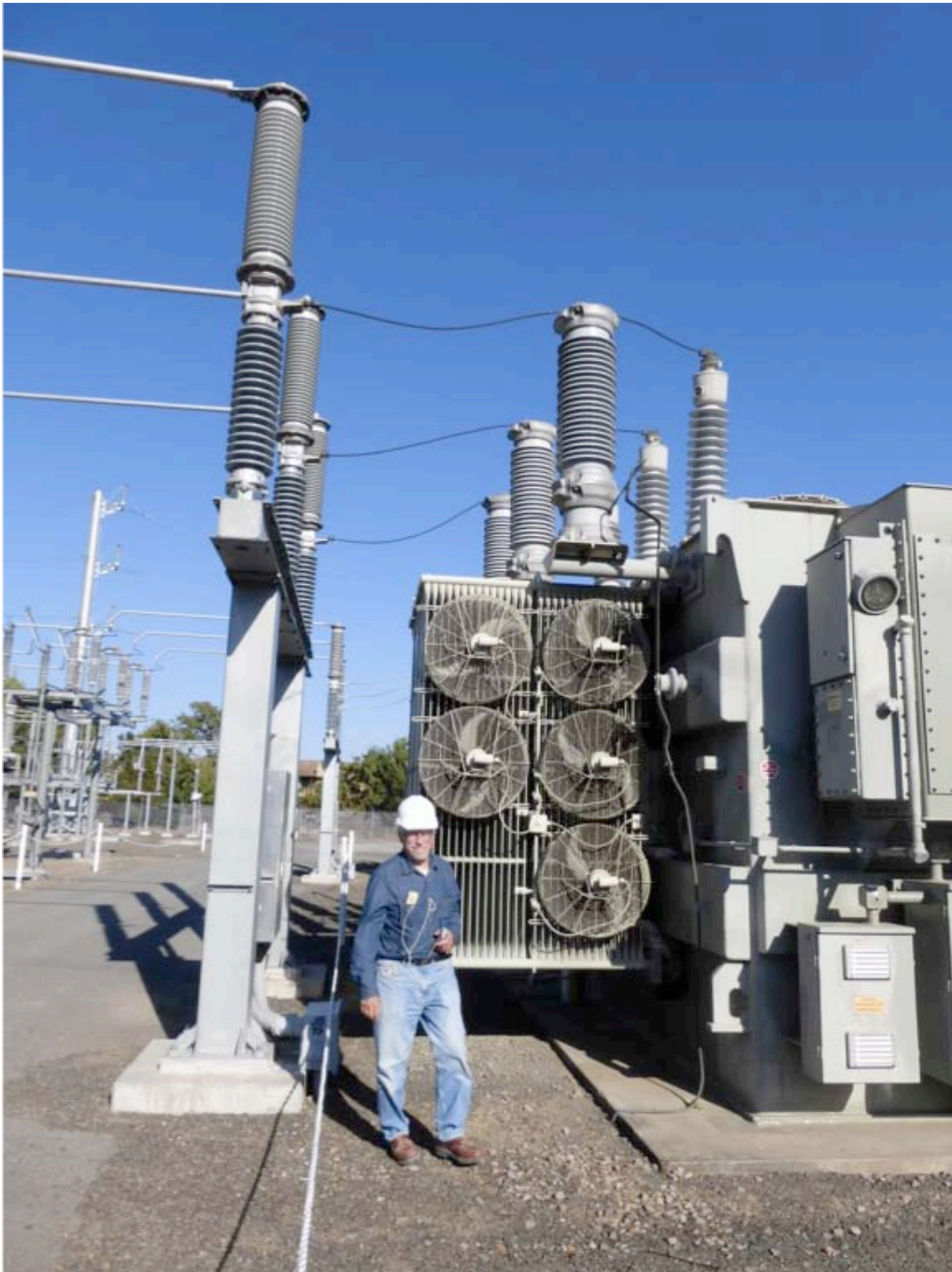
Figure 3-2. Power Transformer
