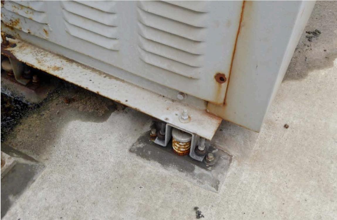
Figure 4-21. Spring-Mounted Motor Assembly
