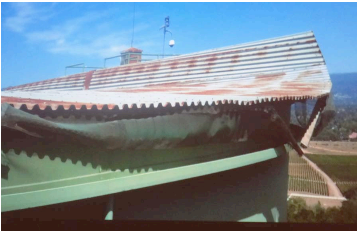
Figure 4-9. Damaged Roof of Steel Tank "B"
