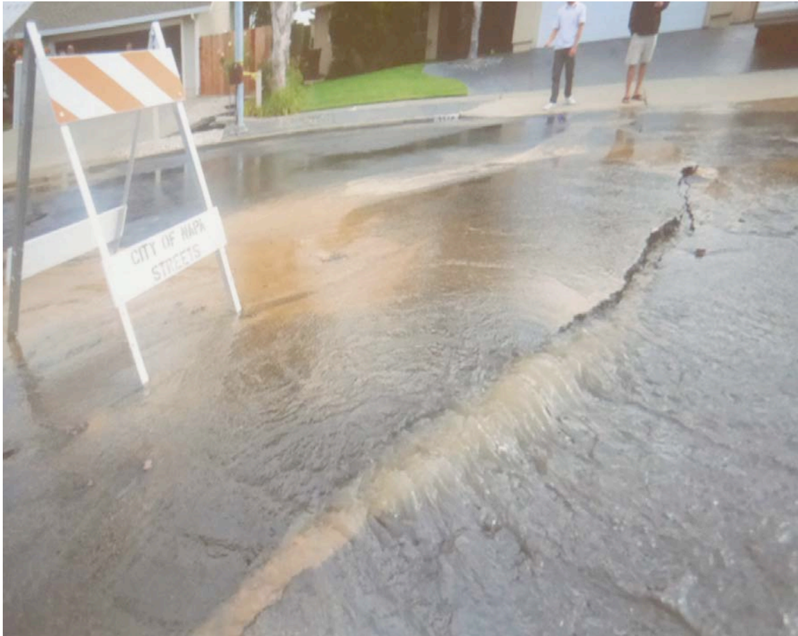
Figure 4-7. Water Leaking from a Damaged Distribution Pipe
