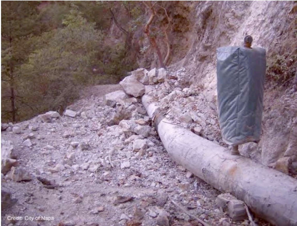
Figure 4-6. Damaged Transmission Pipe due to Rockfall
