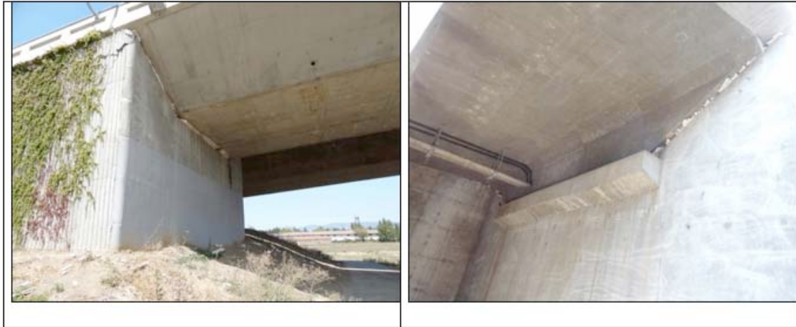
Figure 5-16. Outside and Inside of an abutment on the Napa River (West Imola Avenue) Bridges
