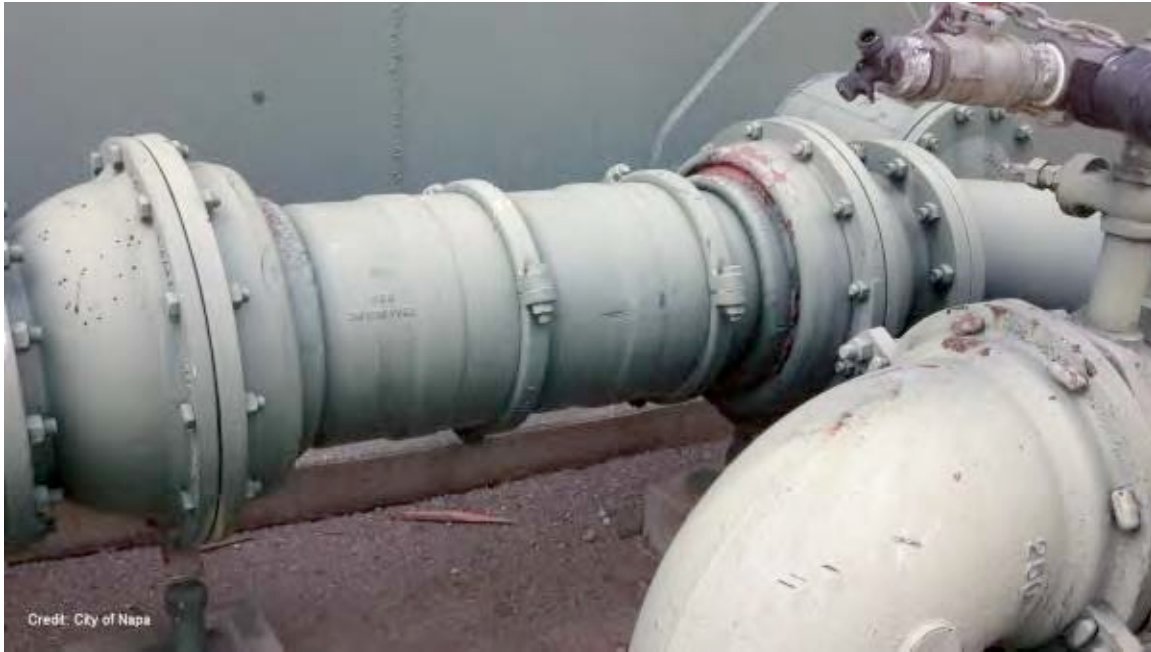
Figure 4-10. Movement of Attached Pipes
