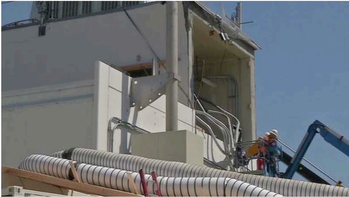
Figure 6-4. Providing External Services to AT&T Building
