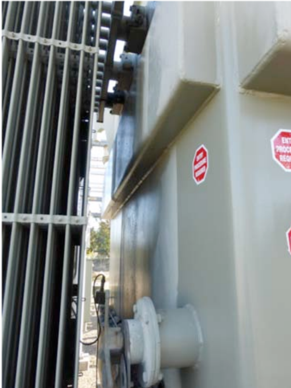
Figure 3-4. Transformer Oil Leak
