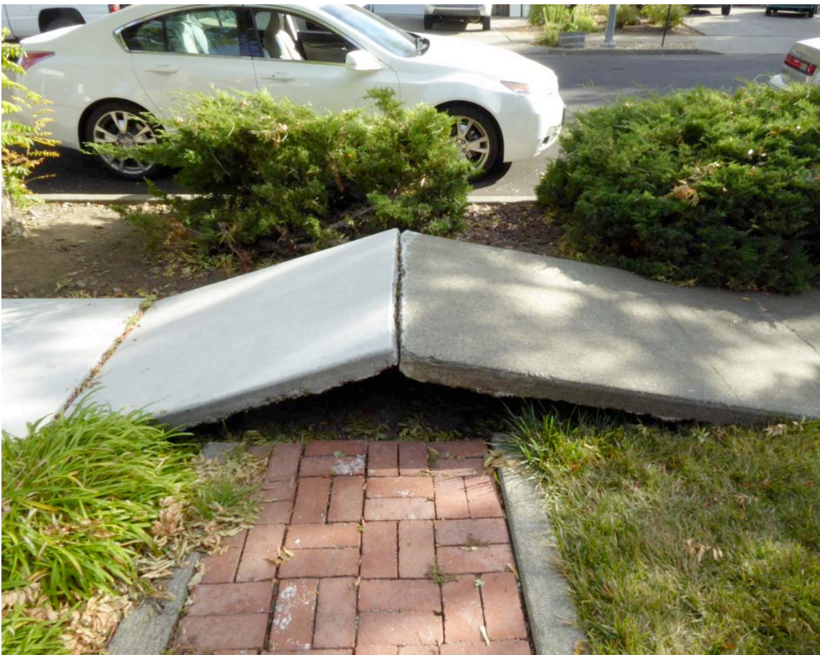
Figure 2-21. Buckled Sidewalk at Fault Offset Location
