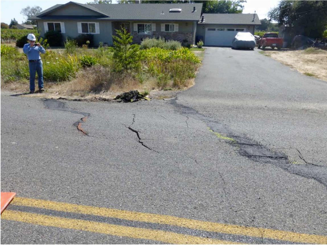
Figure 2-25. Repaired and newly formed cracks in street
