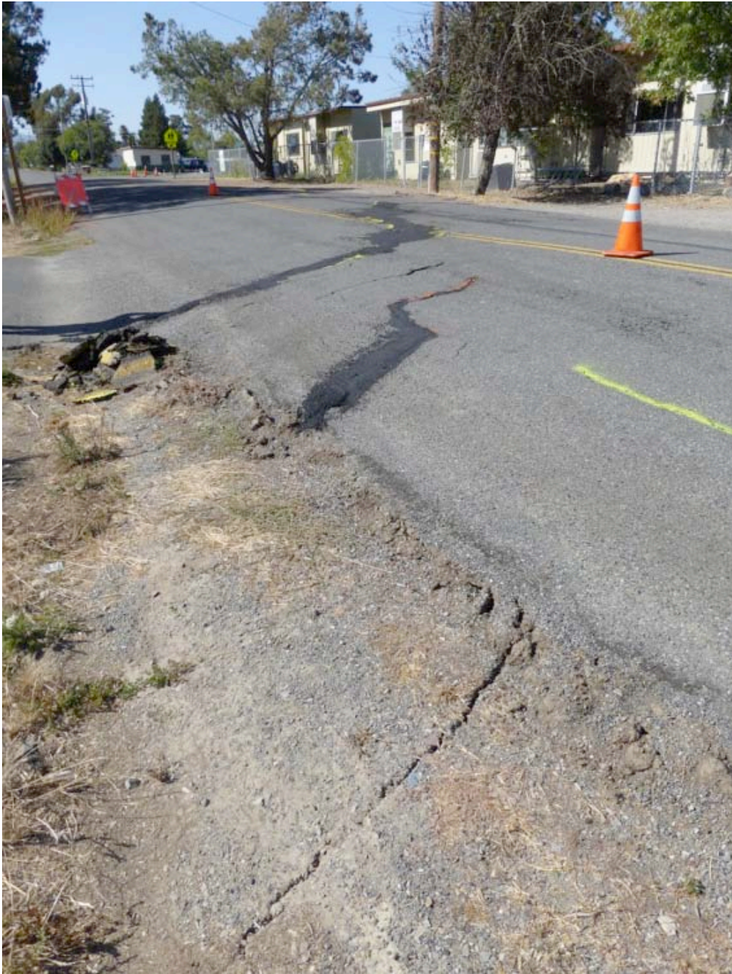
Figure 2-26. Road cracks (repaired and new), looking northerly
