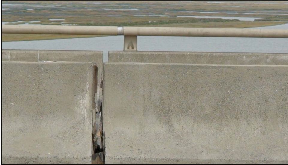
Figure 5-10. Damage to the Napa River Bridge was Permanent Longitudinal Displacement at the Expansion Joints
