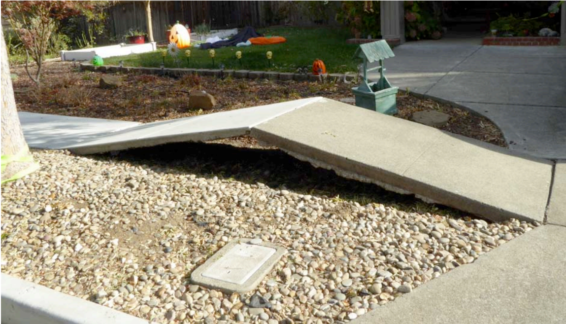
Figure 2-20. Buckled Sidewalk at Fault Offset Location
