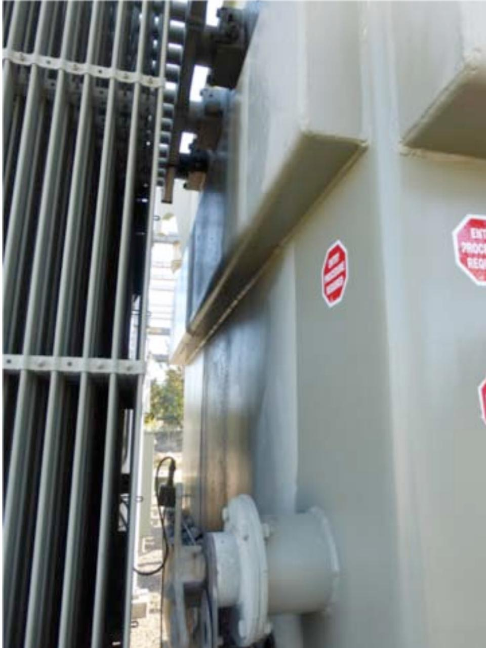
*Figure 3-4. Transformer Oil Leak*
