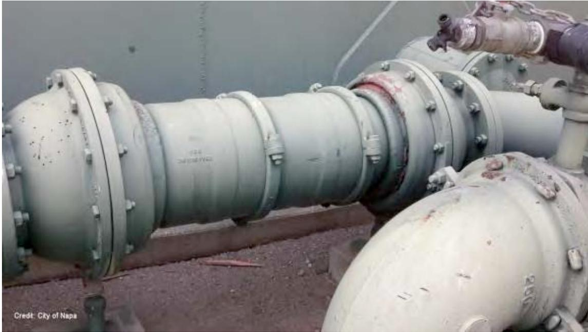
*Figure 4-10. Movement of Attached Pipes*
