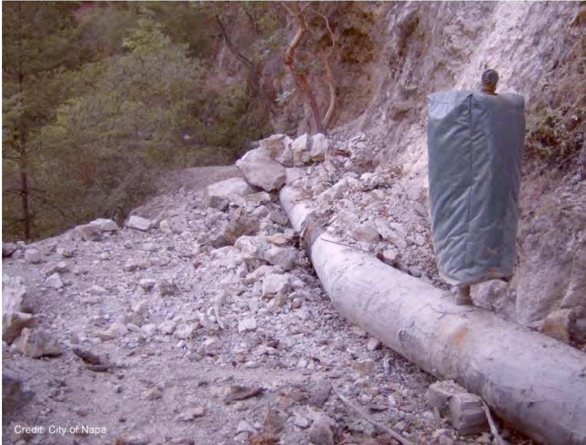
*Figure 4-6. Damaged Transmission Pipe due to Rockfall*
