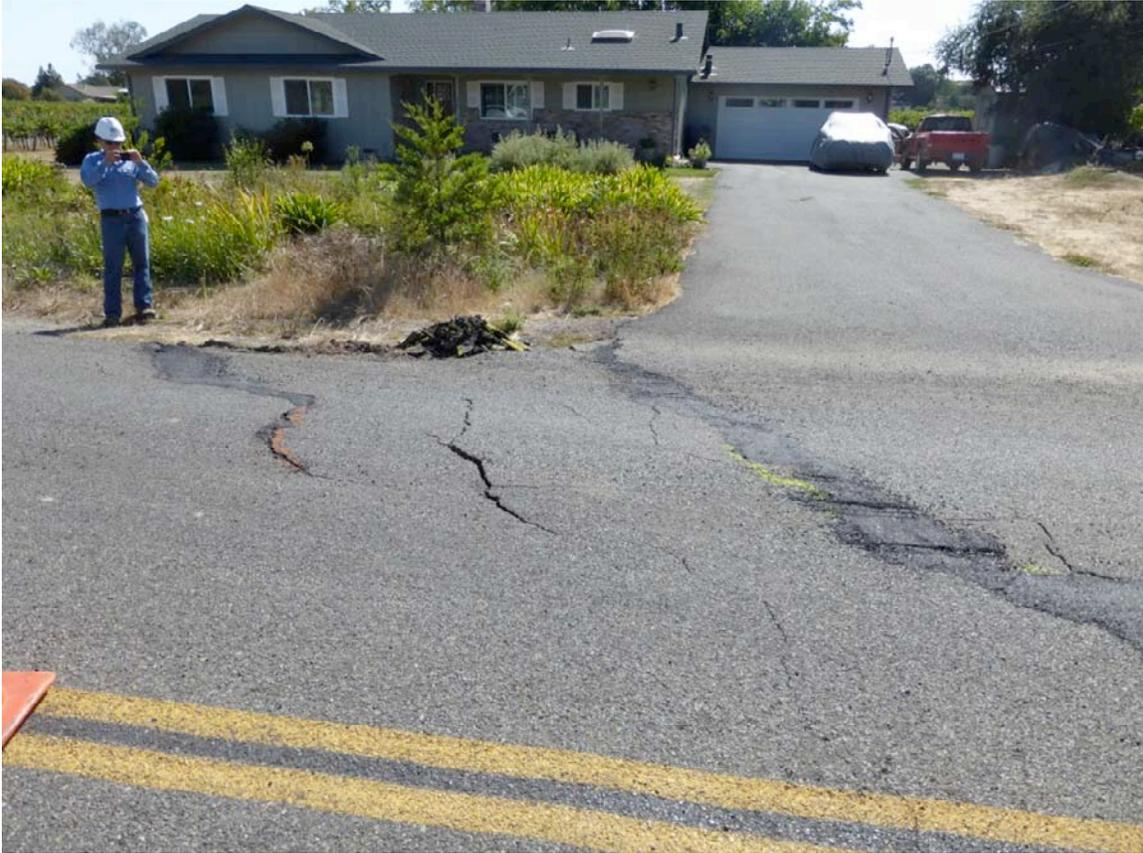
*Figure 2-25. Repaired and newly formed cracks in street*
