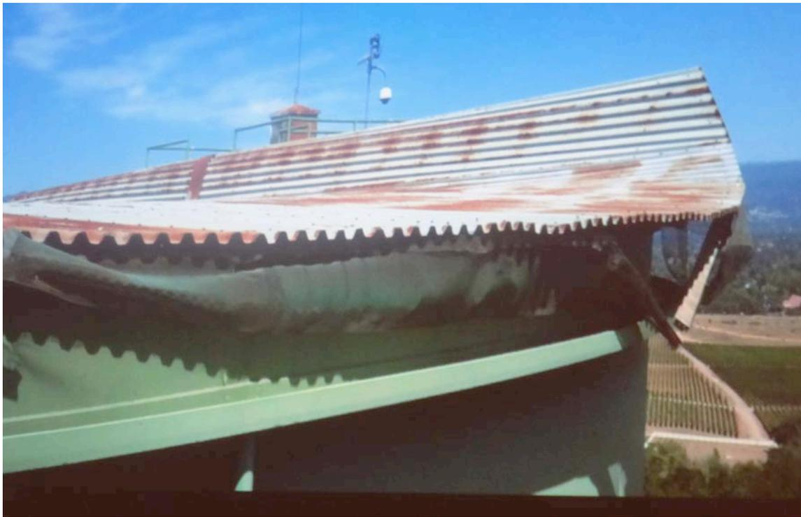
*Figure 4-9. Damaged Roof of Steel Tank "B"*
