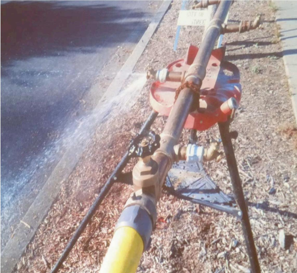
*Figure 4-15. Hose Bib Used During Recovery*
