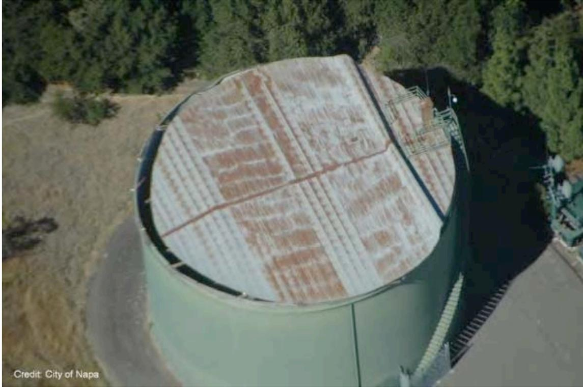
*Figure 4-8. Damaged Roof of Steel Tank "B"*
