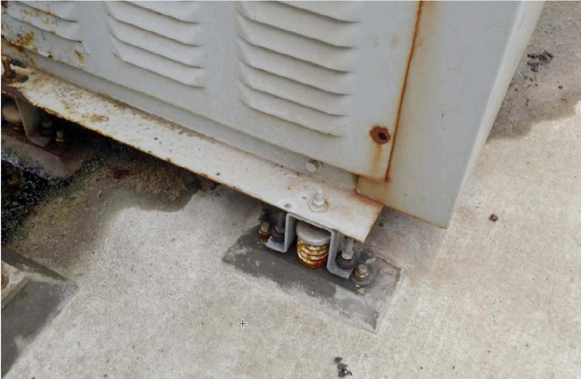
*Figure 4-21. Spring-Mounted Motor Assembly*
