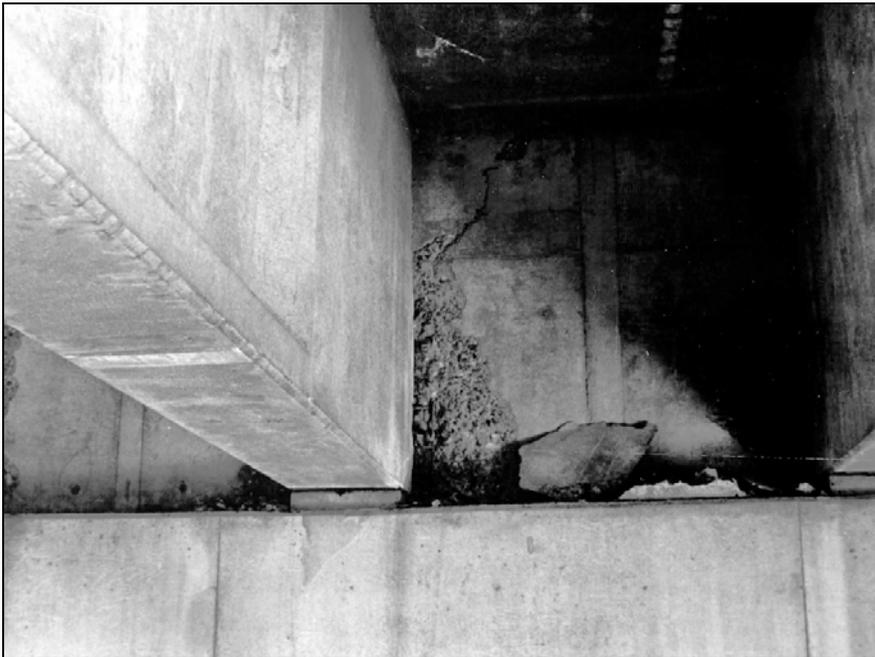
*Figure 5-5. Damage to Napa River Bridge during the Loma Prieta 1989 Earthquake*
