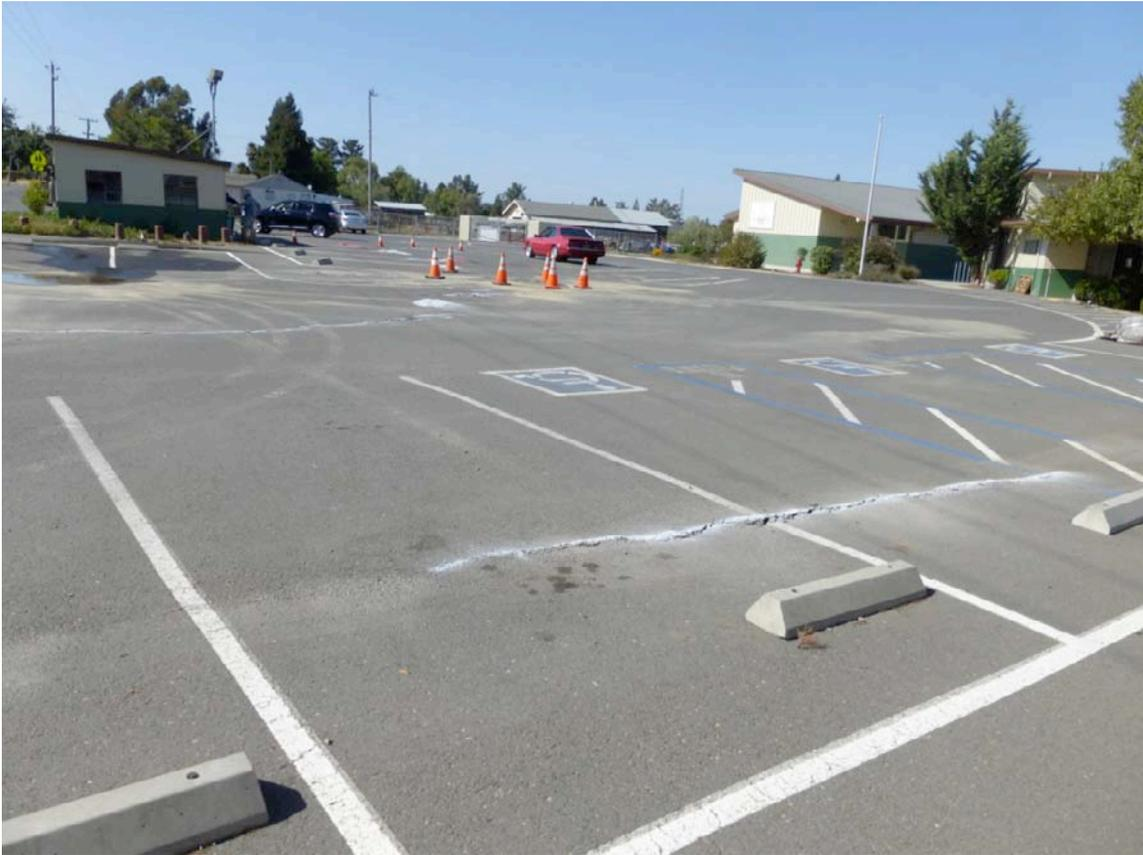
*Figure 2-27. Parking lot cracks, looking northerly*
