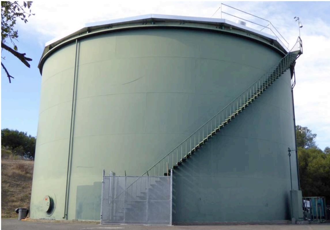
*Figure 4-11. Tank B, with New Aluminum Dome Roof*
