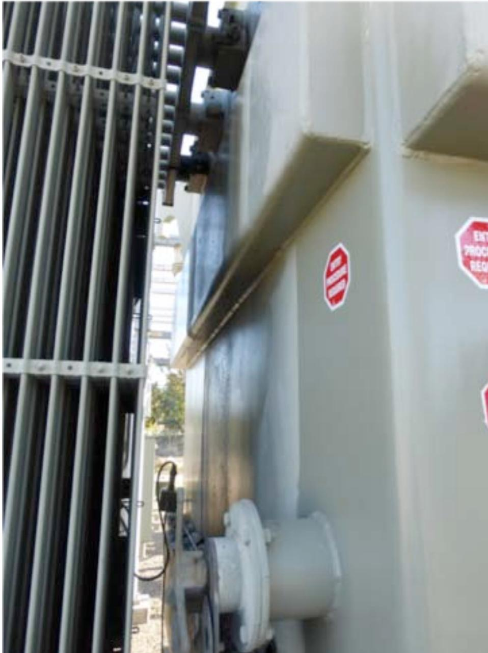
*Figure 3-4. Transformer Oil Leak*
