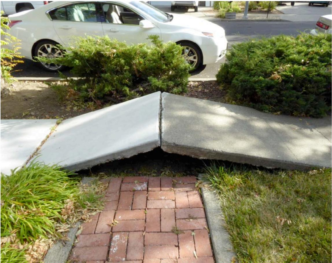
*Figure 2-21. Buckled Sidewalk at Fault Offset Location*
