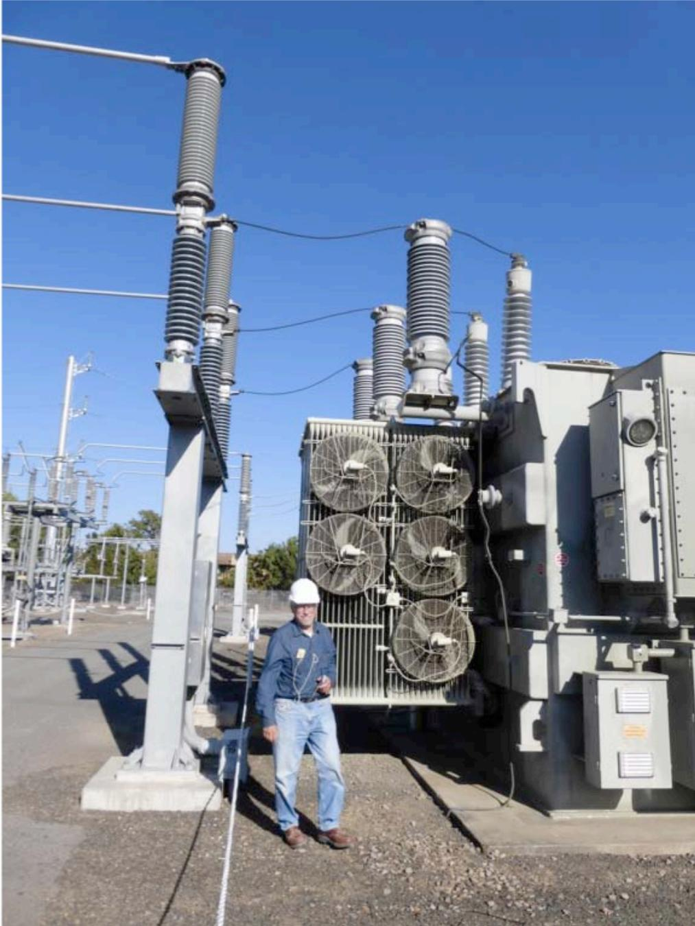
*Figure 3-2. Power Transformer*
