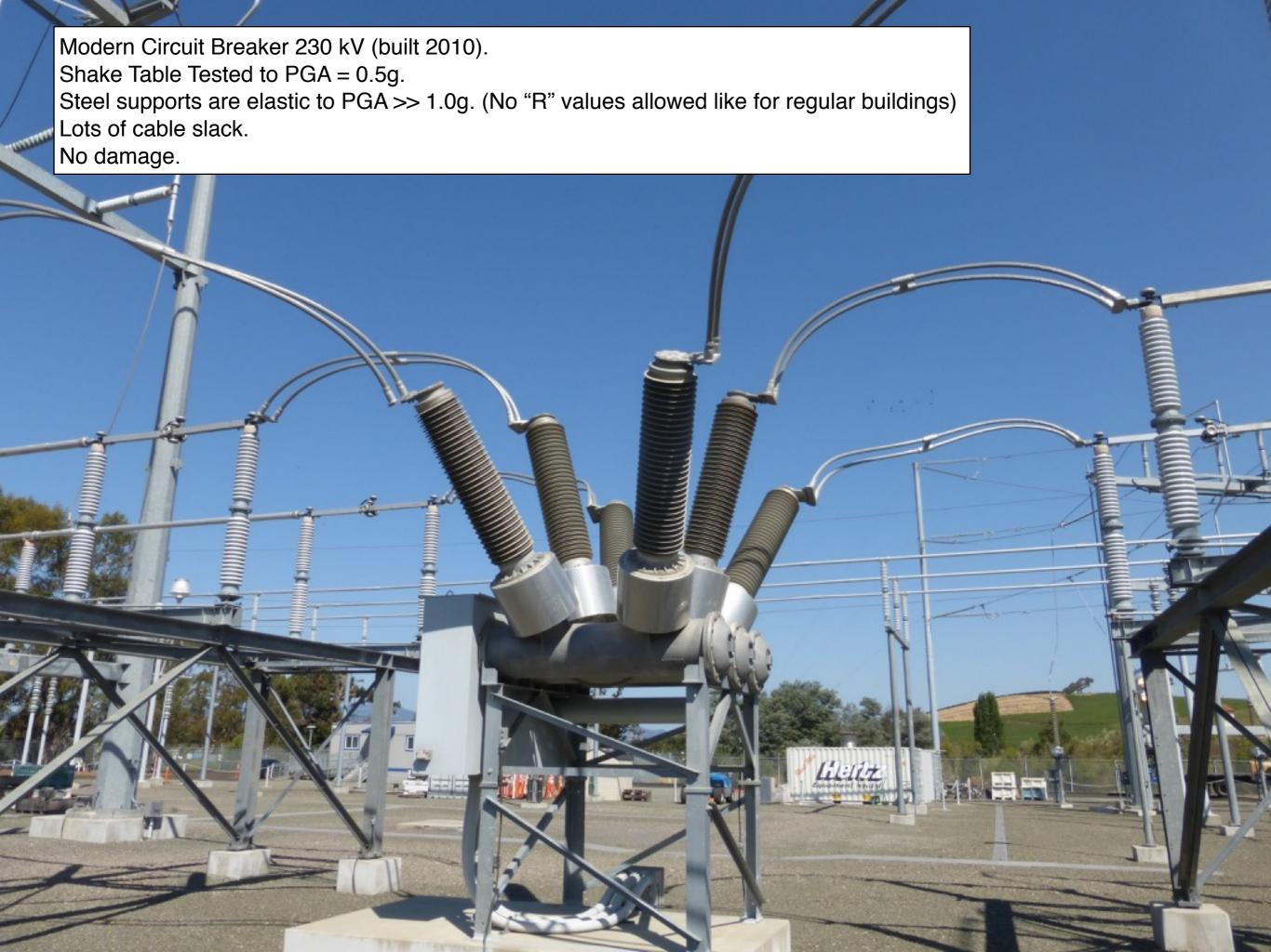
230 kV Horizontal Break switch atop heavily braced frame.
