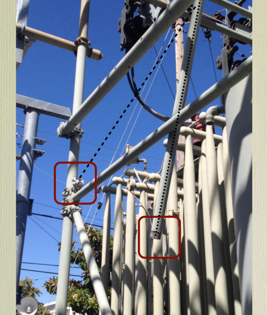
12 kV Circuit Breaker and switches some settlement
