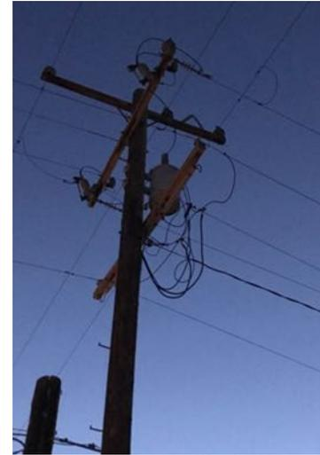
Secondary neutral wrapped around an energized phase leading to burn down.
