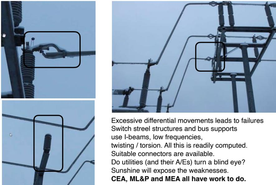
Excessive differential movements leads to failures
