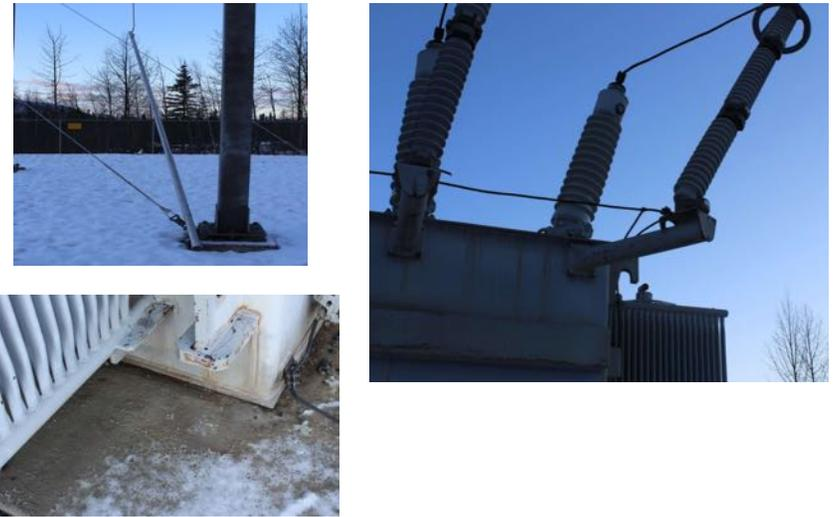
Rigid Bus. Surge Arrestors. Transformer slid, breaking 2 bushings. + 2 SAs.
