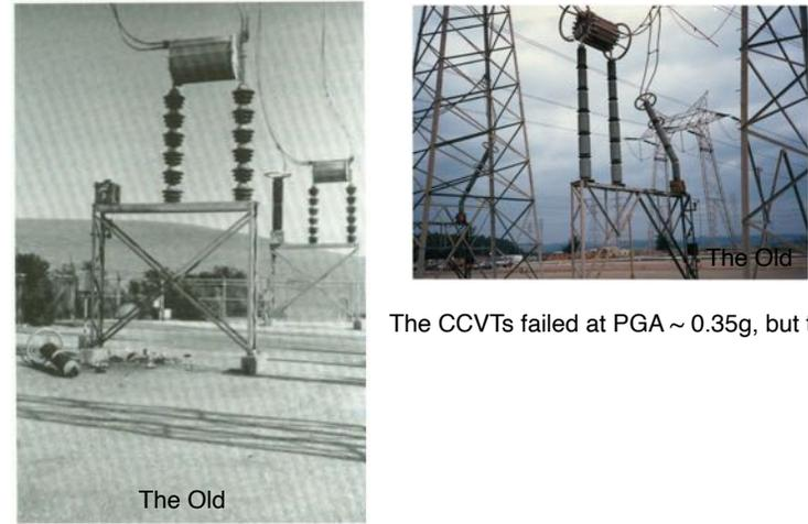
The CCVTs failed at PGA ~ 0.35g, but the WTs did not
