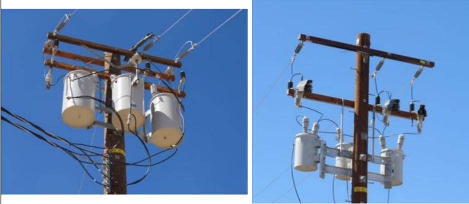
3 Transformer Frames: High W, Low Frequency, High Wire “snapping” forces, High Torsion = high displacement demand on drop wires
