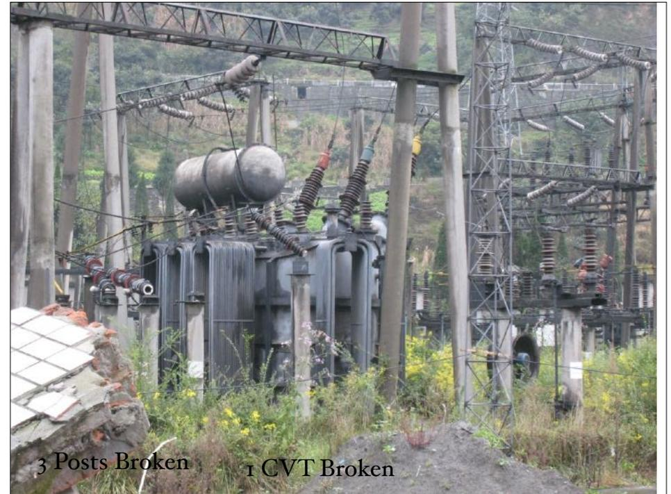
3 Posts Broken      1 CVT Broken
