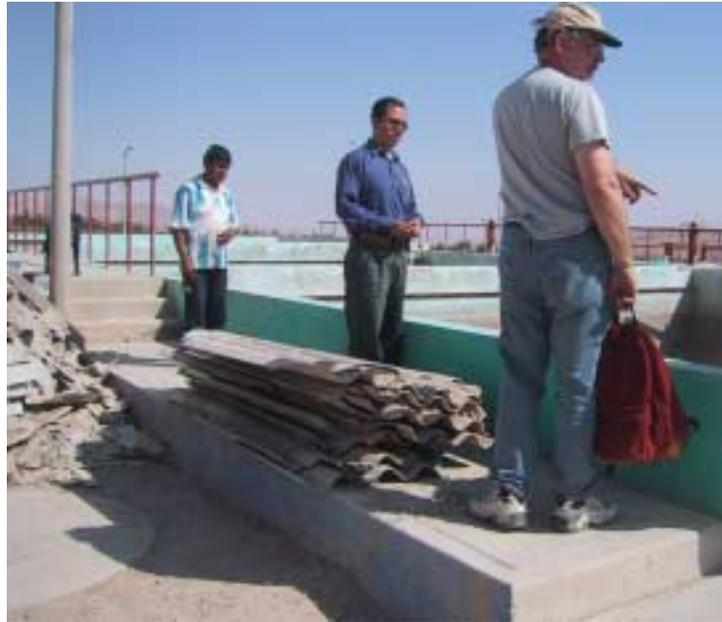
*Figure 4-12. Broken Baffles, Moquegua WTP*
