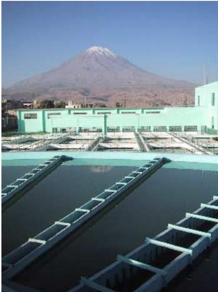
*Figure 4-5. Metal Troughs – Out of Alignment (El Misti in background)*
