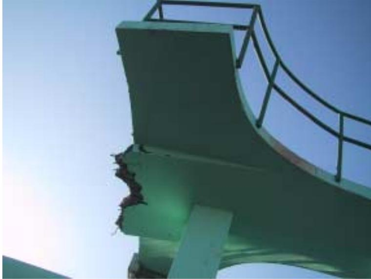
*Figure 4-8. Damage to Reinforced Concrete Walkway*
