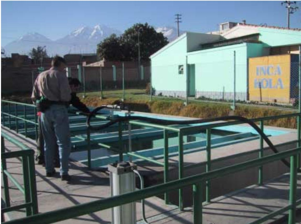
*Figure 4-2. Arequipa WTP. No damage to concrete troughs, no sloshing over freeboard*
