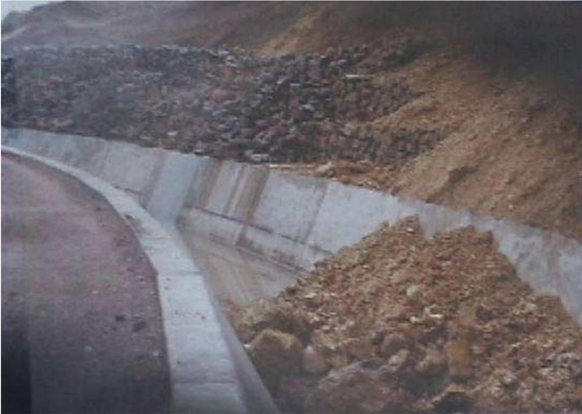
*Figure 5-4. Landslide Debris into Canal Near Moquegua*
