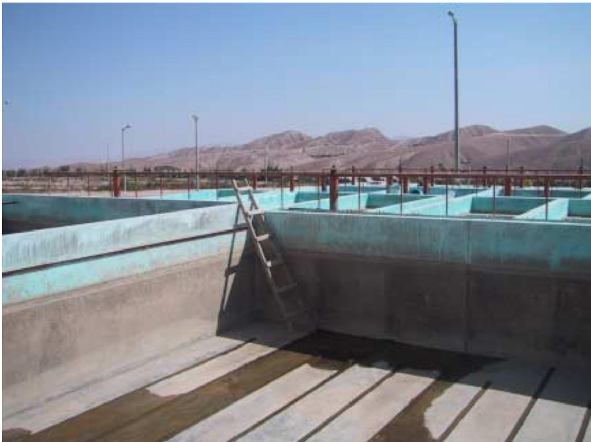
*Figure 4-11. Primary Flocculation Basin, Moquegua WTP*
