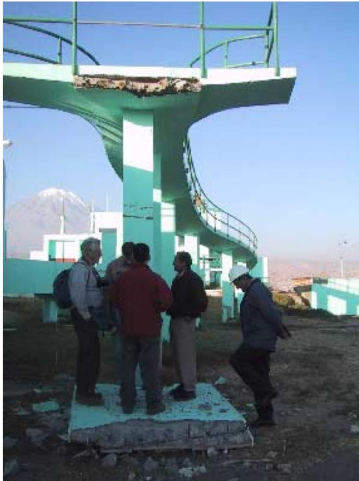
*Figure 4-9. Damage to Reinforced Concrete Walkway*
