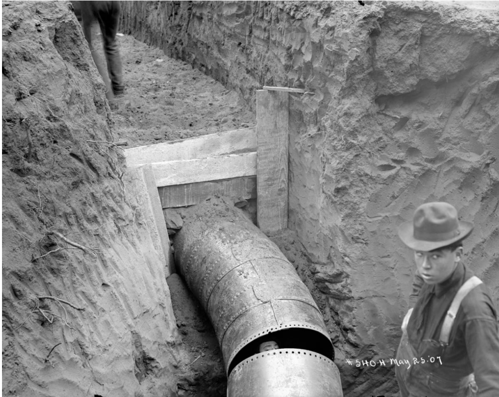
Figure 4. Installation of Wrought Iron Riveted Pipe, 1907
