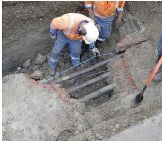
**Figure 11. Exposing the Damaged XLPE-Type Cables, Location 6**
