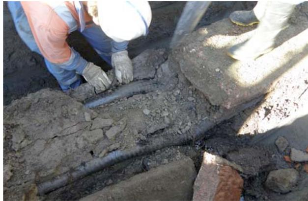
**Figure 6. Exposing the Damaged Oil-Type Cables, Location 1**
