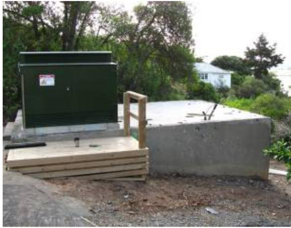
**Figure 19.** Slab mounted transformer installed on the slab where St. Andrews URM substation building used to stand before it was damaged by the February 22, 2011 earthquake.
