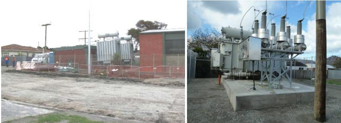
**Figure 17.** Brighton substation. a) Left: Significant settlement and sinking of transformer buildings. b) Right: Circuit breaker and transformer at the end of the temporary line shown in Fig. 10.
