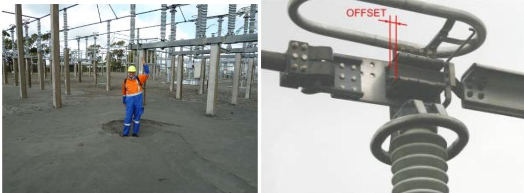
**Figure 8** a) Left: Significant soil liquefaction at Bromley substation. One of the authors is standing inside a sand “volcano.” b) Right: 1 cm offset at a disconnect switch in Bromley substation
