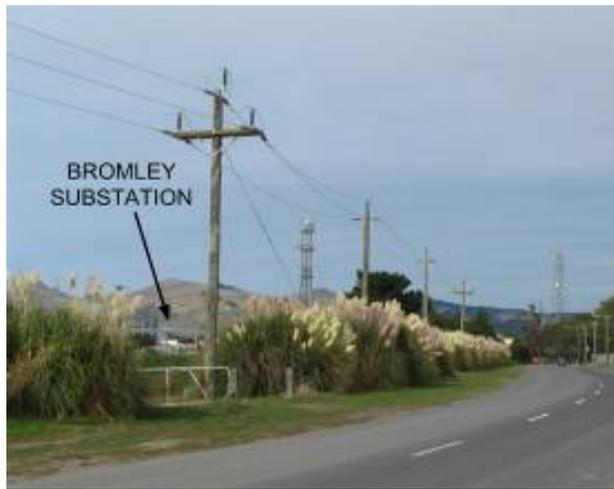
**Figure 10.** The temporary 66 kV line installed from Bromley substation to restore service in the Brighton-Dallington area.
