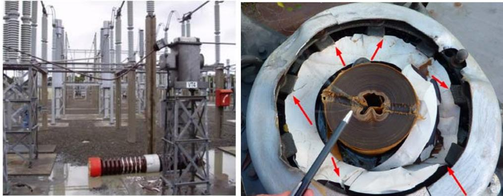
**Figure 7** Broken 220 kV CVT insulator mounting showing finger clamps. The arrows in the photo on the right indicates fatigue induced cracks initiated in the porcelain edges in contact with the corner of the finger clamps. (photos: Transpower)
