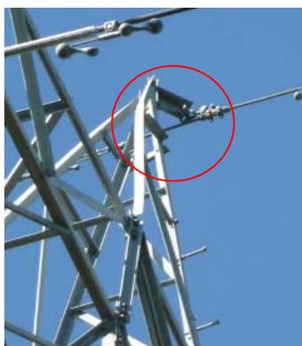
**Figure 3.** Bended steel brace supporting a guard conductor in a lattice tower (photo: Transpower).
