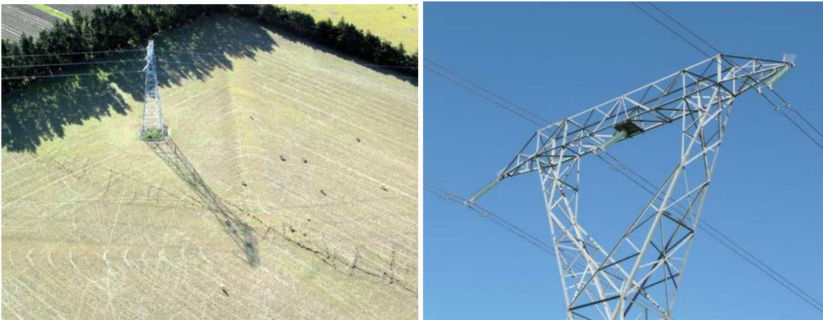
**Figure 2.** a) Left: Surface fault near a steel lattice tower of the ROX-ISL-A line. b) Right: Displaced insulators on a steel lattice tower as a result of the surface fault offset (photos: Transpower).
