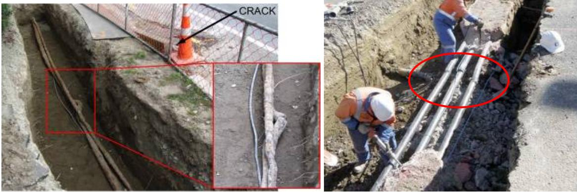
**Figure 13.** a) Left: An apparent crack induced fault in a 11 kV underground cable. b) Right: 66 kV underground line along Armagh street damaged by soil liquefaction (Photo: Orion).
