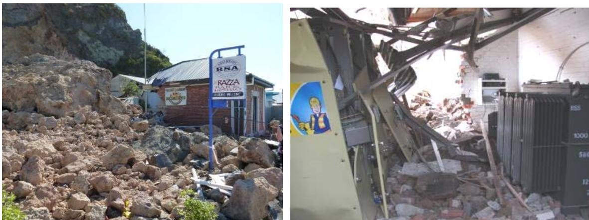
**Figure 18.** Damaged substation building by rock fall in Sumner. a) Left: Exterior. b) Right: Interior.
