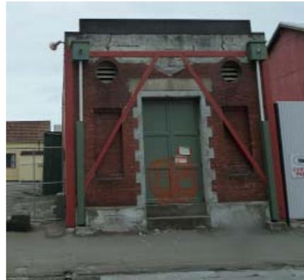
**Figure 20.** Two examples of seismically reinforced URM substations good performance. Notice the damage in the home next to the substation shown in the photo on the left.
