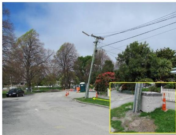
**Figure 5.** Tilted pole for 400 V power distribution being supported by a concrete block. Poles are shared with communications service providers.
