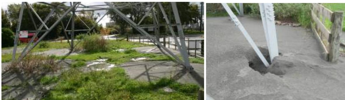
**Figure 9.** Examples of soil liquefaction at the base of steel lattice towers.
