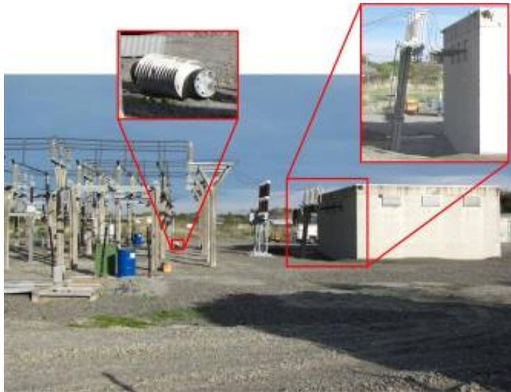
**Figure 16.** Damage from soil liquefaction at Pages substation. The details show a damaged bushing (left) and tilted supporting structure at the conductors entrance to the transformer building (right) which had experienced a small settlement.
