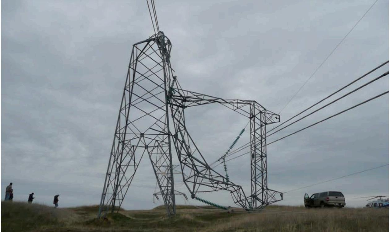
*Figure 2. Collapsed 500 kV Transmission Tower due to High Wind, 2010*
