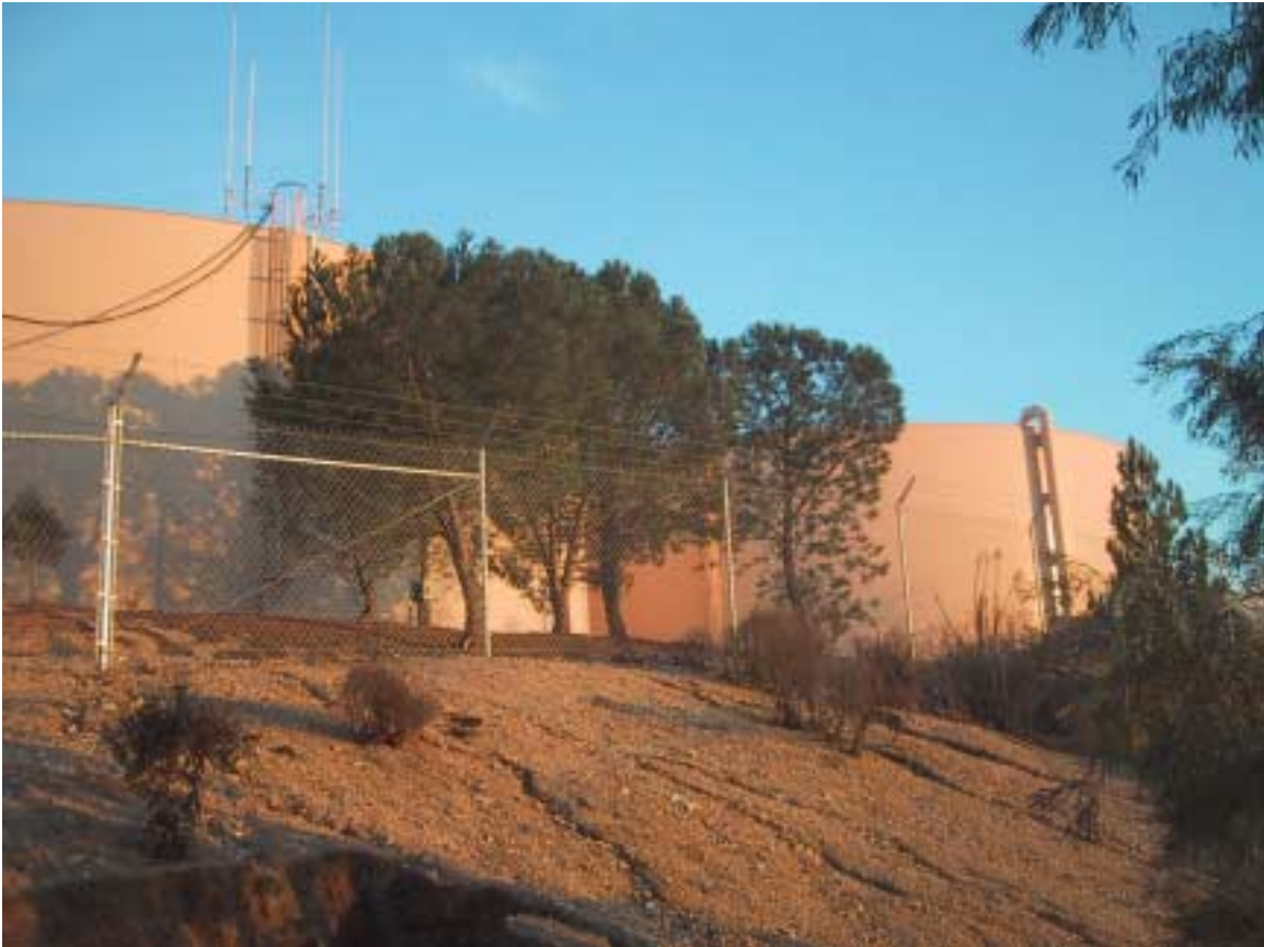
Figure 1. Paso Robles Golden Hill Tanks (North Tank on left)
