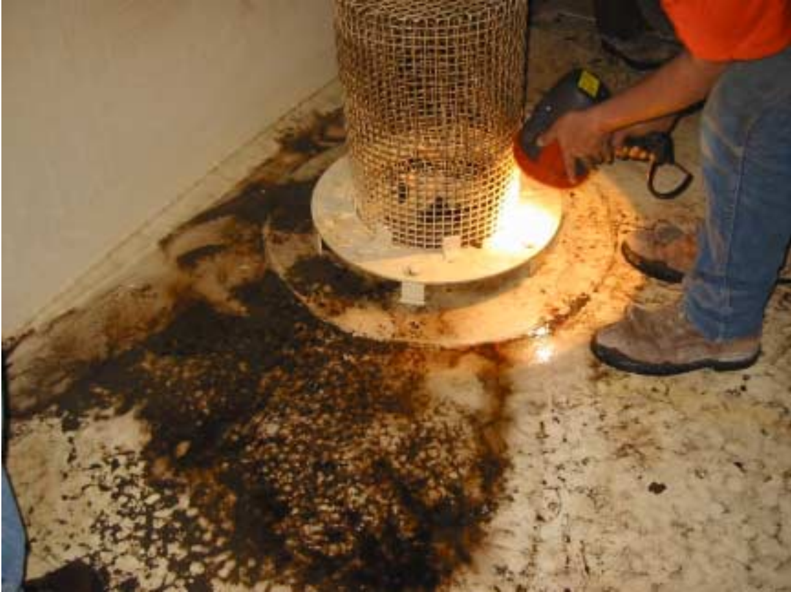
Figure 4. North Tank, Outlet Near Tank Wall
