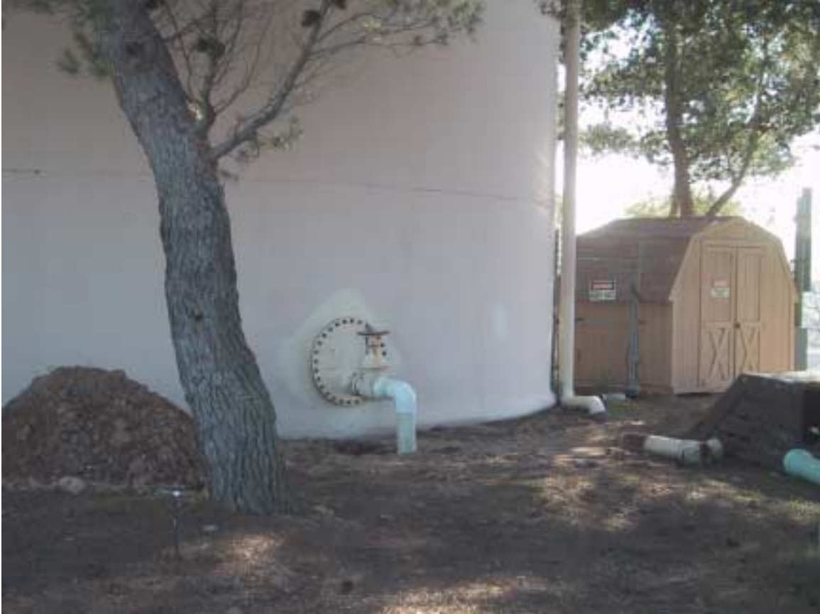
Figure 8. Tank with Elephant Foot Buckle
