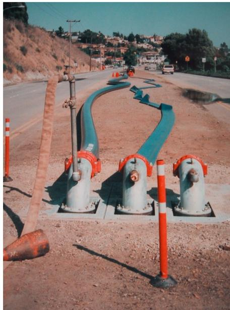
Figure 3. Flex Hose Attached to Manifold Outlets
