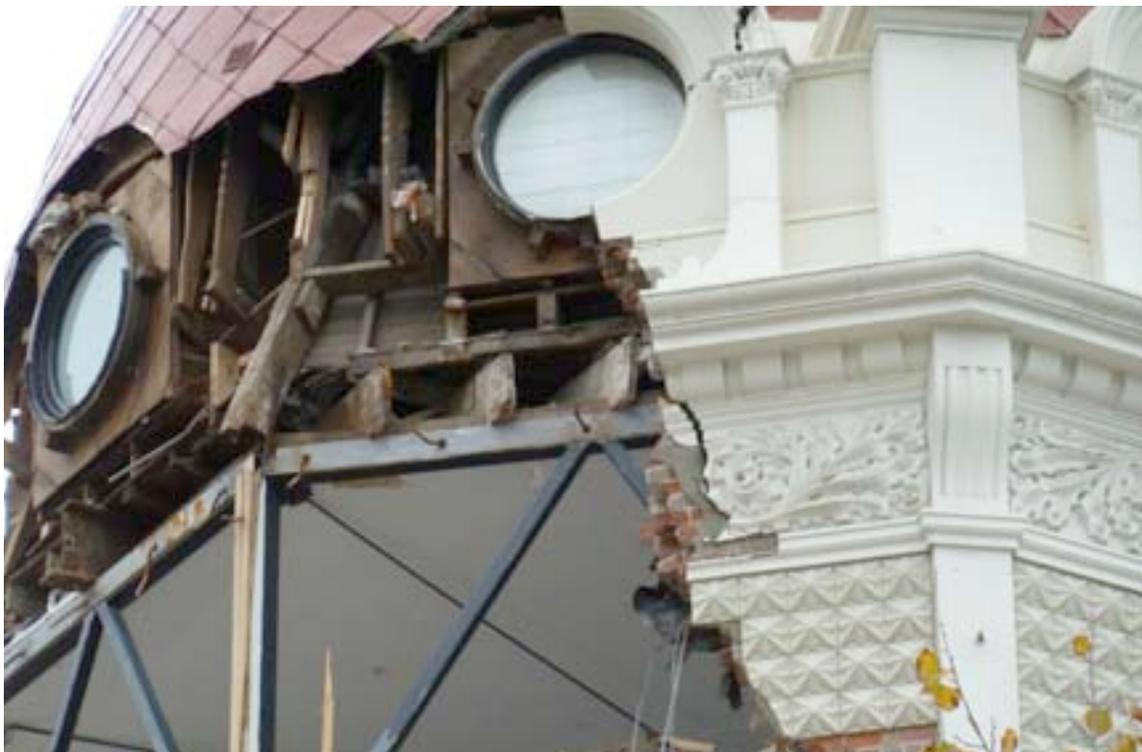
*Figure 16-24. Interior Steel Frame of Damaged Tourism Building, February 2011*
