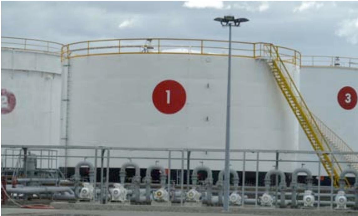
*Figure 8-2. Undamaged Steel Tanks at Woolston*
