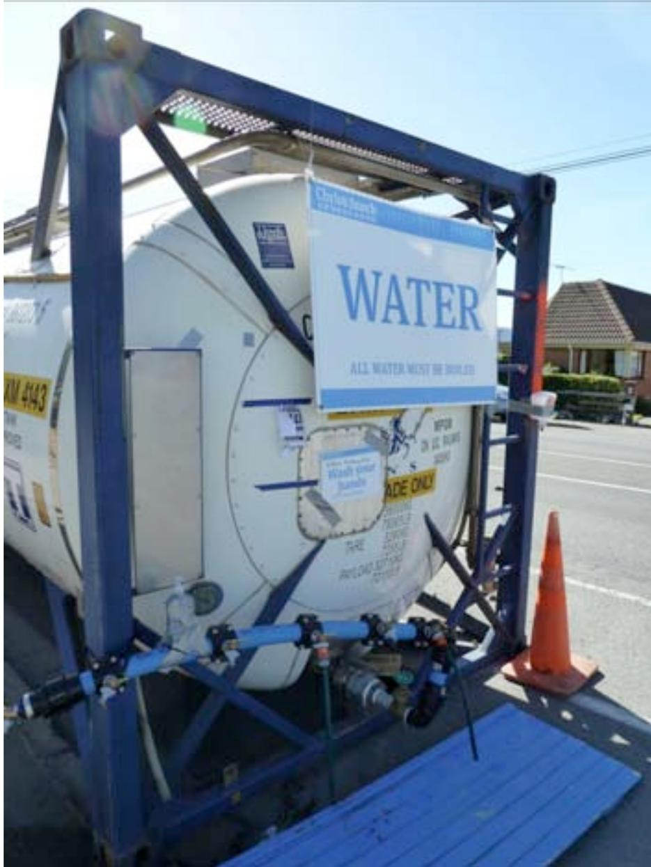
*Figure 6-37. Deployed Water Tank and Hose Bib Manifold*
