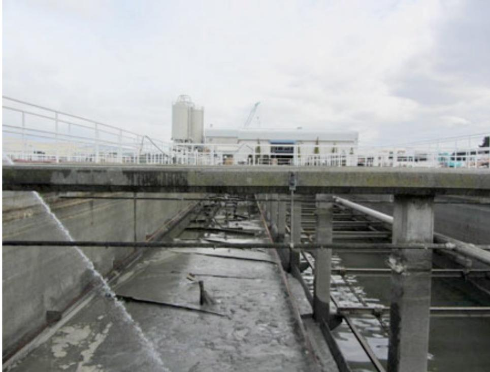
*Figure 7-45. Primary Settling Basins Cleaning, Bromley WWTP*
