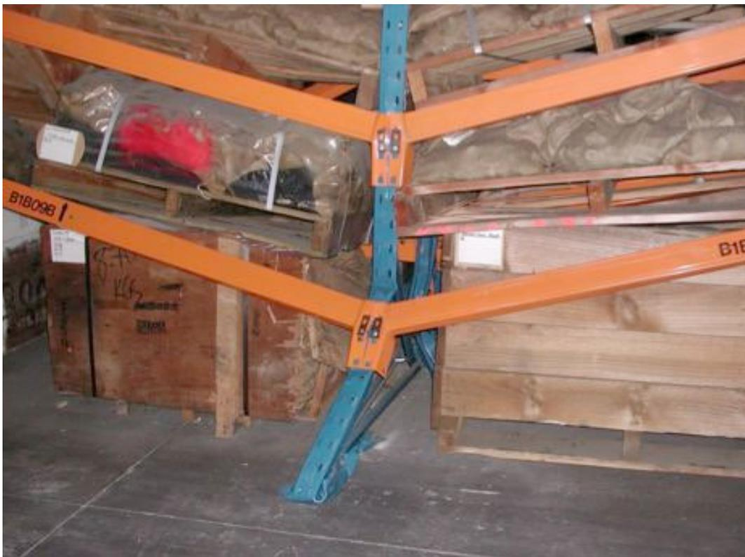
*Figure 17-3. Damaged Column Leg, Addington Warehouse*
