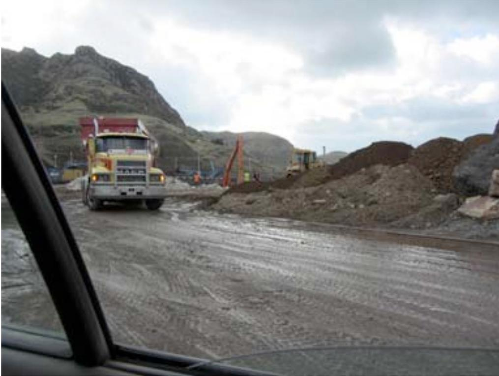
*Figure 9-27. Processing and placement of rubble for the Te Awaparahi Bay reclamation.*
