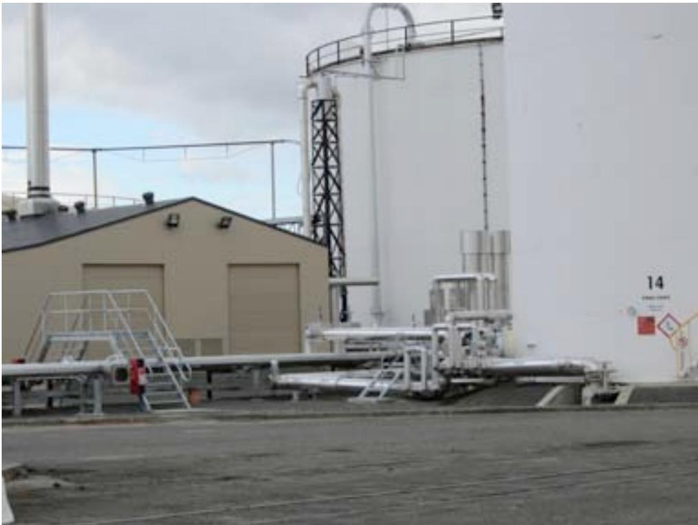
*Figure 9-36. Pipe connections to tank at the Lyttelton Port oil berth tank farm.*
