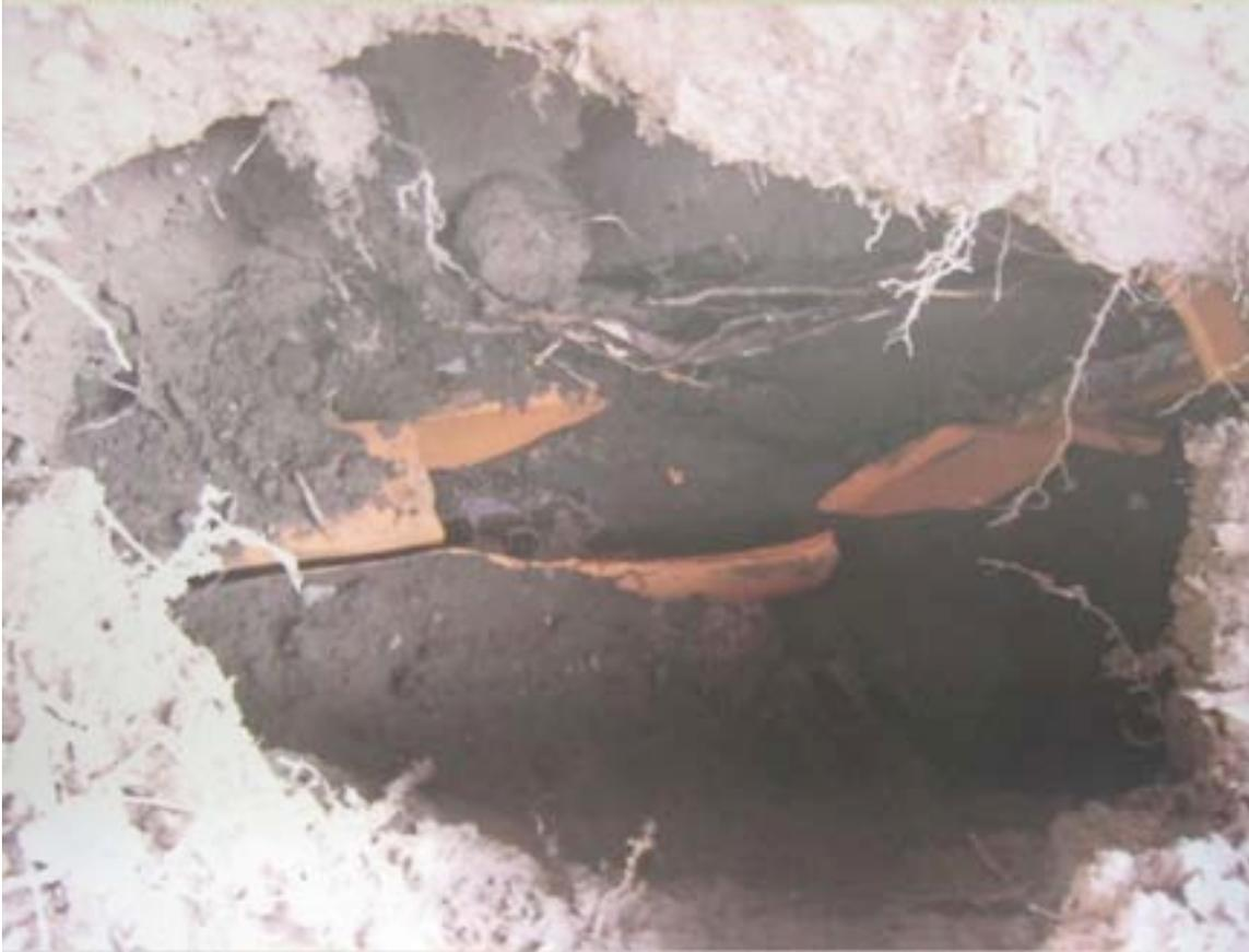
*Figure 7-17. Repair of Vitrified Clay Sewer Pipe*
