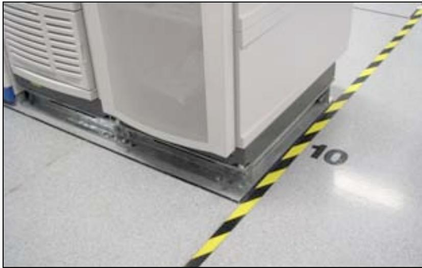
*Figure 5-10. Equipment anchoring, Vodafone.*
