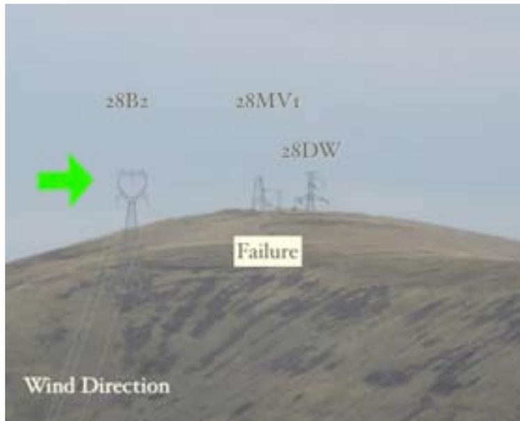
*Figure 6. Case Study 2. Collapsed Tower 14179 Due to Wind Load*
