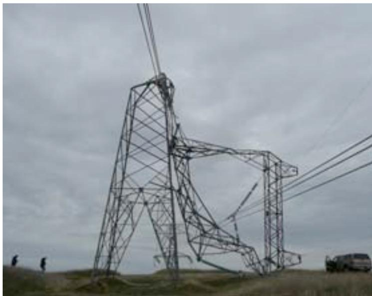
*Figure 7. Case Study 2. Collapsed Tower Due to Wind Load*
