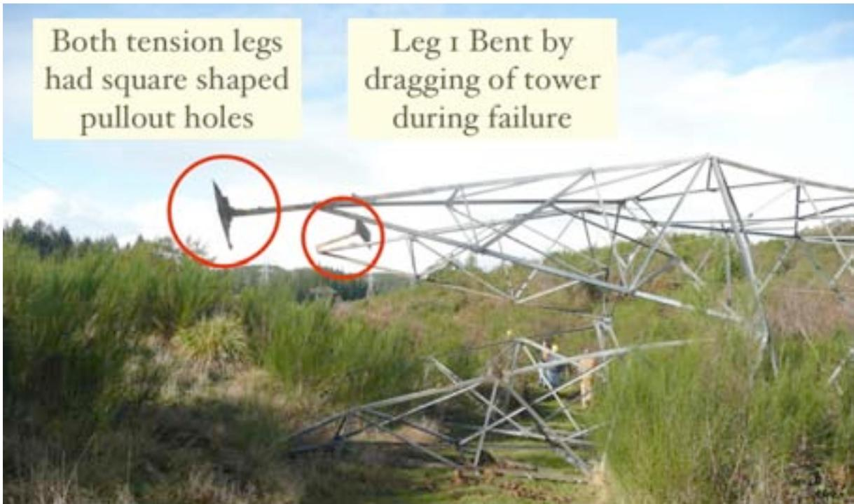
Figure 4. Case Study 1 Collapsed Tower Due to Wind Load
