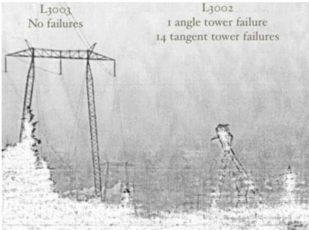
*Figure 8. Case Study 3. Collapsed Tower Due to Ice Load*
